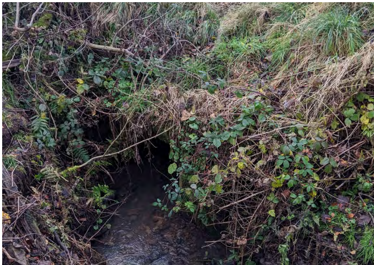
Photo 6 – Unnamed watercourse passing beneath the Edinburgh - Glasgow railway line through a box culvert
