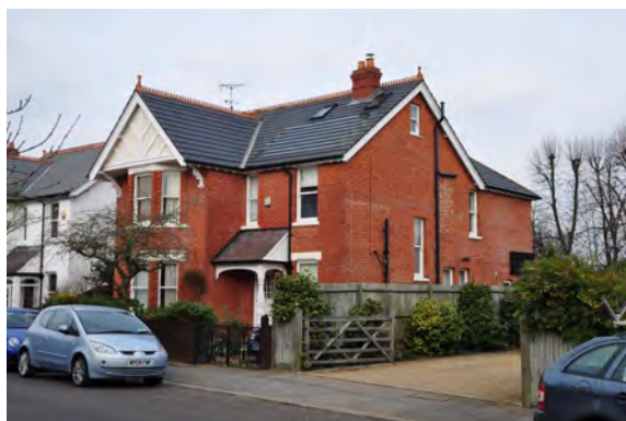
Solar panels on traditional roofslope
