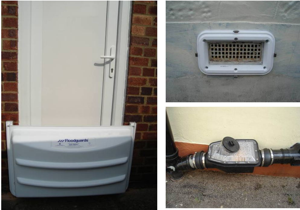
Figure 5-2 Examples of flood barriers, air bricks and non-return valves
