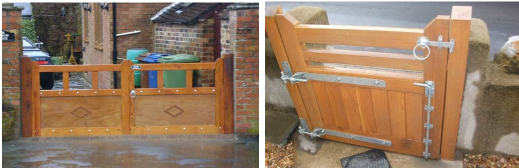
Figure 5-3 Example of flood gates
