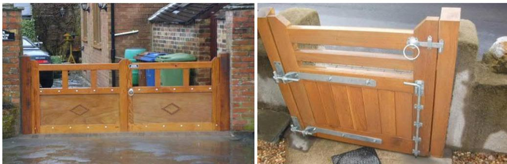
Figure 5-3 Example of flood gates
