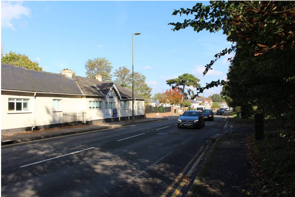
Image EDP 10: View of the cast iron listed customs post (to left) within its setting looking north-east along Portsmouth Road.
