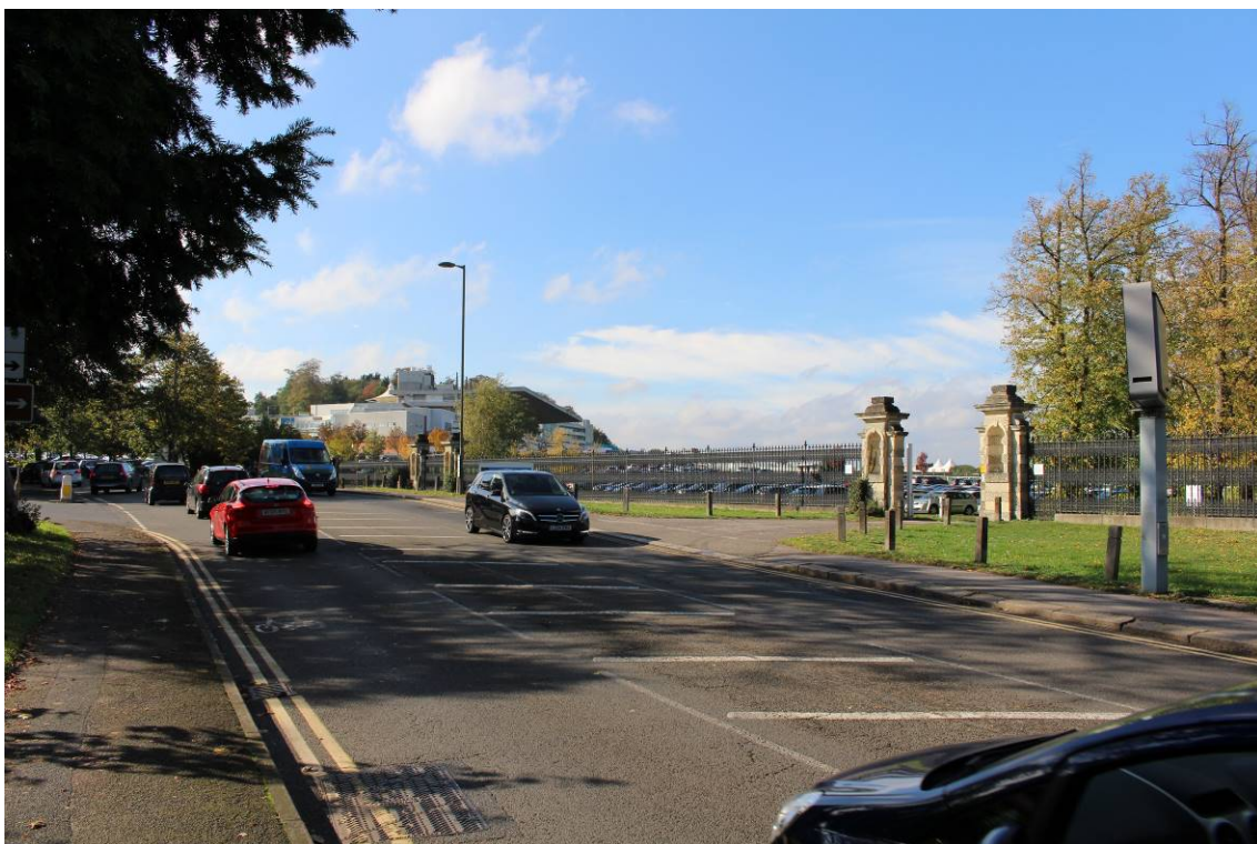
Image EDP 2: Gates and Railings to Sandown Park Racecourse listed as Grade II, looking west, showing the context of the railings in relation to the grandstand and racecourse beyond.
