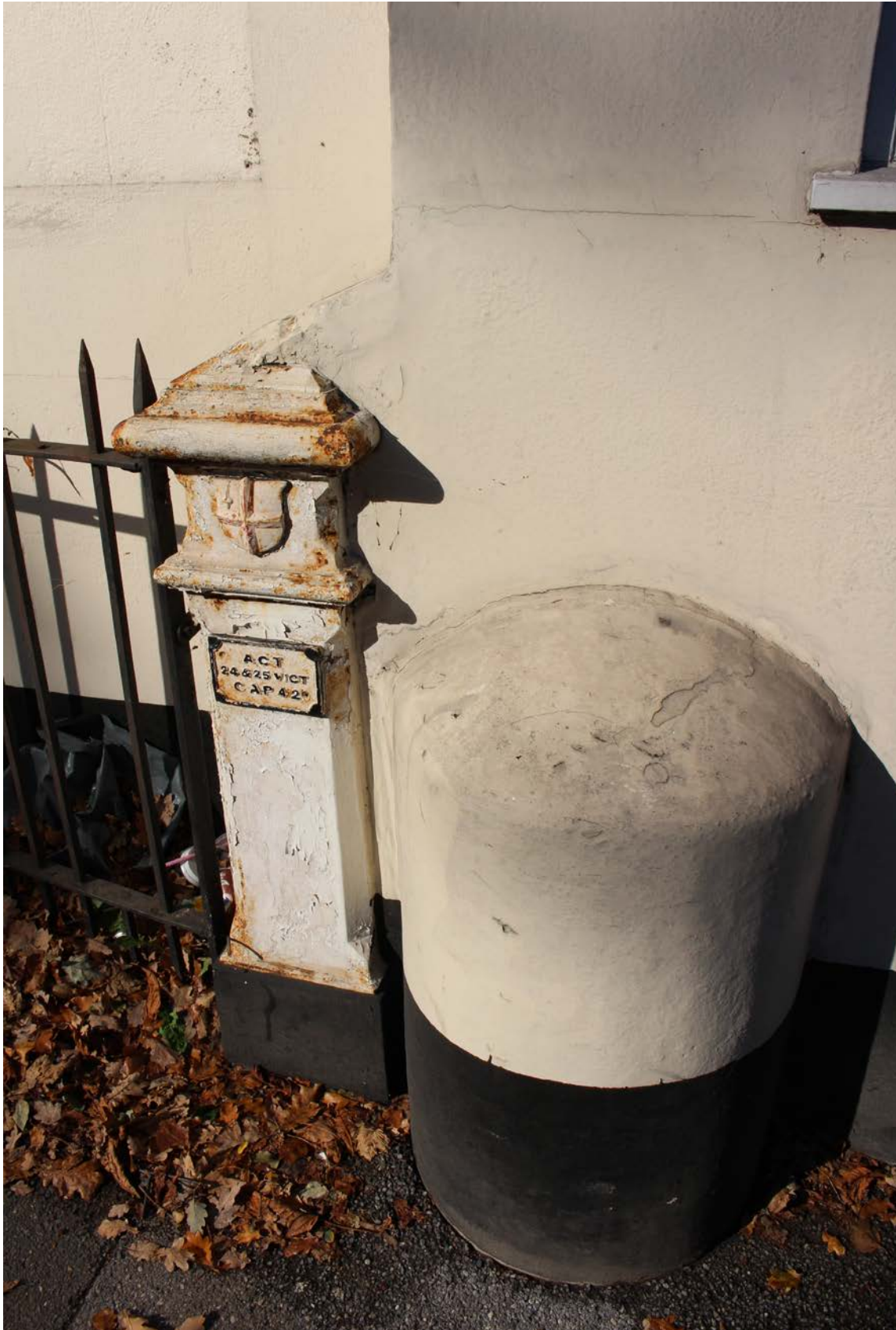
Image EDP 9: View of the cast iron listed customs post (to left) with unknown, non-designated post to right.
