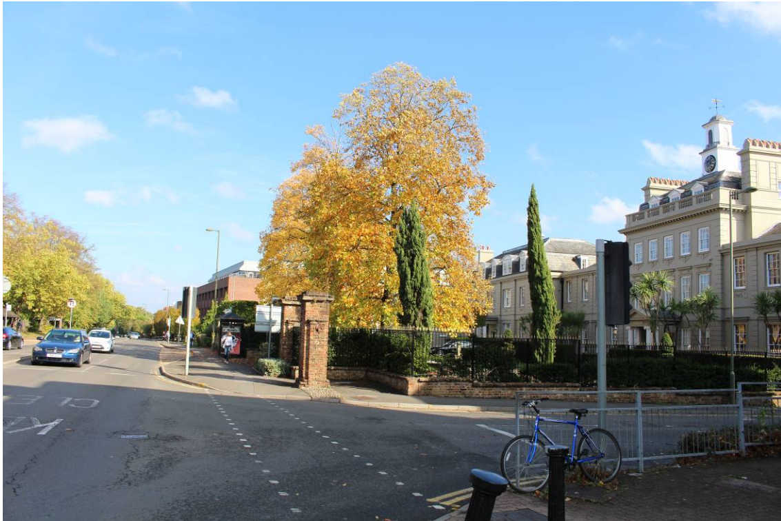
Image EDP 12: View of Sandown House from the west, looking north-east, showing its principal elevation and relationship to the Portsmouth Road. Also note the large-scale office building within its setting to the northeast.
