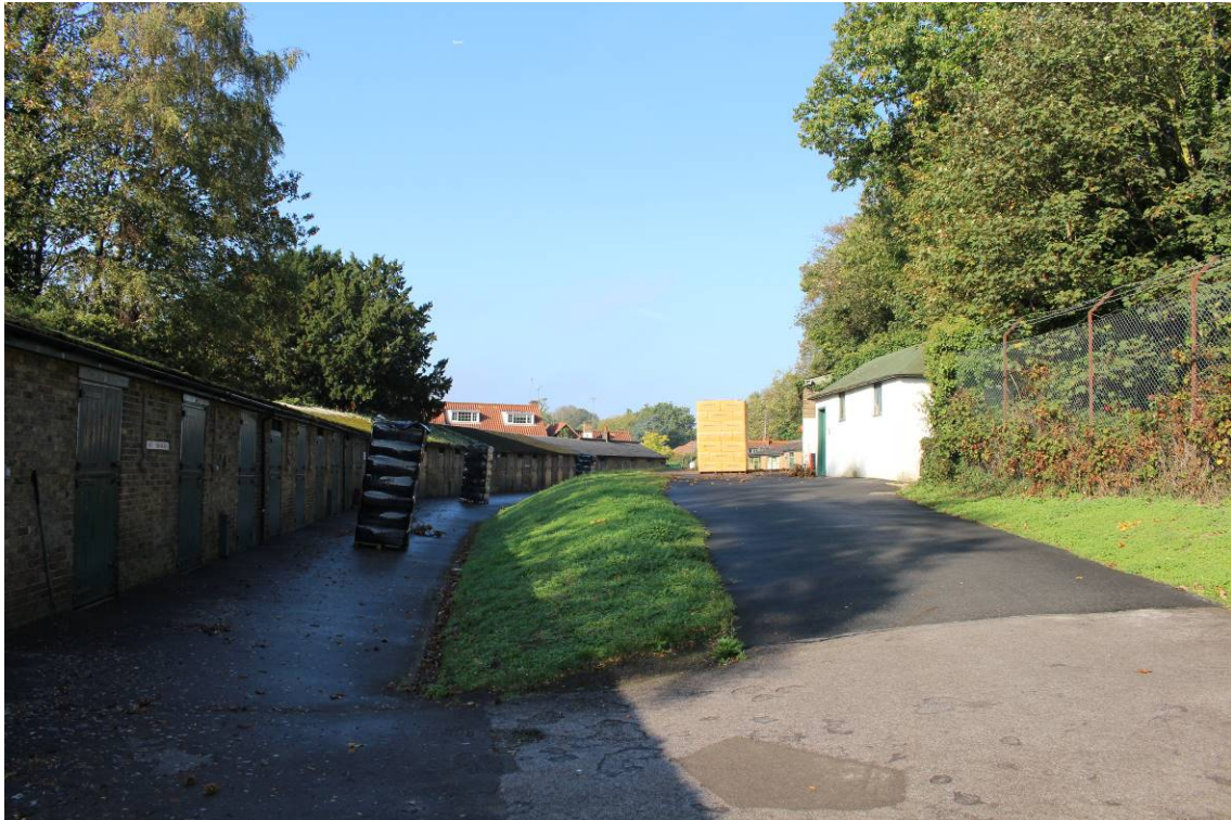
Image EDP 32: View of Site 1 showing the terracing, looking west.
