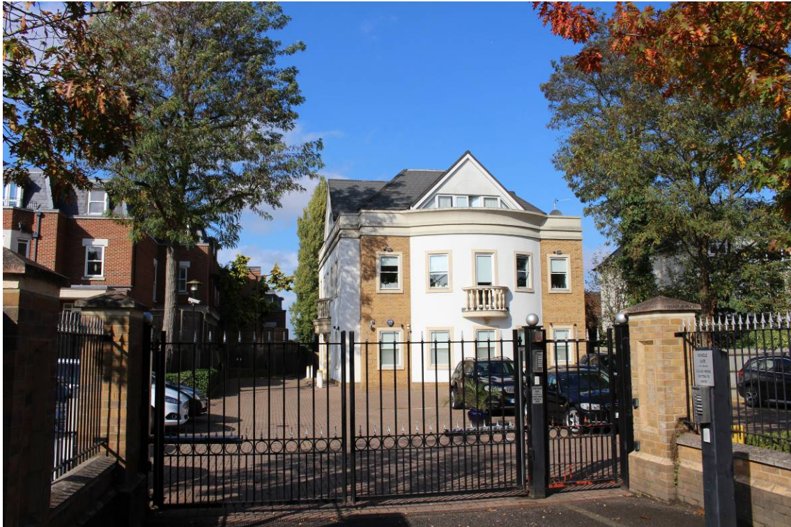
Image EDP 22: View of the setting of Myrtle Cottages further to the west along Myrtle Road, showing the replacement large dwellings of larger scale set further back within their plots.
