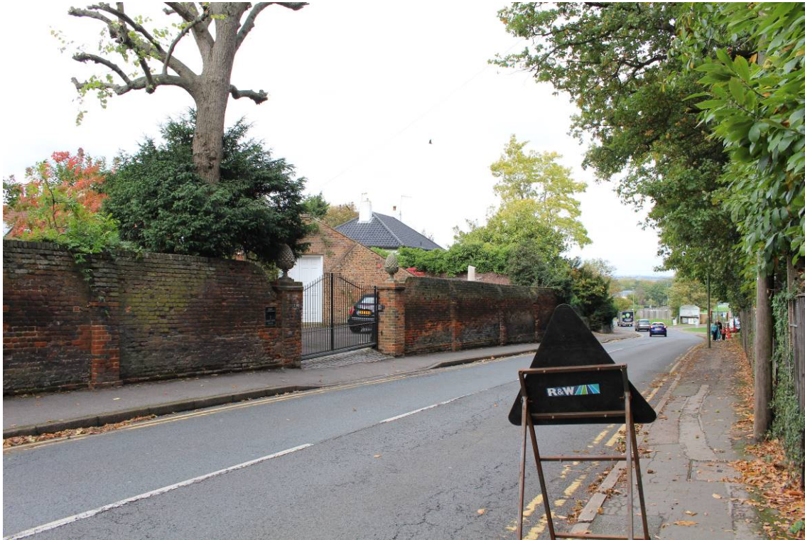
Image EDP 14: View of the Grade II listed walls, looking north-west. They enclose the Grade II listed Orangery and Garden reach cottage with little experience of them from the street.
