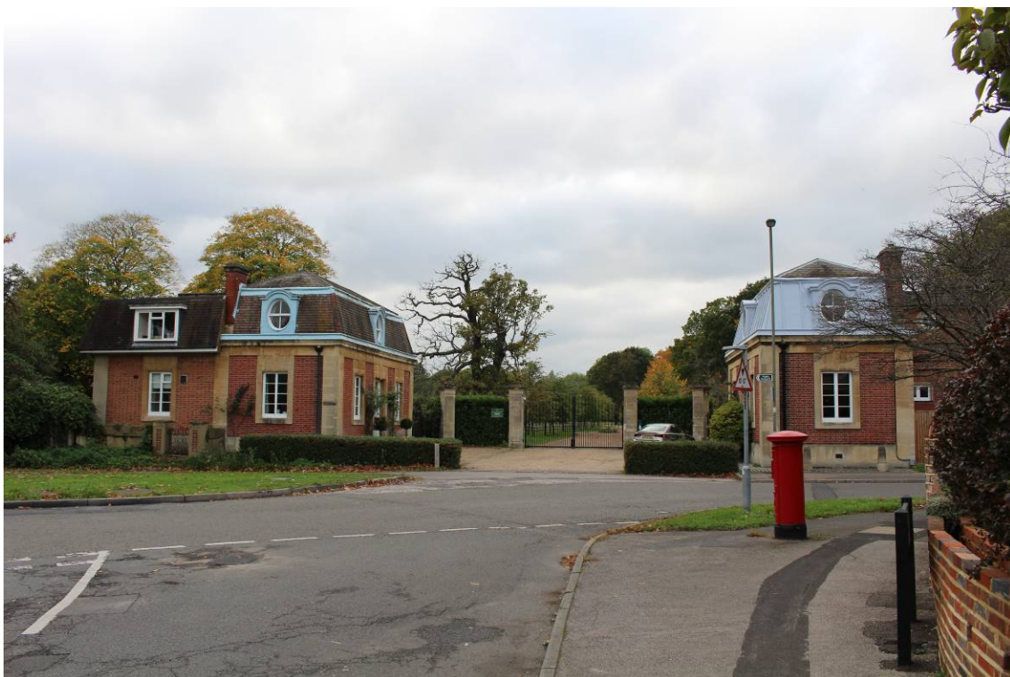
Image EDP 29: View of the locally listed lodges to the north-west of the site. Looking west.
