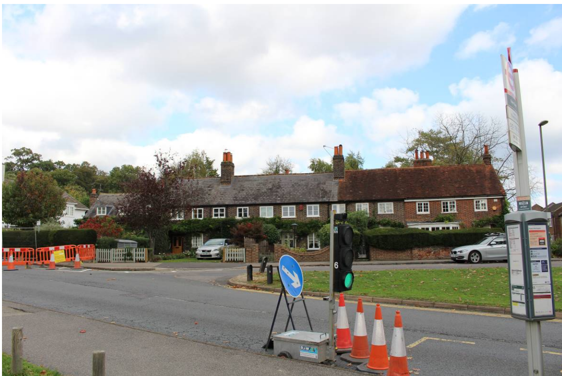
Image EDP 19: The row of Grade II listed cottages listed as Encott, Westeria, The Cottage and Force Cottage, Nos 28 To 34 Esher Green.
