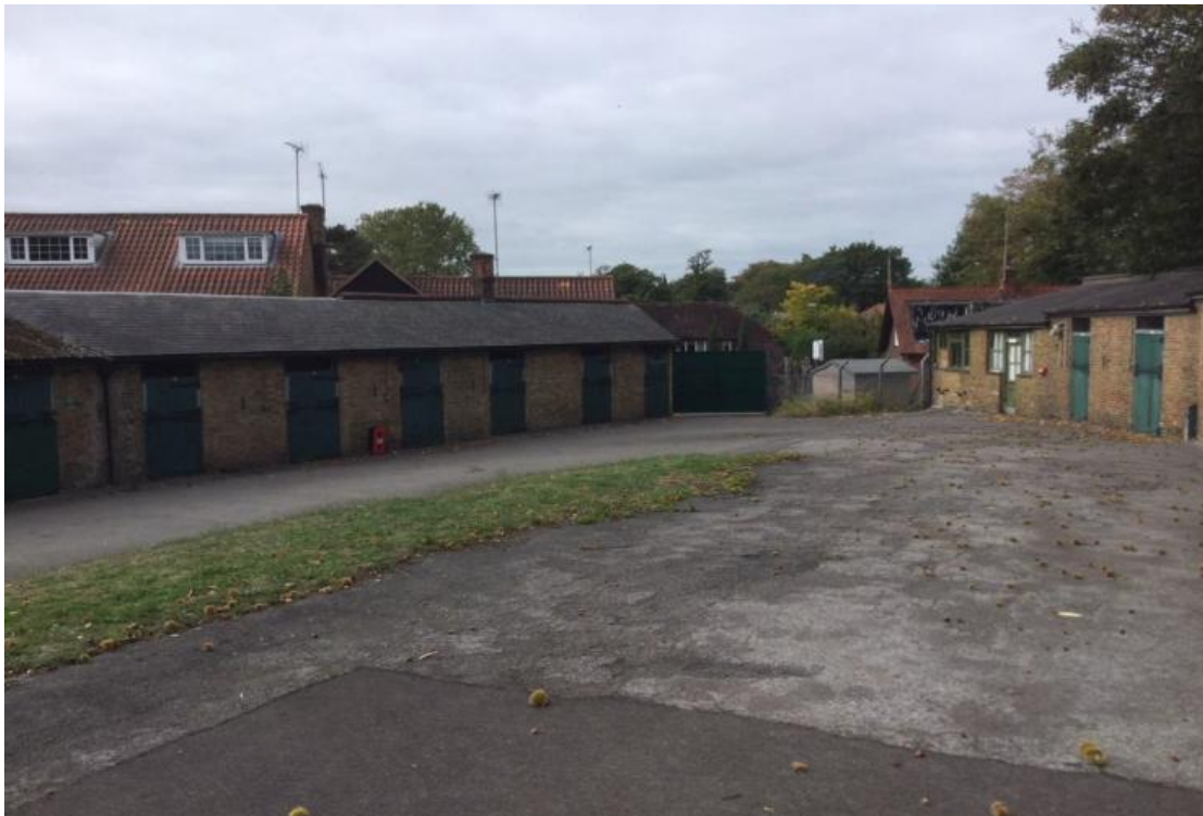
2661/OPA-S1/P2: Site 1 facing southwest towards Moor Lane
