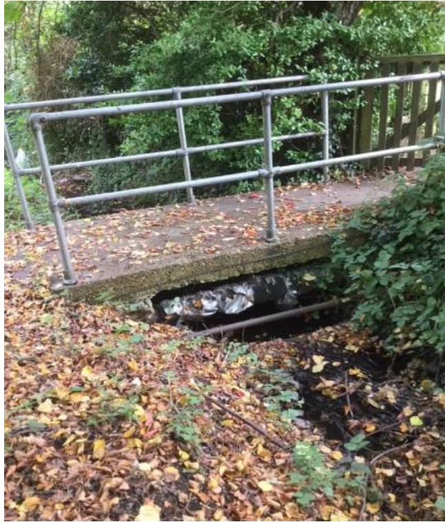
2661/OPA-S3/P5: Example of pipe crossing watercourse
