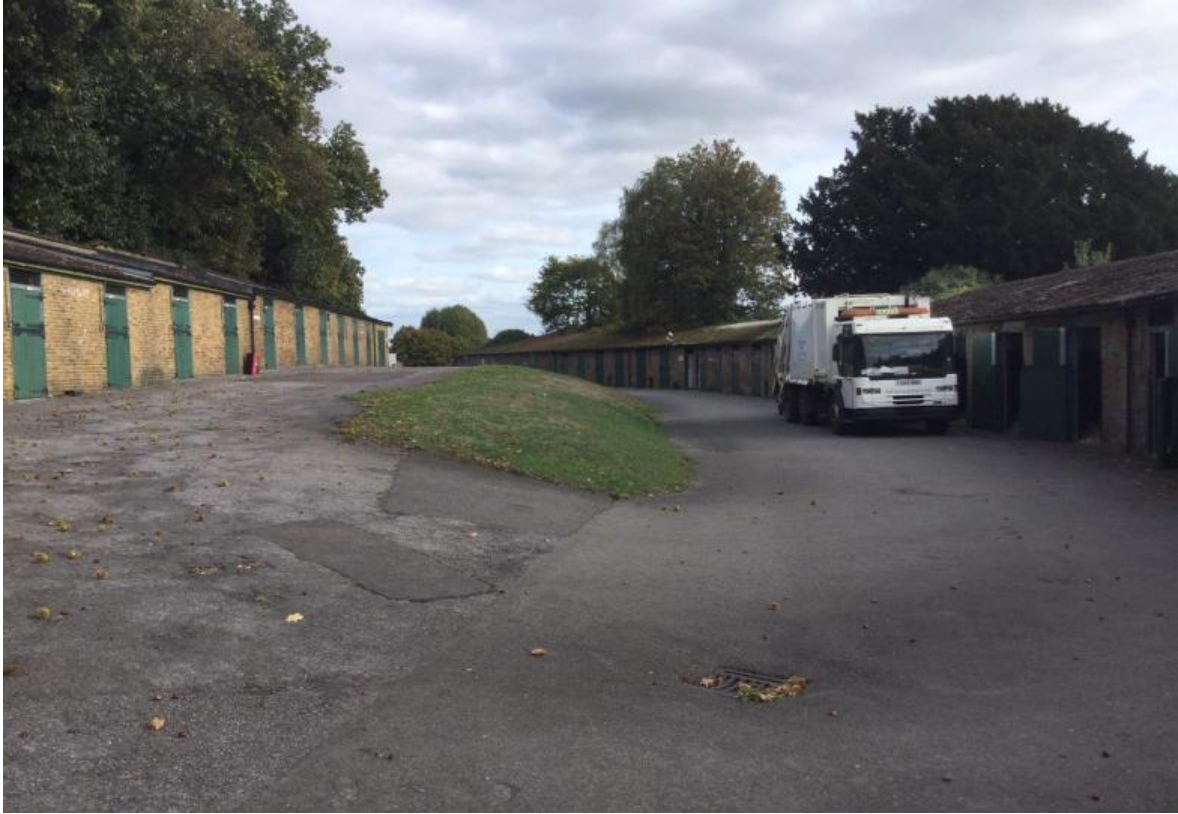
2661/OPA-S1/P3: Site 1 facing southeast
