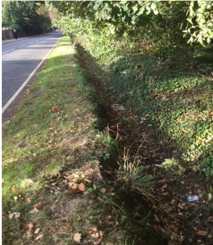
2661/OPA-S4/P2: Drainage ditch along Station Road
