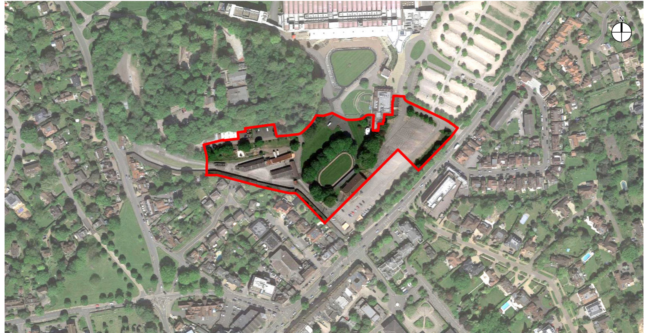
Fig. 11: Existing aerial view of Site A - Racecourse Operational Facilities
