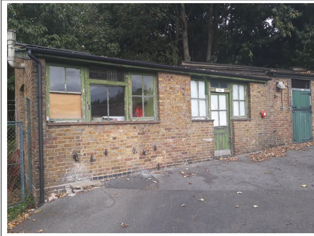
Photo 4 - Storage unit at west end of Site 1
