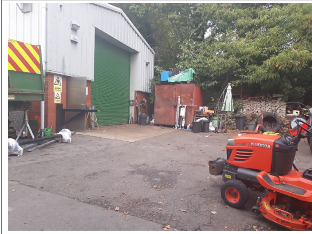
Photo 9 – Maintenance workshop 40m northwest of Site 1
