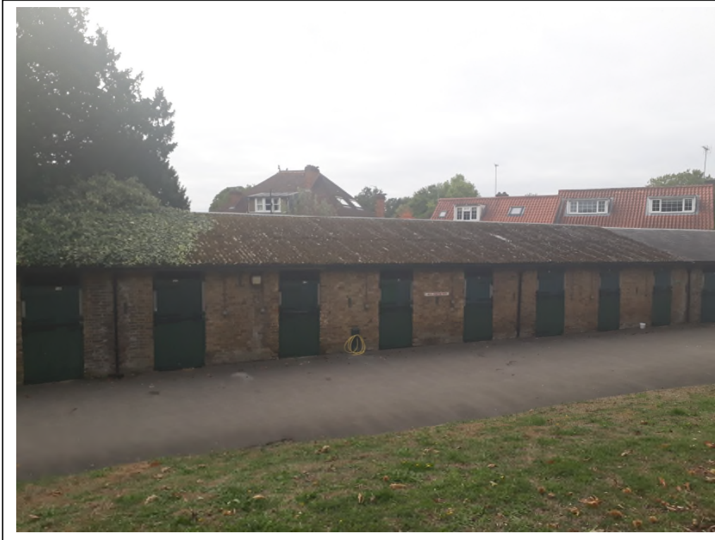
Photo 3 – Stables along south of Site 1 with possible cement bound asbestos roofing
