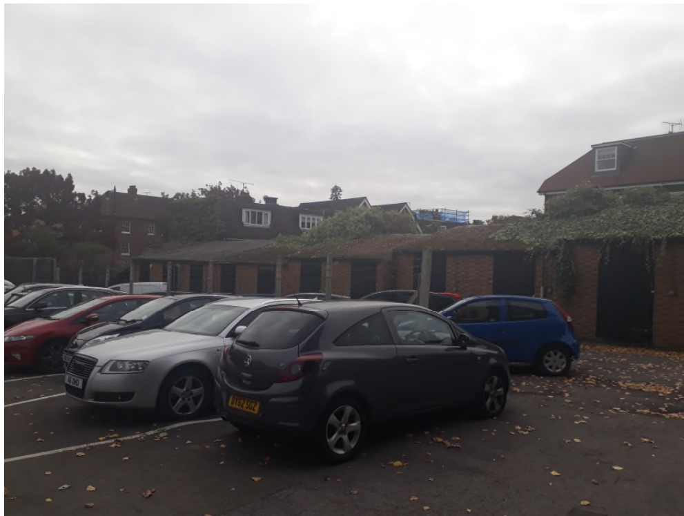
Photo 33 – Stables with possible cement bound asbestos roofing in west of Site 2
