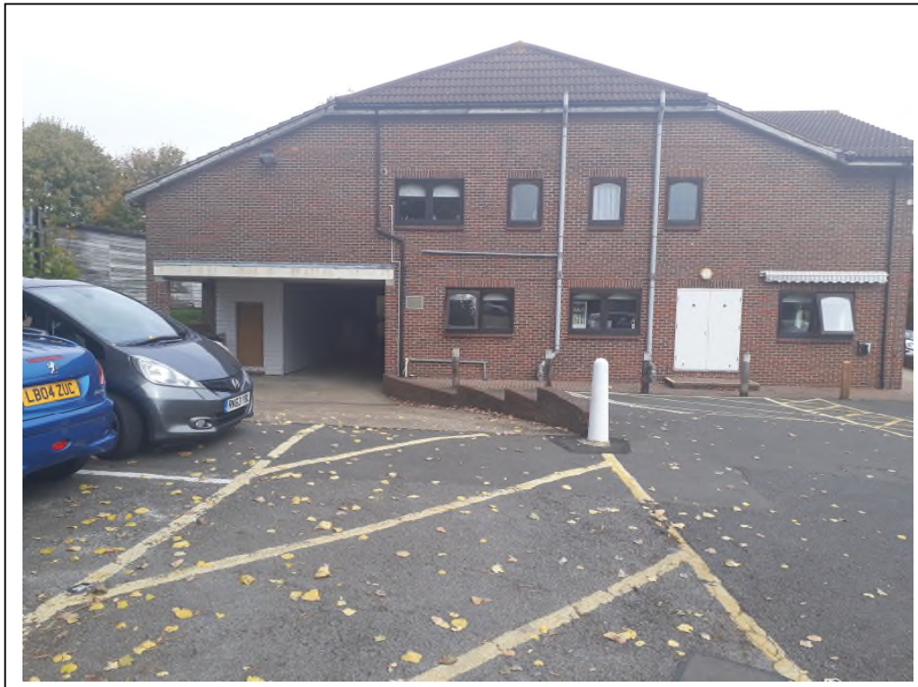
Photo 32 – western end of building at Site 2
