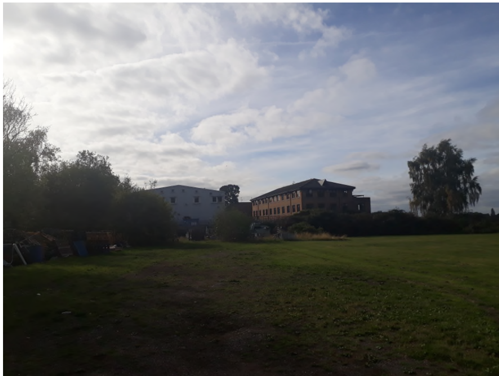
Photo 23 – Looking to west at Site 4 with pallets in and bins at western end
