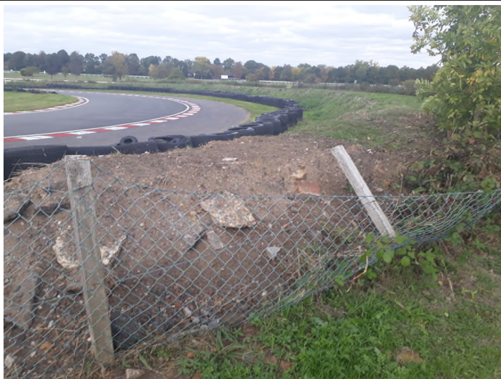
Photo 44 – Bunding around Karting Track
