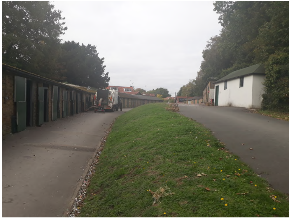
Photo 1 – Looking towards the west at Site 1 showing difference in ground level
