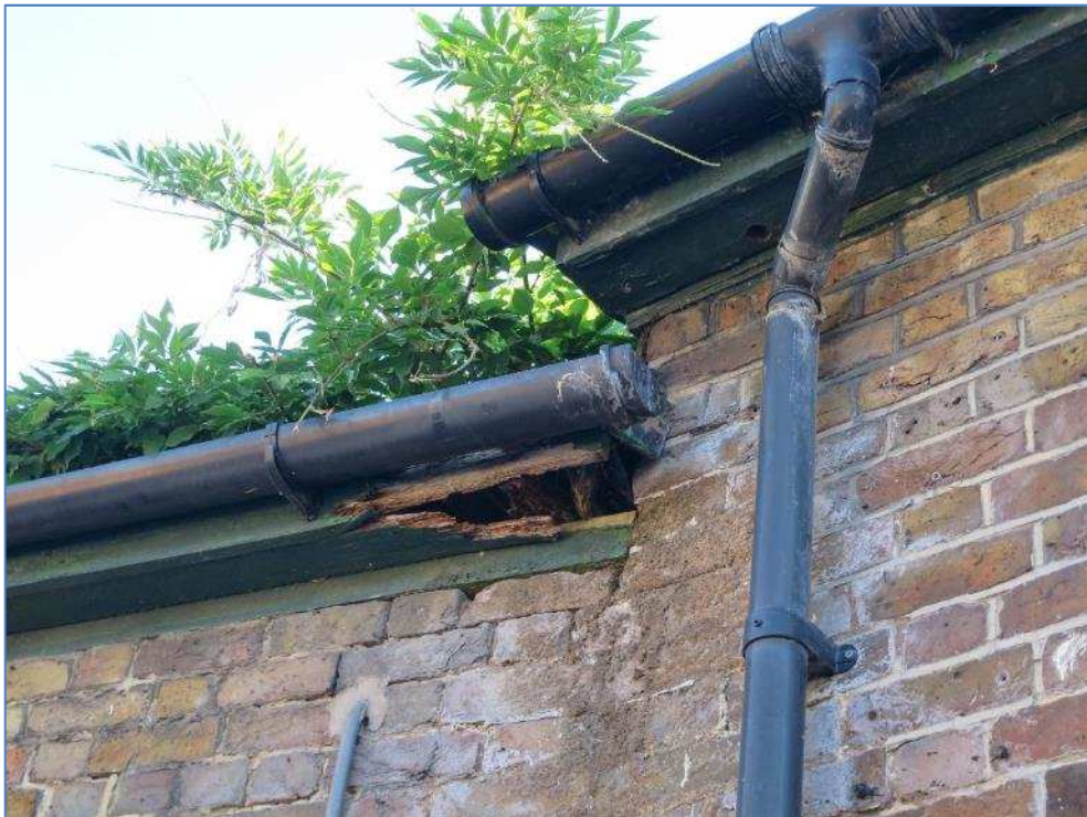
5-37 Timber eaves boarding rotting heavily between stables 53 & 54
