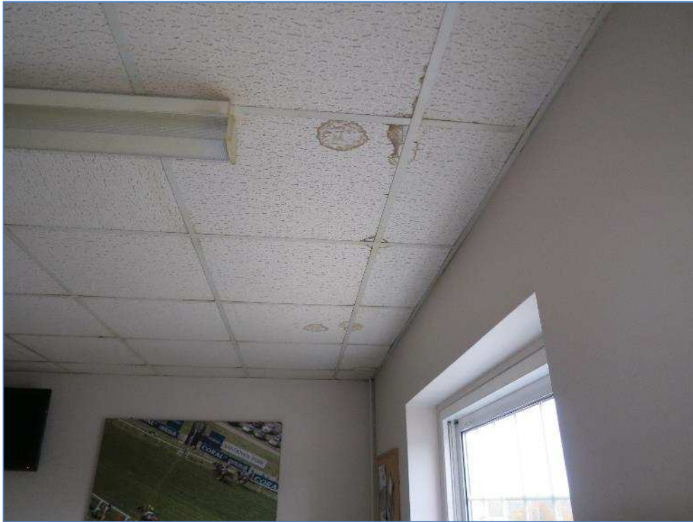
4-08 Damp damage to ceiling in jockeys rest room
