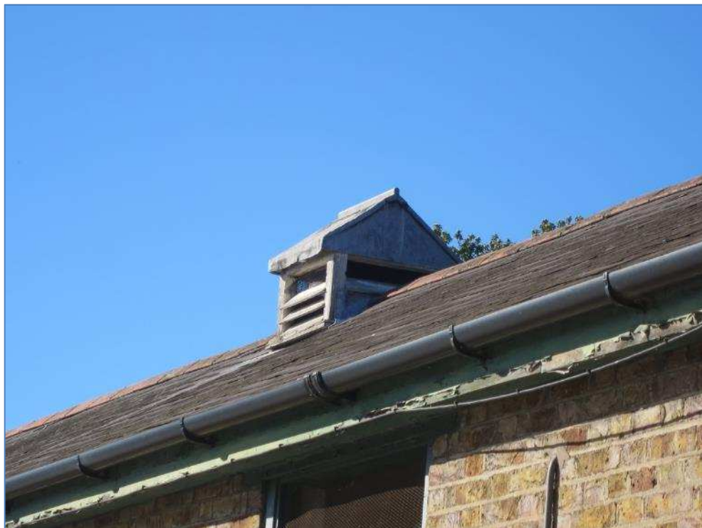
5-11 Timber roof vent box breaking up
