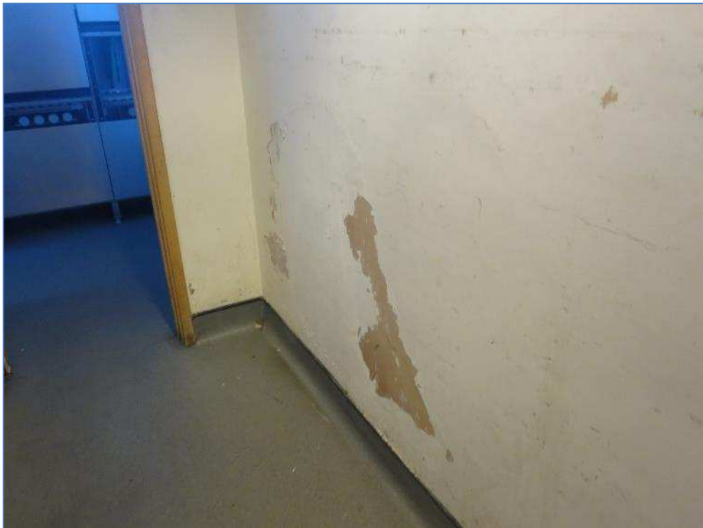
8-08 Water damage to wall in corridor to kitchen
