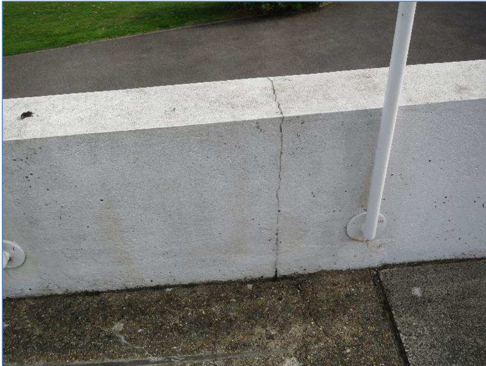
7-56 Crack in end wall of terrace adjacent ramp
