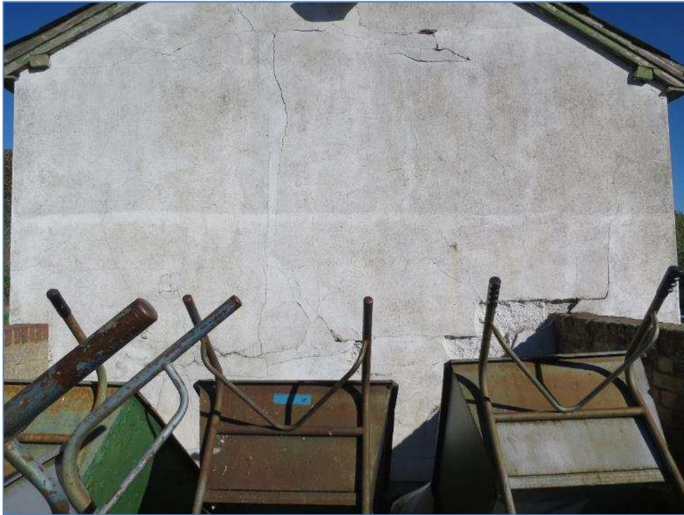
5-16 External render spalled and spalling to end wall
