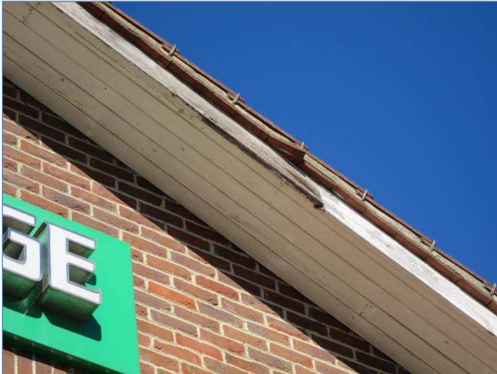
3-01 Loose roof tile over main entrance
