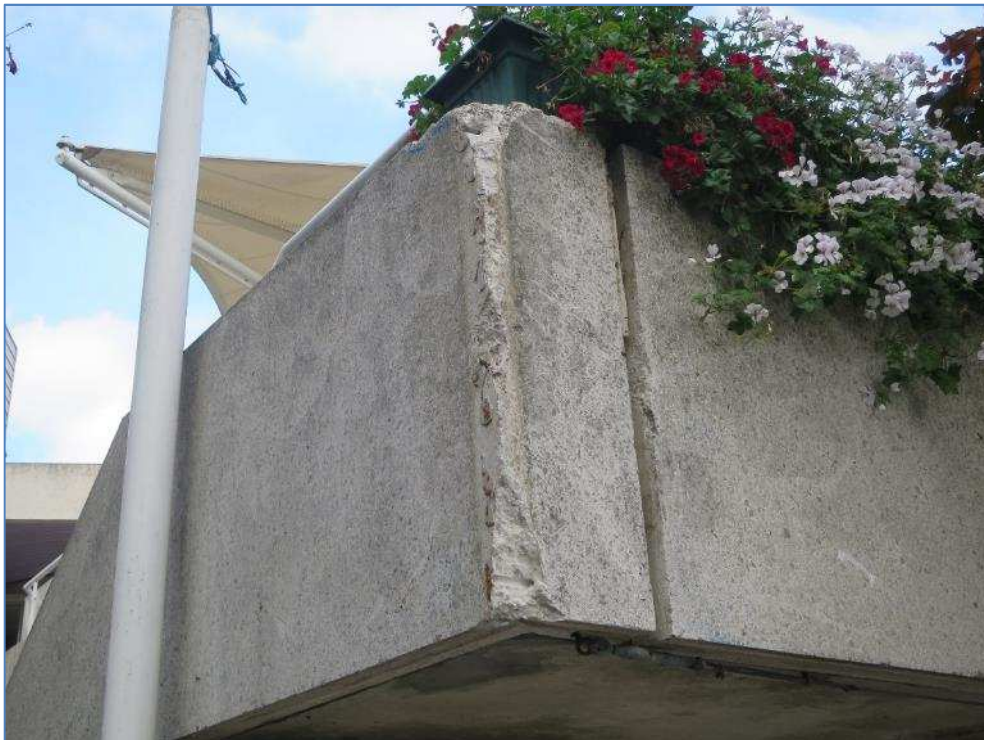
7-09 Minor movement of precast concrete unit due to impact damage
