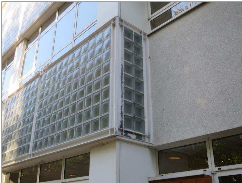
8-02 Paint peeling from steel around feature windows
