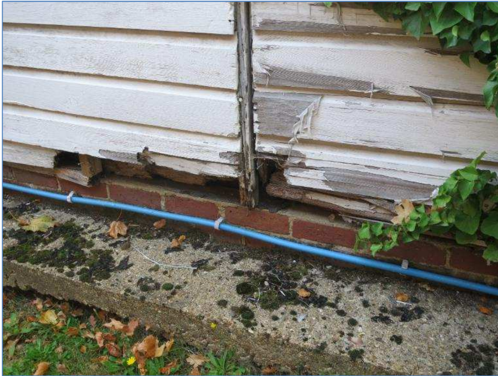
6-03 Timber cladding rotting heavily
