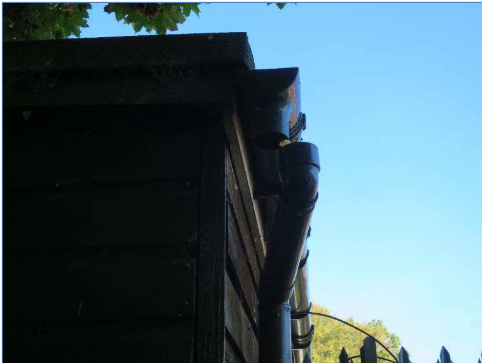
6-04 Gutter downpipe damaged
