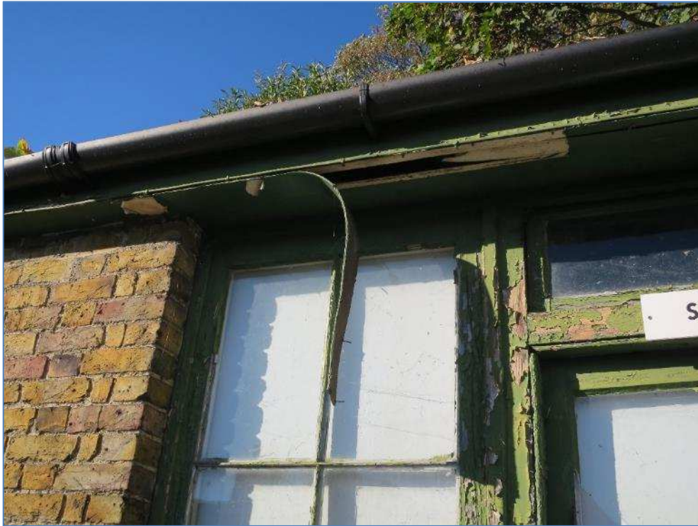
5-24 Timber eaves boarding working loose
