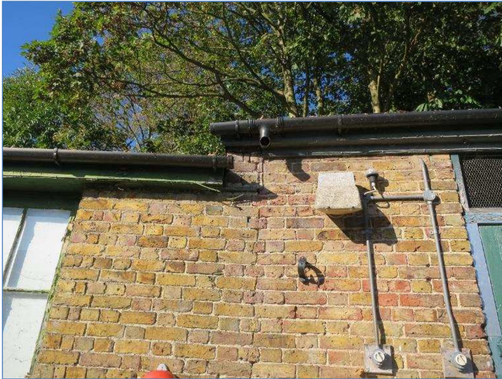
5-22 Gutter downpipe missing near stable 110
