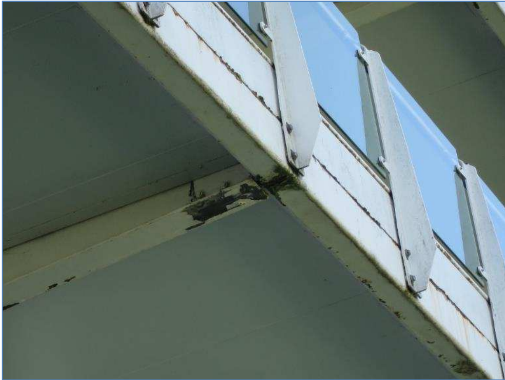
8-03 Surface rust to balcony support steelwork
