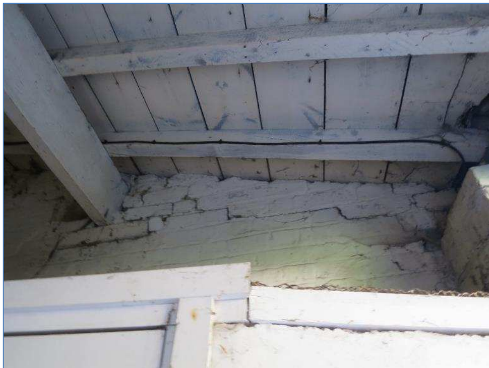
5-29 Cracks in wall to tack boxes 19-24 adjacent stable 17
