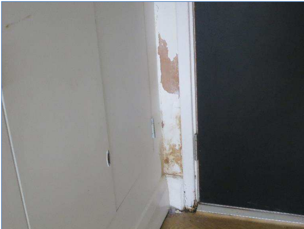
7-05 Water damage to wall in media centre entrance foyer
