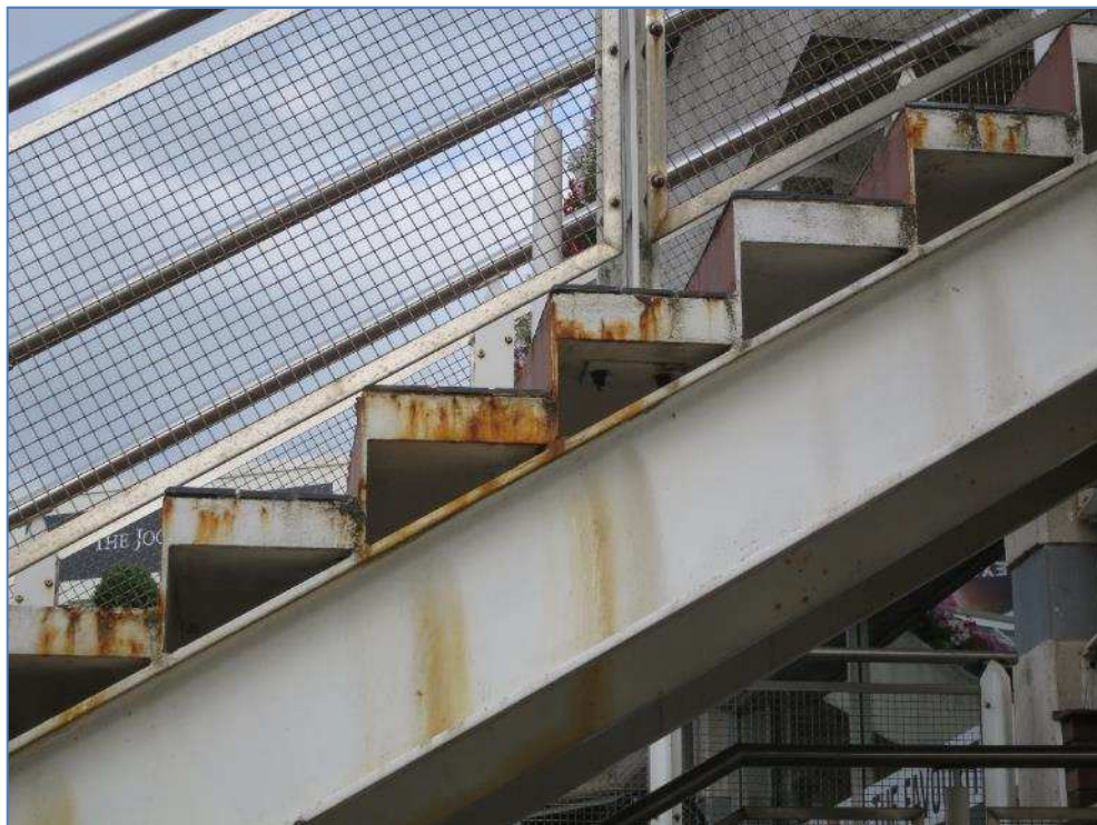
7-03 Surface rust to steelwork to staircase
