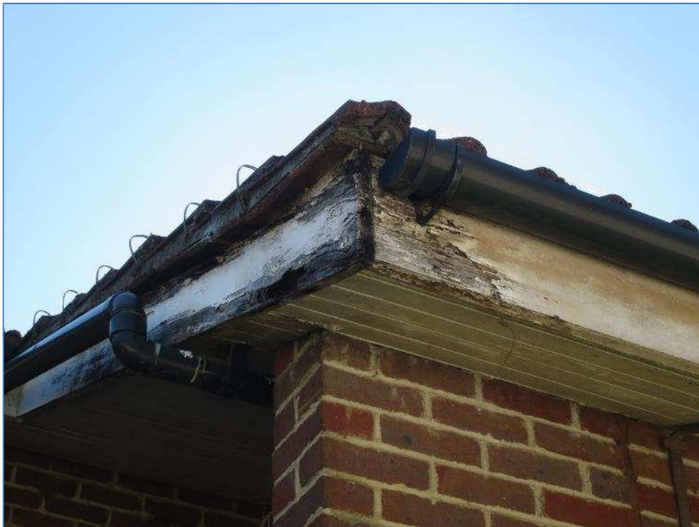
3-04 Timber fascia on rear elevation rotting heavily
