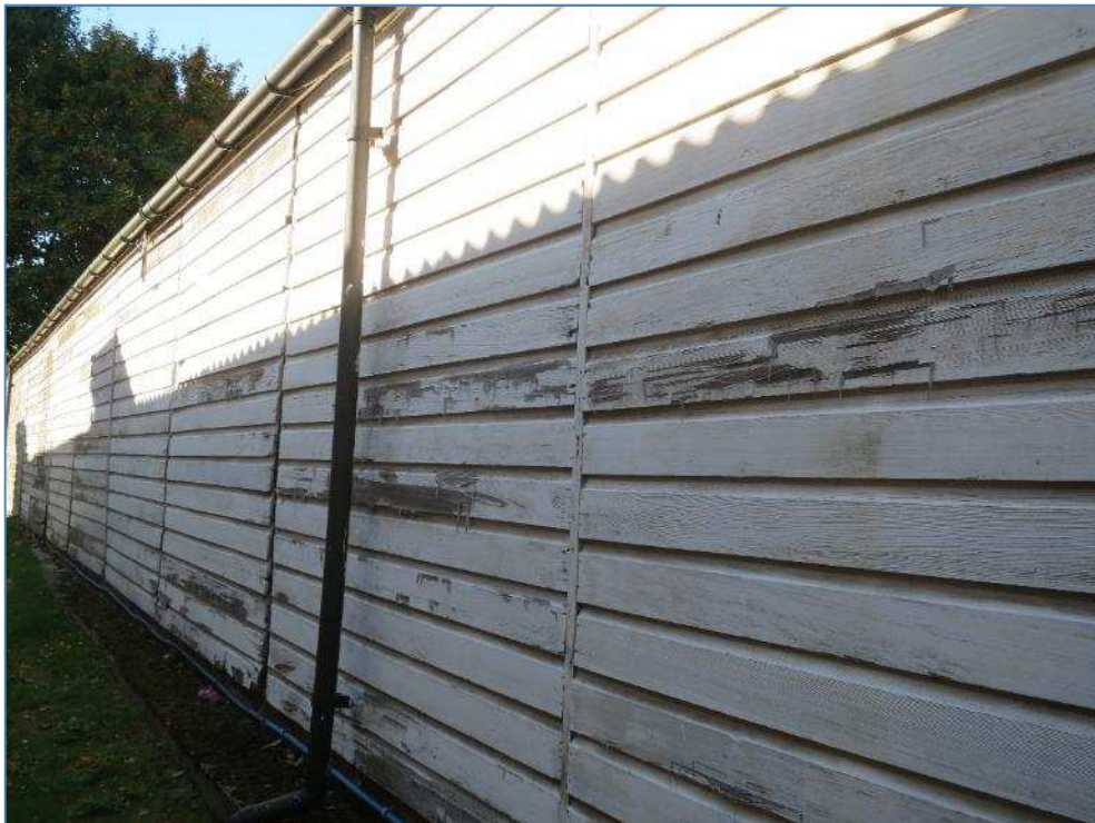
6-01 Paint peeling heavily from timber cladding
