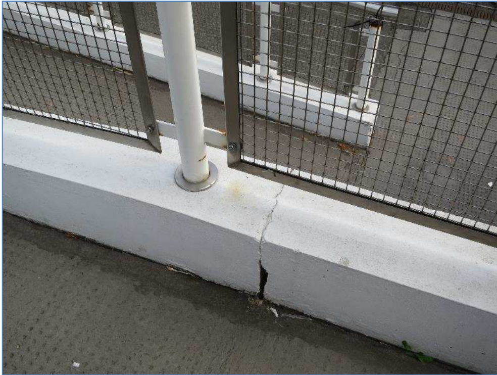
7-54 Cracks in concrete wall to ramp
