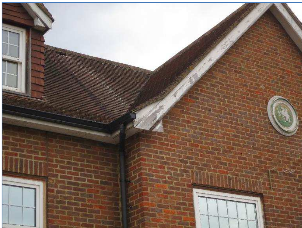
4-03 Heavy rot to timber fascia
