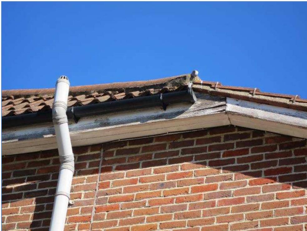
3-02 Timber eaves boarding rotting
