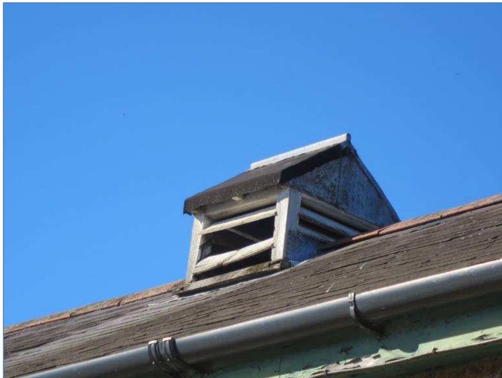
5-10 Timber roof vent box breaking up
