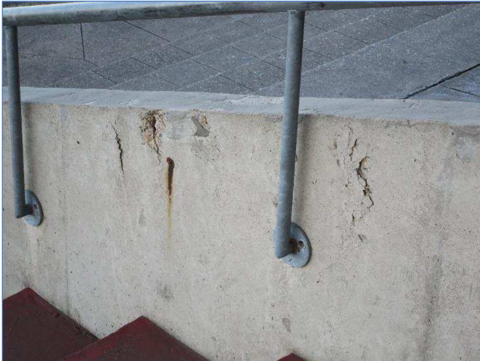
7-46 Concrete spalling on vomitory wall
