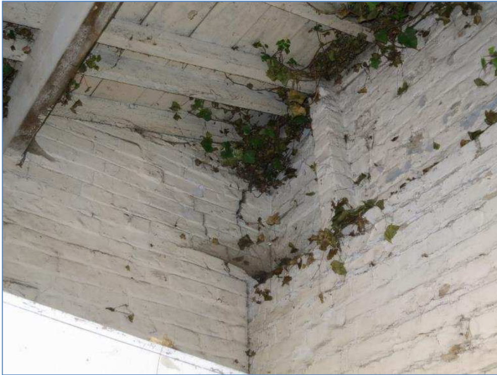
5-32 Crack in wall in tack boxes 13-19 adjacent stable 32
