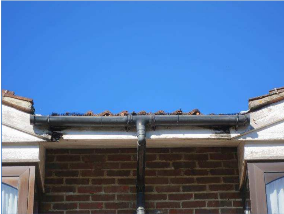
3-03 Timber eaves boarding rotting
