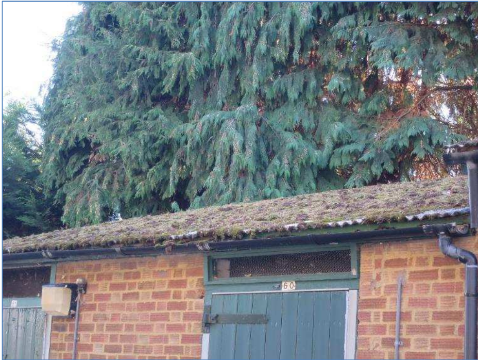
5-26 Heavy moss build up on roof
