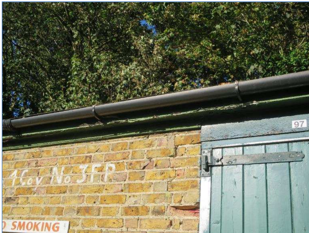
5-20 Paint peeling from timber eaves boards with minor rot
