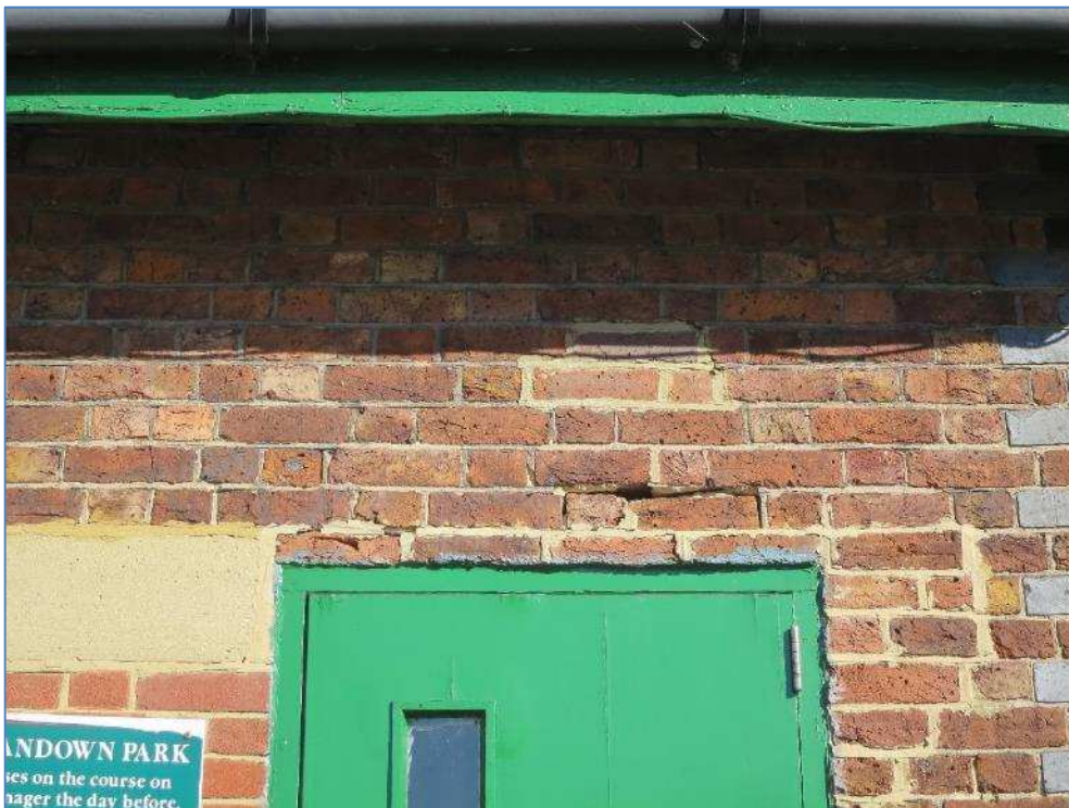
5-03 Loose brick over door to stable manager's office
