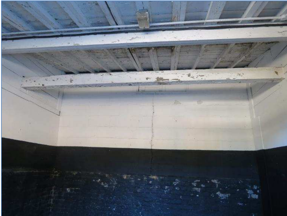
5-36 Crack in rear wall of stable 46
