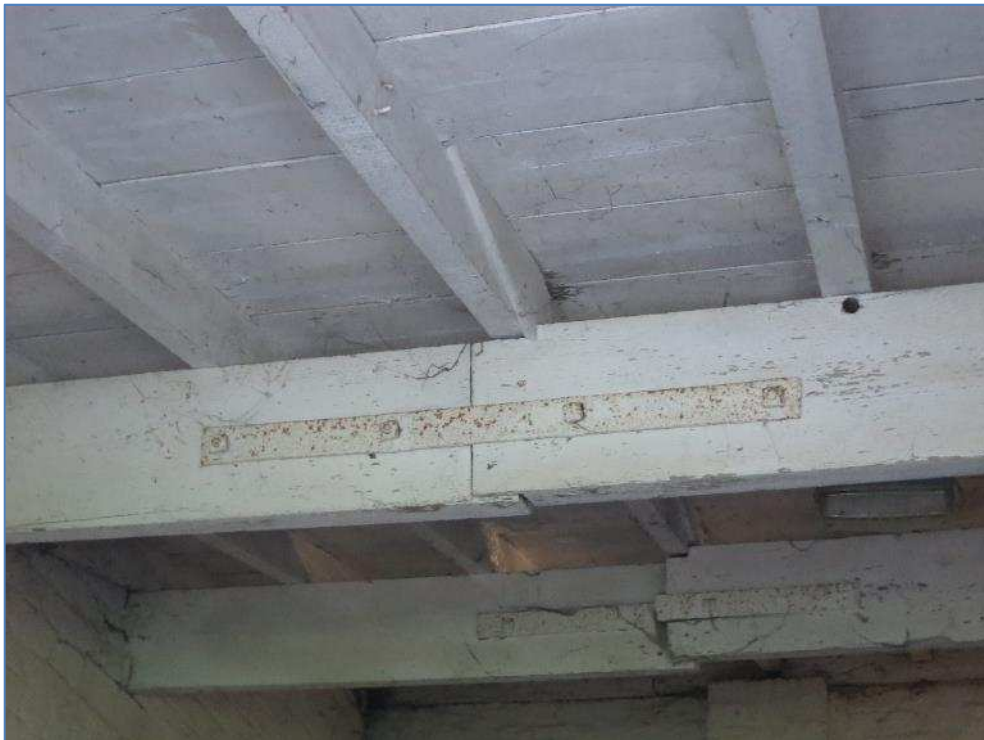
5-31 Minor surface rust to roof timber tie straps
