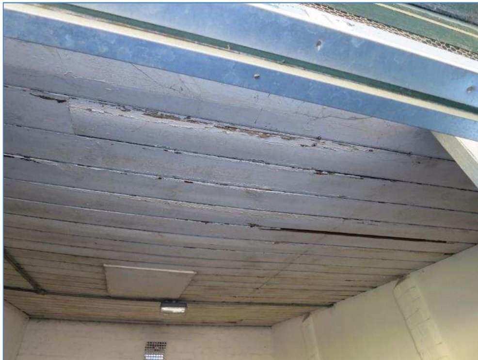
5-28 Timber soffit boarding rotting in stable 1
