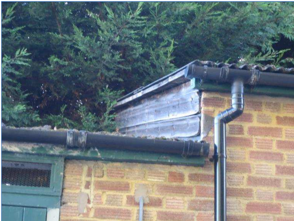
5-39 Roof step timber to stable 63 rotting and warping heavily
