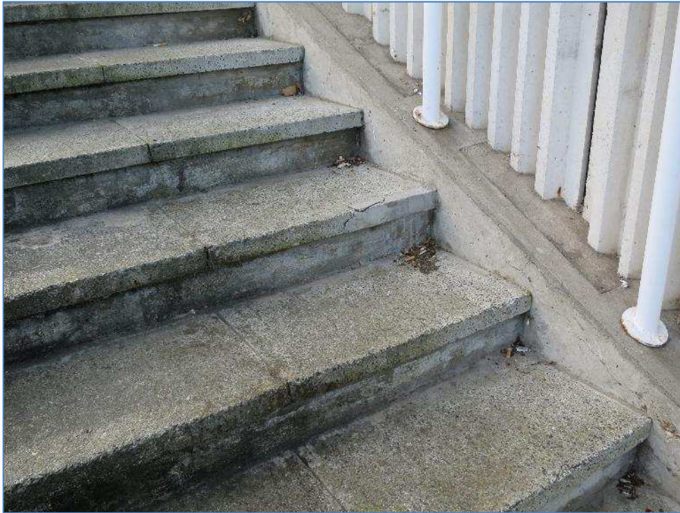
7-50 Concrete repair failing
