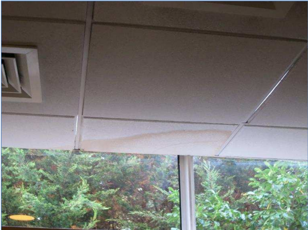
8-05 Water damage to ceiling in gent's toilet
