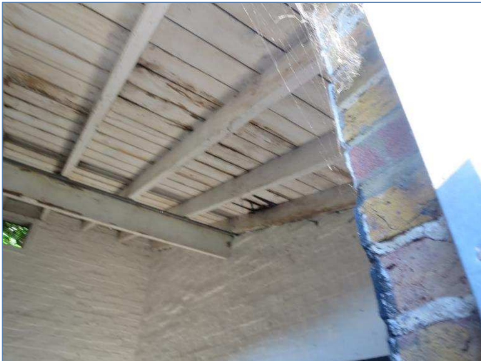
5-19 Minor rot to timber soffit boarding in stable 103
