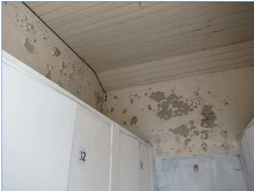
5-12 Paint peeling heavily from walls in tack boxes 31-36
