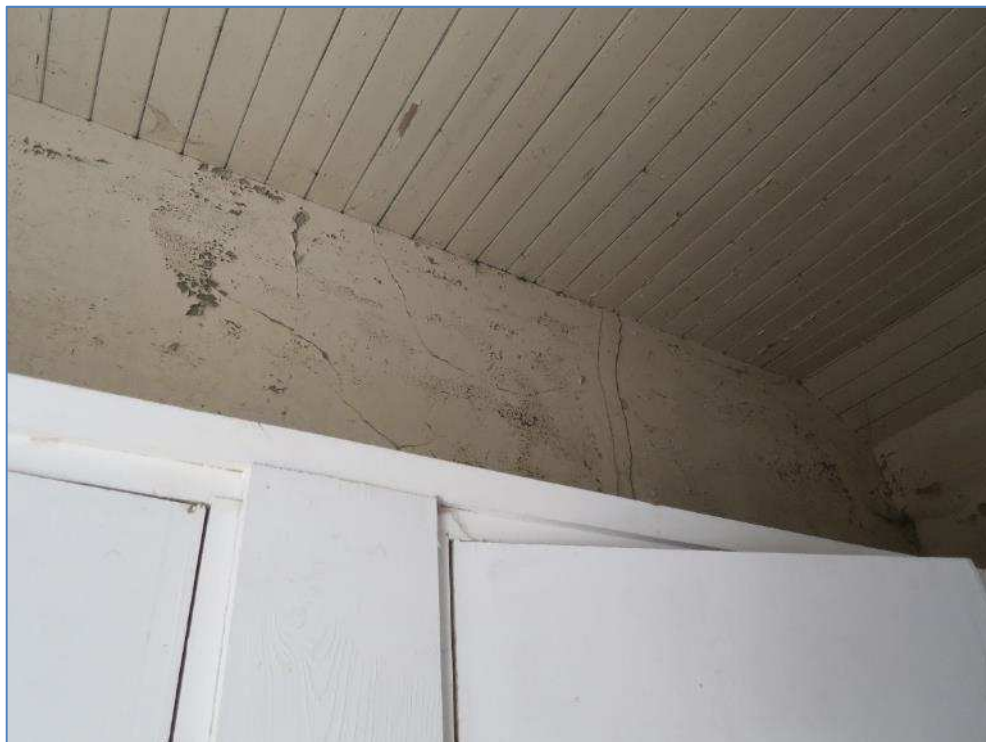
5-13 Cracks in end wall of tack boxes 7-12
