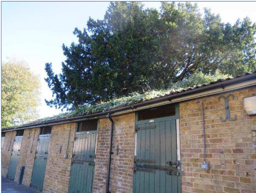
5-25 Plant growth on roof
