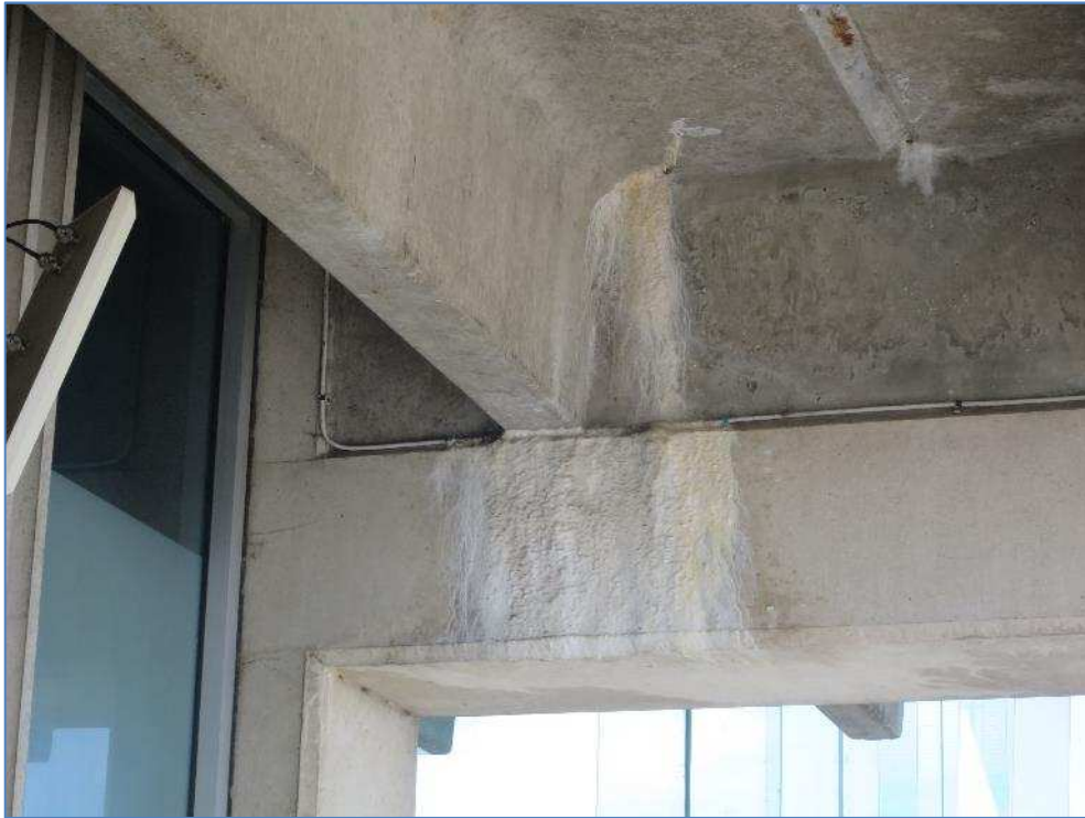
7-52 Leaching through concrete terrace
