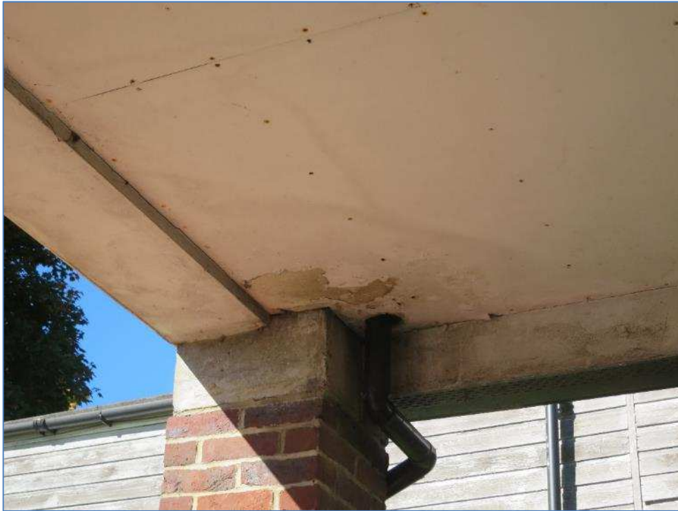
3-05 Water damage to soffit of carport
