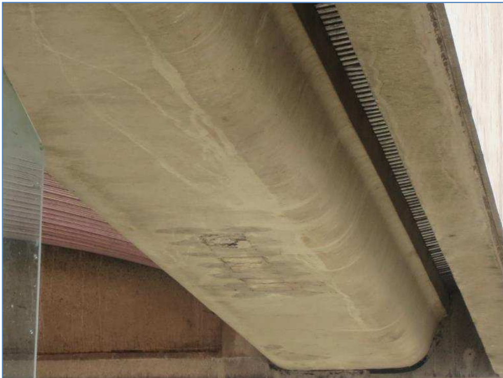
7-13 Minor area of concrete spalled to roof beam
