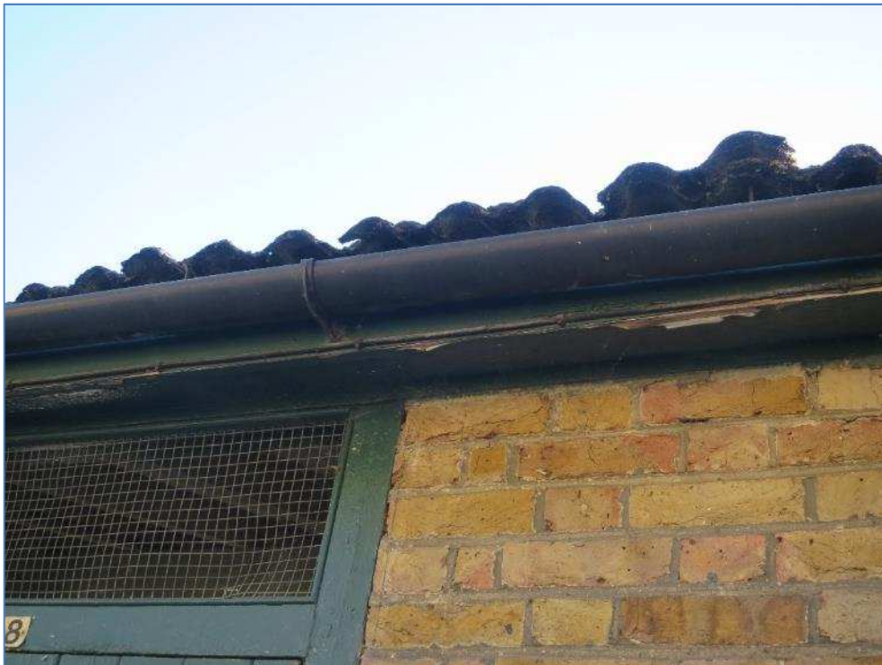
5-27 Asbestos roof sheeting fraying at edges
