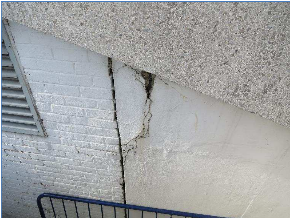
7-57 Cracks in render to end wall of stand
