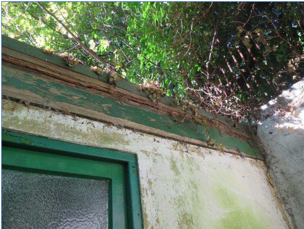
5-17 Timber eaves boards rotting heavily to toilet block
