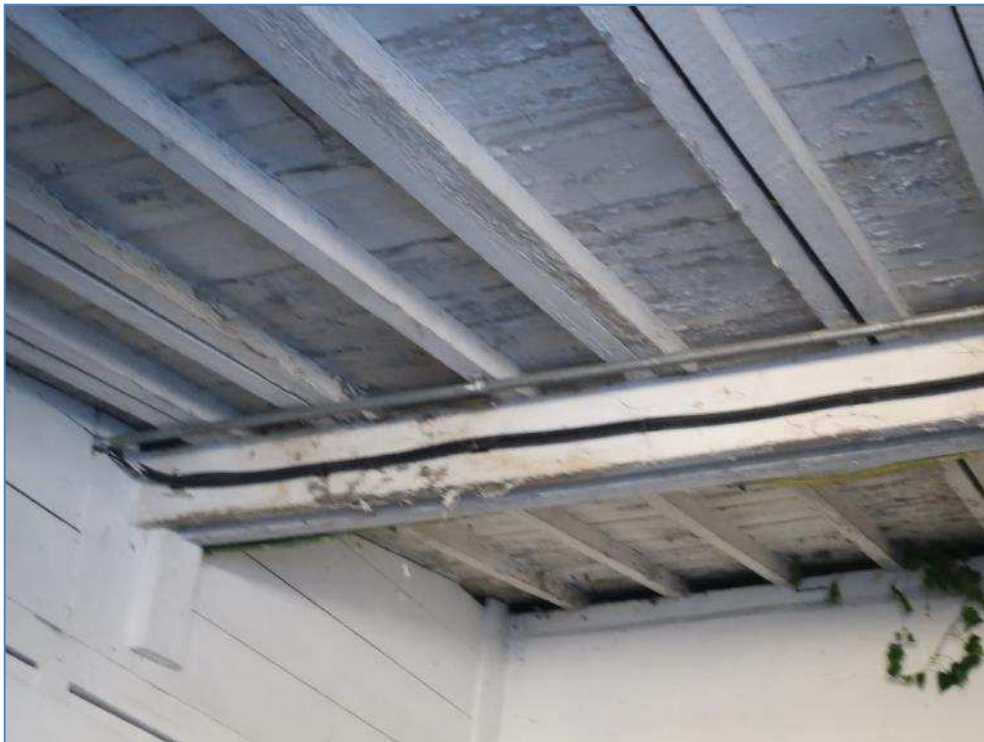
5-33 Timber soffit boarding rotting in stable 49
