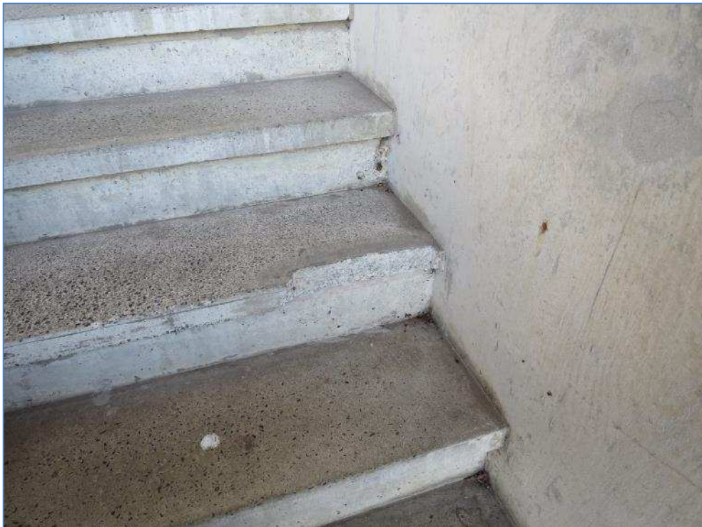
7-47 Section of concrete step spalled
