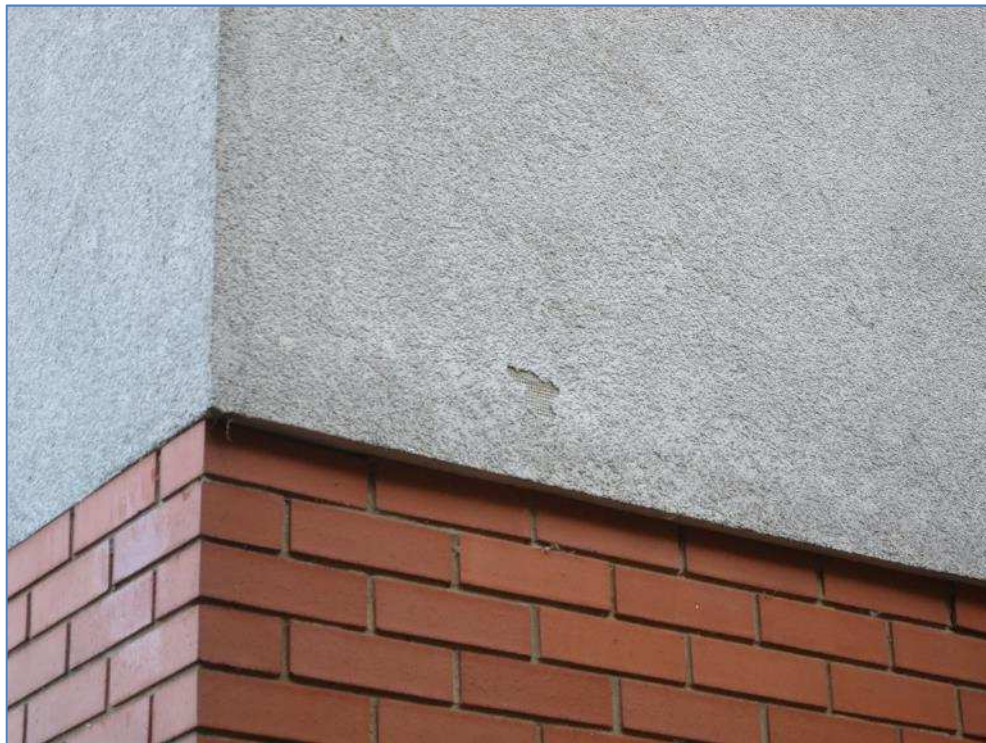
8-01 Minor area of render spalled new bin store
