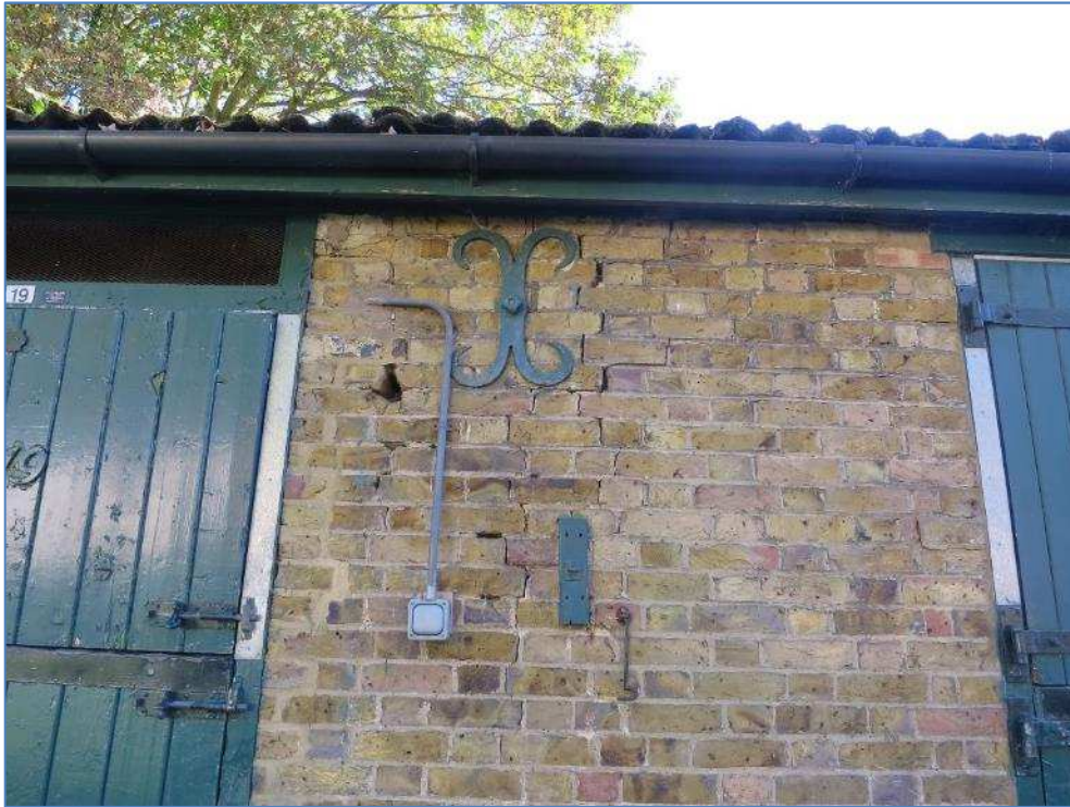
5-30 Crack in wall between stables 18 & 19
