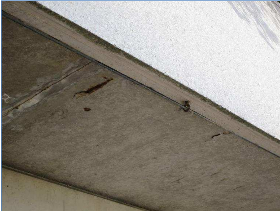
7-08 Concrete spalling on underside of viewing terrace new Champagne Bar
