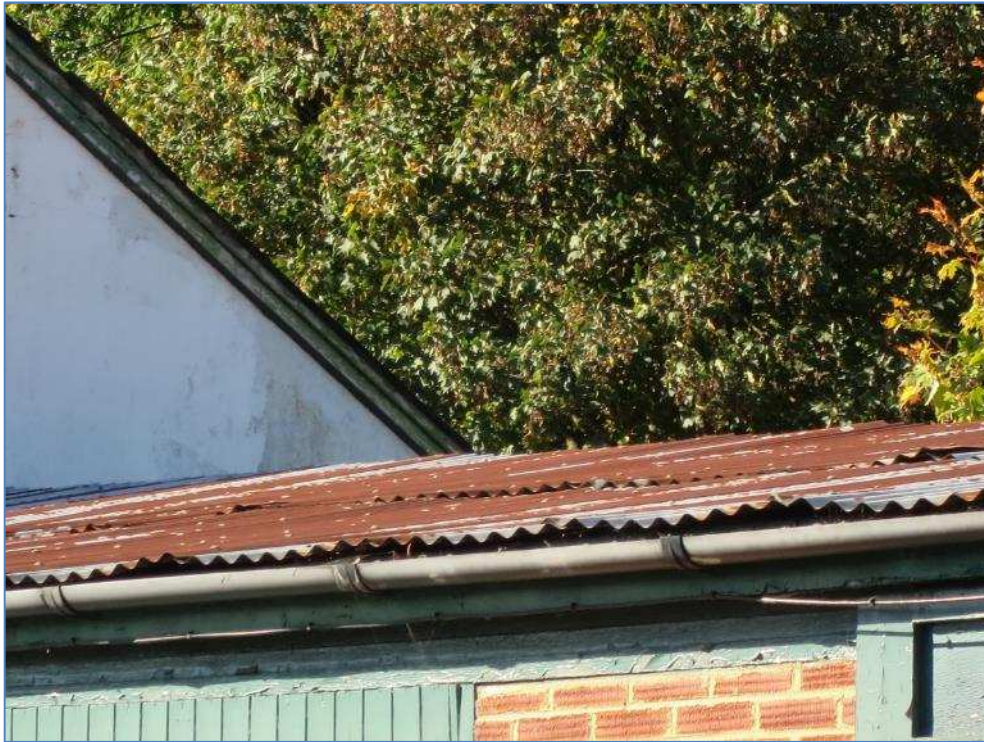
5-02 Corrugated roof sheeting rusting heavily
