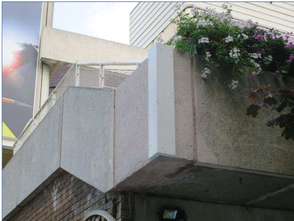
7-10 Impact damaged precast unit replaced with insitu concrete
