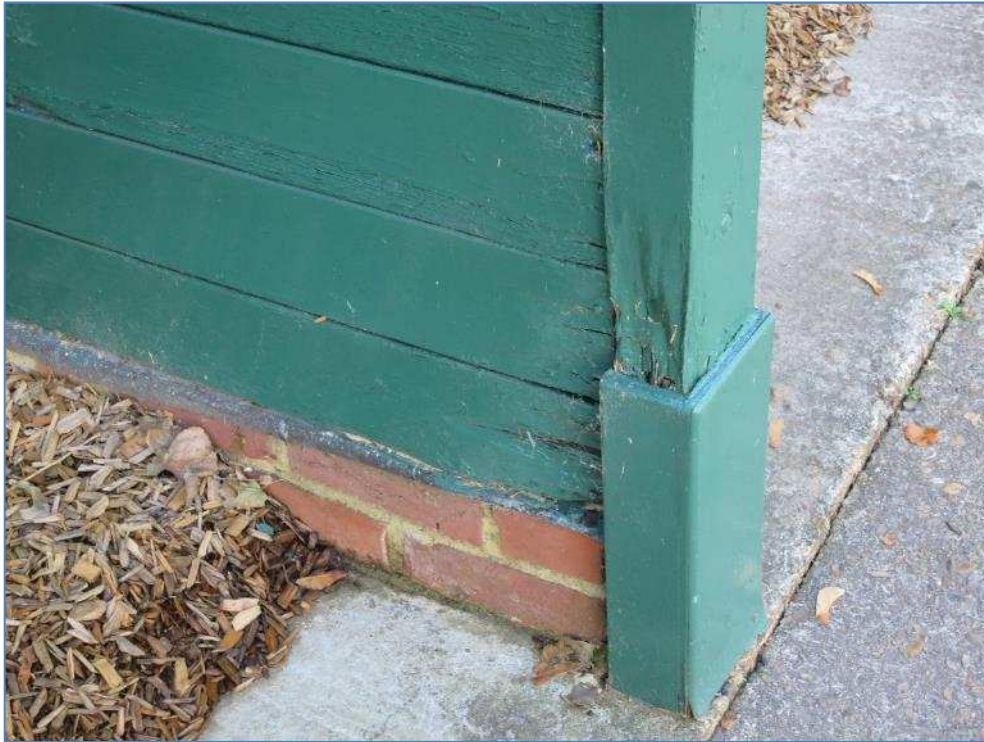
6-06 Timber to saddling box rotting
