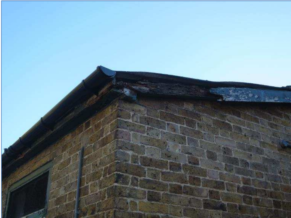
5-38 Timber eaves boarding rotting heavily outside stable 56
