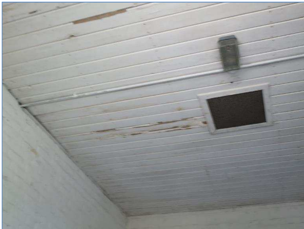
5-07 Timber soffit boarding rotting in stable 72
