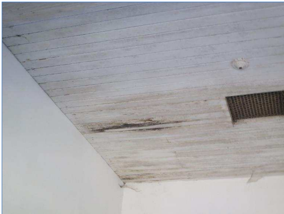
5-15 Timber soffit boards rotting in stable 96
