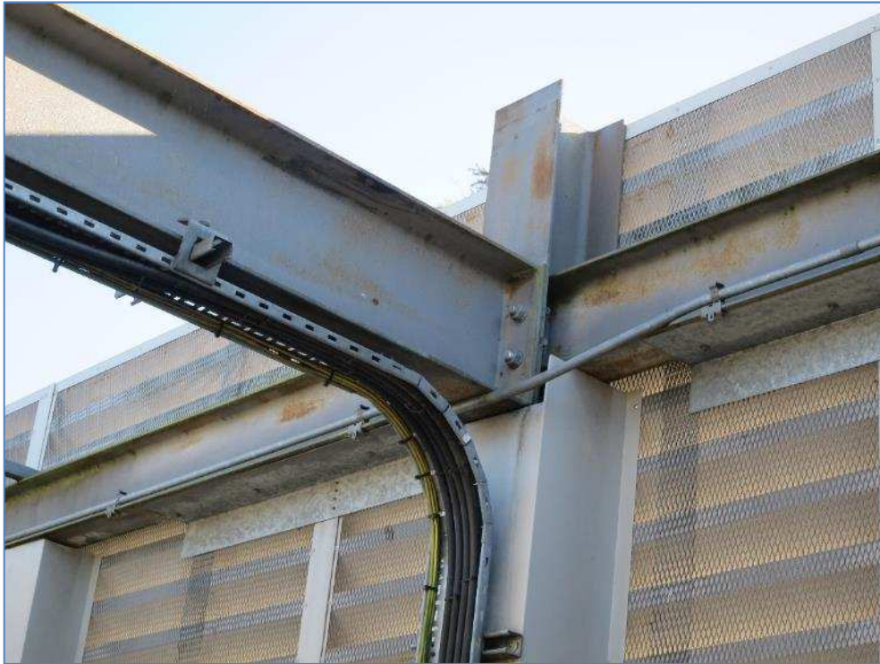
8-13 Minor surface rust to plant enclosure support steelwork
