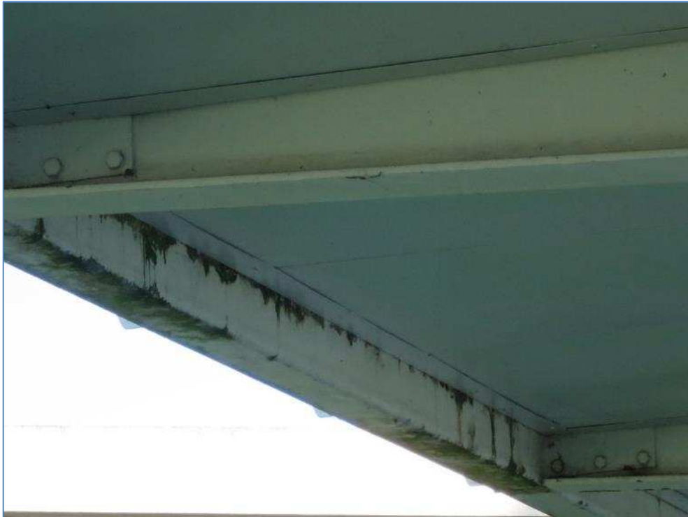
8-07 Surface rust to balcony support steelwork
