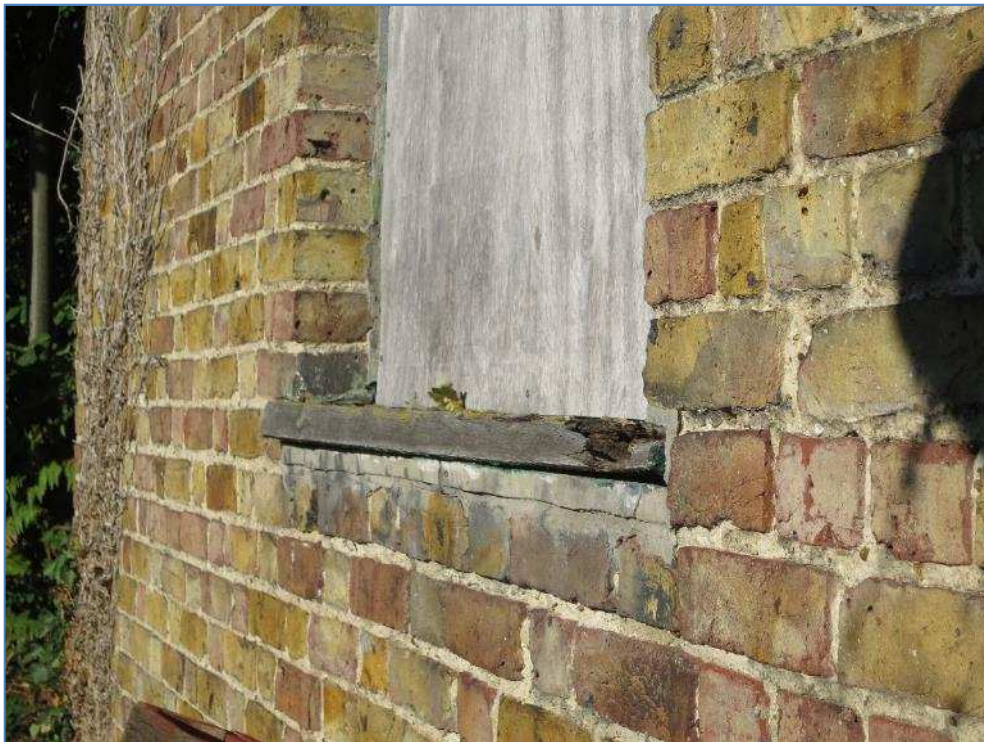
5-23 Timber window frame rotting heavily
