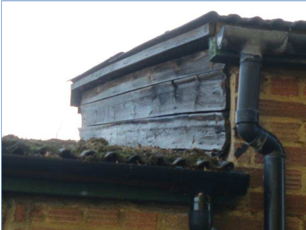
5-40 Roof step timber to stable 65 rotting and warping heavily
