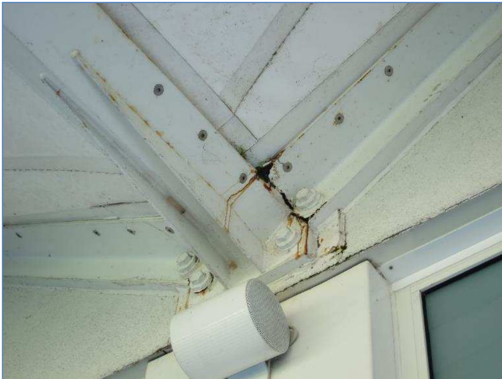
8-10 Minor surface rust to roof canopy support steelwork
