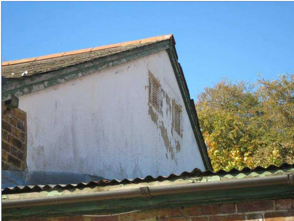
5-09 Paint peeling from end wall of stable 81
