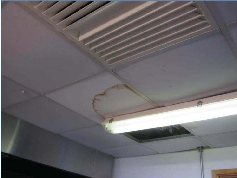
8-09 Water damage to ceiling in kitchen
