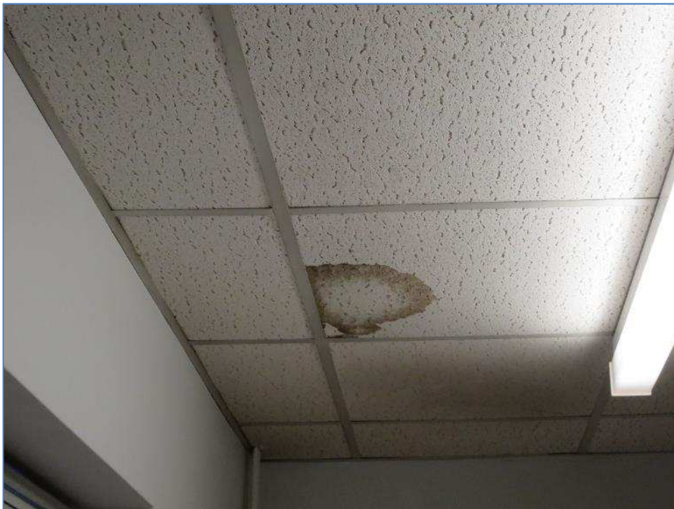
4-06 Damp damage to ceiling in lady jockeys toilet
