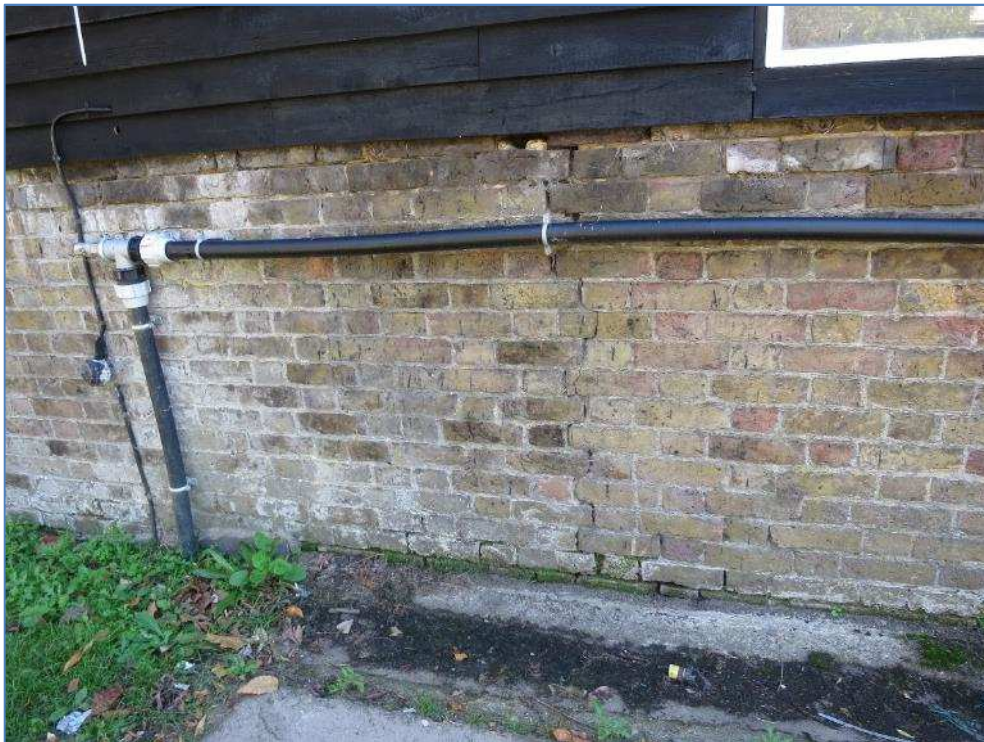
5-01 Cracks in brickwork to rear of veterinary unit
