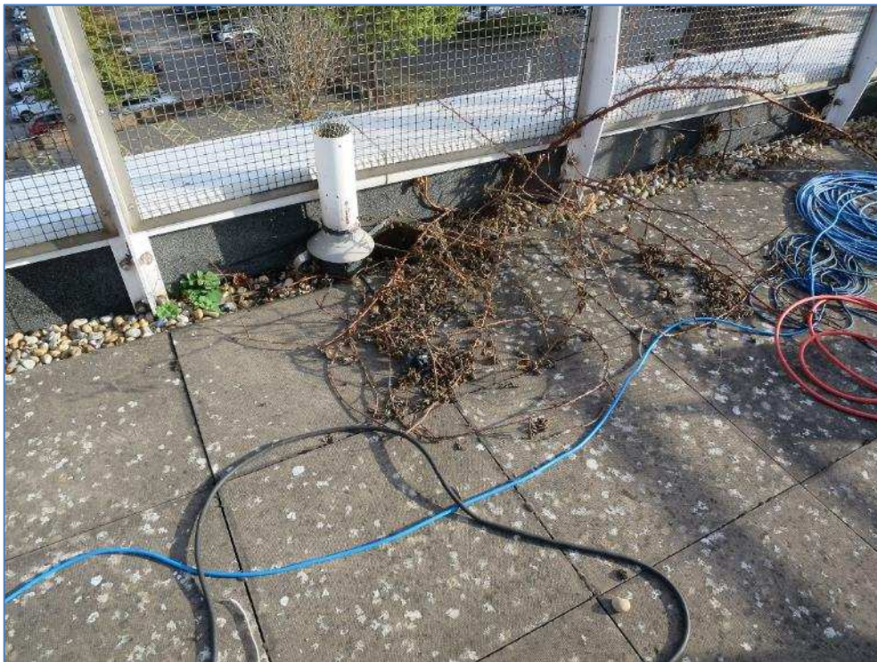
7-04 Plant growth on roof of media centre
