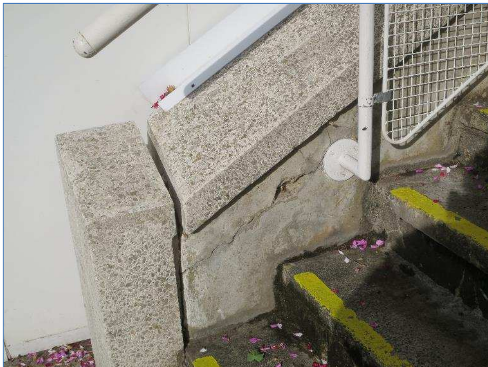
7-11 Cracks in concrete to central staircase
