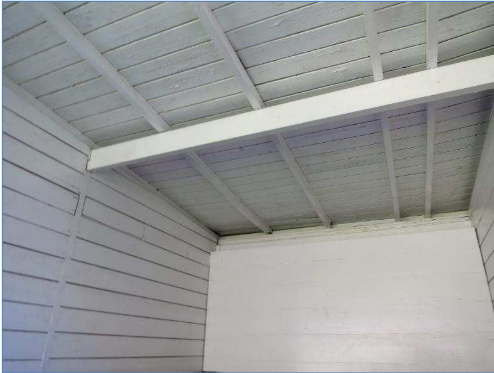
6-05 Timber soffit boarding warping
