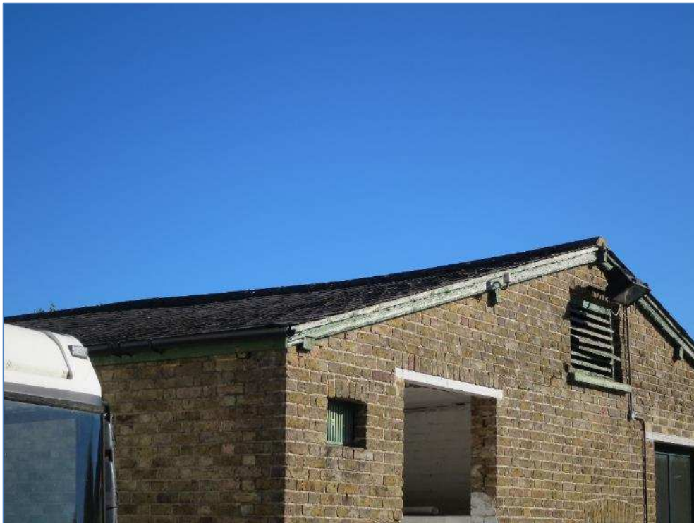
5-05 Roof ridge sagging over stables
