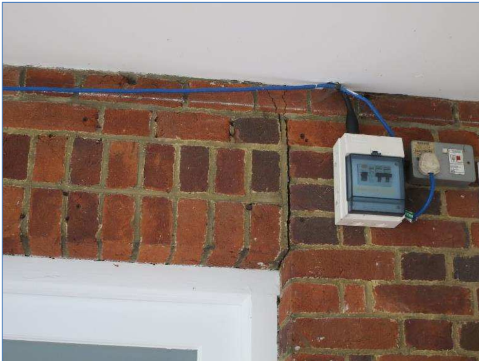
4-05 Crack in brickwork at end of lintel
