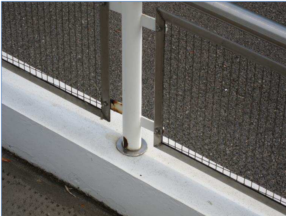
7-55 Surface rust to barrier where finishes have failed
