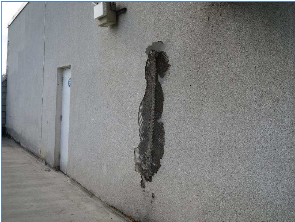
7-51 Render spalled on side wall to stand
