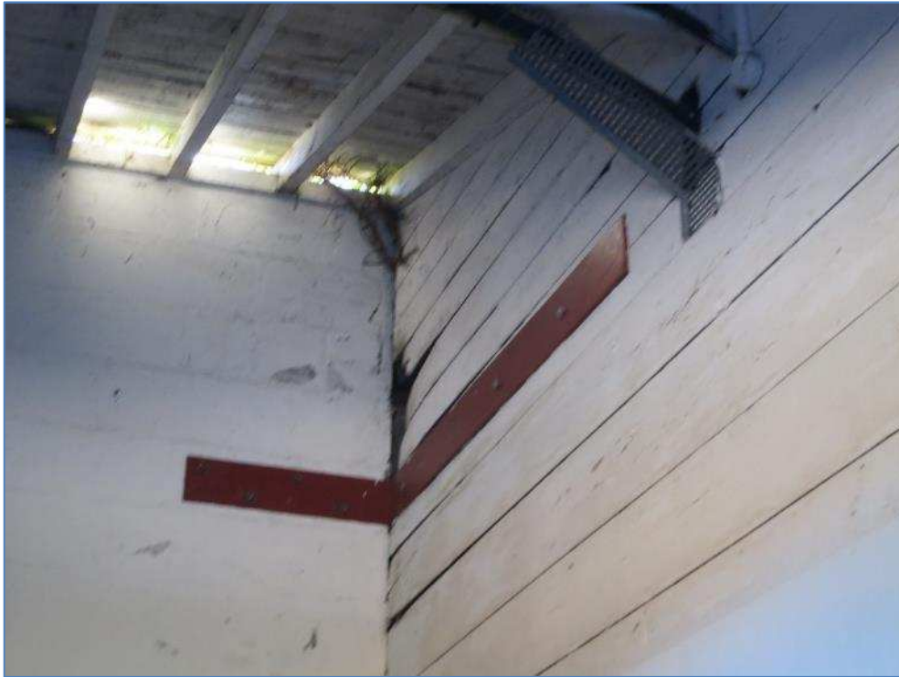
5-34 Wall timber rotting heavily in stable 51
