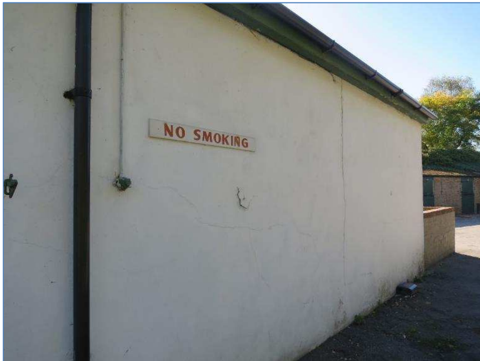
5-14 Cracks and loose render to external wall
