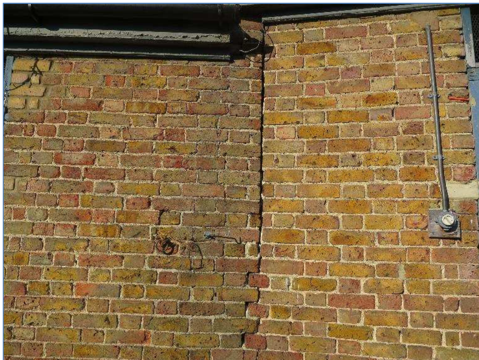
5-21 Crack in wall at step between stables 108 & 109
