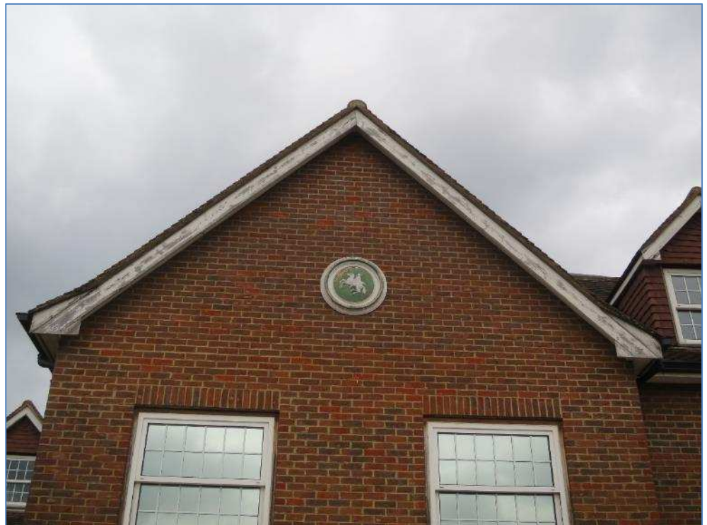
4-02 Paint peeling heavily from timber fascias
