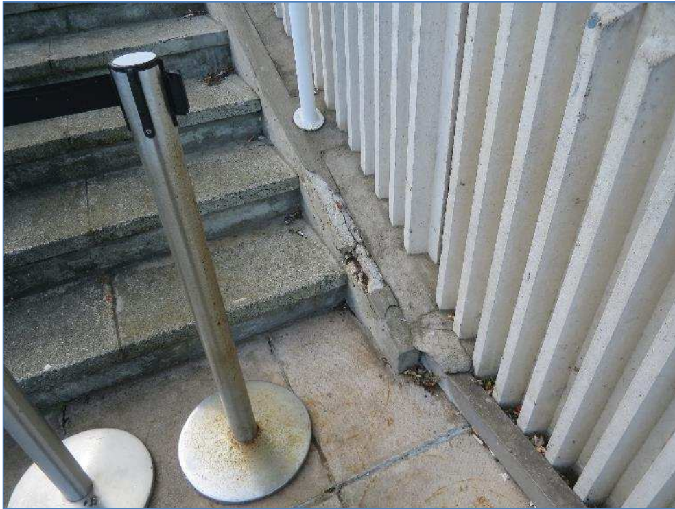
7-48 Concrete spalling on side wall to steps
