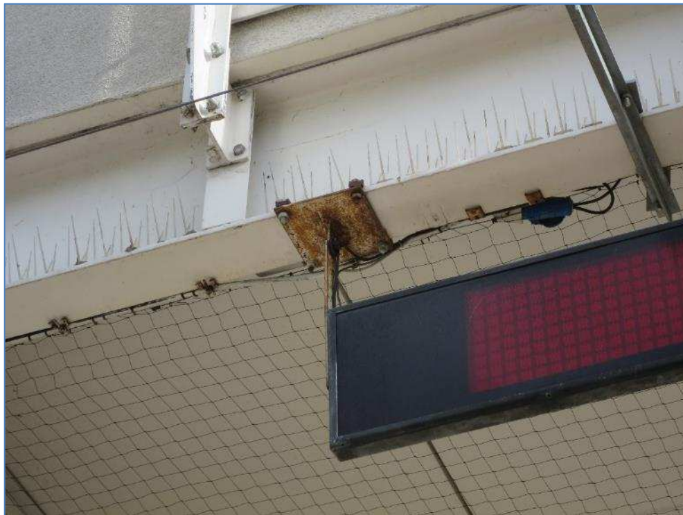
7-02 Illuminated sign support bracket rusting
