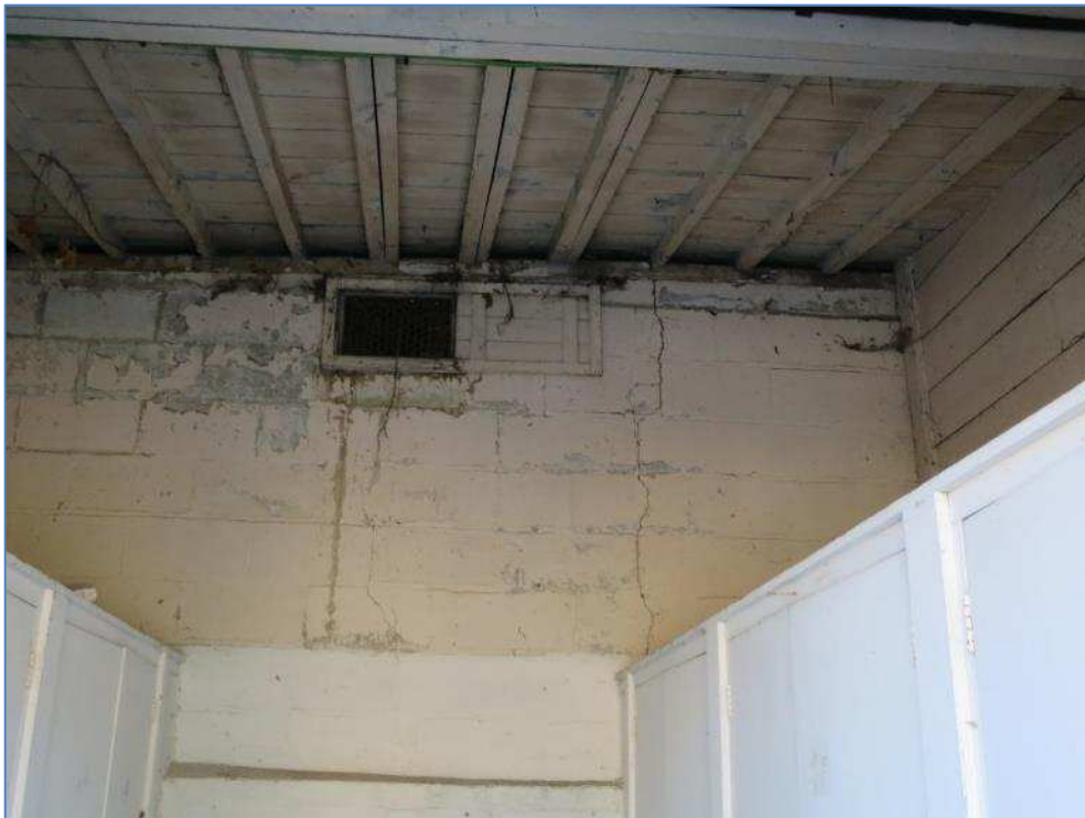
5-35 Cracks in rear wall of tack boxes 1-6
