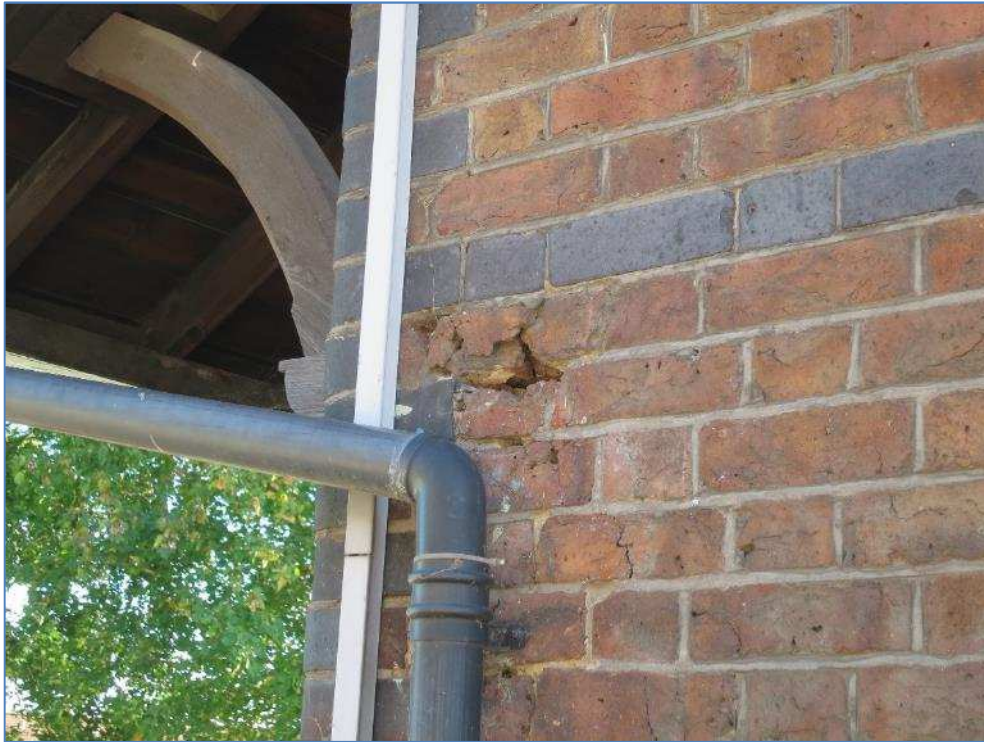
5-04 Bricks spalling on end wall of entrance building
