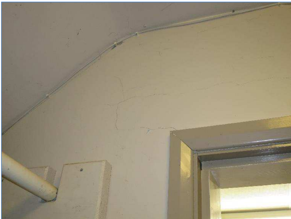
4-07 Minor cracks in wall in valets store room
