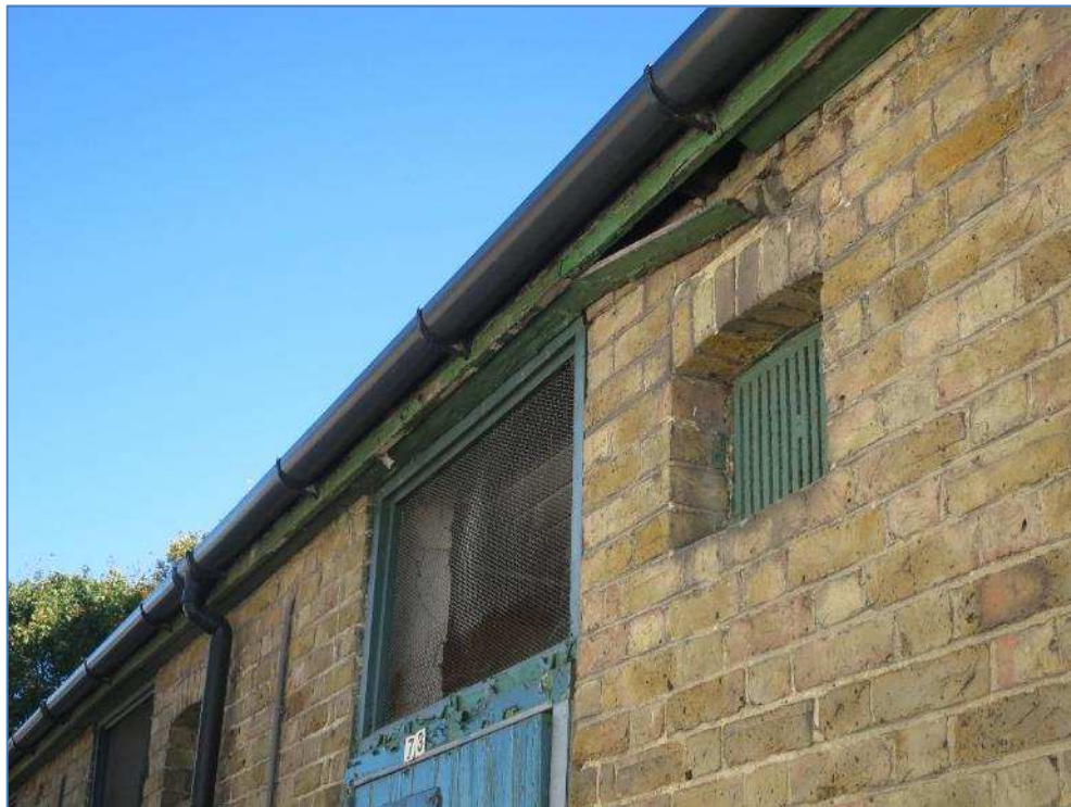
5-06 Eaves soffit board working loose
