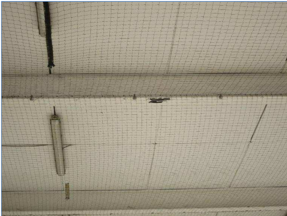
7-01 Paint peeling from media centre support steelwork
