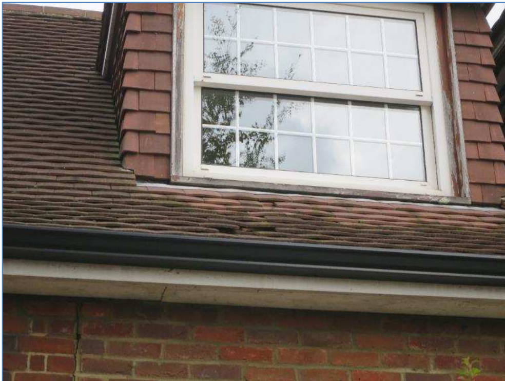
4-01 Missing and damaged roof tiles outside male jockeys
