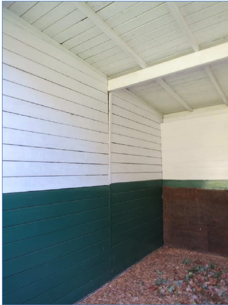
6-06 Timber infill between panels working loose
