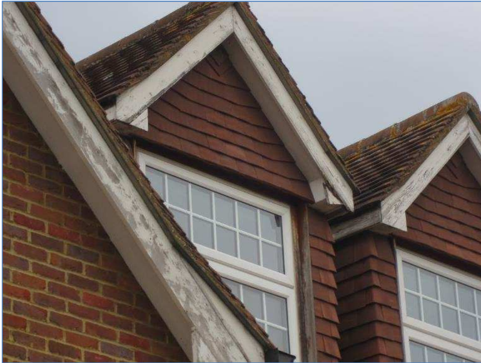
4-04 Heavy rot to timber fascias
