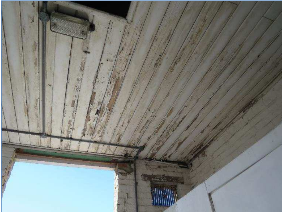
5-08 Damp and rot to timber soffit boards in tack boxes 25-30
