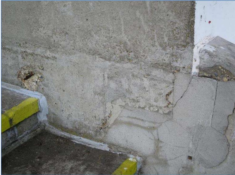
7-42 Concrete spalling on Esher Hall 3 wall
