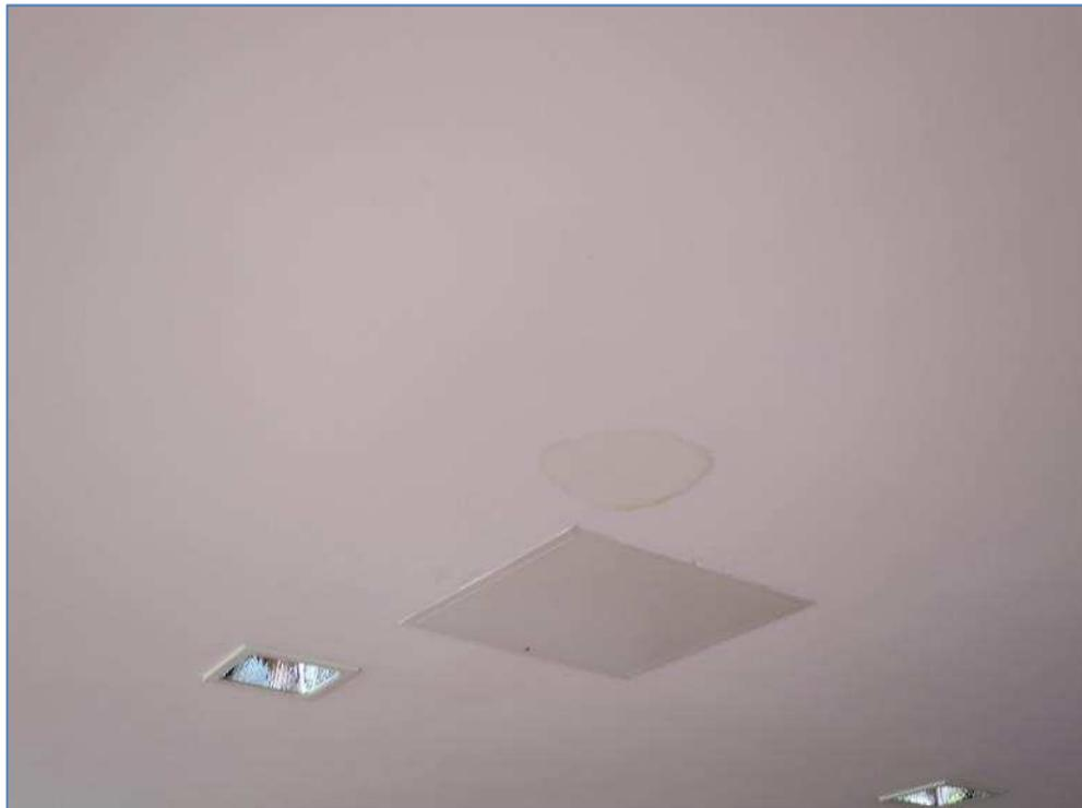
7-20 Water damage to ceiling by side door to Esher Hall
