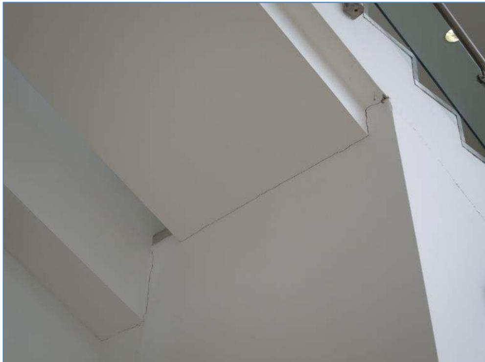
7-24 Cracks between escalator and wall below
