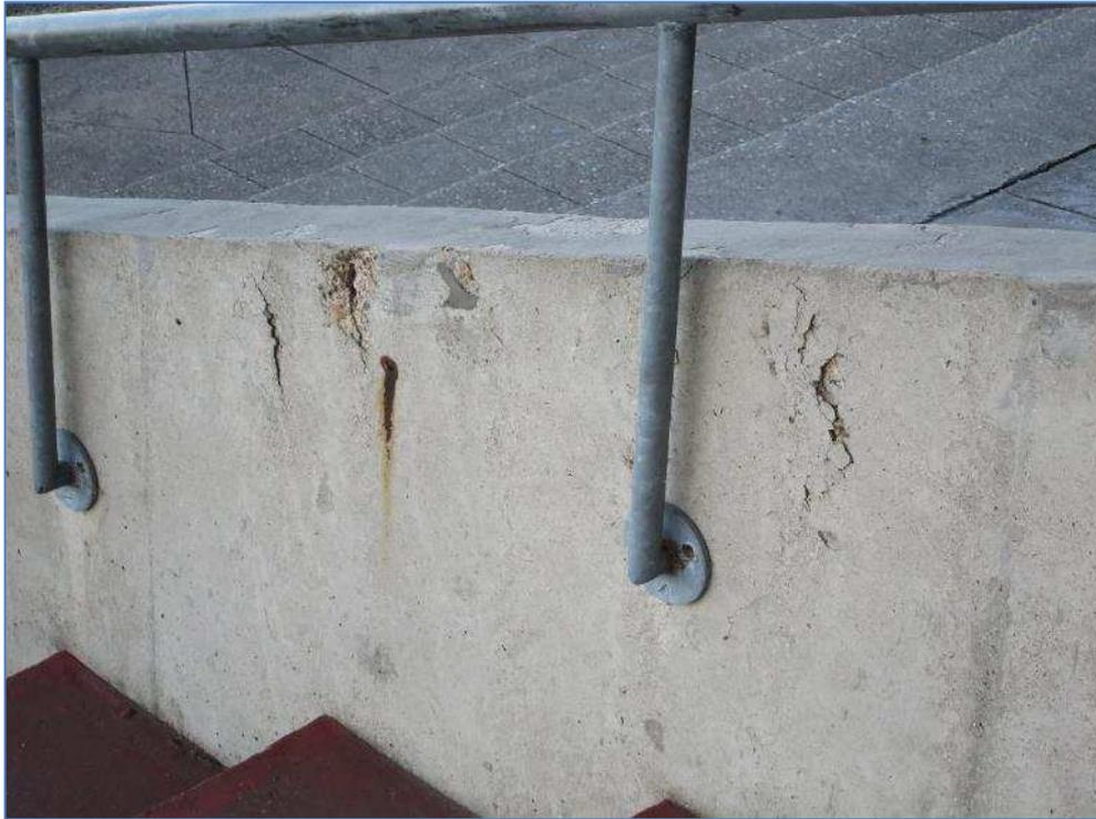
7-46 Concrete spalling on vomitory wall
