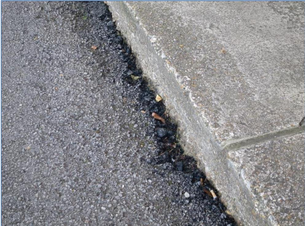
7-34 Gap between concrete steppings and asphalt
