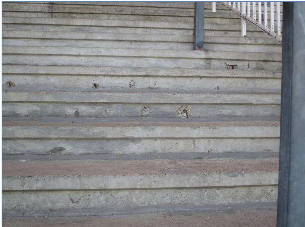
7-36 Concrete spalling on front terrace
