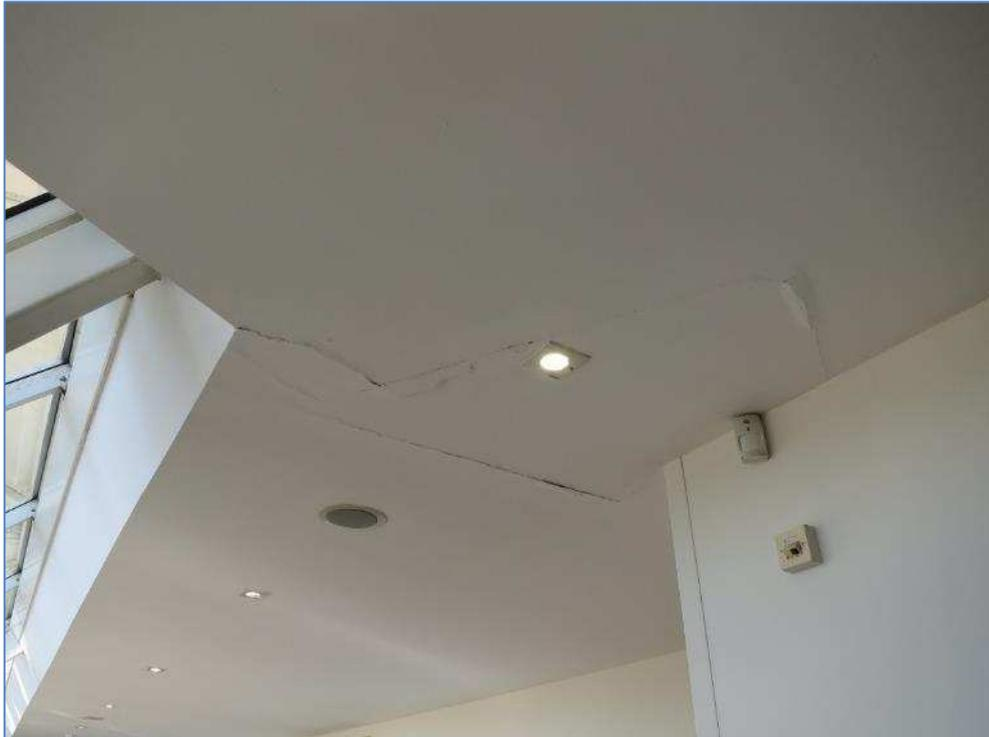
7-30 Cracks in ceiling in corridor
