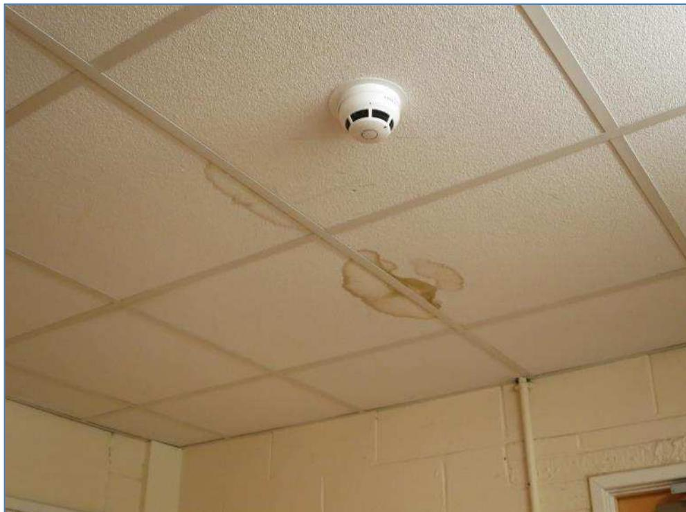
7-21 Water damage to ceiling in switch room lobby
