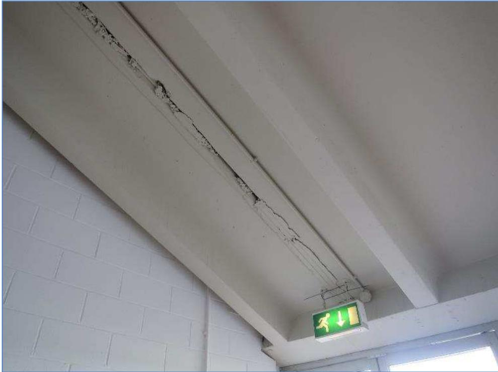
7-26 Infills between precast concrete units partly spalled
