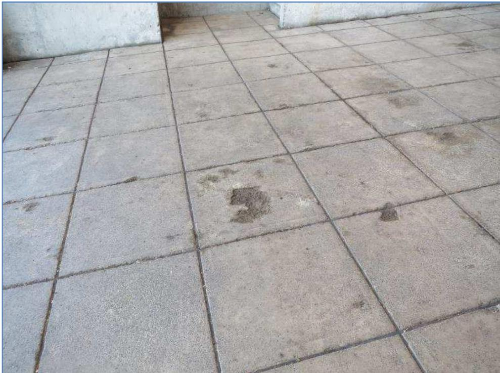
7-45 Top surface of paving slabs spalling
