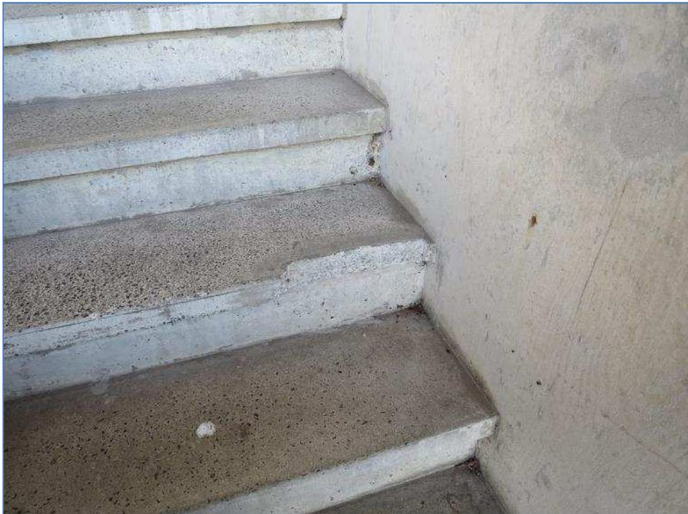
7-47 Section of concrete step spalled
