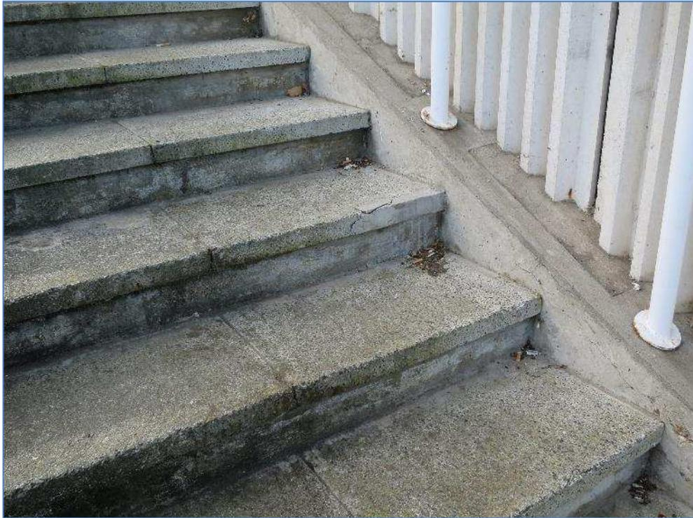
7-50 Concrete repair failing
