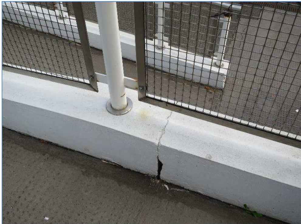
7-54 Cracks in concrete wall to ramp
