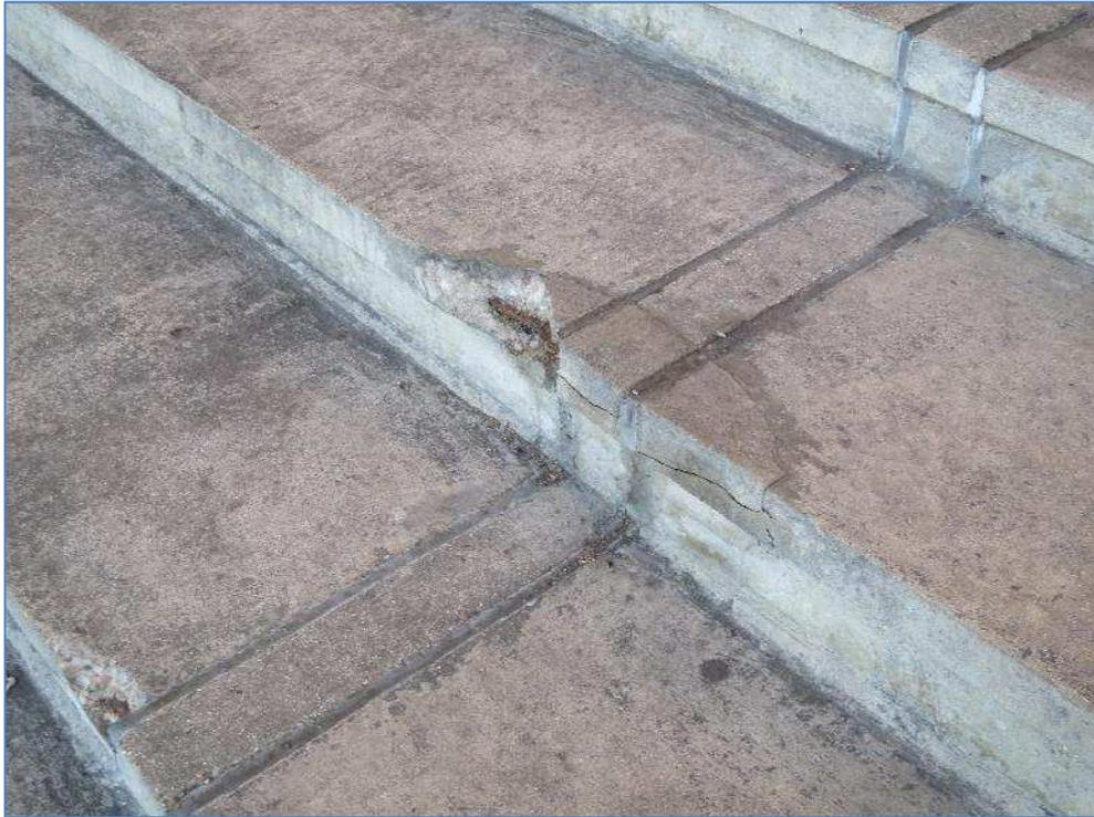
7-38 Concrete spalling on front terrace
