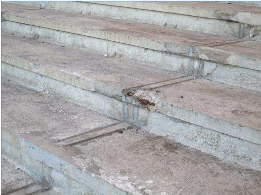
7-39 Concrete spalling on front terrace
