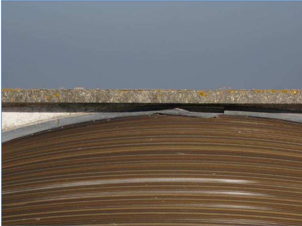
7-16 Flashing to polycarbonate roofing working loose
