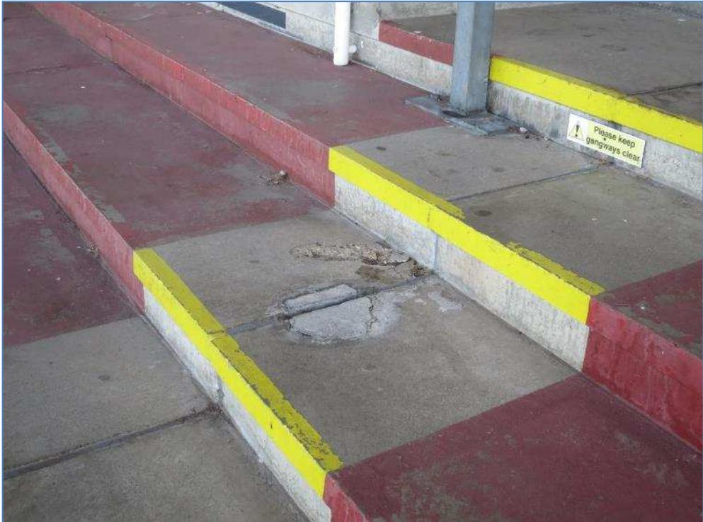
7-35 Concrete spalling on front terrace
