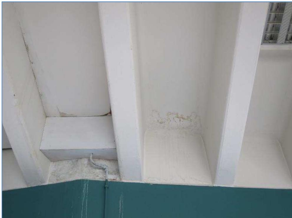
7-25 Damp damage to ceiling in Sports Bar
