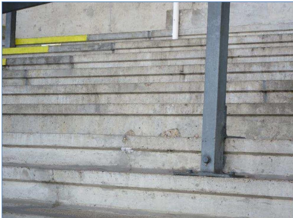
7-37 Concrete spalling on front terrace
