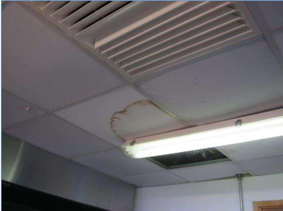
8-09 Water damage to ceiling in kitchen
