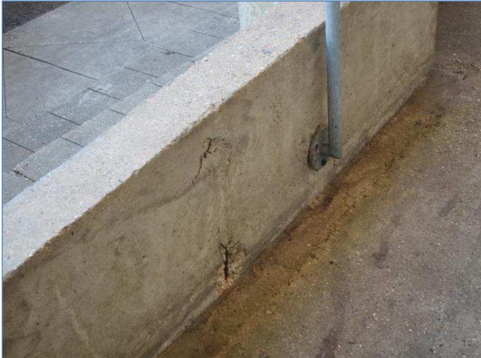
7-44 Concrete spalling on wall to disabled viewing
