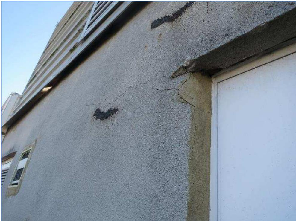
7-17 Minor cracks in render to service tower
