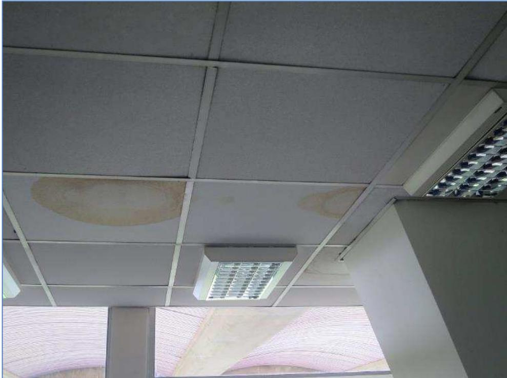
7-32 Damp damage to ceiling in press box
