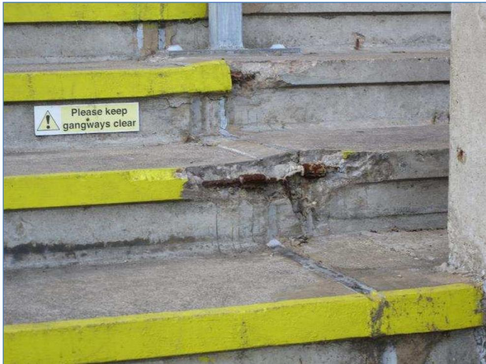
7-40 Concrete spalling on front terrace
