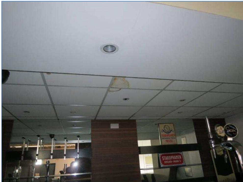
7-28 Damp damage to ceiling in Chasers Bar
