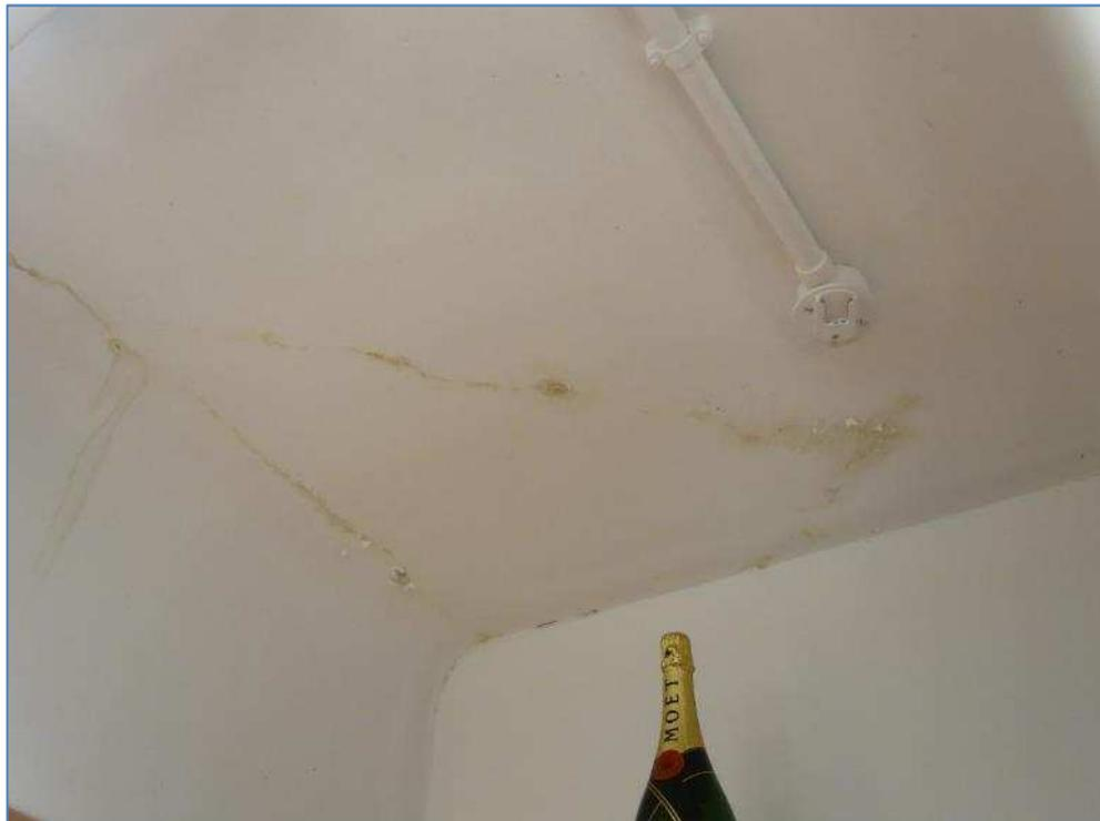
7-18 Damp damage to ceiling in Esher Hall bar
