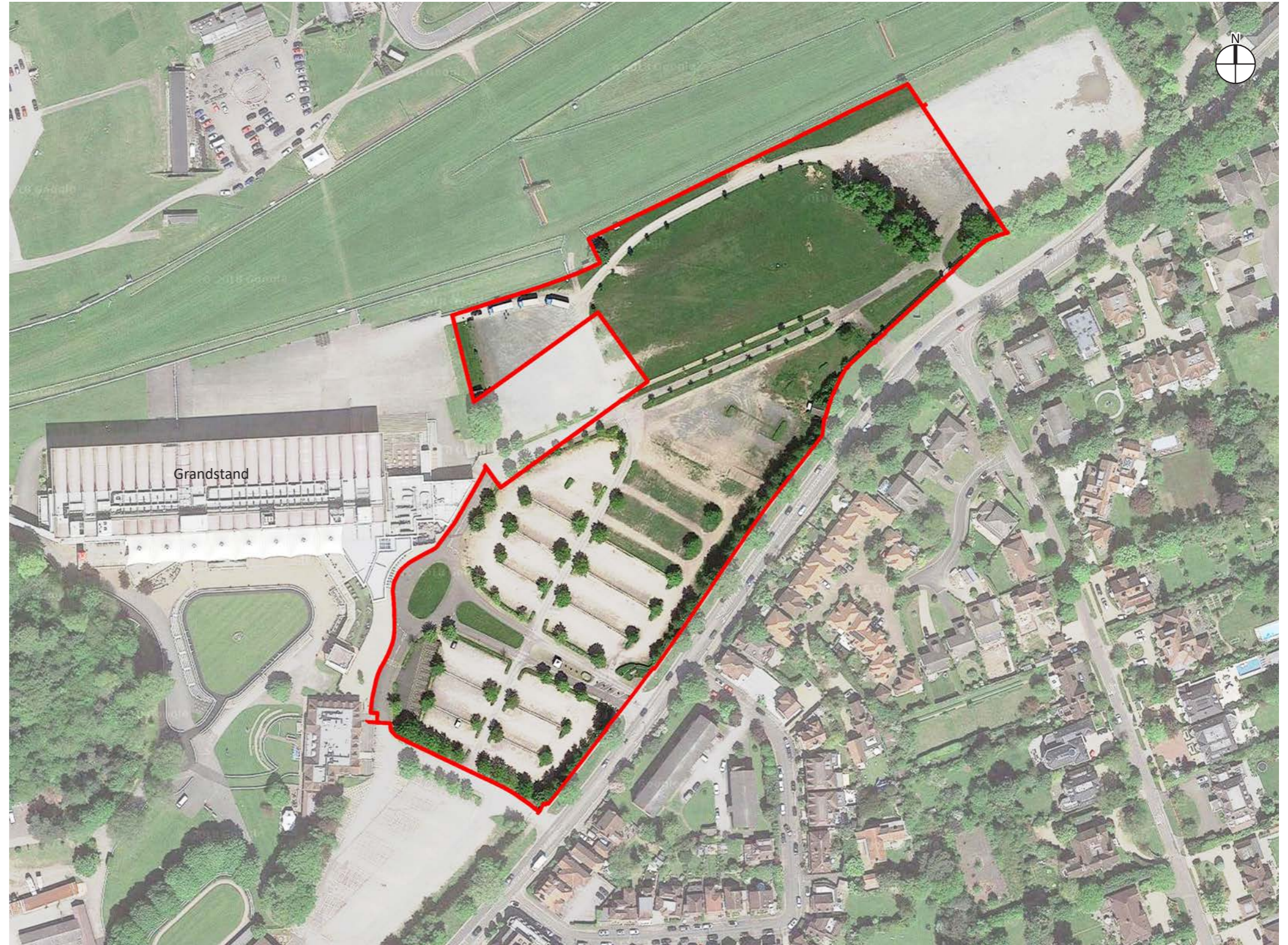
Fig. 17: Existing aerial view of Site F - Optimisation of the Car Park & main entrance frontage
