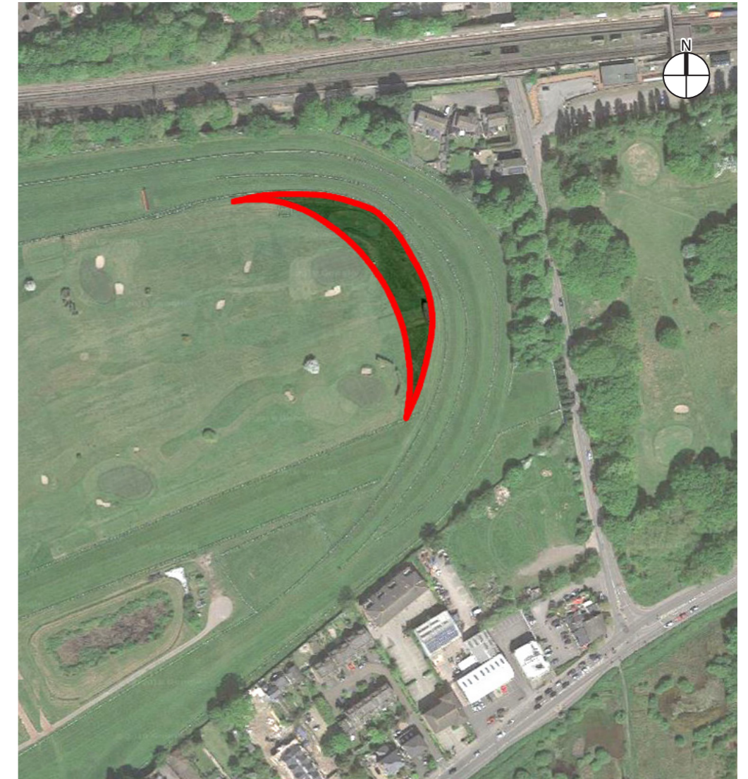
Fig. 16: Existing aerial view of Site E2 - Track Widening
