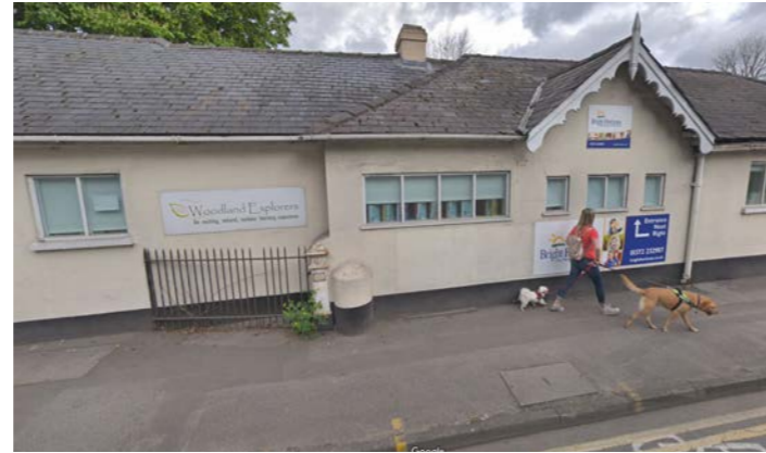
2 - Street view of nursery building and Grade II listed post on Portsmouth Road
