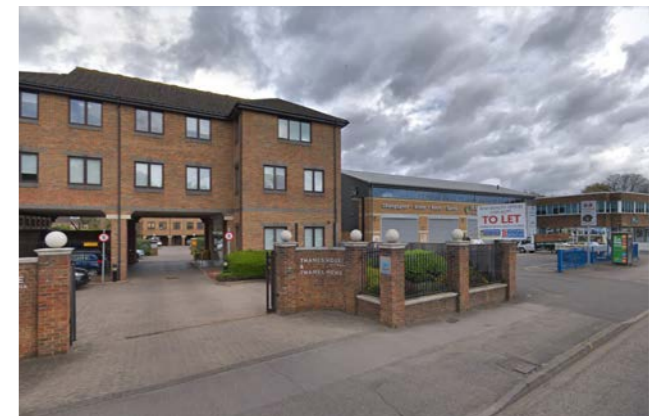
Photo 12 - Commercial buildings along Portsmouth Road
