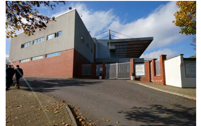
6 - View from within Site B towards the eastern end of the Grandstand
