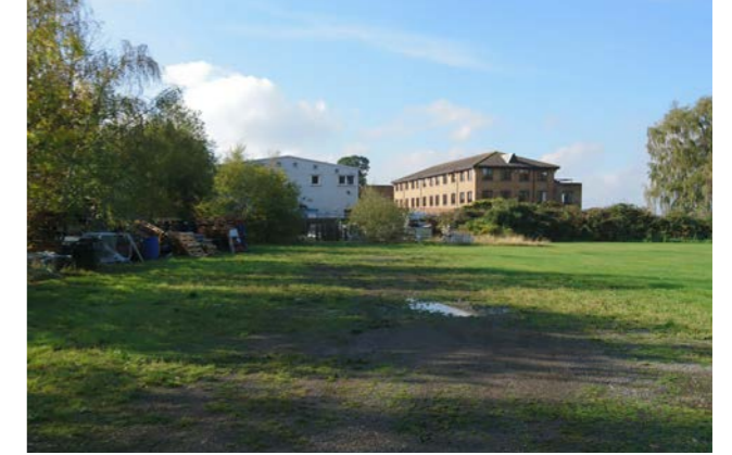
5 - View from within Site 4 towards Thames Mews offices
