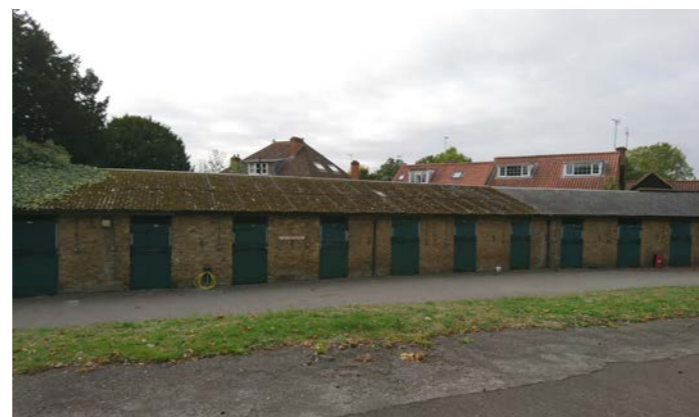
7 - View of the existing stables
