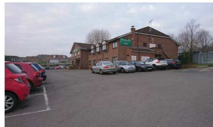
8 - View from within Sandown Park towards the Lodge
