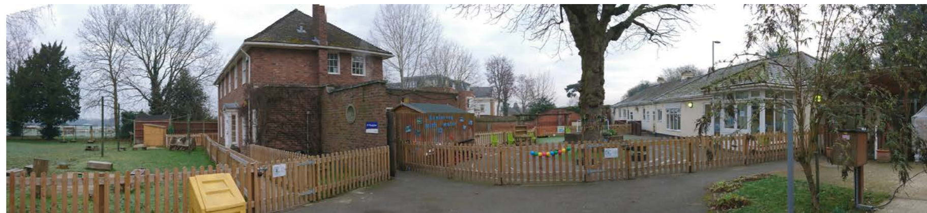
8 - View from within Site 5 towards existing Nursery building
