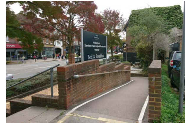
3 - Step and Ramp access from the pedestrian entrance down to the High Street
