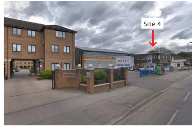
1 - Street view of adjacent buildings to Site 4 along Portsmouth Road
