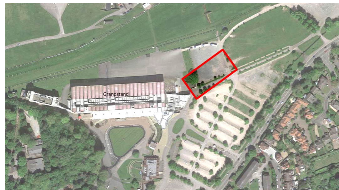
Fig. 20: Existing aerial view of Site B - Hotel
