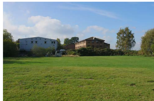
6 - View from within Site 4 towards Thames Mews offices
