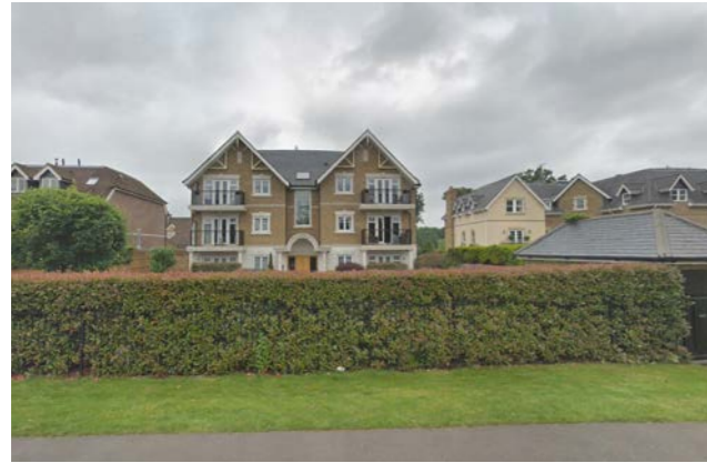
1 - Street view from More Lane, adjacent to Site 3, illustrating the built form close to the site.
