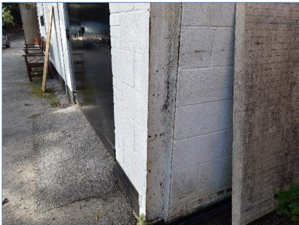
5-42 Paint peeling from steel frame of maintenance workshop
