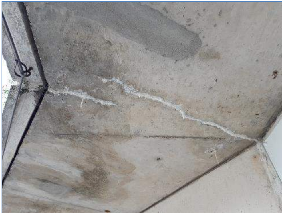
7-08 Areas of leaching on soffit of viewing terrace
