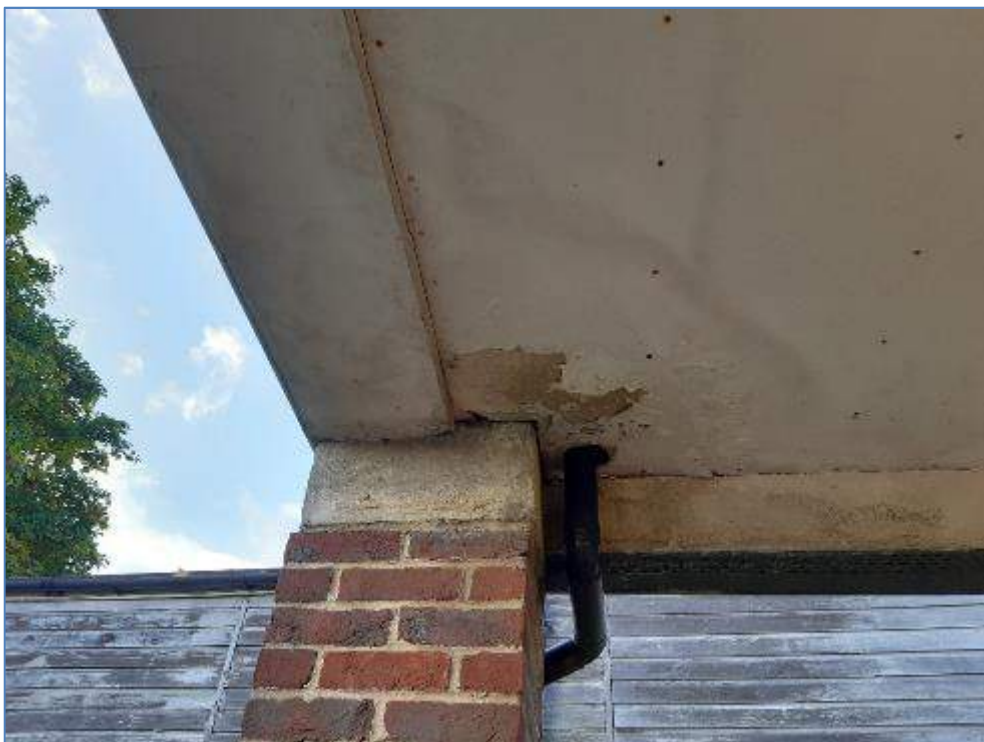
3-04 Water damage to soffit of carport
