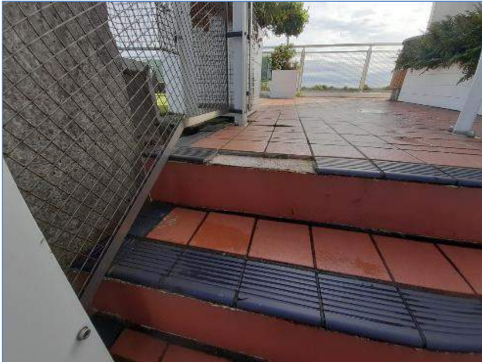
7-04 Tiles missing at top of stair to terrace
