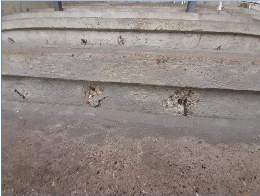
7-34 Vertical sections of front terrace steppings spalling
