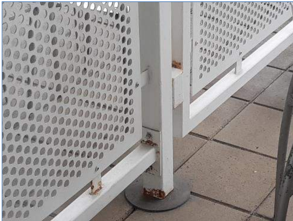
8-08 Rust at base of dividing barriers on balconies
