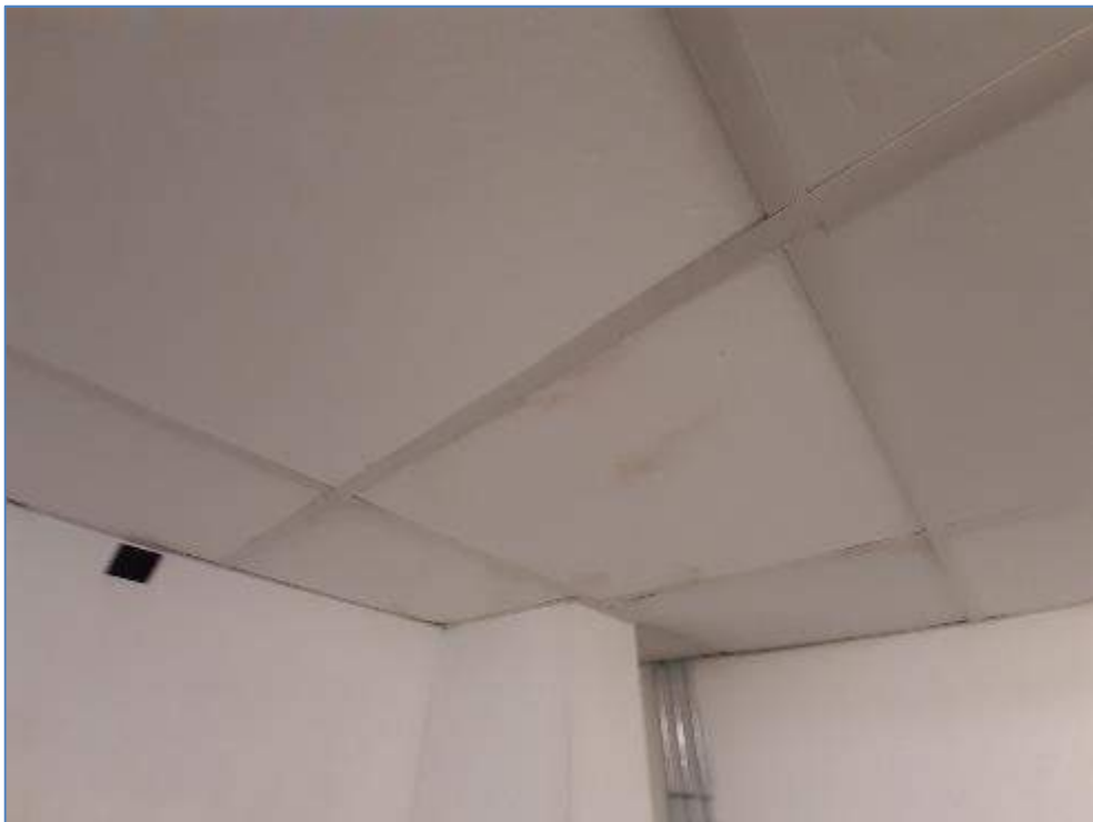
8-03 Minor damp in kitchen ceiling
