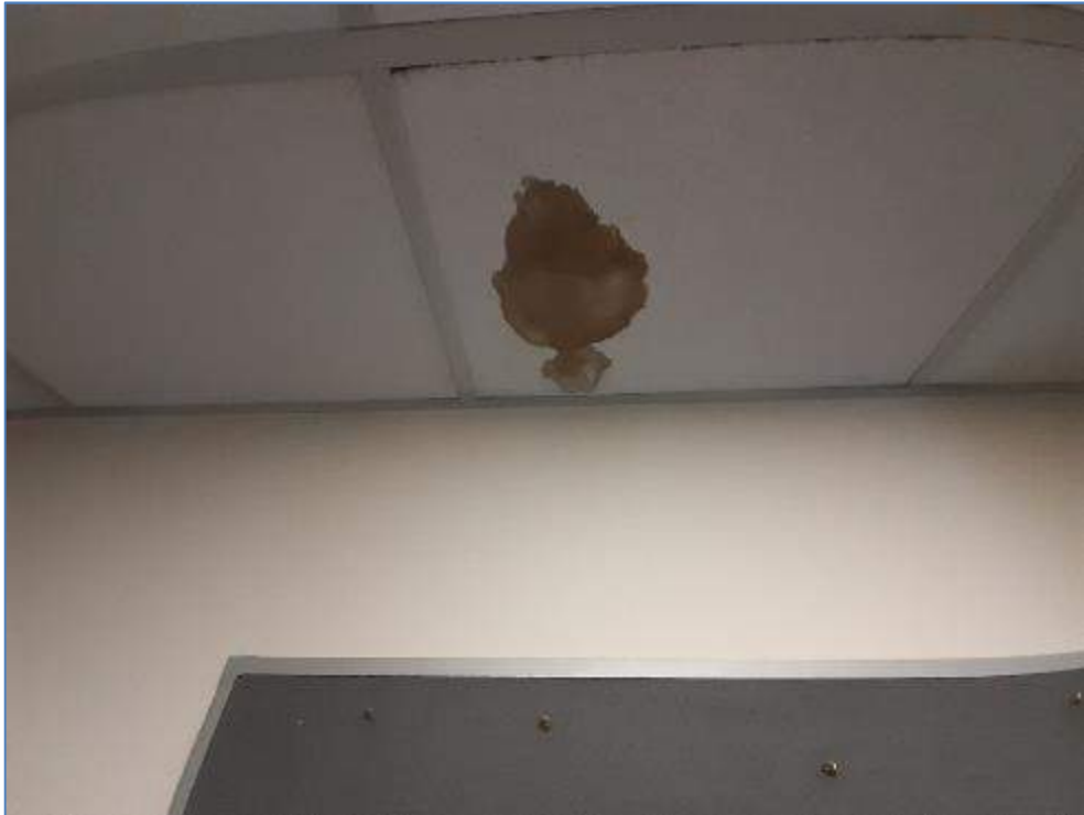
7-22 Minor damp in ceiling of organisers office
