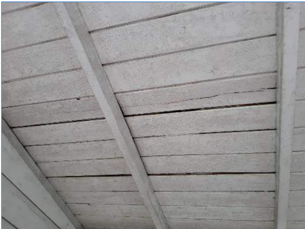
6-04 Timber soffit boards warping in some places
