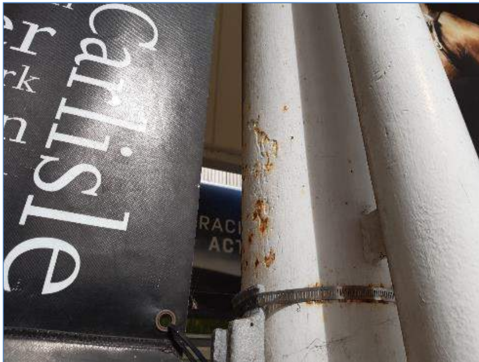
7-06 Minor surface rust to steel frame
