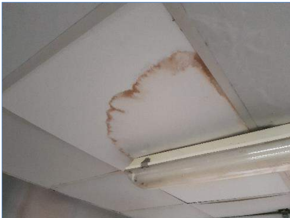
8-09 Water damage to ceiling in kitchen
