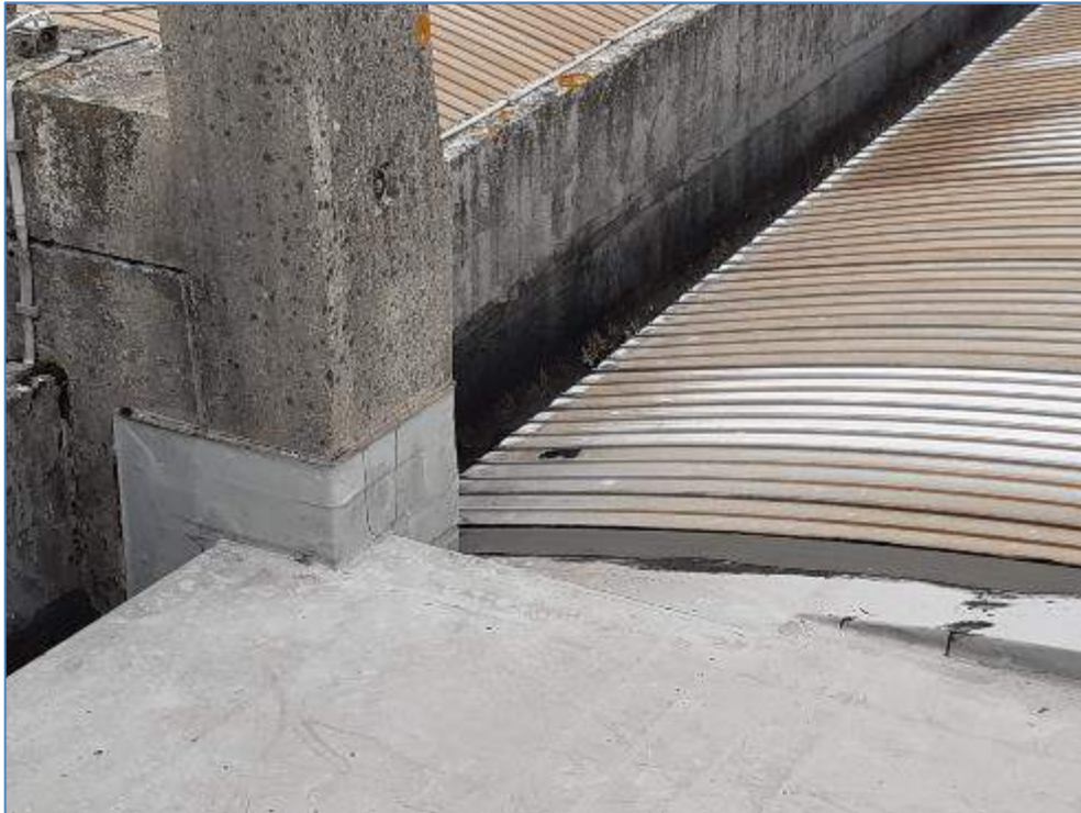
7-16 Some sections of roof infill panels damaged
