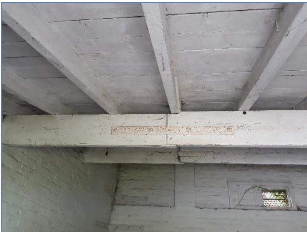
5-30 Surface rust to tie straps on timber beams
