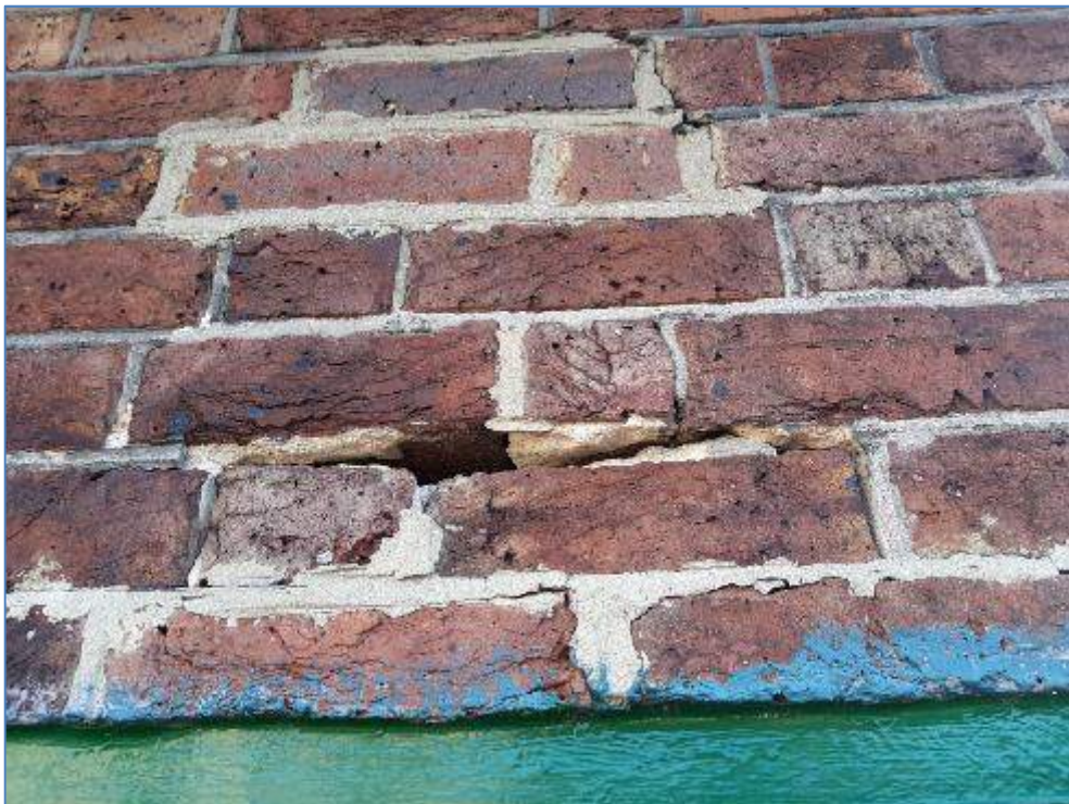
5-04 Loose bricks and cracking over stable manager door
