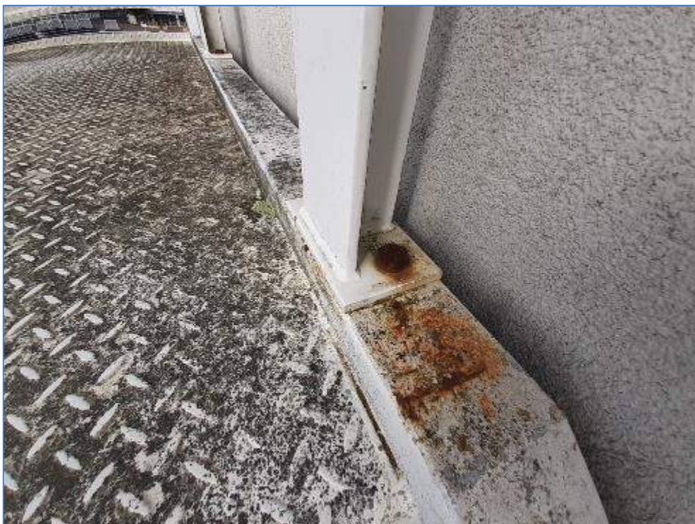
7-05 Bolts rusting on steel stair handrails
