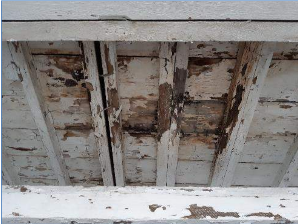
5-33 Timber soffit boarding rotting heavily in stable 46
