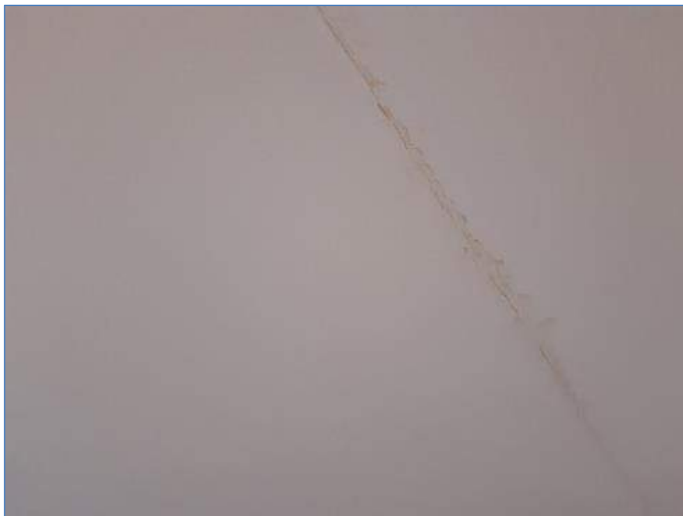
4-11 Minor damp in ceiling of offices
