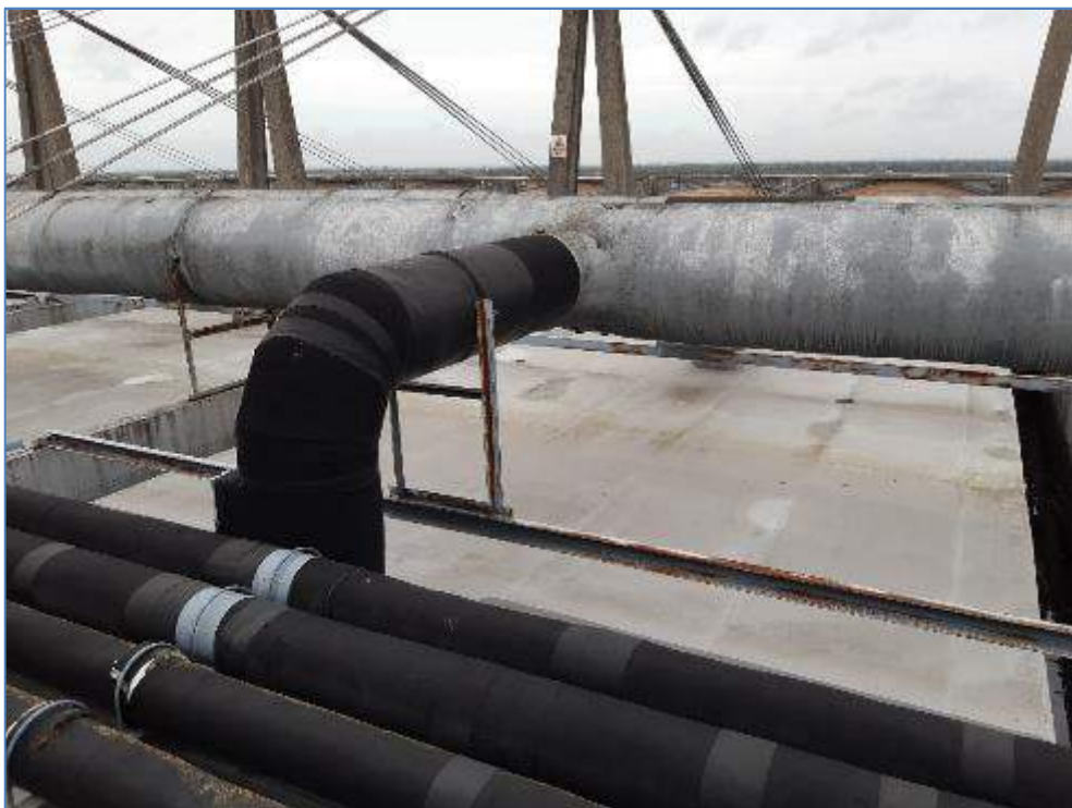
7-15 Secondary steelwork for plant equipment is rusting
