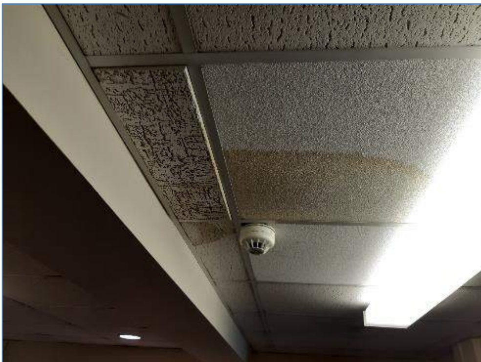
4-09 Water damage in ceiling of Stewards Room
