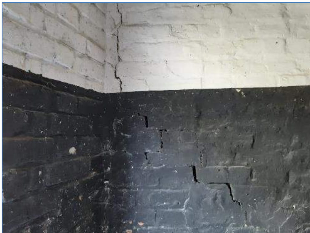
5-26 Crack in dividing wall of stable 17 and the tack boxes
