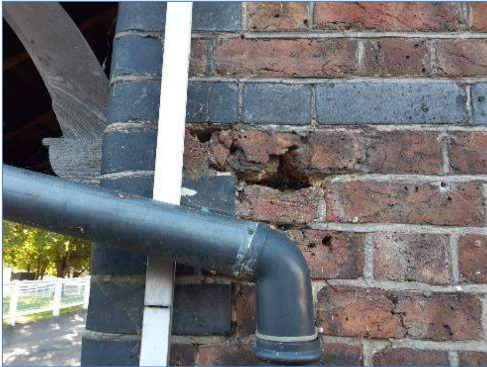
5-07 Damaged brickwork on external corner of veterinary block
