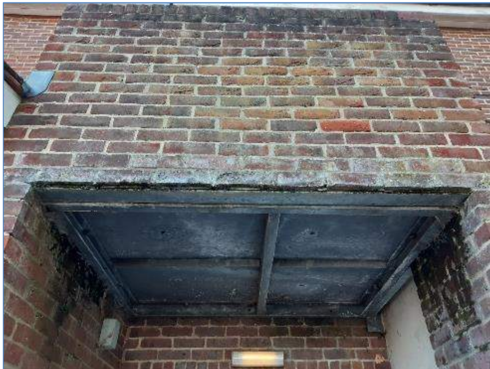
3-01 Bricks spalling over side entrance
