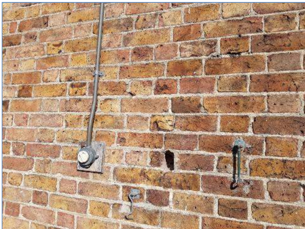
5-12 Damaged areas of brickwork
