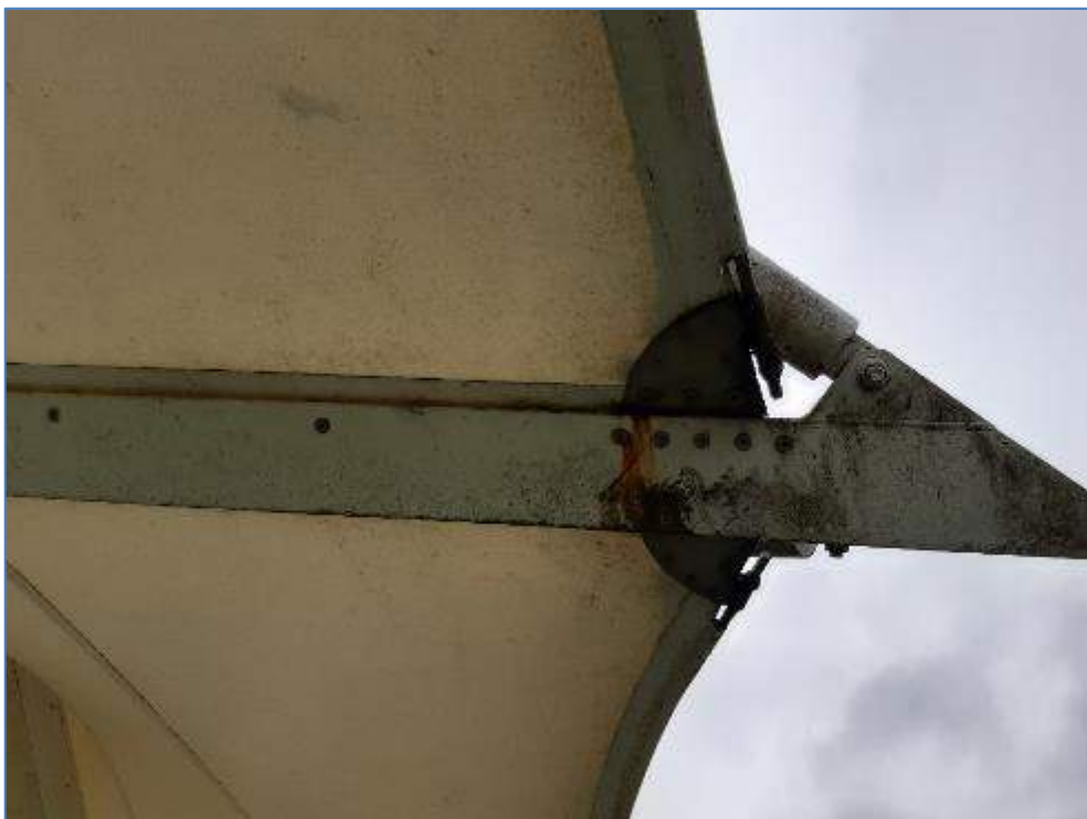
8-11 Surface rust to canopy support steel over balconies
