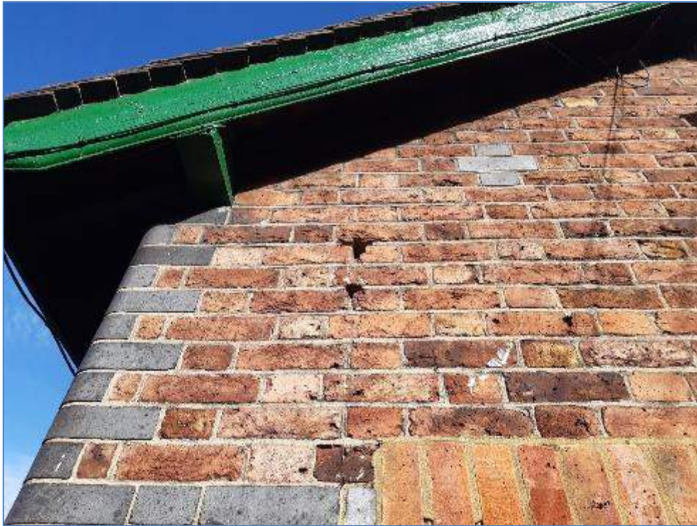
5-05 Bricks spalling on end wall
