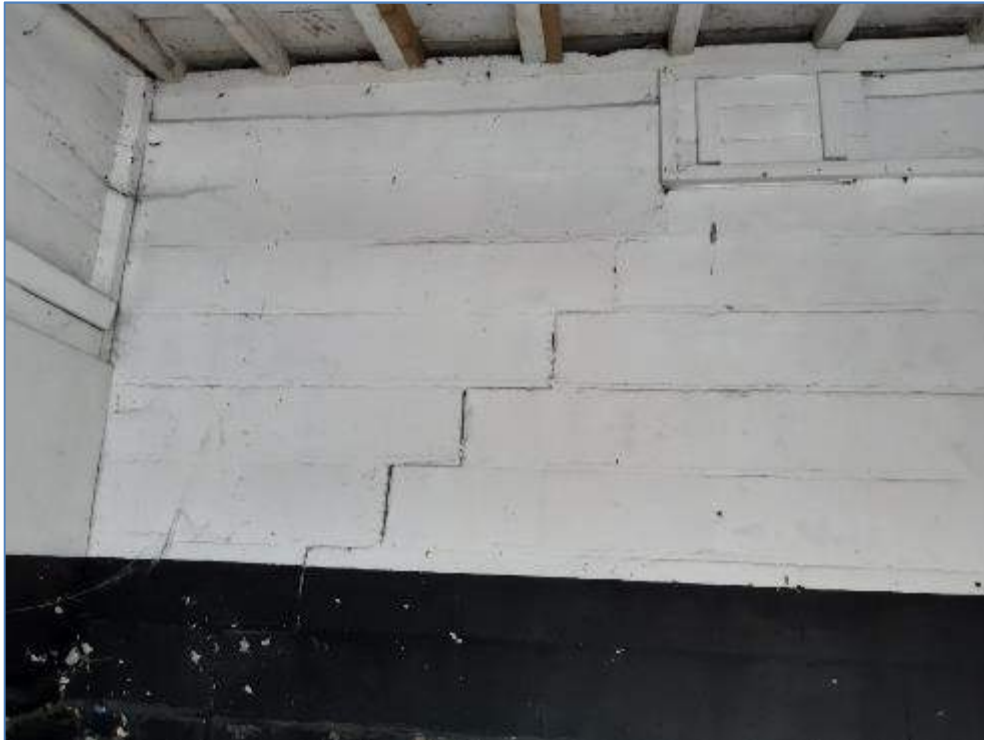
5-37 Diagonal crack in rear wall of stable 48
