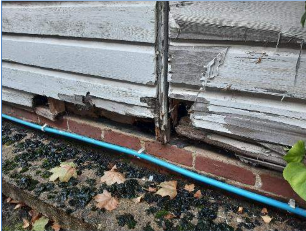
6-03 Timber cladding decaying heavily in places
