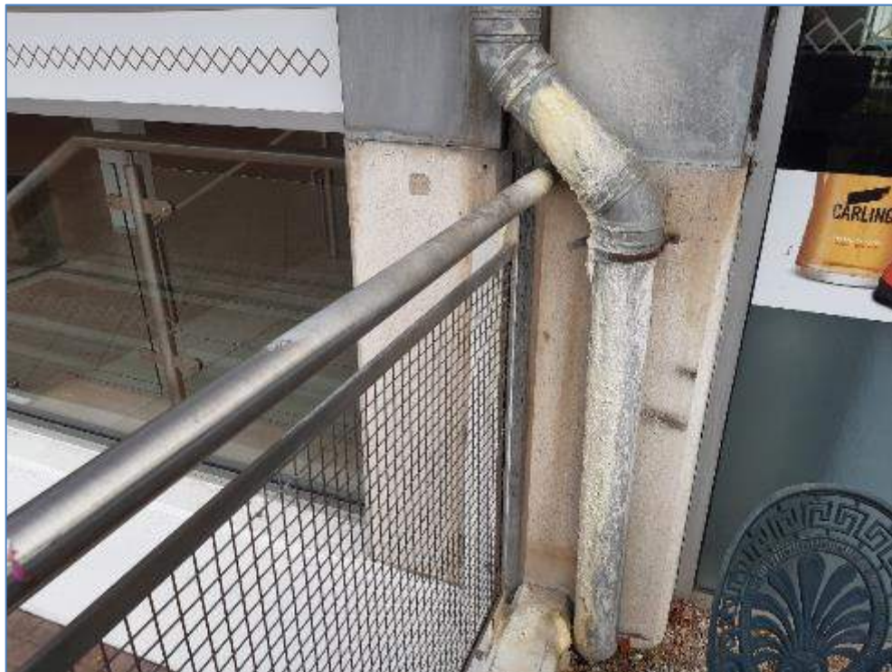
7-10 Substance leaking onto handrail and downpipe underneath terrace
