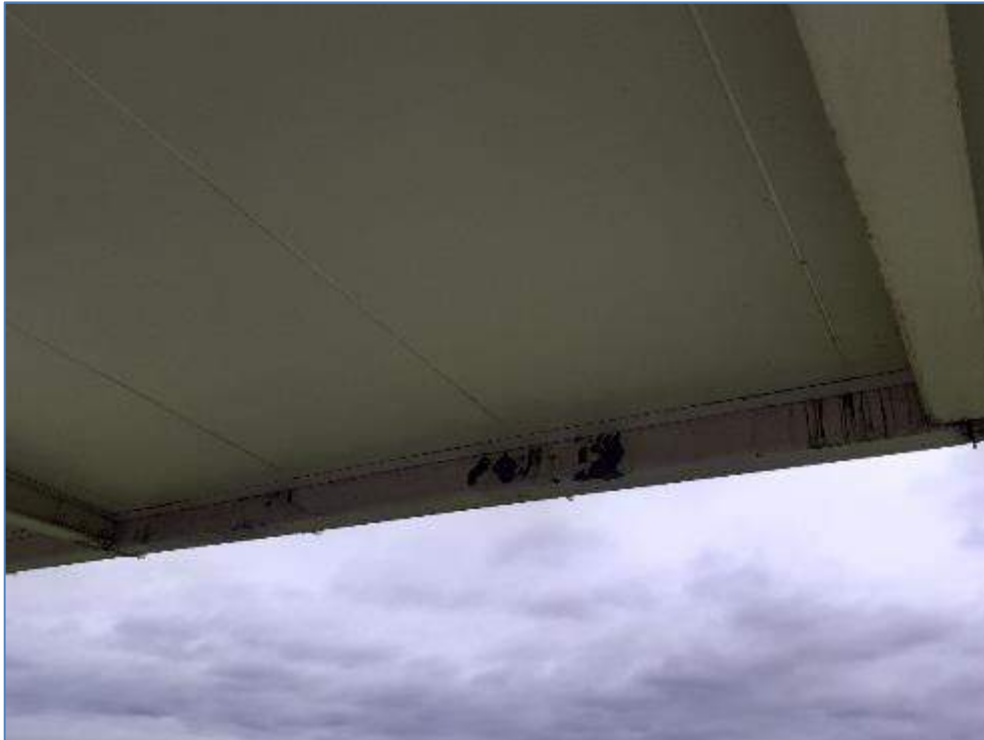
8-10 Minor surface rust to support steelwork over balconies
