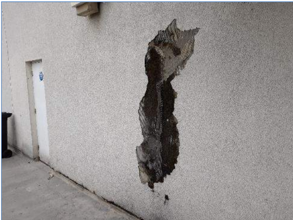
7-43 Section of wall render has spalled
