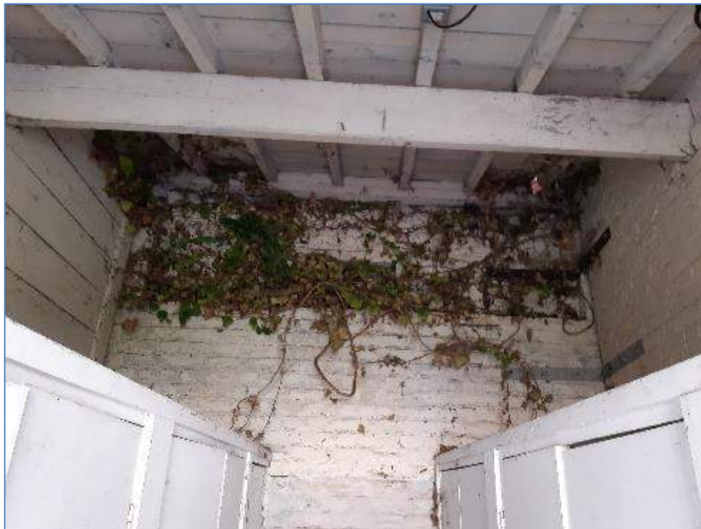
5-27 Plant growth to rear wall of tack boxes
