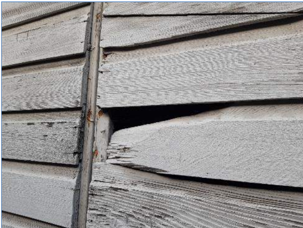
6-02 Timber cladding damaged in places
