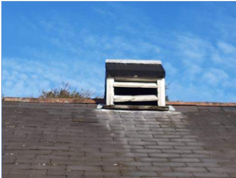
5-11 Roof vent boxes breaking up
