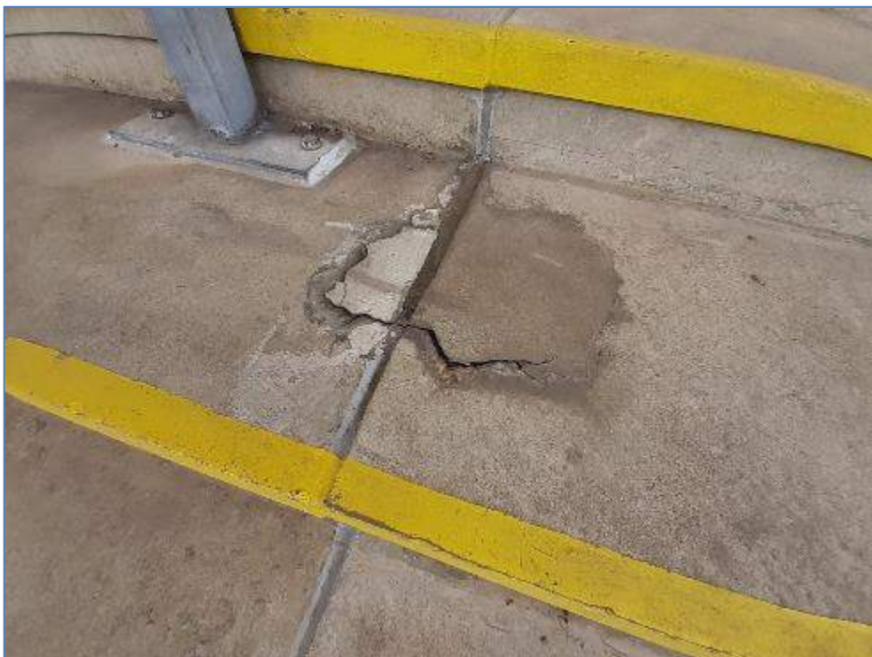
7-29 Concrete spalling on front terrace
