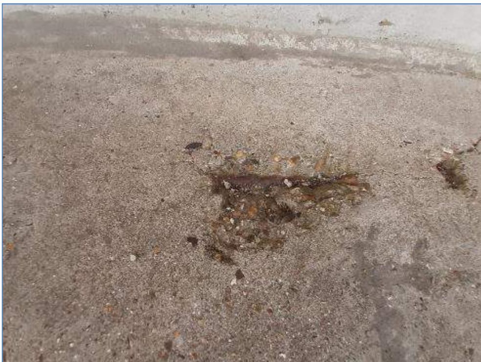
7-31 Concrete spalling on front terrace
