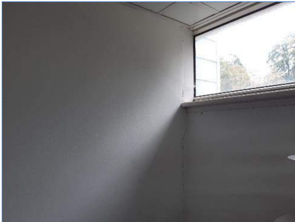
8-12 Crack in corner of kitchen
