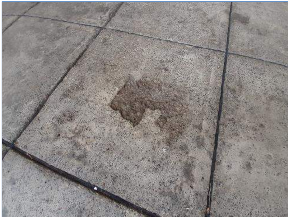
7-40 Top surface of paving slabs spalling
