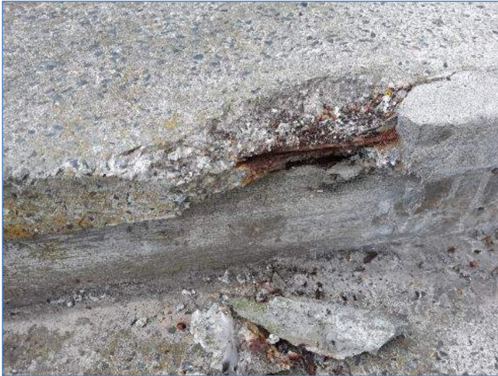
7-42 Concrete spalling on steps, exposing rebar
