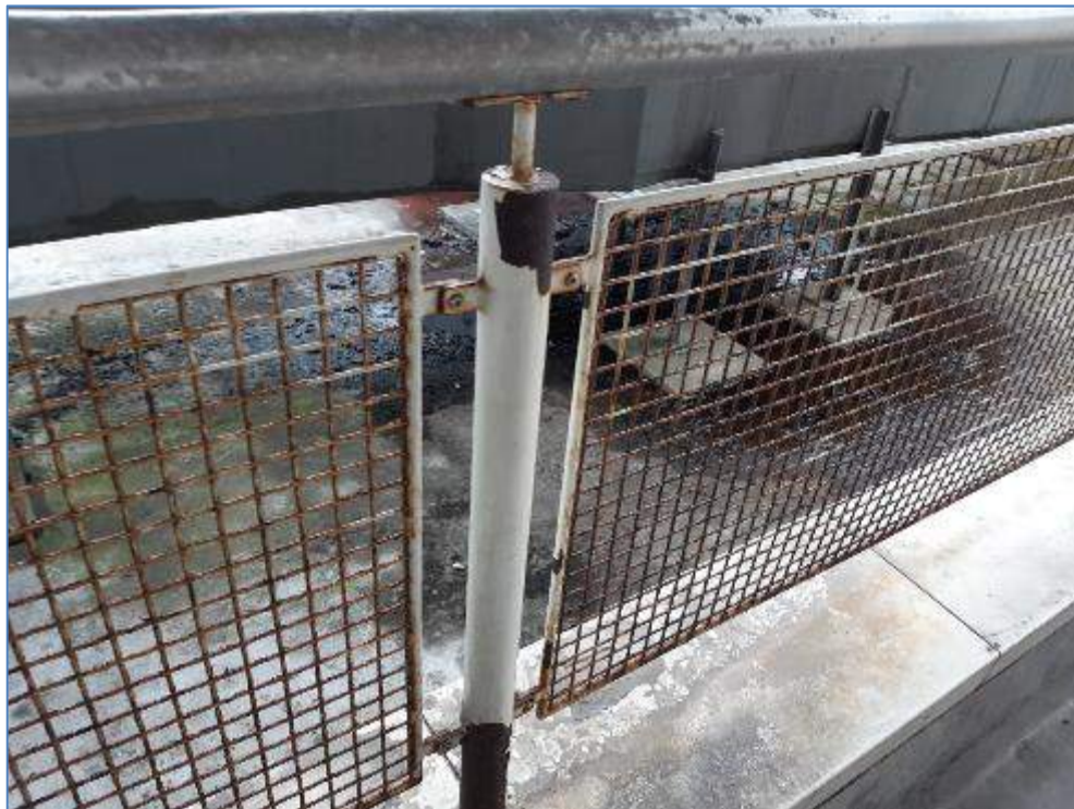
7-44 Balustrades and infill panels corroding
