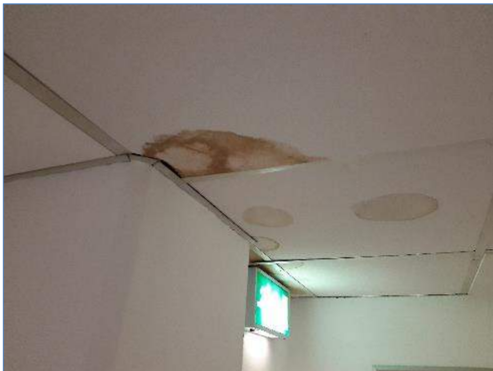
7-25 Damp in ceiling of men's toilets
