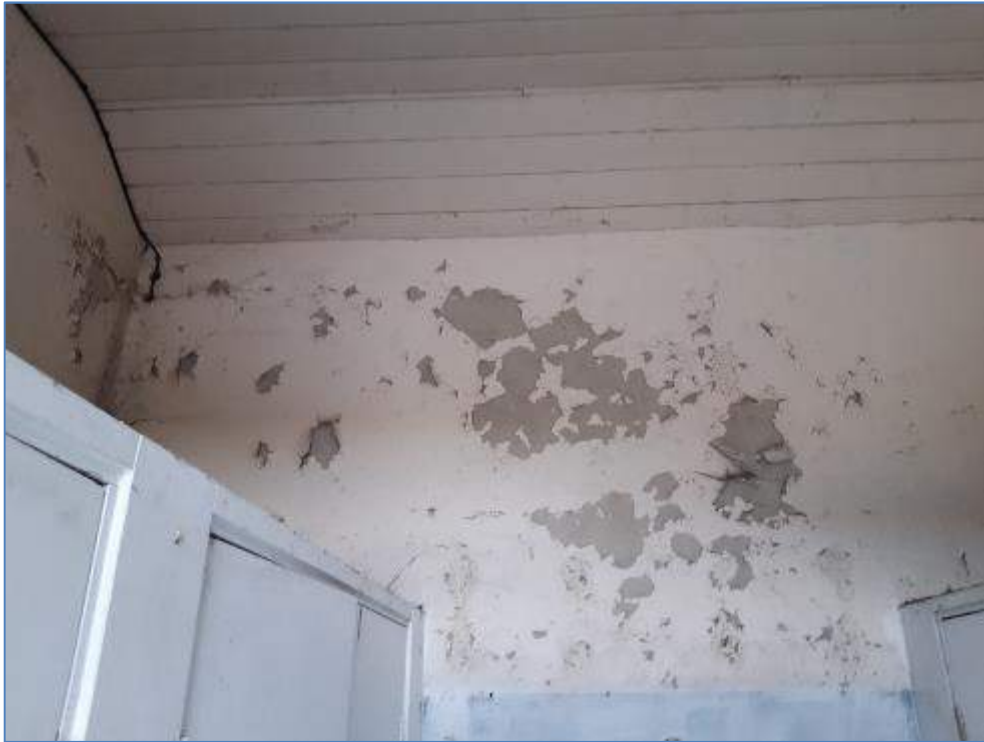
5-13 Paint peeling from walls by tack boxes
