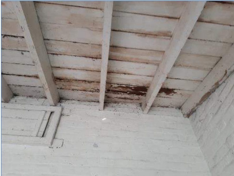
5-17 Timber soffit boards decaying in several places
