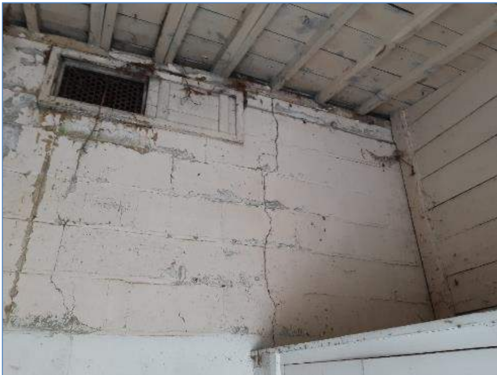
5-35 Cracks in rear wall of tack boxes
