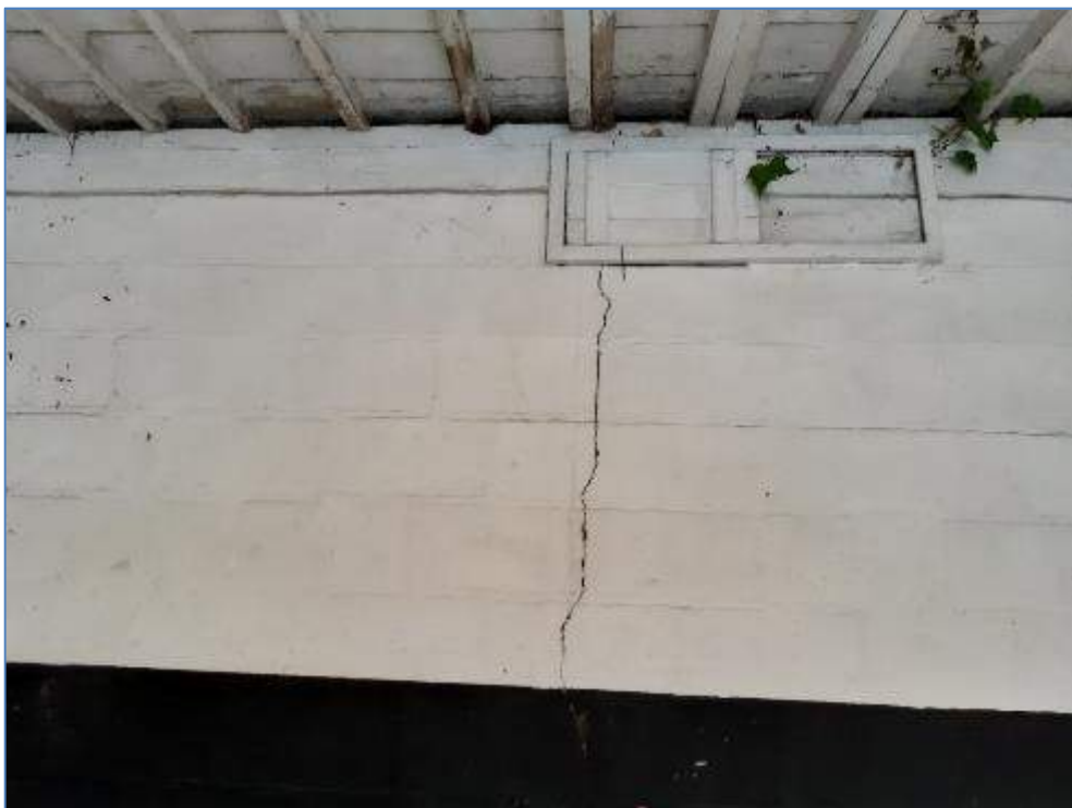
5-36 Vertical crack in rear wall of stable 52
