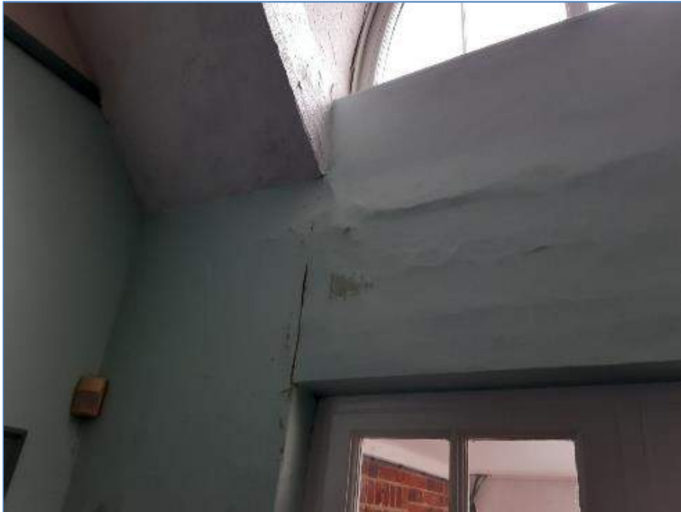
4-08 Cracking and damp damage over door
