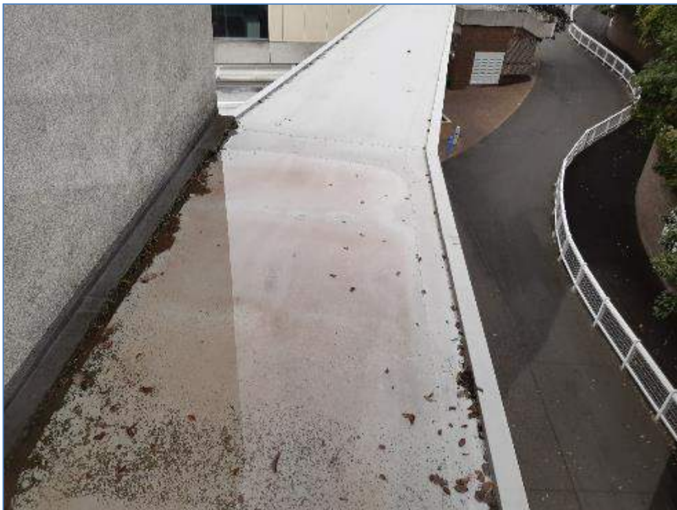
8-19 Water ponding on roof of link bridge
