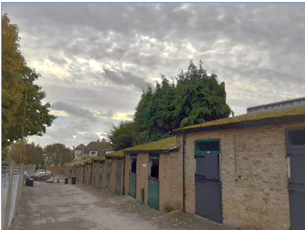
5-38 Heavy moss growth on stable roofs
