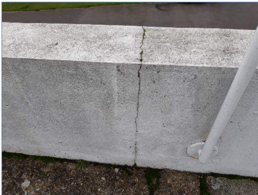
7-47 Cracks in concrete wall to steps
