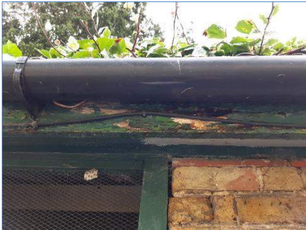
5-25 Timber eaves board decaying
