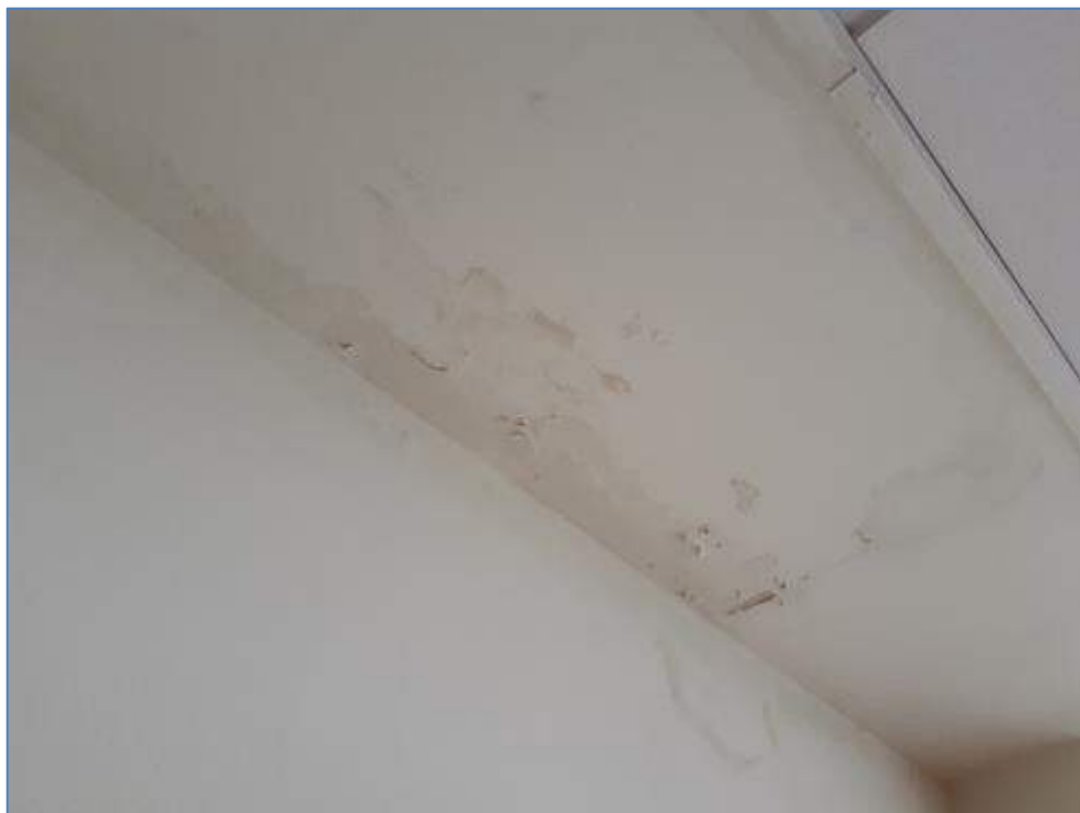
8-13 Damp in ceiling of box 3.3
