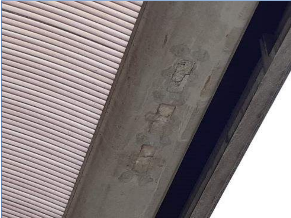
7-14 Concrete spalling from roof beams
