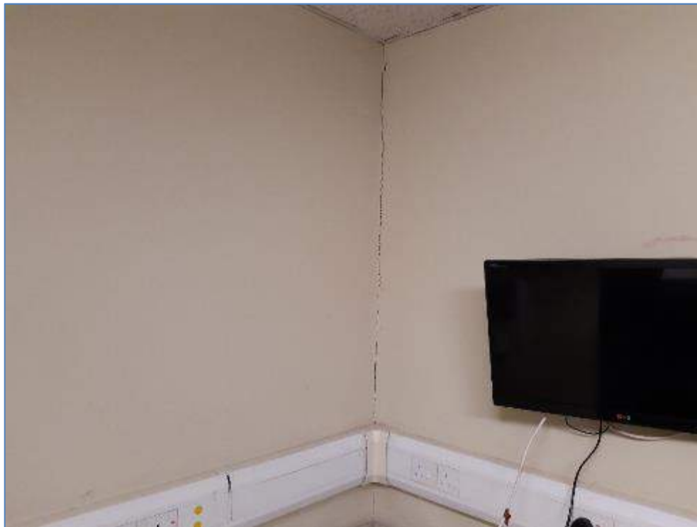
4-10 Minor crack in corner of Broadcast office
