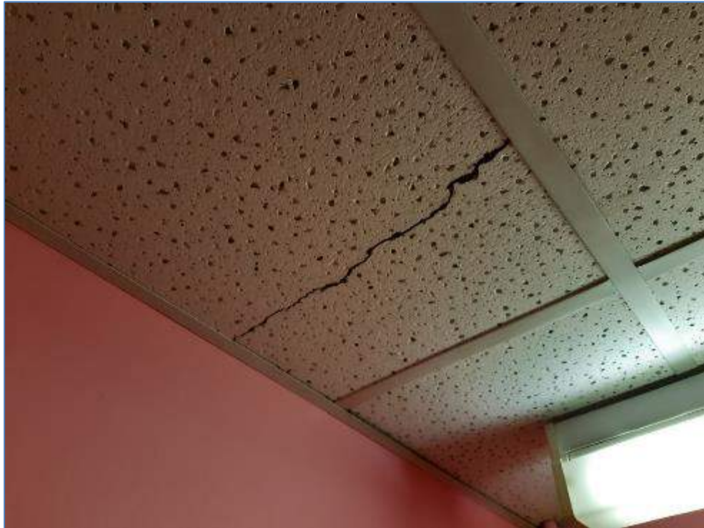
3-07 Crack in ceiling of female toilet
