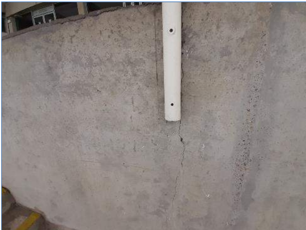
7-37 Crack in rear dividing wall
