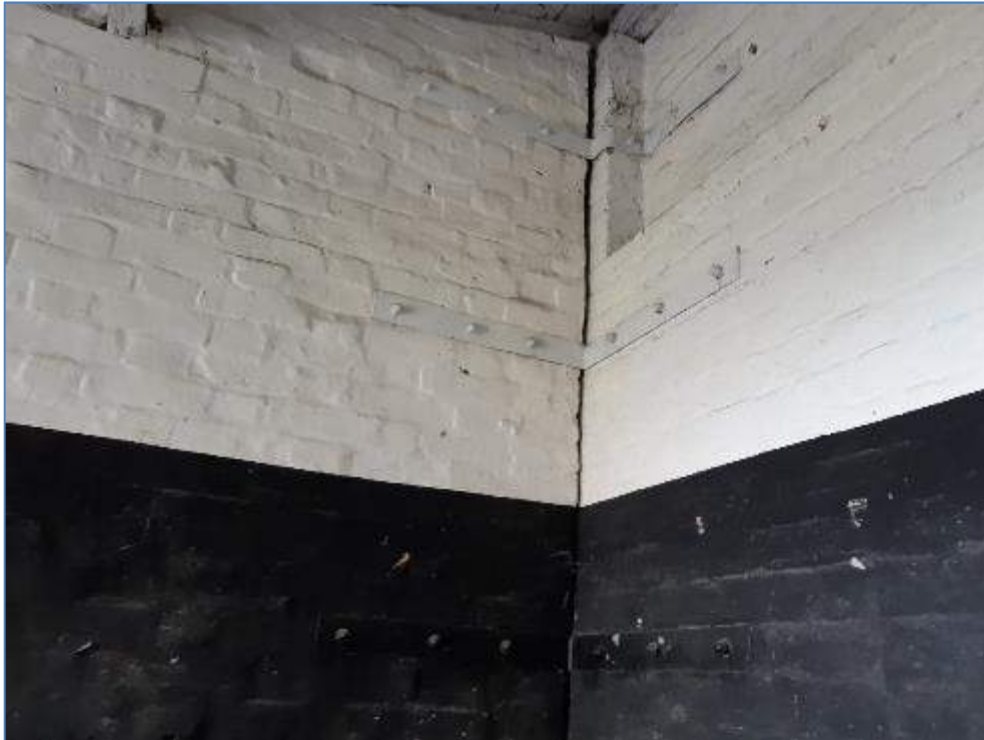
5-29 Cracking in corners of stables, restraint straps have been installed previously
