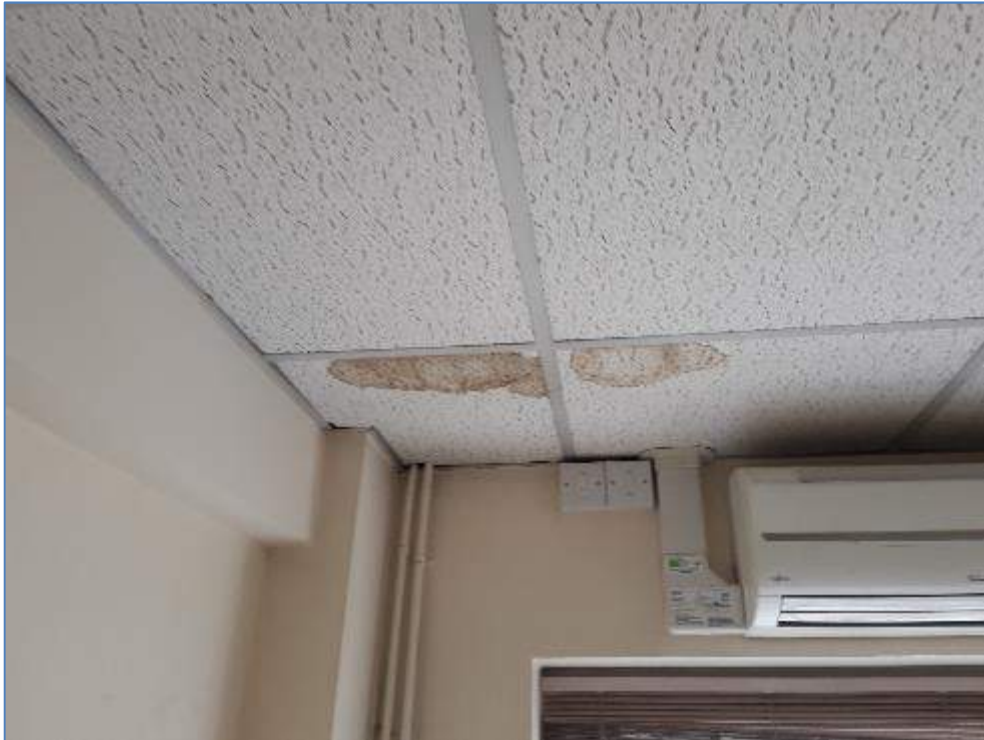
4-04 Damp damage to ceiling in offices
