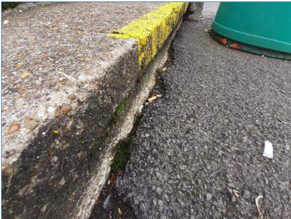
7-27 Gap between concrete steppings and asphalt
