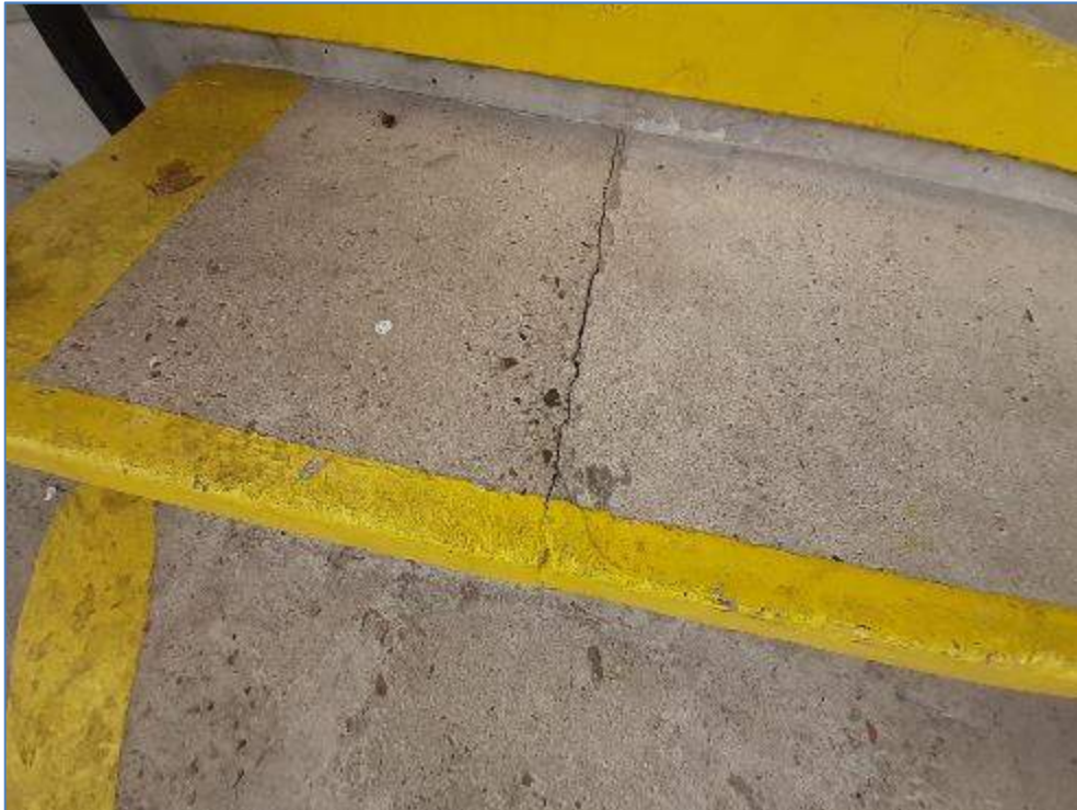
7-36 Cracking in front seating terrace steppings
