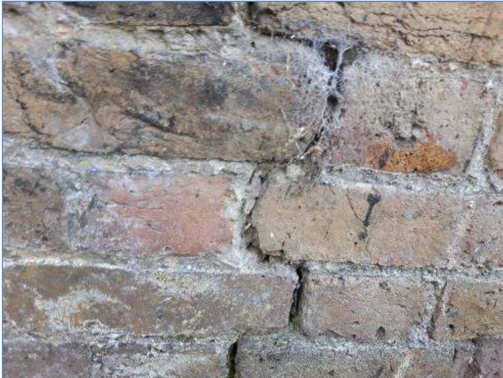
5-01 Cracks in brickwork to rear elevation
