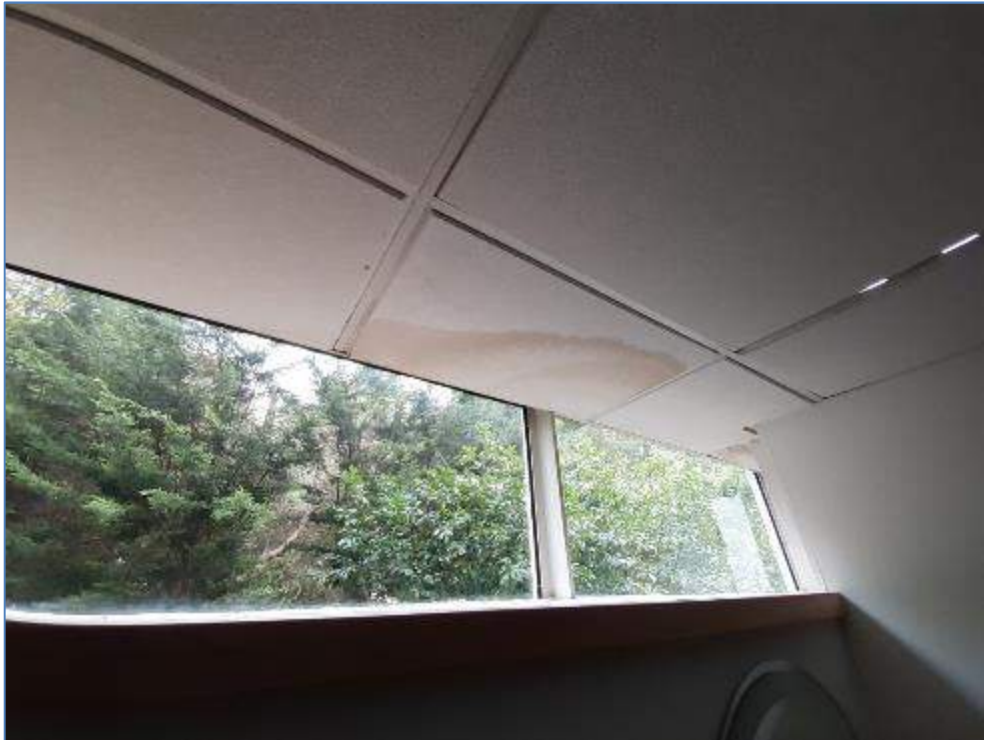
8-04 Damp in ceiling of male toilets
