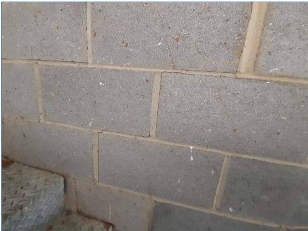
8-15 Cracking in block wall of stairs going up to roof
