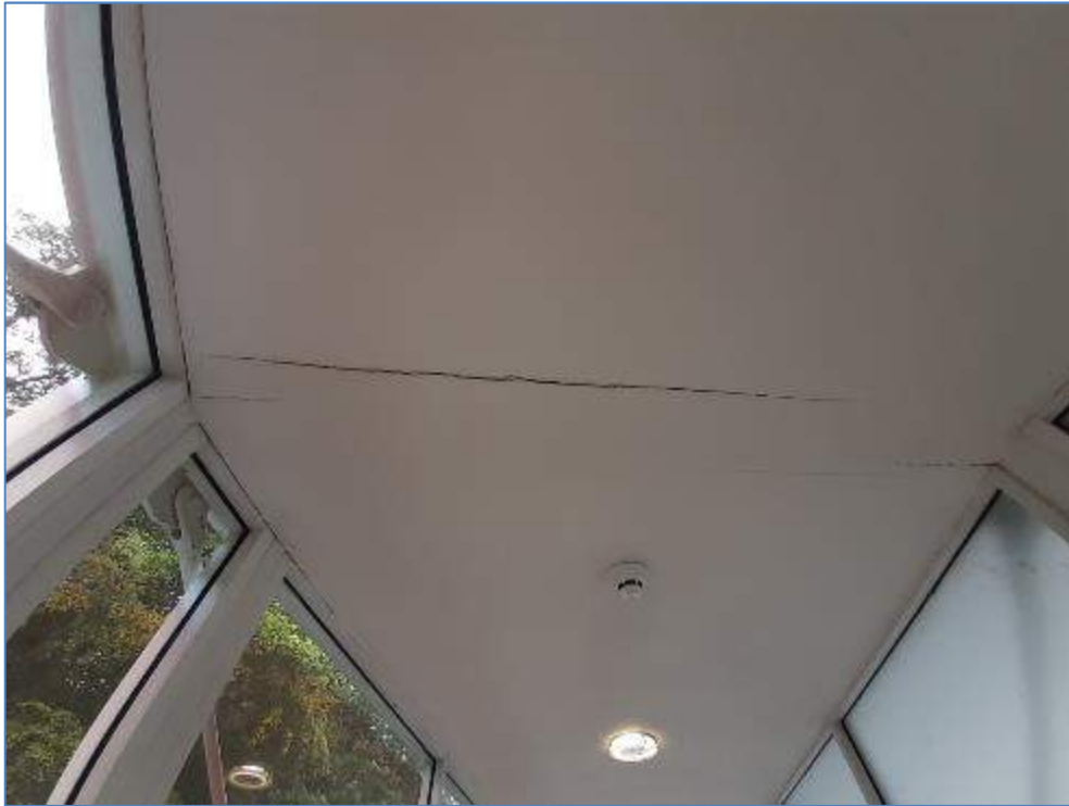
8-18 Cracking in ceiling of link bridge
