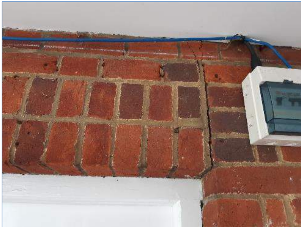
4-02 Crack in brickwork at end of lintel
