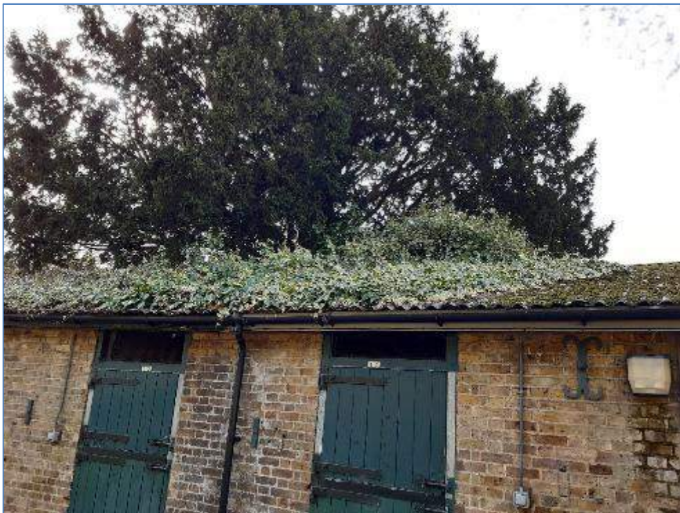
5-24 Heavy plant and moss growth on stable roofs
