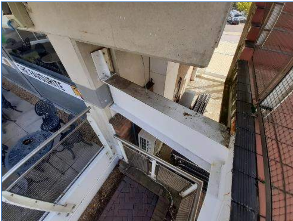
7-01 Minor spots of rust to steel frame of media centre
