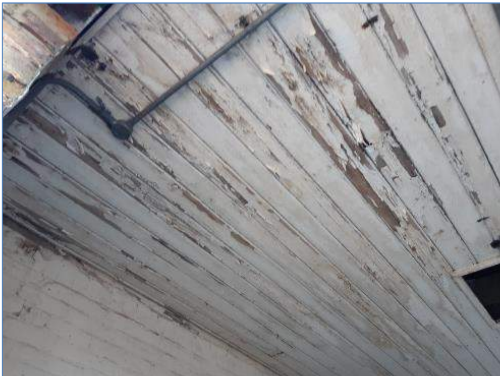
5-10 Timber soffit boards rotting in several stables
