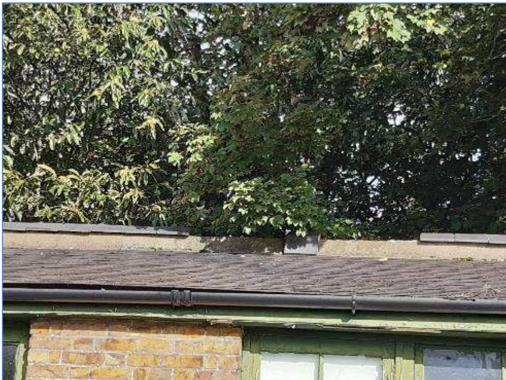
5-22 Copings missing from roof ridge
