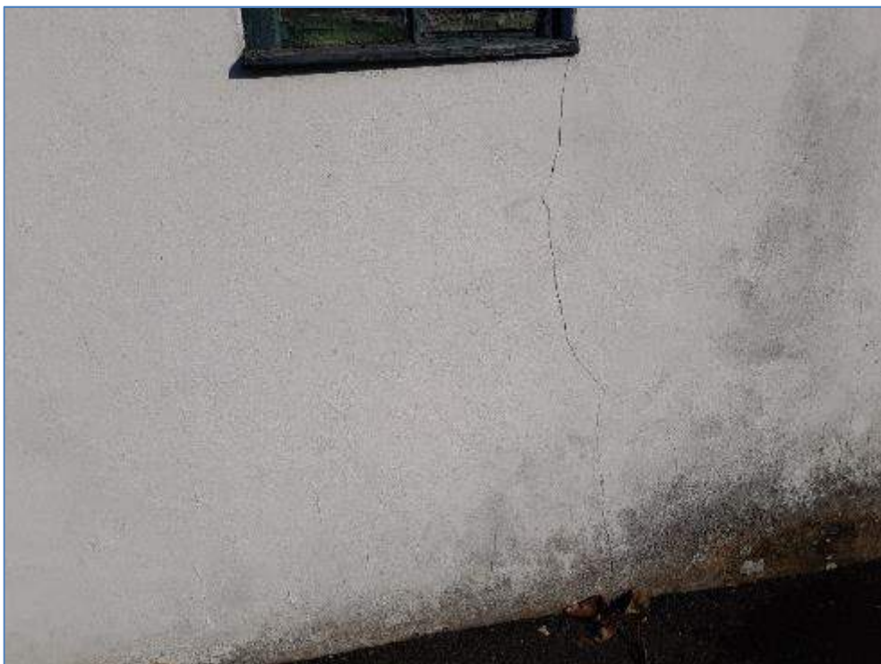
5-16 Cracking in external render
