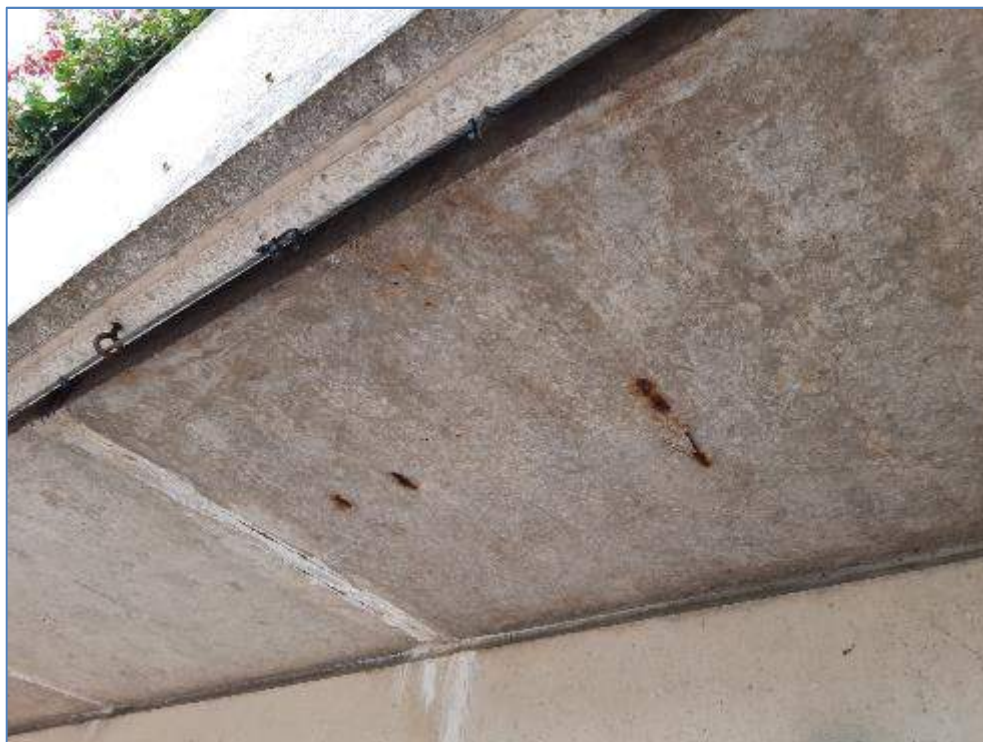
7-07 Concrete spalling on soffit of terrace, rebar can be seen corroding
