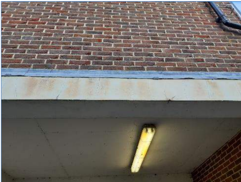
3-05 Cracks in lintel over carport
