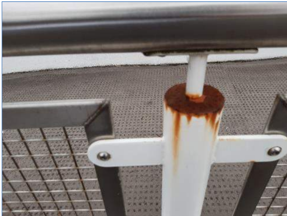
7-46 Surface rust to barriers
