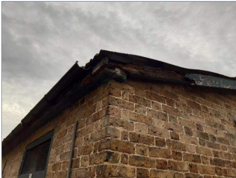
5-41 Timber fascia board decaying
