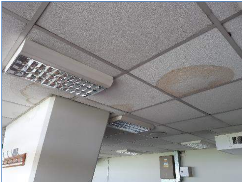
7-24 Damp damage to ceiling in press box
