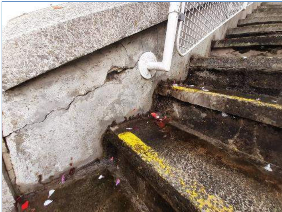
7-12 Cracking in concrete of central steps
