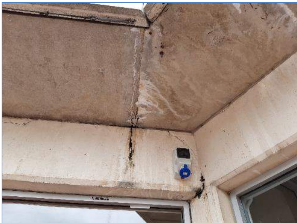
7-11 Cracking in soffit and corner of viewing terrace
