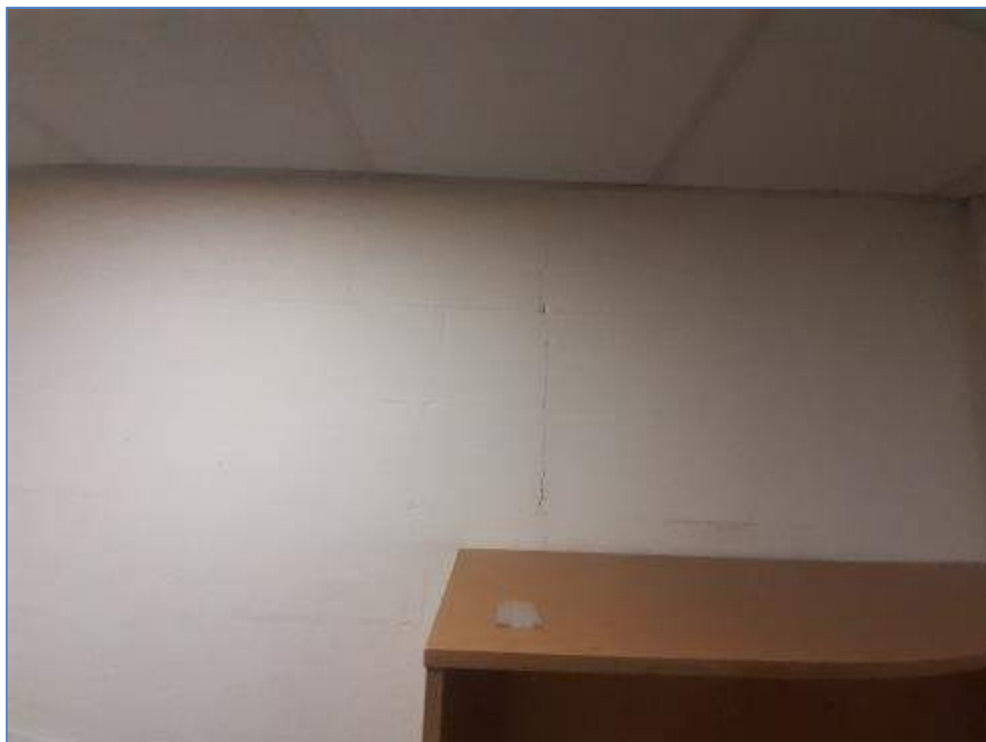
7-21 Cracking in wall of organisers office
