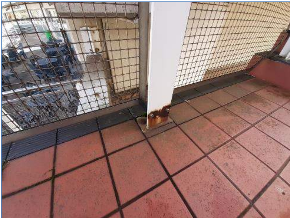
7-03 Steel riser plates to handrails rusting
