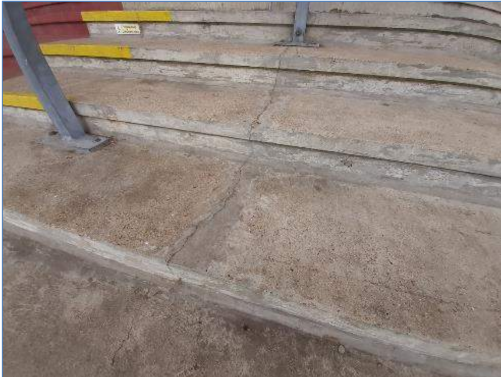
7-28 Cracking running down front terrace steps
