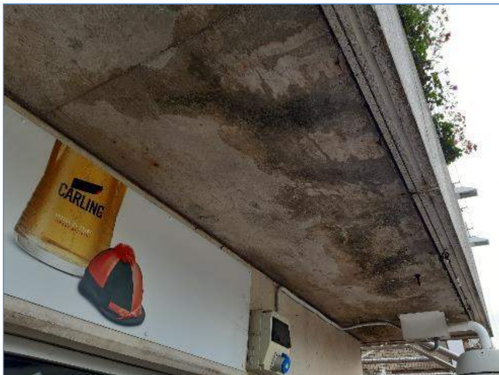
7-09 Damp on soffit of viewing terrace
