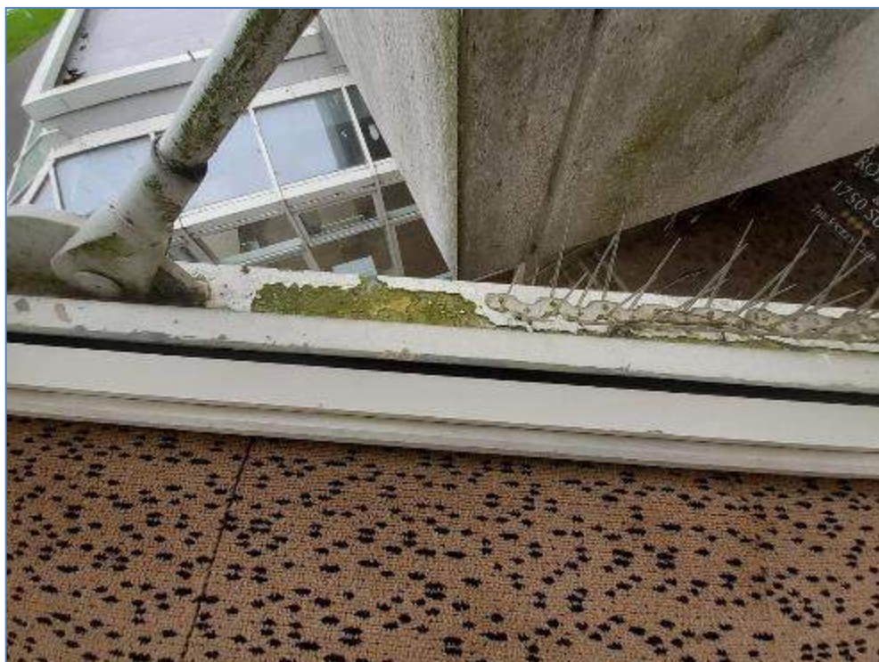
8-17 Paint peeling from link bridge support steelwork
