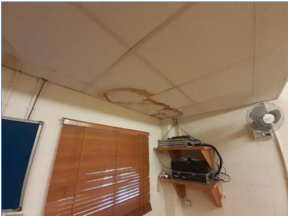
7-17 Damp in ceiling of switch room / staff kitchen area
