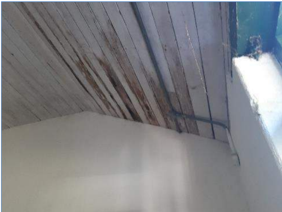
5-14 Damp in soffit boards of several stables
