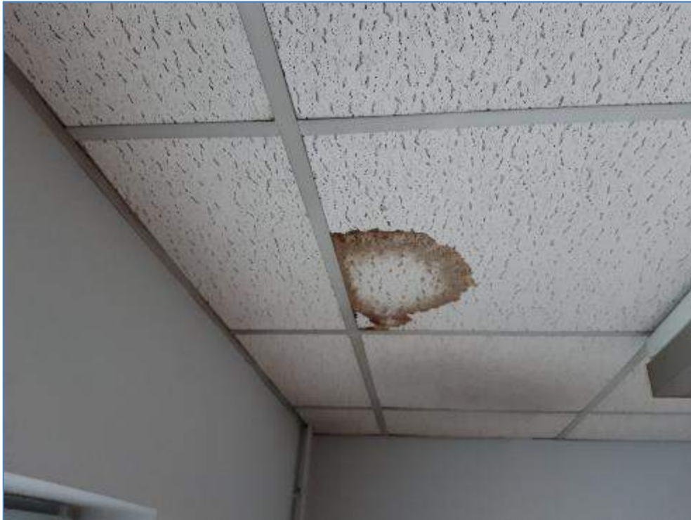
4-06 Damp damage to ceiling in lady jockeys changing room
