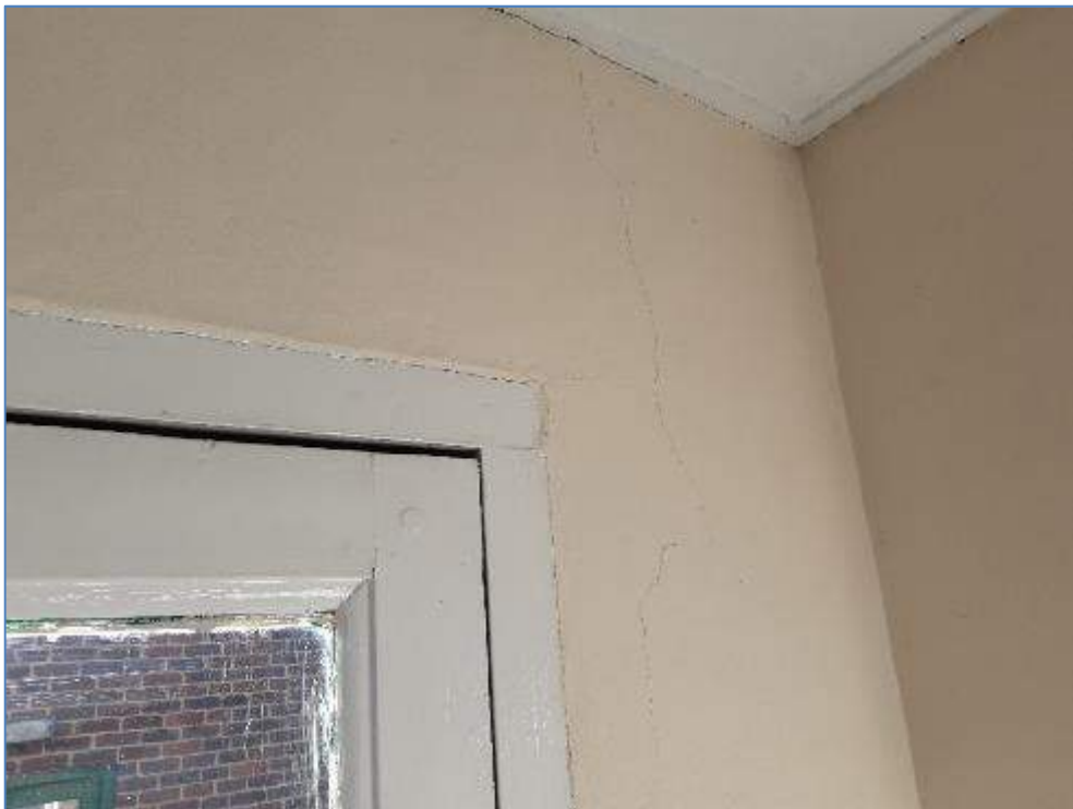
5-06 Cracking internally in the stable managers office
