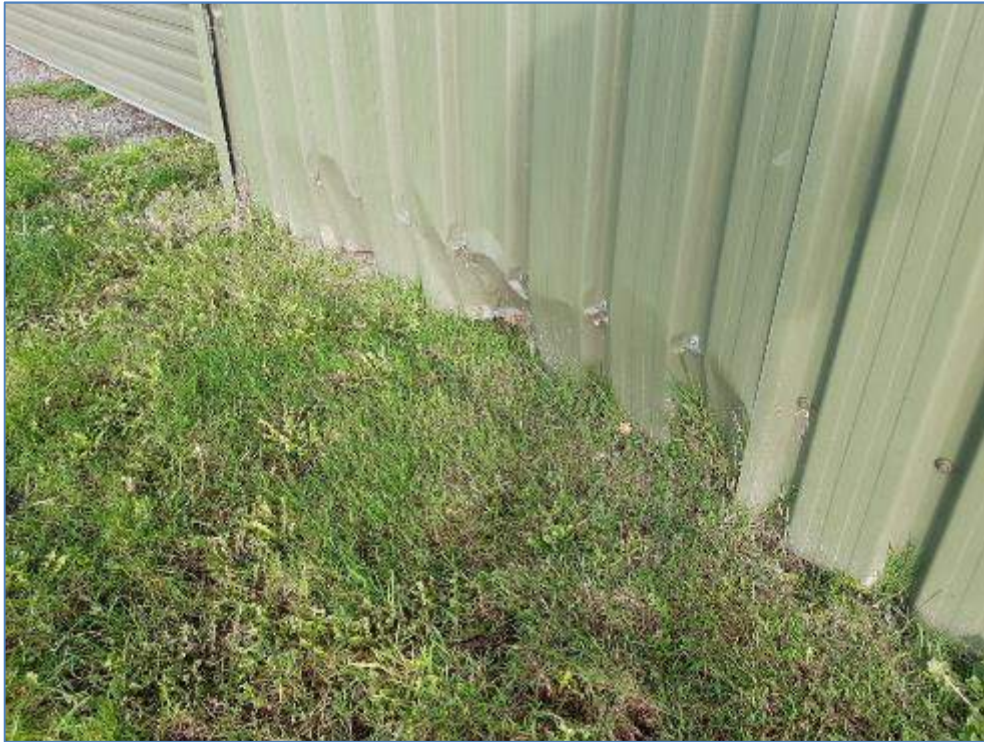
9-01 Steel cladding damaged in places
