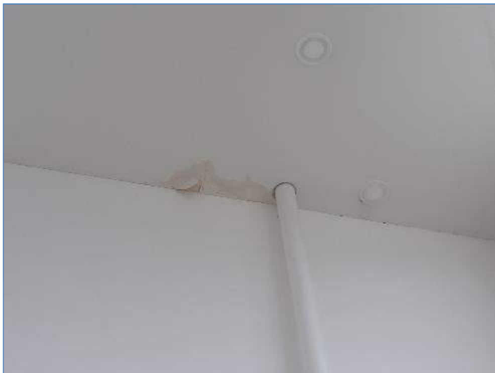
7-19 damp in ceiling over ramp in main entrance
