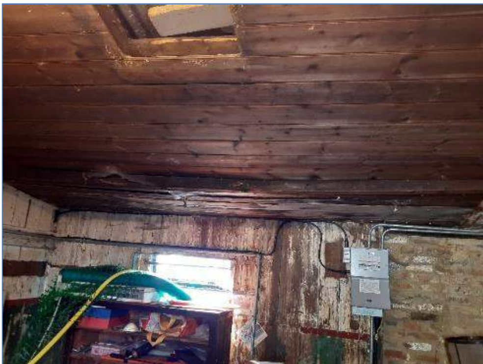
5-02 Timber beam sagging in maintenance store
