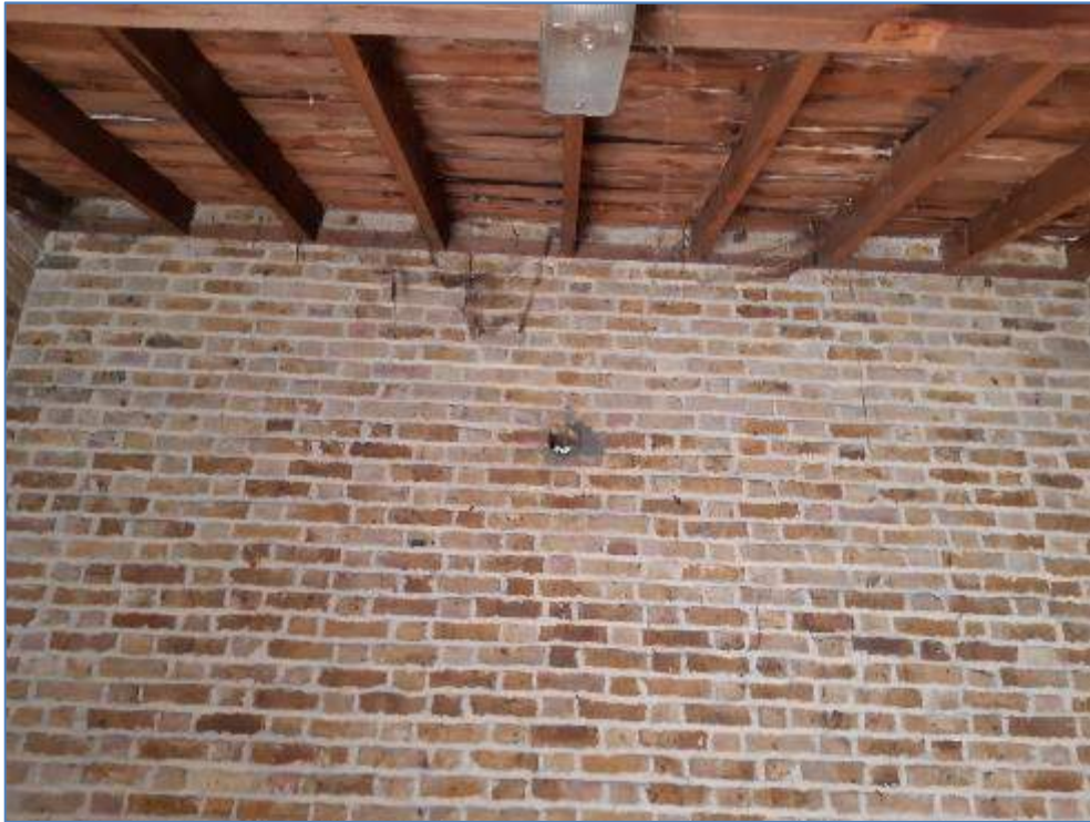
5-23 Brick missing from rear wall of store
