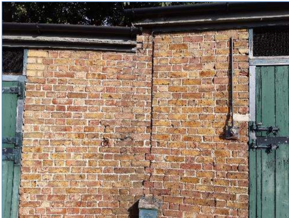
5-19 Crack in wall at steps between stables
