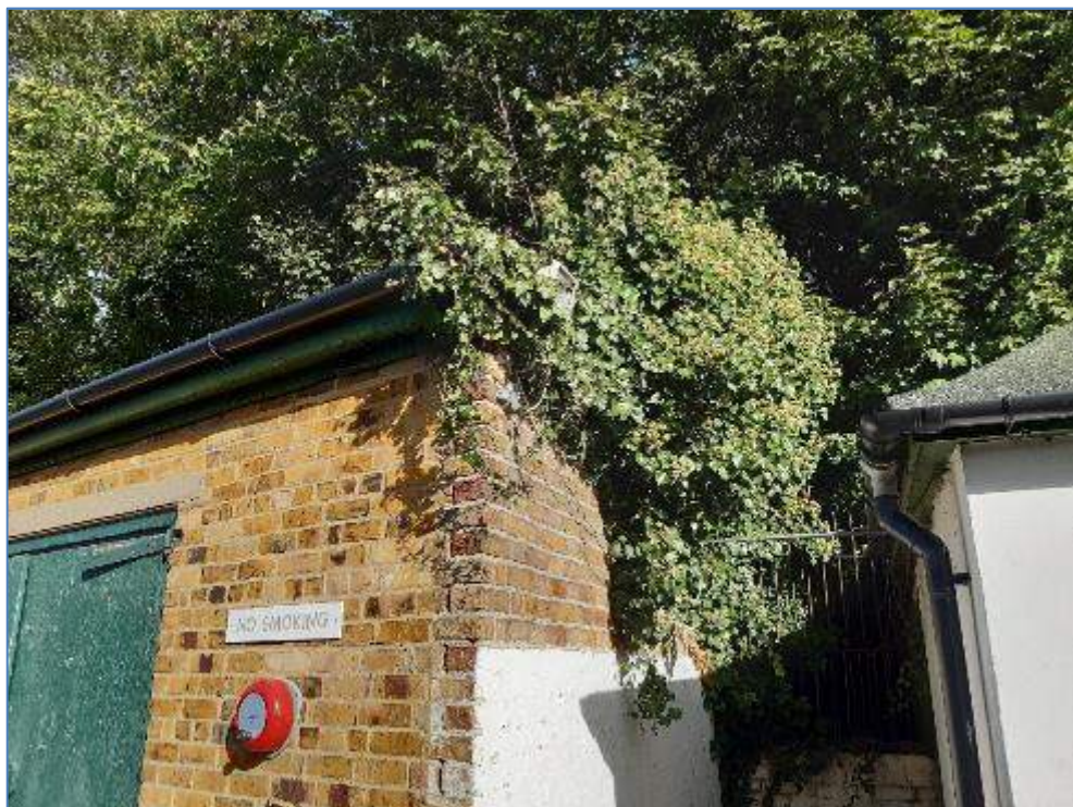
5-20 Heavy plant growth on end wall of stores
