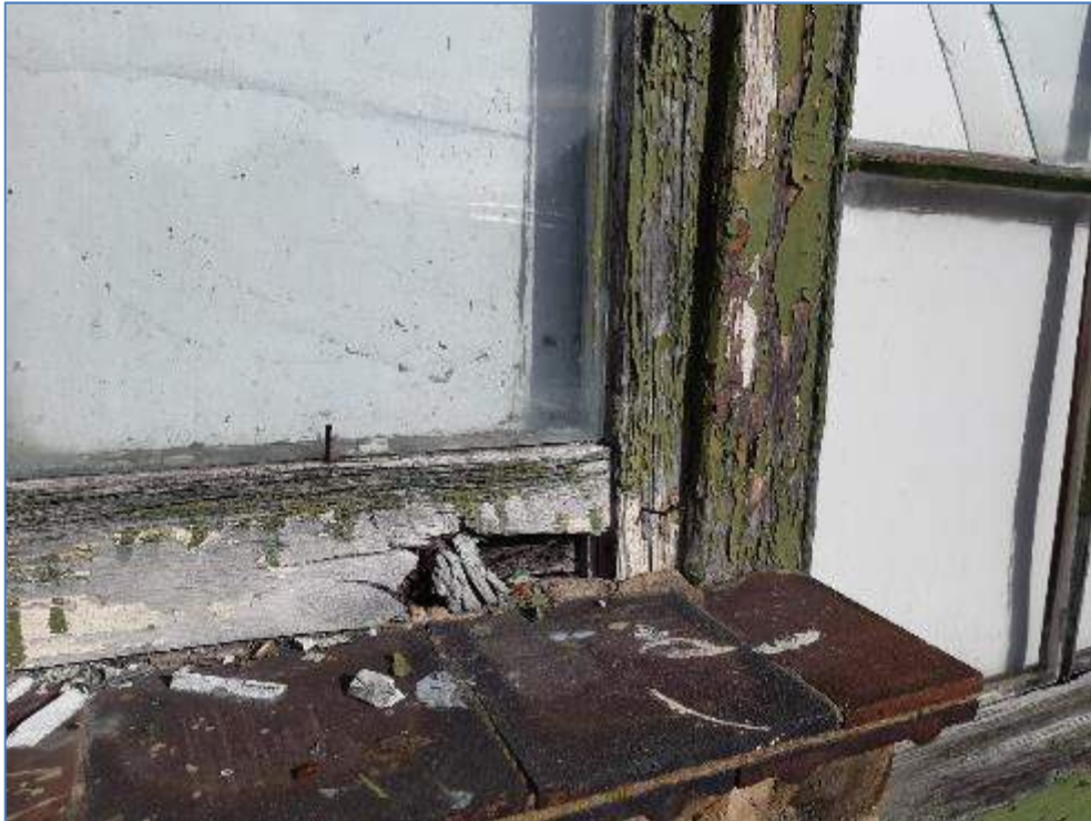
5-21 Timber window frames decaying
