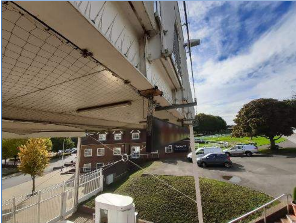
7-02 Brackets to illuminated sign rusting
