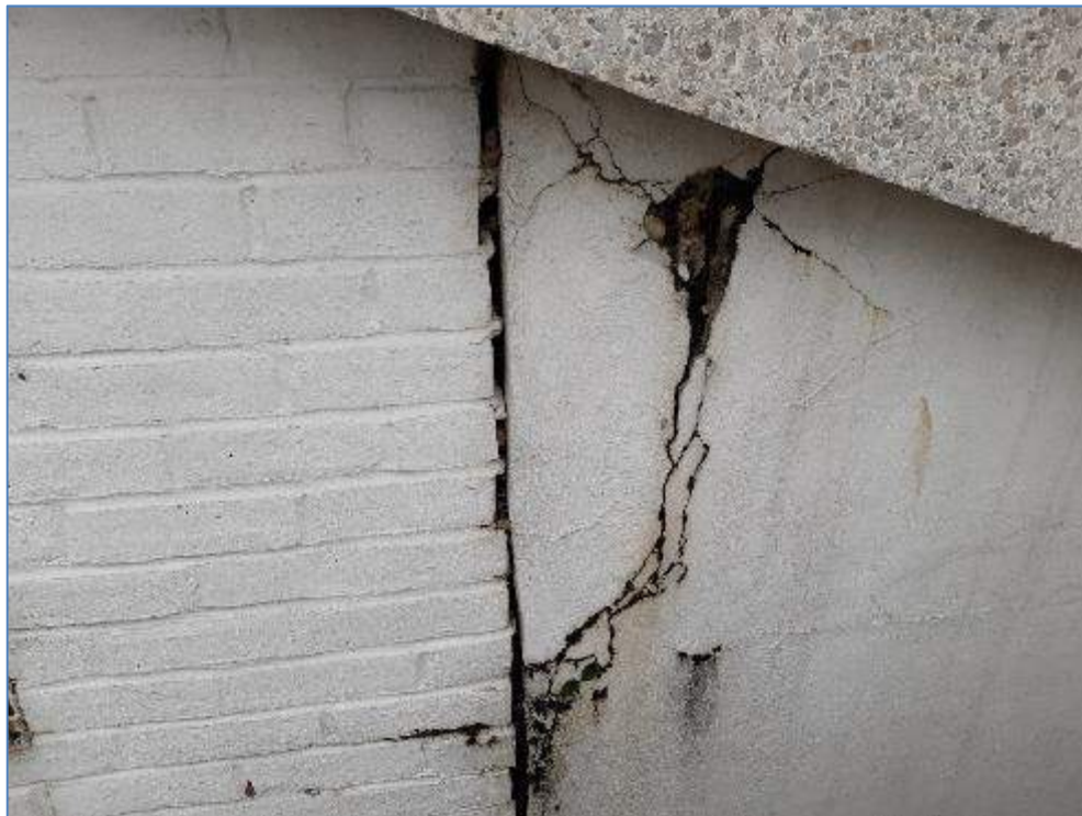
7-48 Cracks in render to terrace end wall
