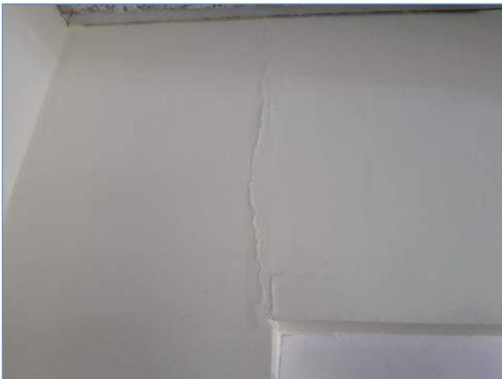
3-06 Crack over door in dining room
