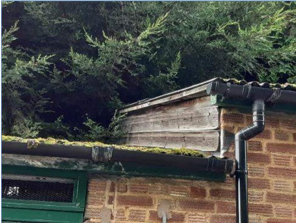
5-39 Timber step boarding decaying and warped in places
