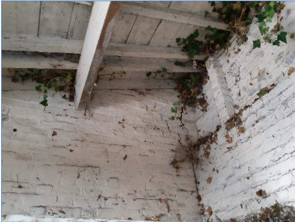
5-31 Cracking and plant growth to tack box walls
