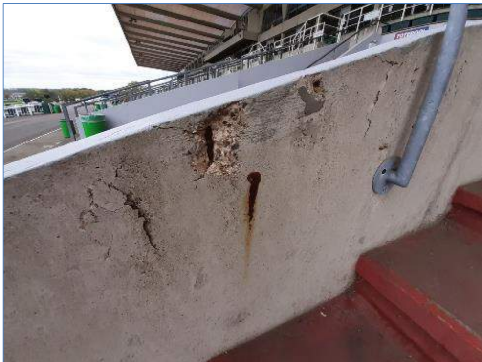
7-41 Concrete wall to vomitory spalling and exposing rebar
