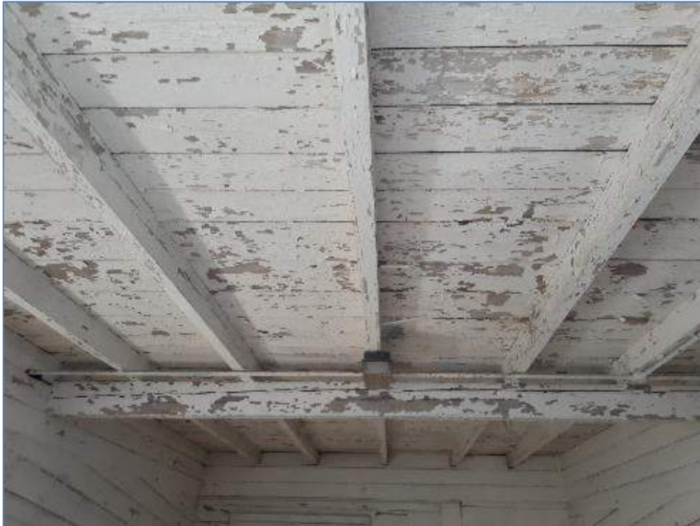
5-03 Paint peeling from soffit boards
