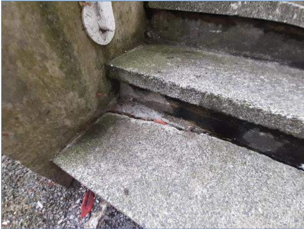
7-26 Crack in steps to terrace from Brasserie
