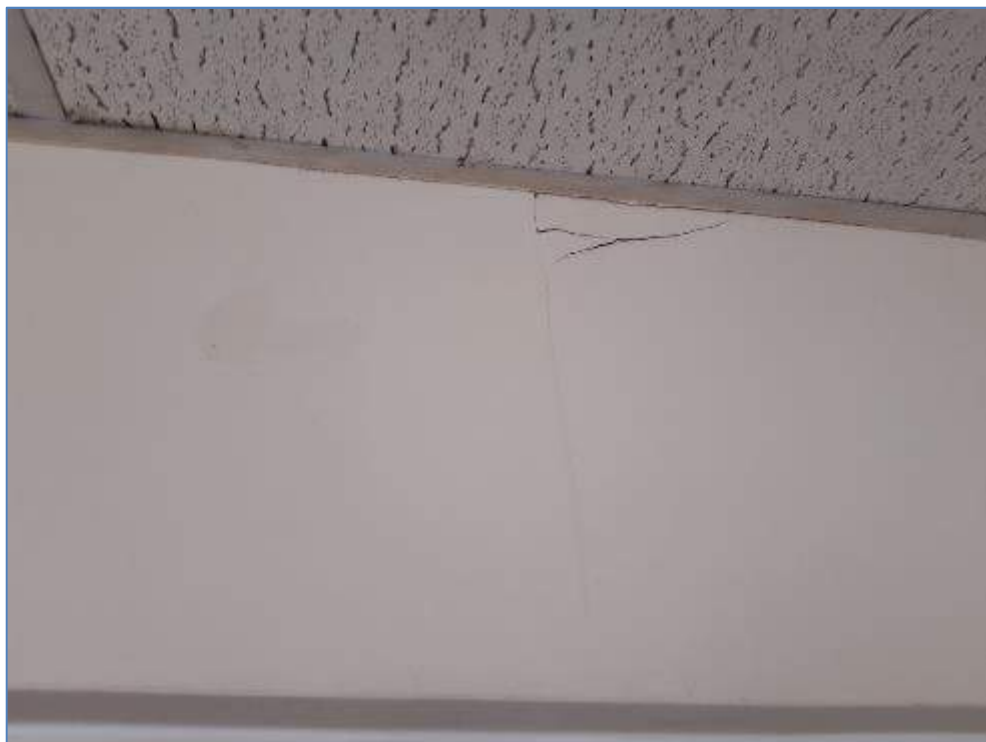
4-03 Minor cracking in office walls
