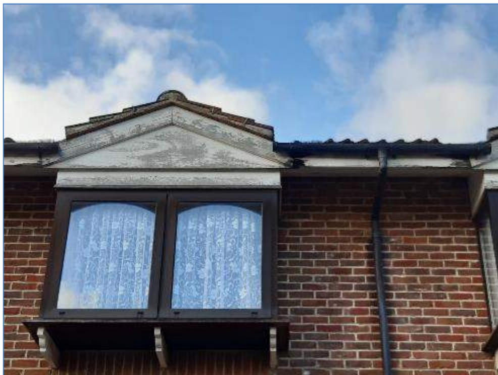
3-02 Timber fascias rotting adjacent to feature windows
