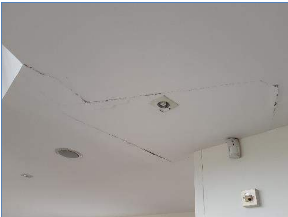
7-23 Cracks in ceiling of foyer by main entrance
