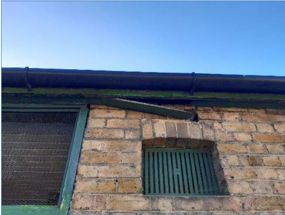
5-09 Eaves soffit board loose over stable 73
