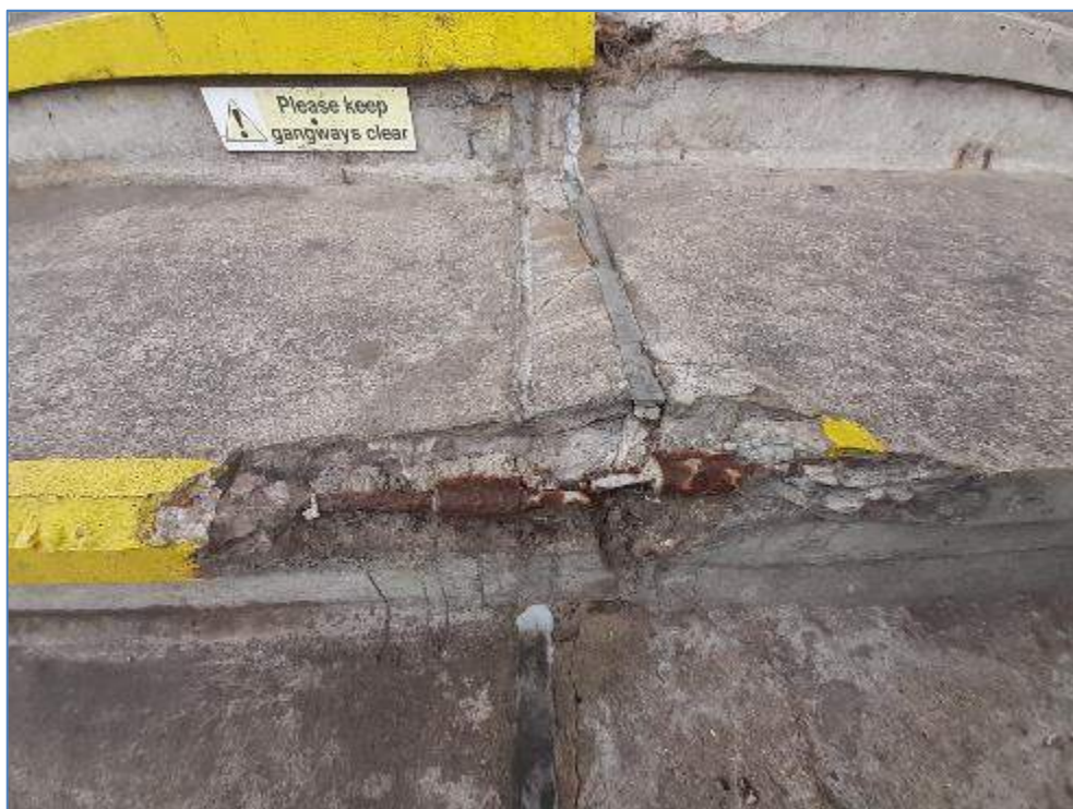
7-33 Concrete spalling heavily, exposing rebar on front terrace
