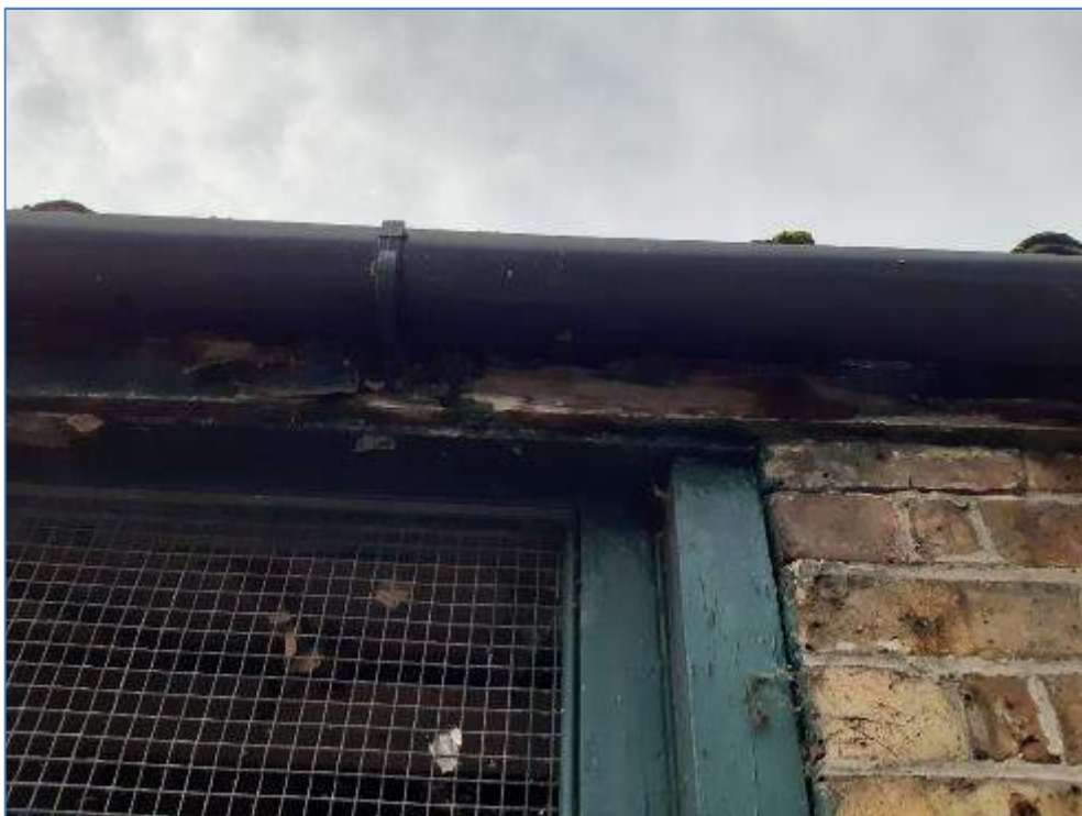
5-32 Timber eaves decaying
