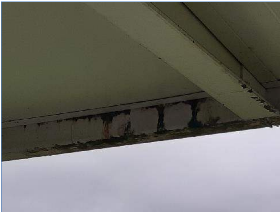
8-07 Surface rust to balcony support steelwork
