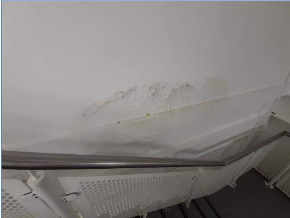
8-14 Wall spalling in service stairs
