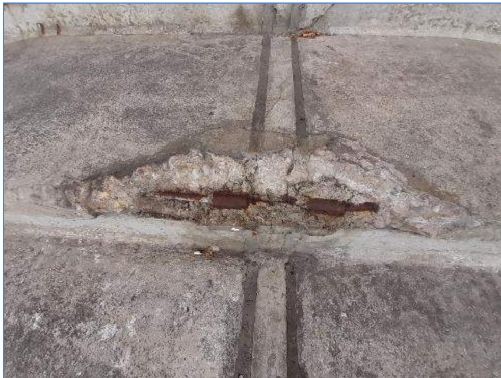
7-32 Concrete spalling heavily, exposing rebar on front terrace
