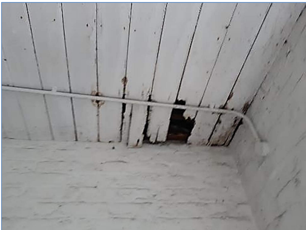
5-40 Timber soffit boards decaying in stable 57
