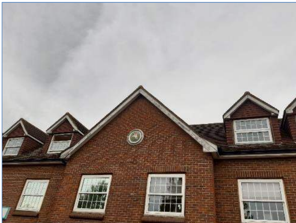
4-01 Paint peeling from timber fascias
