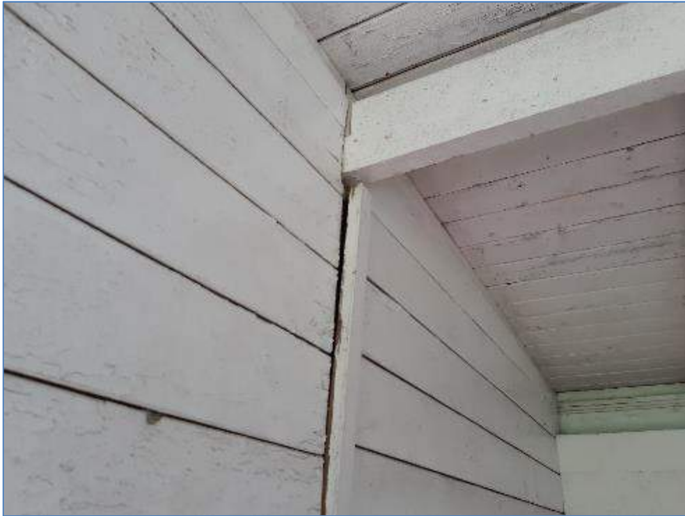
6-05 Timber infill section working loose
