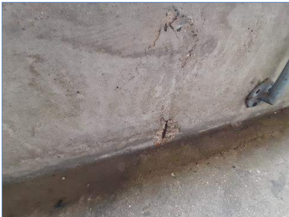
7-39 Concrete spalling on wall of disabled ramp
