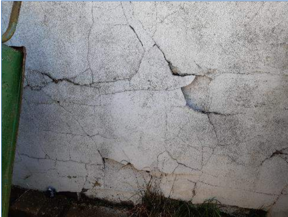
5-15 Render cracking and spalling heavily on external end wall
