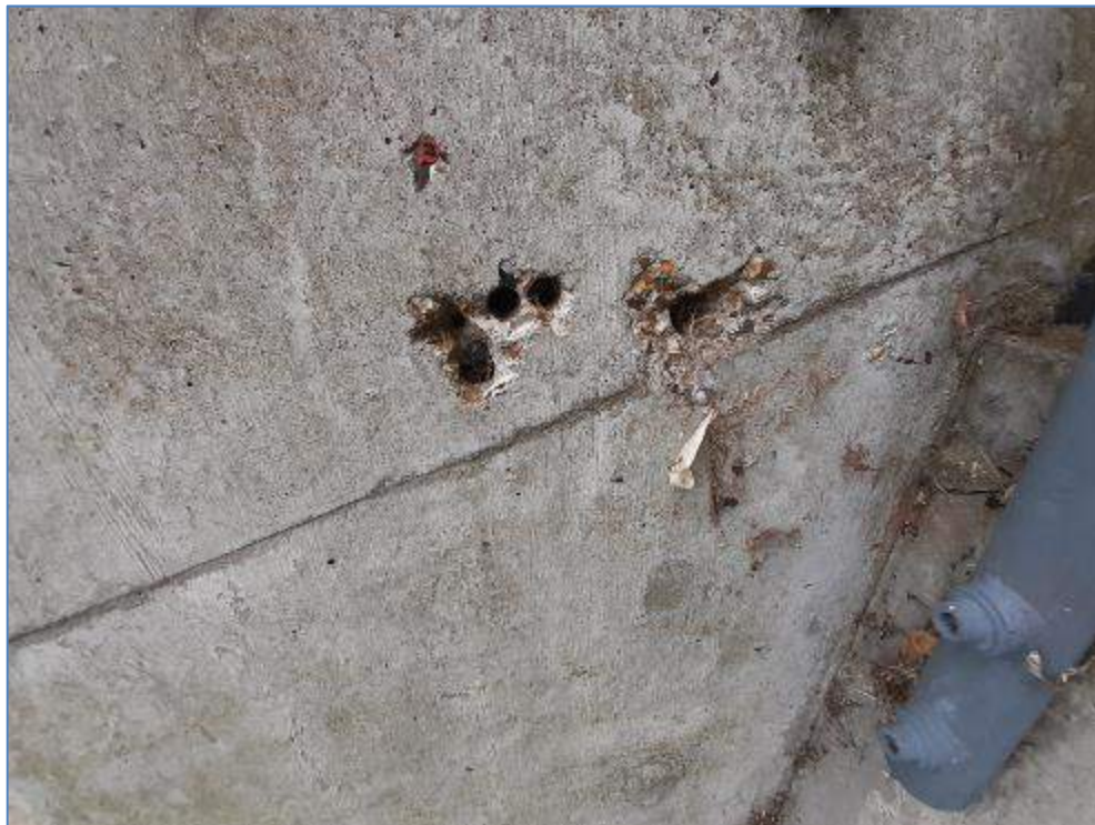
7-38 Concrete spalling on vomitory walls
