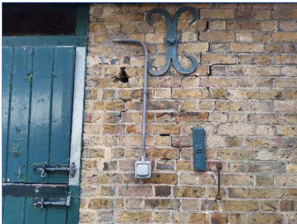
5-28 Crack in external wall of stables
