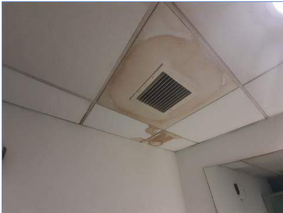
7-18 Damp in ceiling of male toilets
