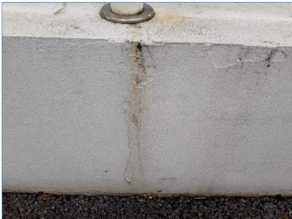
7-45 Cracking in walls to disabled ramp at Esher Hall entrance
