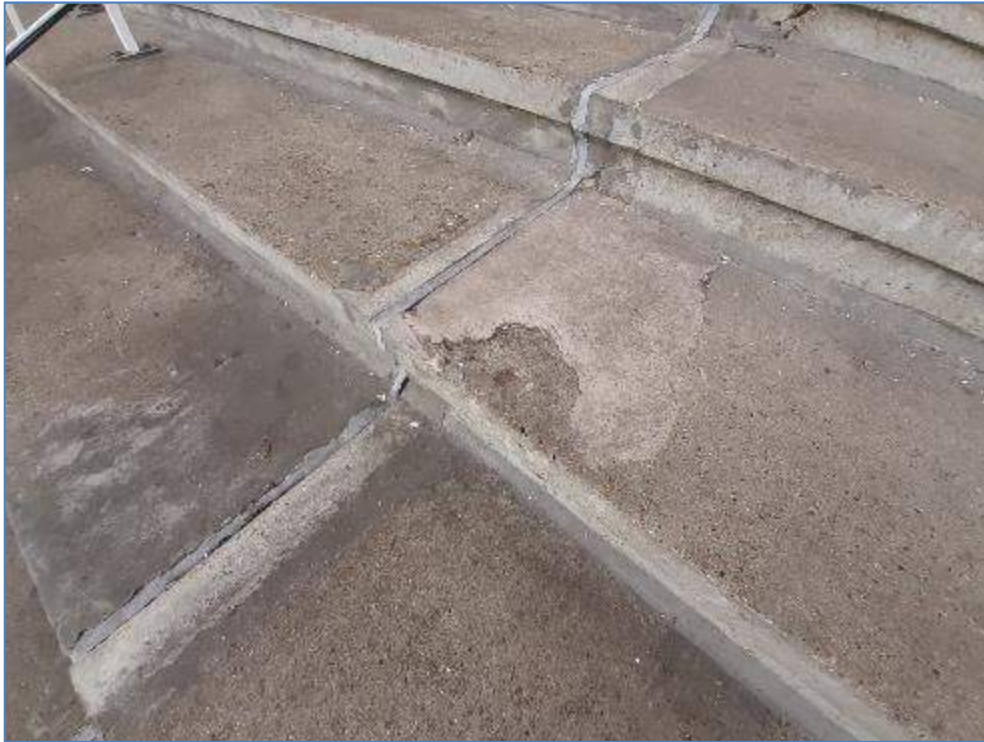
7-30 Concrete spalling on front terrace
