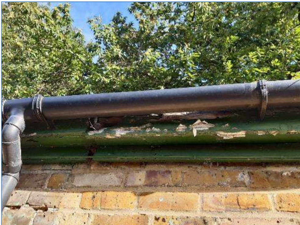
5-18 Paint peeling from timber eaves in several places
