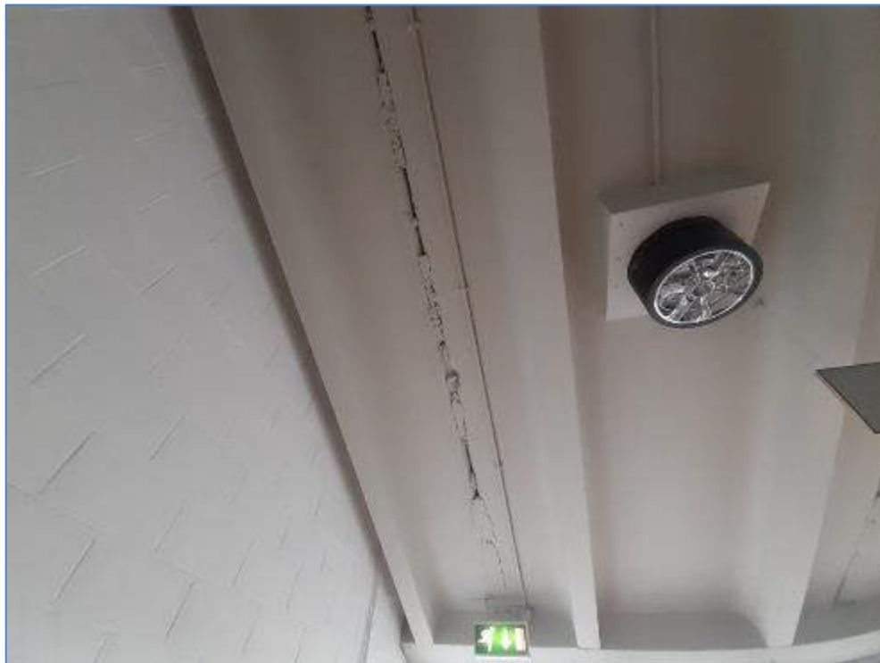
7-20 Joints opening up in precast units over vomitories
