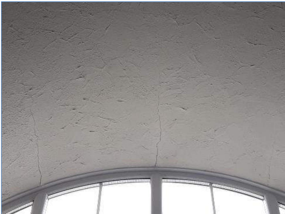
4-07 Cracking in vaults over windows in weighing room
