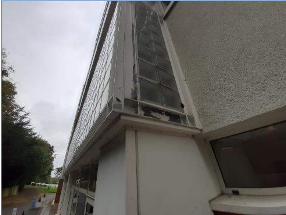
8-02 Paint peeling from steel around feature windows
