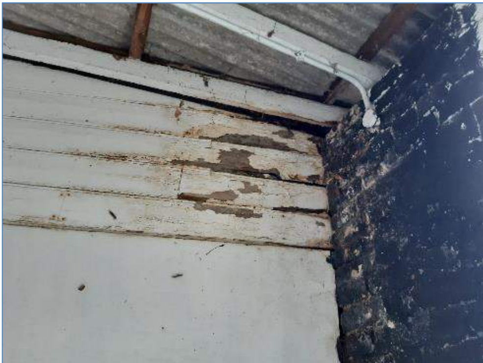
5-34 Wall timber rotting in stable 54
