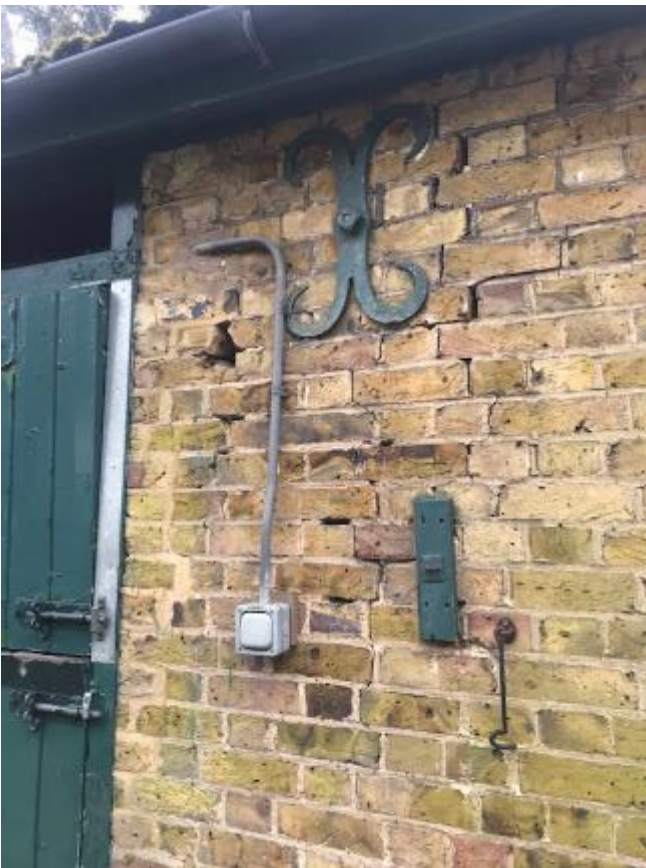
244. Cracked and damaged brickwork to front wall of stable 19.
