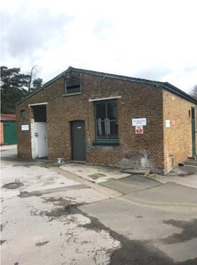
229. Decorations and brickwork to the gable elevation of stable 72 are in poor condition.
