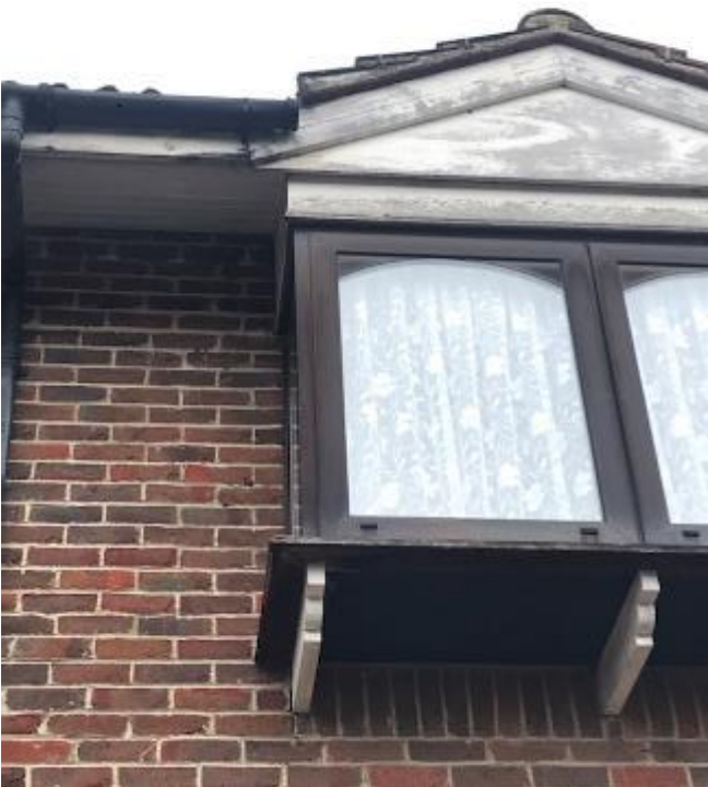
180. Fascias and soffits are in poor decorative order and partially rotten.
