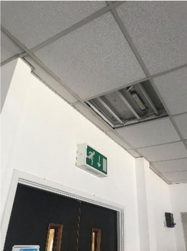
111. Example of faulty light fitting.
