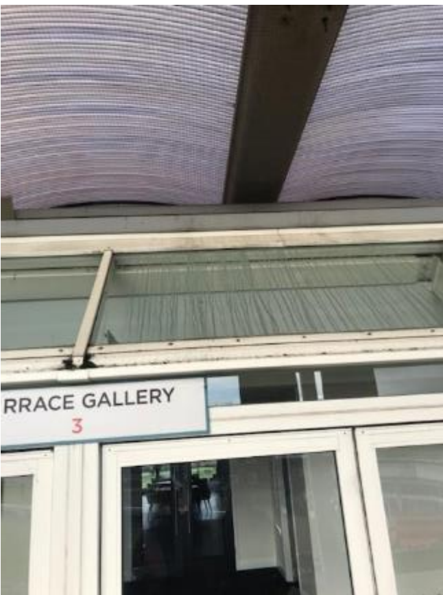
24. Water staining to corridor glazing from leaks from fabric canopy over the terrace.
