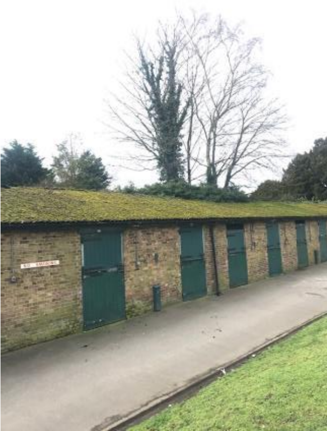
239. Substantial moss cover to brittle asbestos cement stable roofs.
