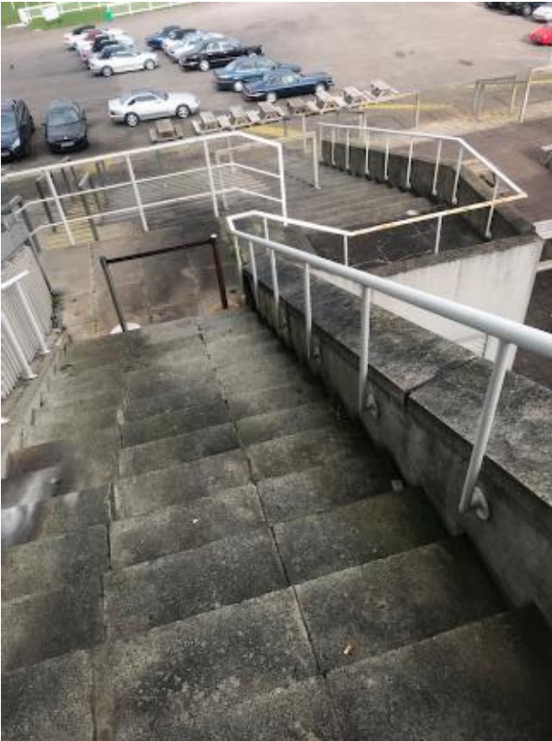
177. External escape stairwell from second floor terrace. Note: staining to pavings from roof/terrace leaks.
