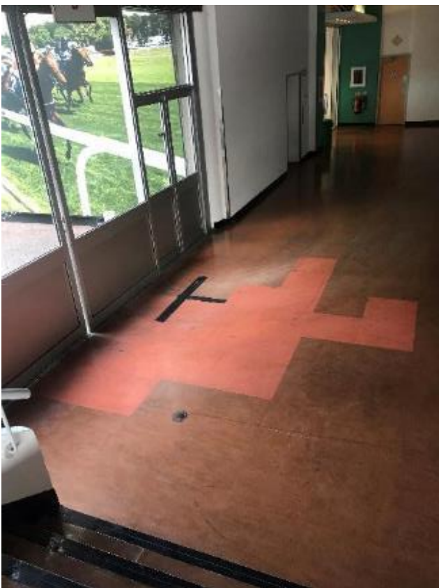
82. Water damaged vinyl floor replaced in non-matching section as original is no longer available. Ongoing water ingress has caused joints to lift which have been taped down to reduce risk of a trip hazard.
