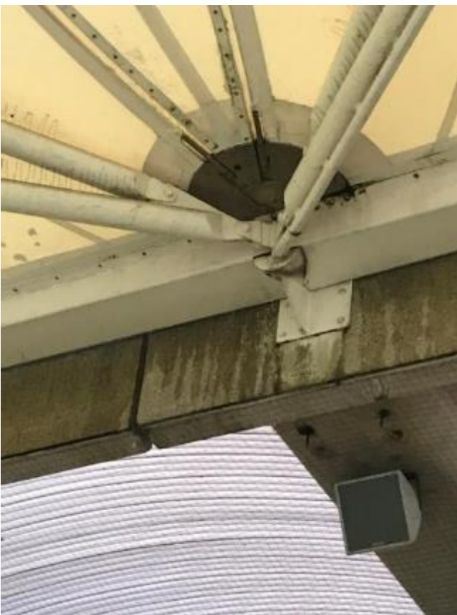
20. Close up of leaking fabric canopy and hopper / gutter detail.
