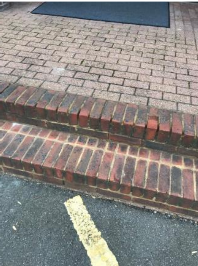
184. Bricks to entrance steps are spalling in part with some perished mortar pointing.
