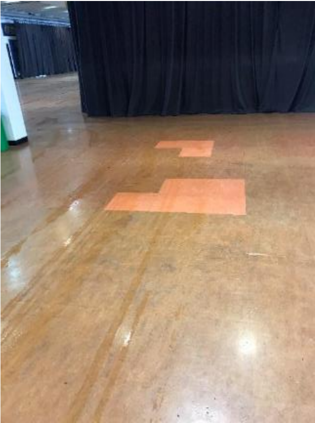
83. Further example of sections of vinyl floor having been replaced with non-matching sections.
