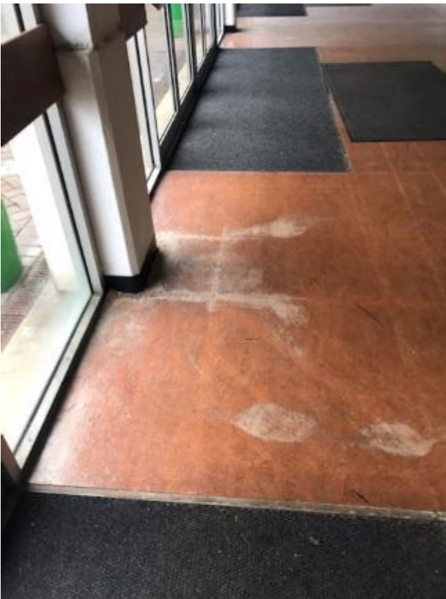
80. Example of heavily stained floor vinyl due to persistent leaks from Parade Ring Terrace.
