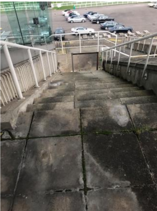
176. External escape stairwell from second floor terrace. Note: staining to pavings from roof/terrace leaks.
