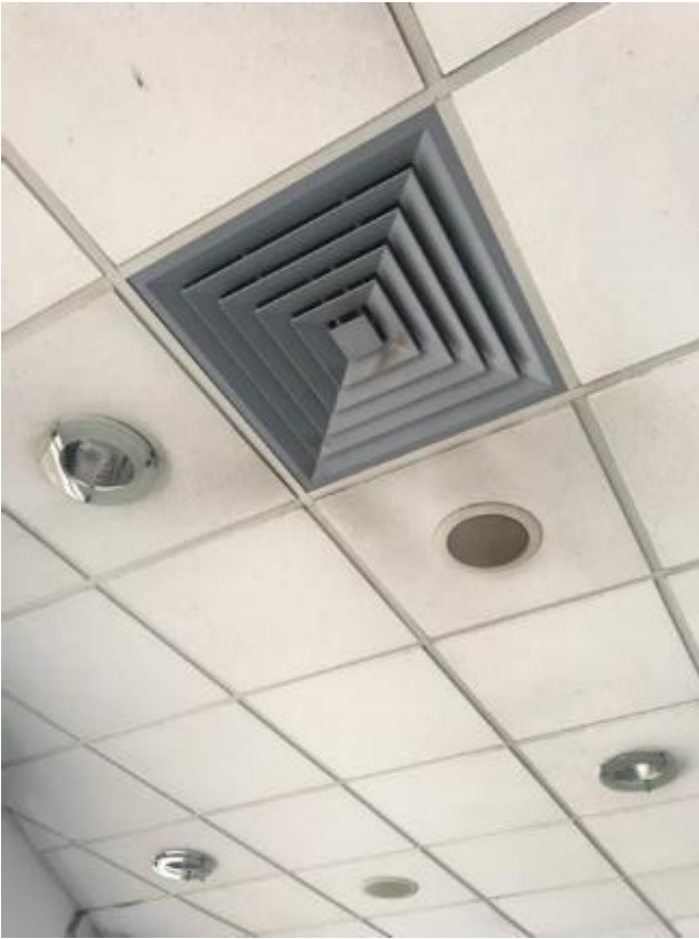
73. Example of heavily soiled ceiling tiles around vent grille.
