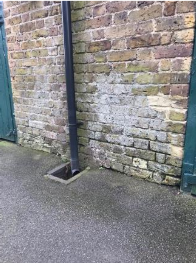
243. Close up of typical example of perished mortar to low level brickwork.
