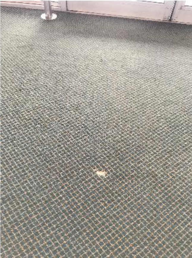
123. Close up of worn and tracked carpet.
