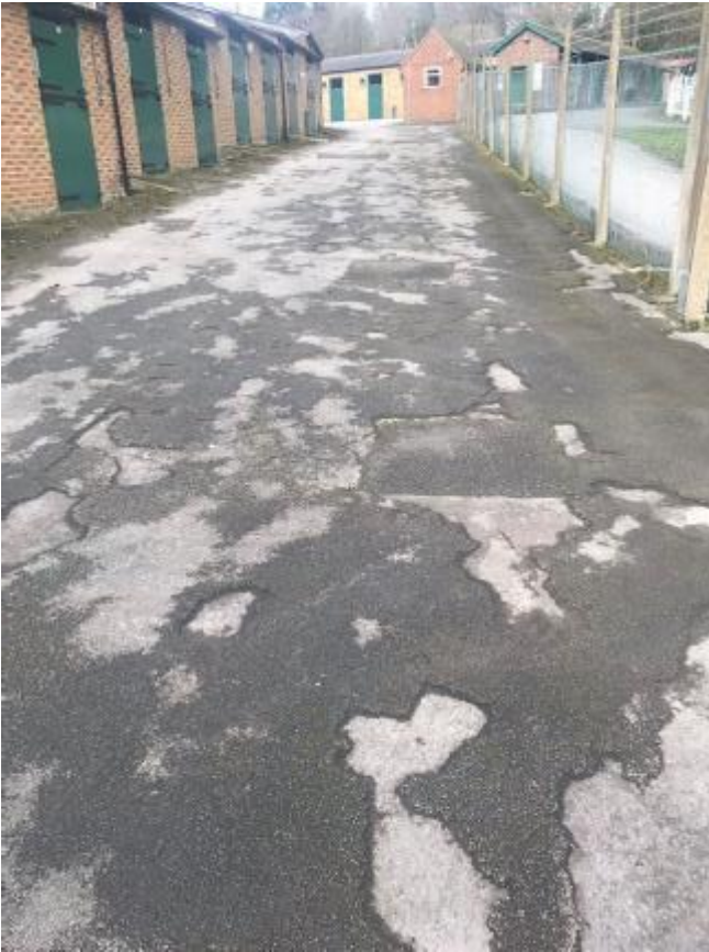
221. The yard surface is breaking up alongside stable block 56 – 69 and a trip hazard for horses and personnel alike.
