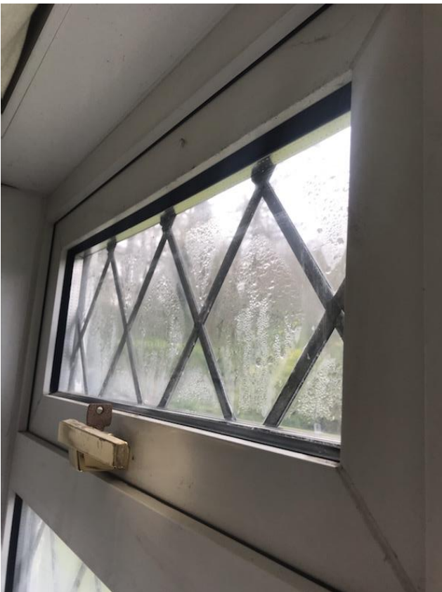
276. Condensation to double glazed windows.
