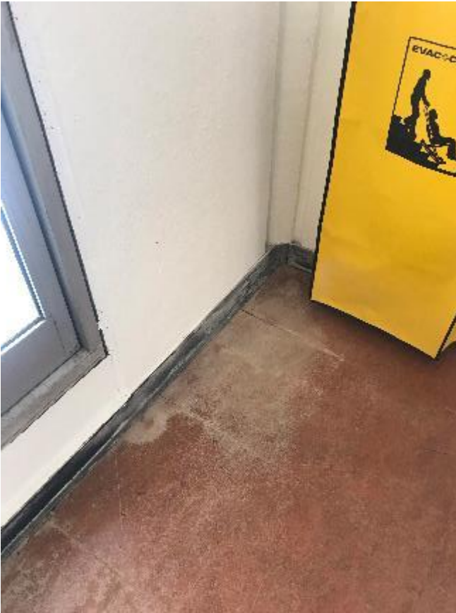
169. Staining/damage to vinyl floor covering due to roof leaks in second floor escape stairwell.
