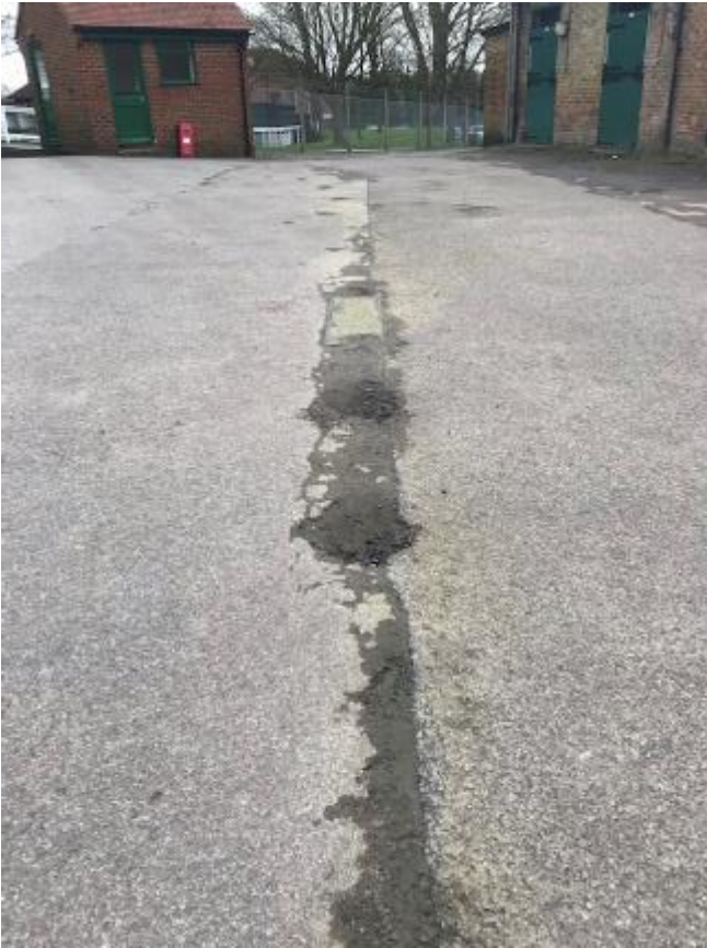
247. Pot holes in yard surface to area between stables 72 and 48.
