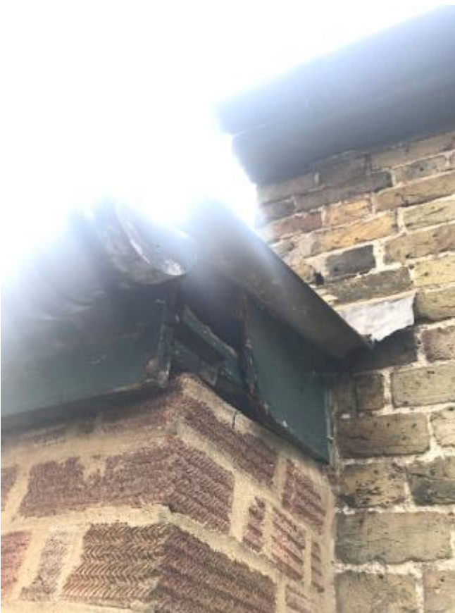
216. Barge boards and fascias are in poor decorative order with some wet rot/missing sections of timber.
