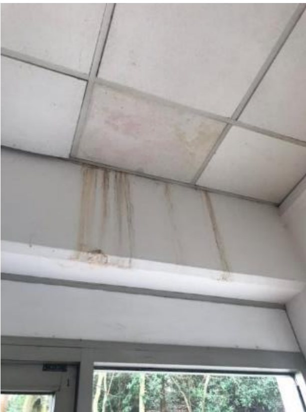
76. Further example of water stained ceiling tiles below Parade Ring Terrace and run marks to wall below from water ingress.
