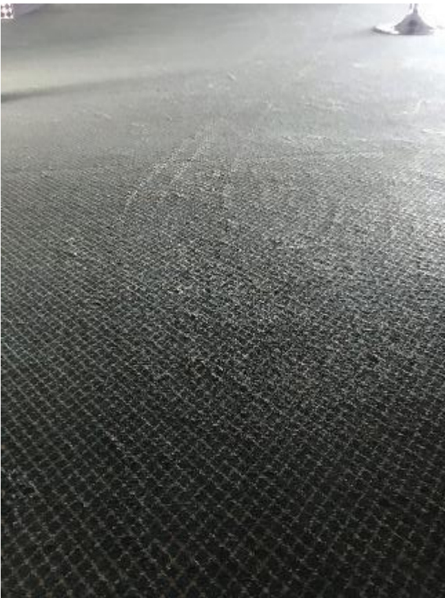
124. Close up of worn and tracked carpet.
