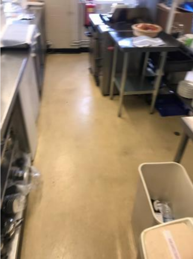
211. Vinyl floor covering in kitchen is marked and soiled.
