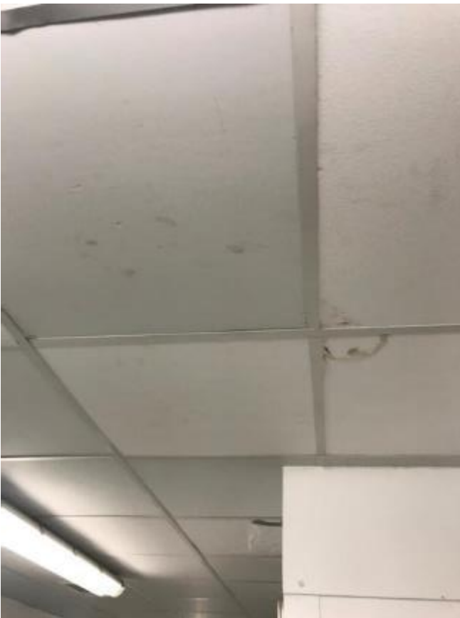
60. Example of damaged ceiling tiles.
