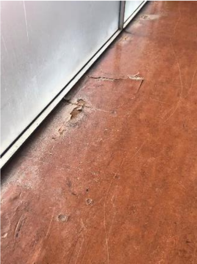
79. Example of damaged and lifting floor vinyl from persistent leaks.
