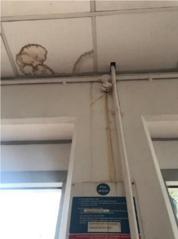
75. Further example of water stained ceiling tiles below Parade Ring Terrace and staining to wall below from water ingress.
