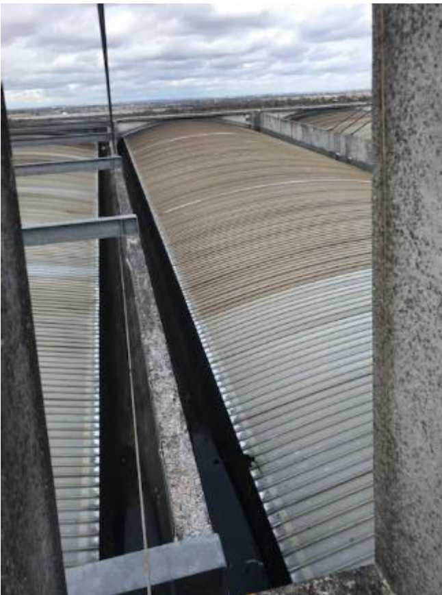
4. Typical discolouration and deterioration of brittle barrel vault canopy sections of roof.
