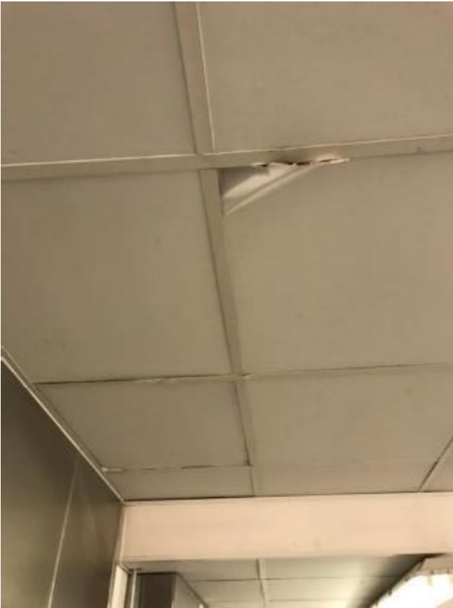
59. Example of damaged ceiling tiles.
