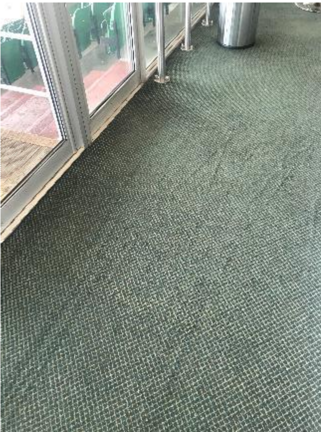
122. Close up of worn and tracked carpet.
