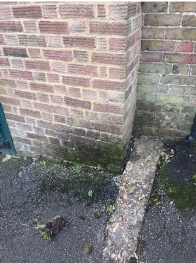
218. Defective rainwater goods are leaking and causing damp staining to the brickwork below.
