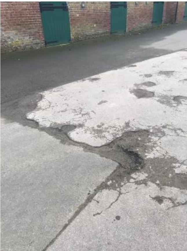
248. Pot holes in yard surface to area between stables 72 and 48.
