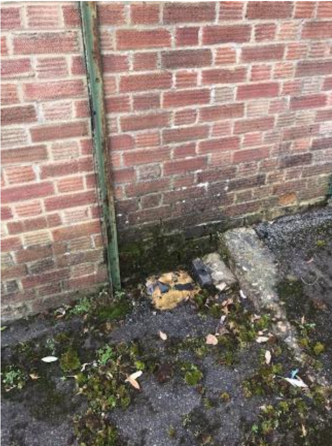
217. Defective rainwater goods are leaking and causing damp staining to the brickwork below.
