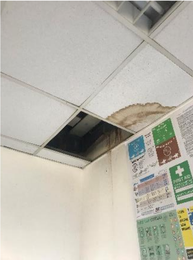
109. Example of missing and stained ceiling tiles with water stains running down the wall.
