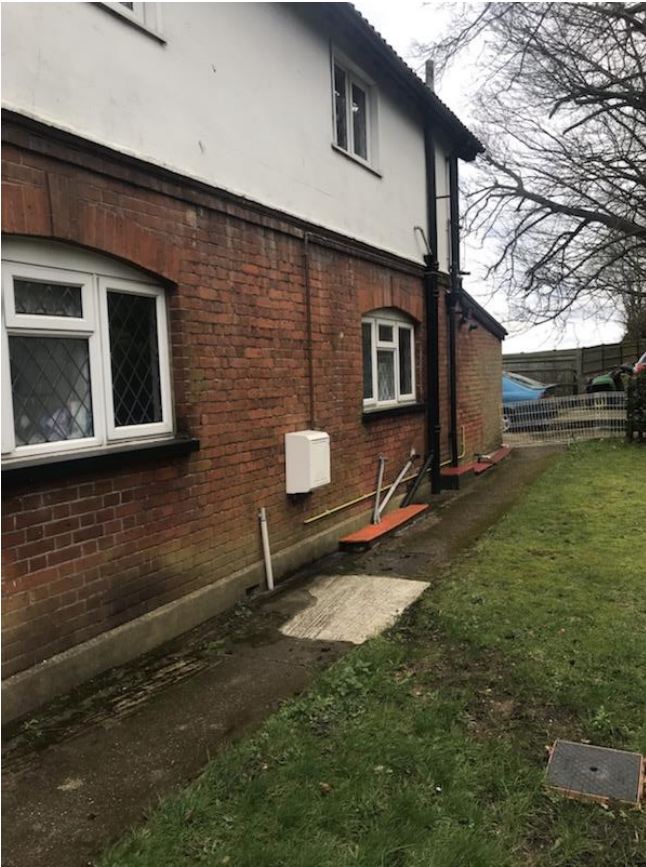
267. Damp stained and patch repointed external brickwork.
