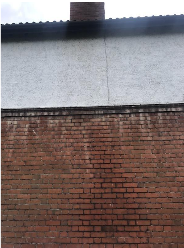
272. Damp and perished mortar pointing in the location of the chimney breast and at low level. Note : also cracked render.
