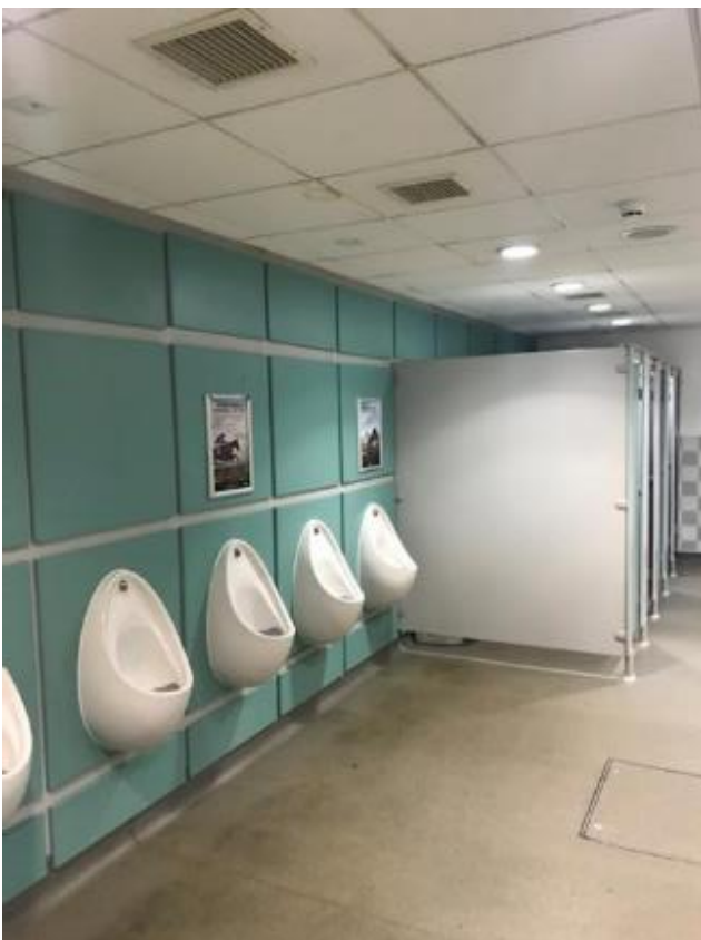
52. Dated Gents Toilets in need of upgrade/modernisation by Customer Standards. Note: heavy staining to sheet vinyl flooring around urinals, also stained and soiled ceiling tiles.
