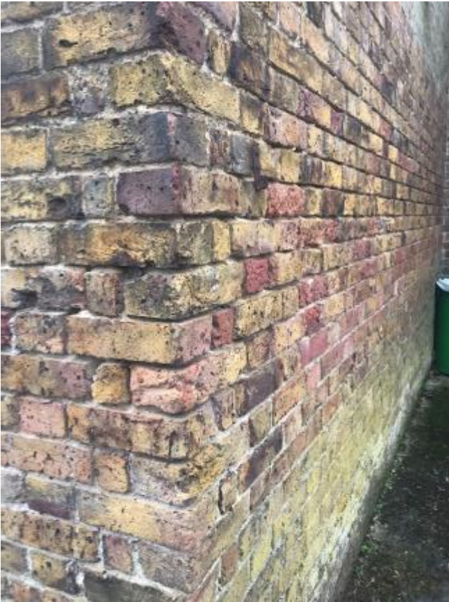
219. Mortar pointing to brickwork is perished in part, notably to the corner of stable 56.
