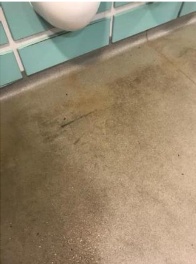
54. Heavy marking/staining to sheet vinyl around urinals in Gents Toilets.
