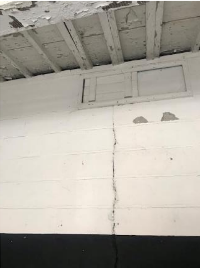
233. Cracking to rear wall of stable 46.
