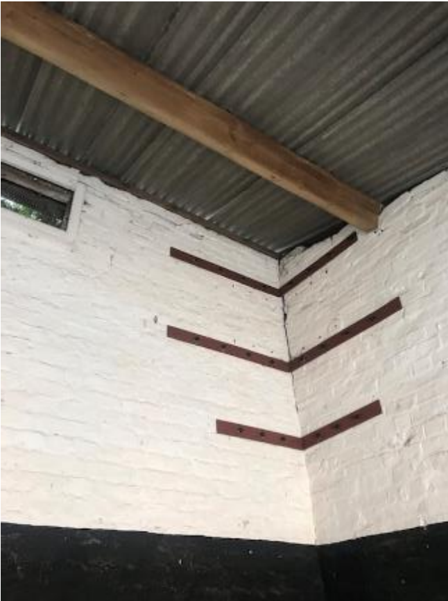
235. Metal strapping applied to restrain rear and side wall of stables 39-42.
