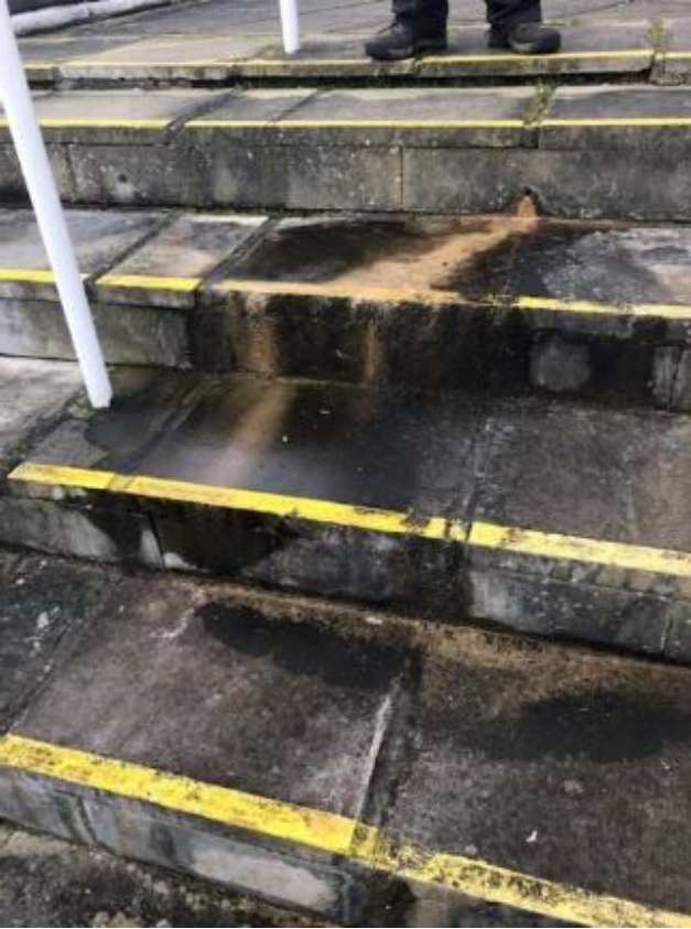
27. Rainwater leaking through the terrace pavings and steppings causing water ingress below.
