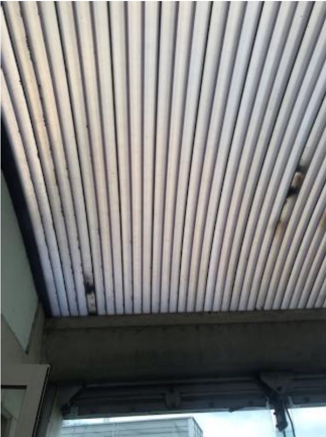
147. Close up of soiled and holed Grandstand barrel vaulted canopy over balconies to Second Floor Boxes.
