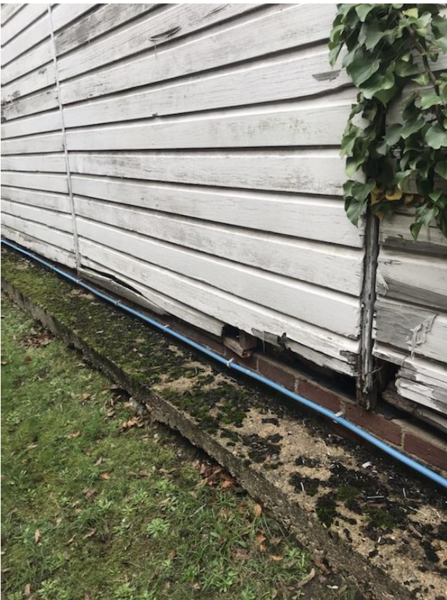
264. Rear elevation of saddling boxes in poor decorative order with some wet rot to the timber cladding.
