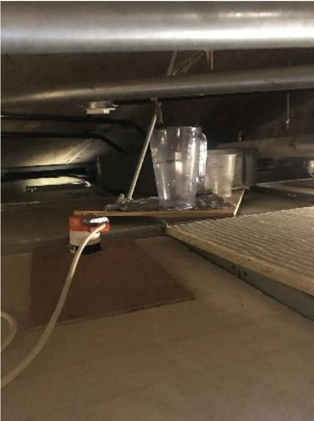
71. Example of buckets strategically placed above ceilings to Champagne Bar to catch leaks.
