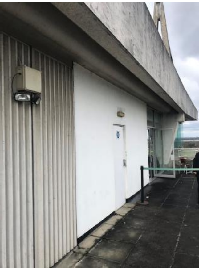
172. Leaks from roof/parapet onto second floor and terrace next to second floor boxes.
