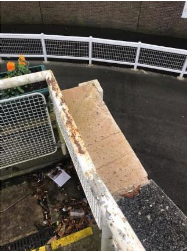
30. Typical corrosion to metal handrails to Terrace.
