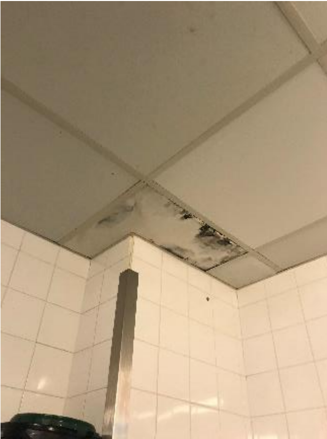
105. Example of water ingress to ceiling.
