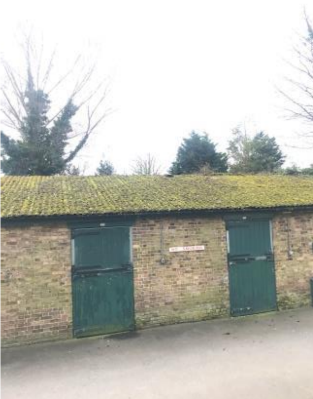
240. Substantial moss cover to brittle asbestos cement stable roofs.
