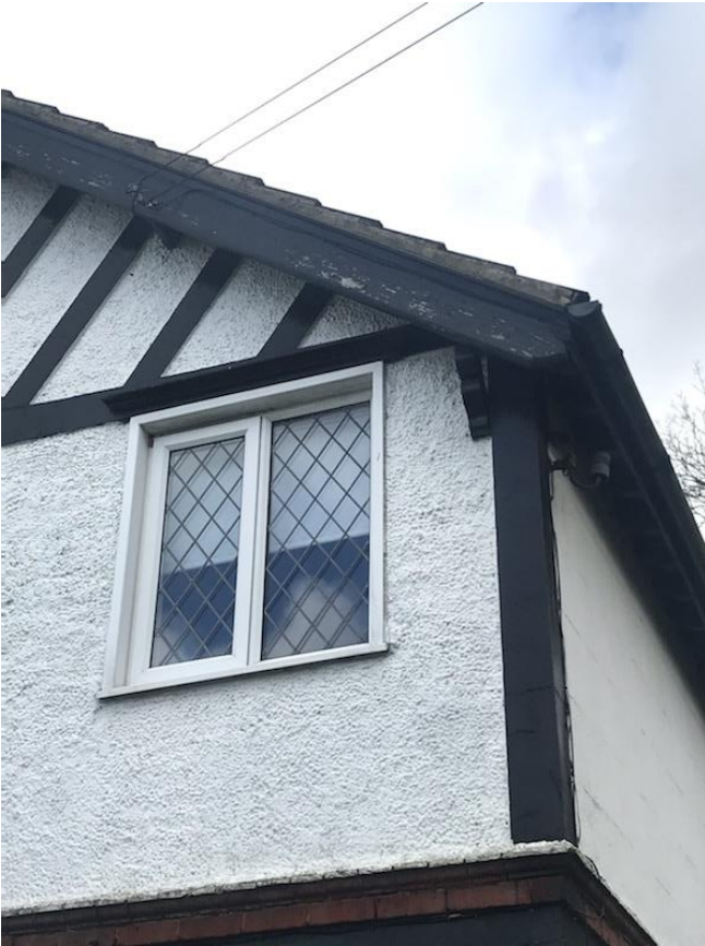
269. Peeling decorations to fascia/barge boards.
