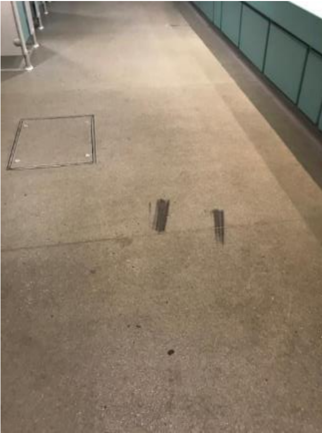
53. Heavy marking/staining to sheet vinyl floor in Gents Toilet.
