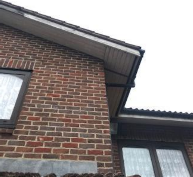
179. Fascias and soffits are in poor decorative order and partially rotten.
