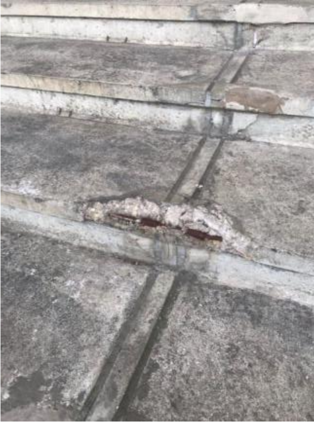
17. Example of spalling concrete risers to steppings due to corrosion of steel reinforcement bars.
