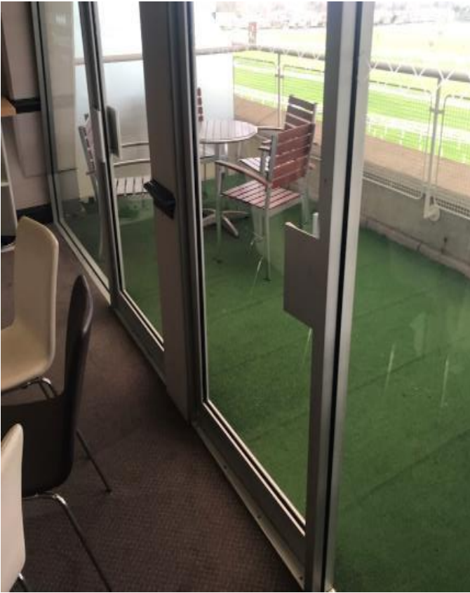
141. Close up of single glazed doors and windows to Second Floor Boxes.
