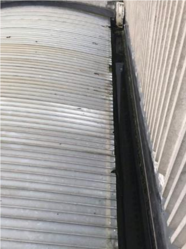
5. Typical close up view of damage to barrel vault canopy sections. UV degradation has caused the barrel vault canopy sections to become brittle.
