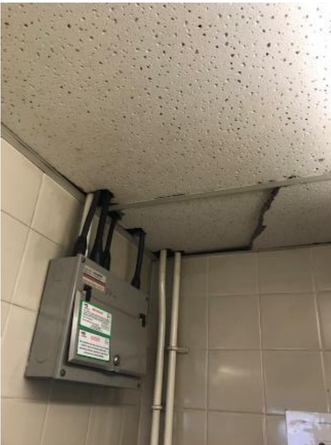
210. Close up of soiled and damaged ceiling tiles to kitchen.
