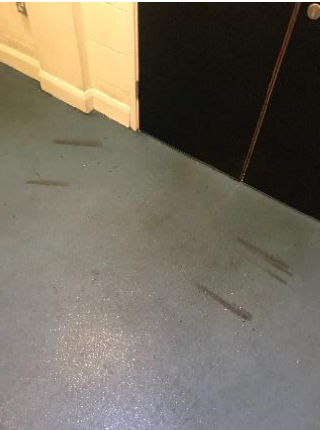
112. Close up example of scuffing/soiling to vinyl floor.
