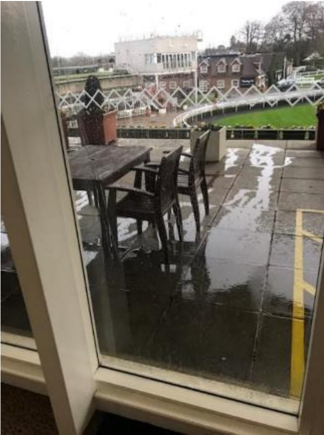
21. View of leaks from fabric canopy cascading down the terrace glazing and across the terrace pavings.
