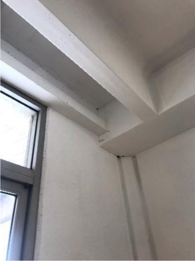
167. Staining from water ingress to corner of escape stairwell.
