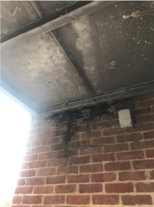
183. Leaks from metal fire escape onto brickwork and surface corrosion to metal staircase.
