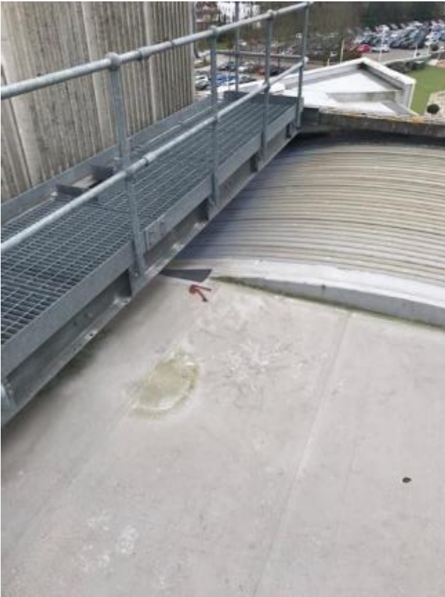
7. Typical example of patch repairs to abutment of flat roof sections and barrel vault canopy sections.
