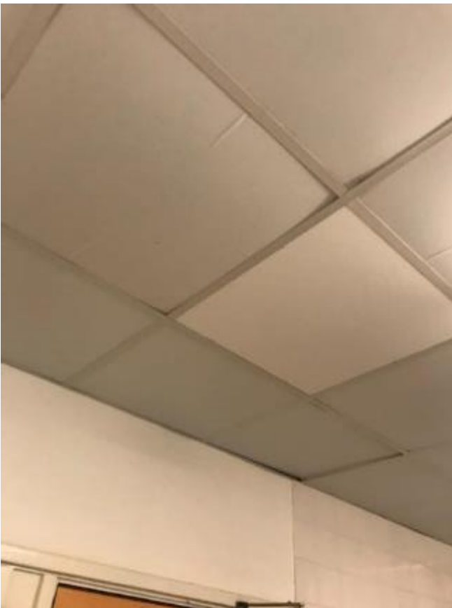
58. Kitchen ceiling tiles replaced following leaks.
