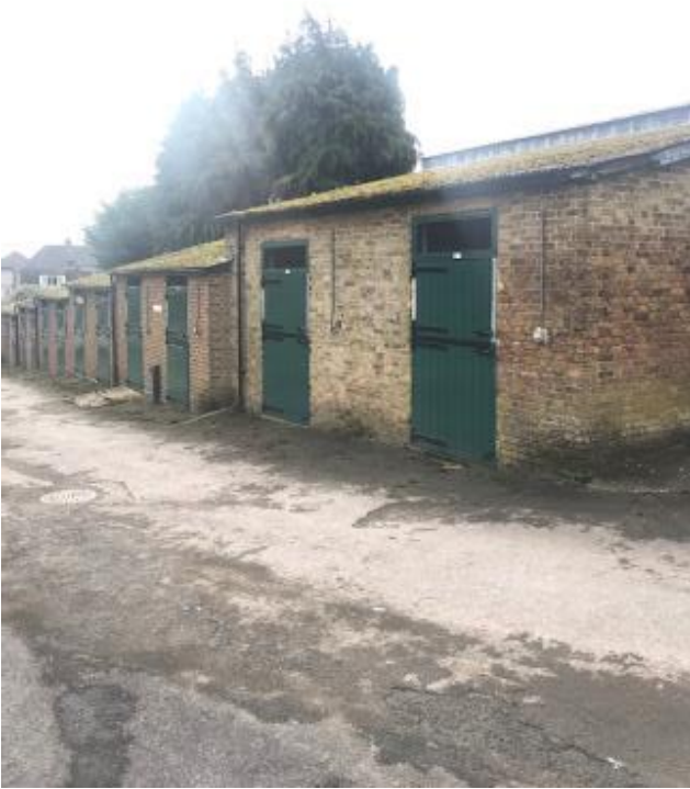
213. Stable Block 56-69. Note : substantial moss/vegetation cover to the brittle asbestos cement roofs.
