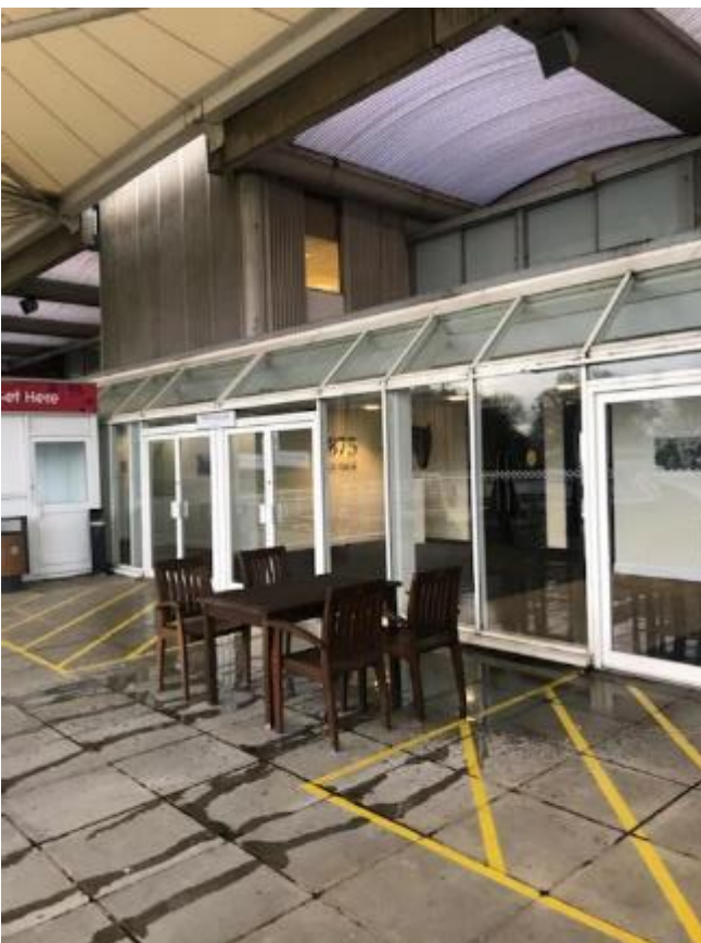
22. View of leaks from fabric canopy cascading down the terrace glazing and across the terrace pavings.
