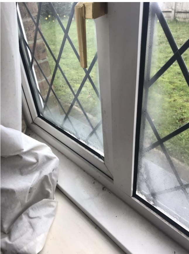
280. Condensation to double glazed window.
