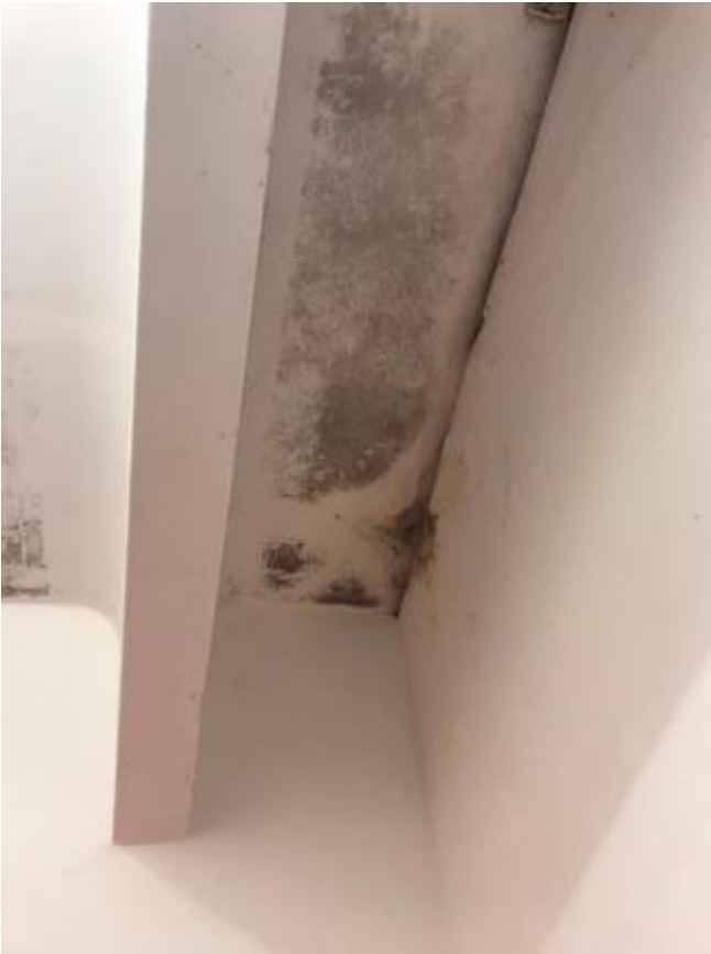
39. Damp staining to ceiling soffit.
