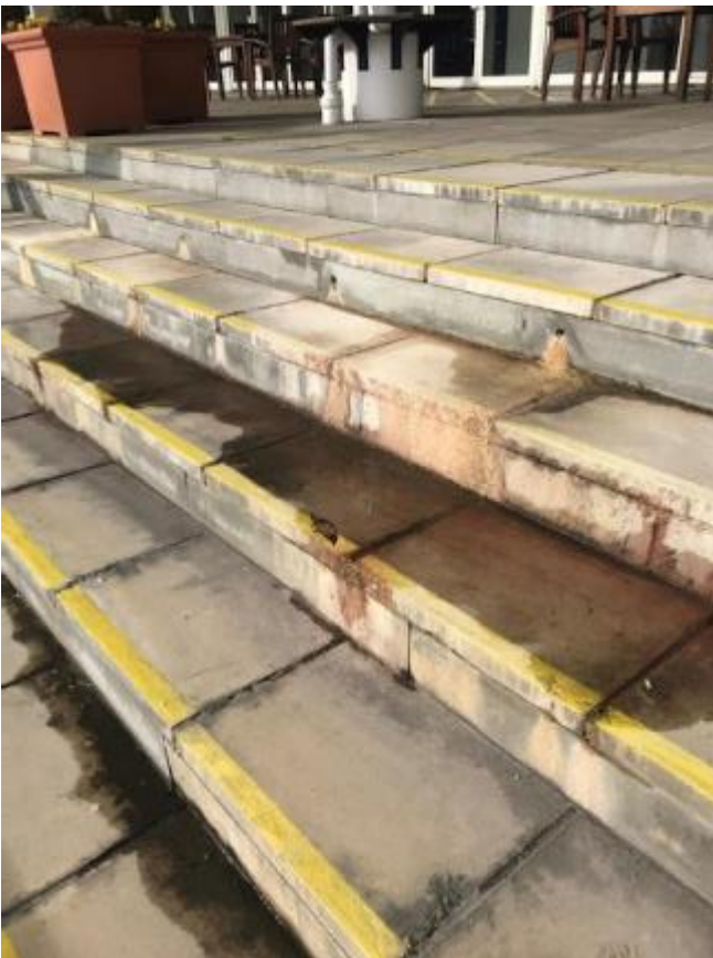
26. Rainwater leaking through the terrace pavings and steppings causing water ingress below.
