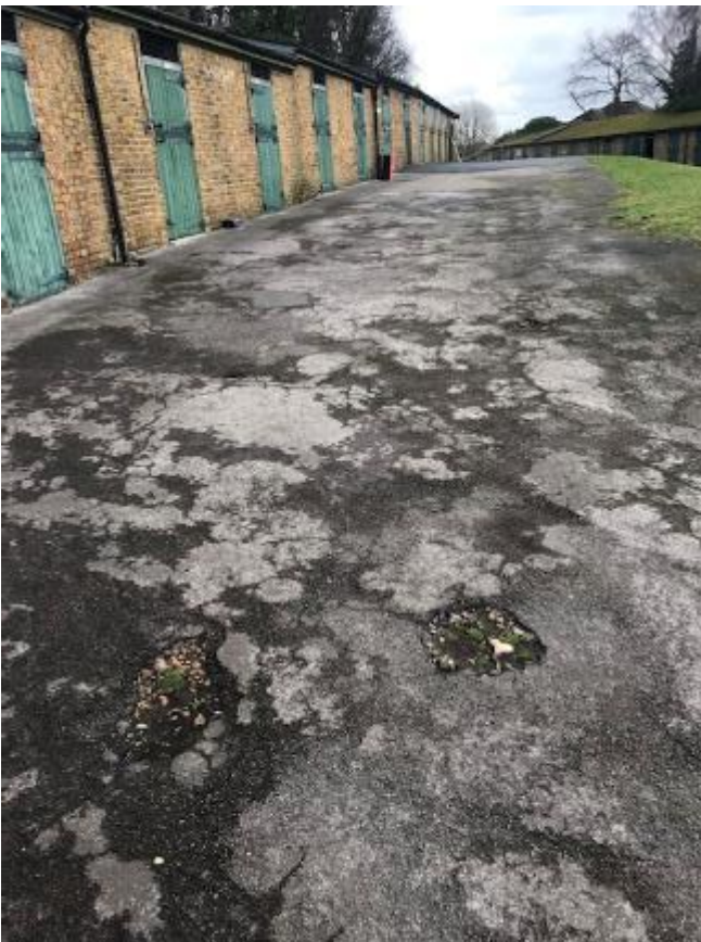
254. Yard surface is breaking up adjacent to stables 104-110.
