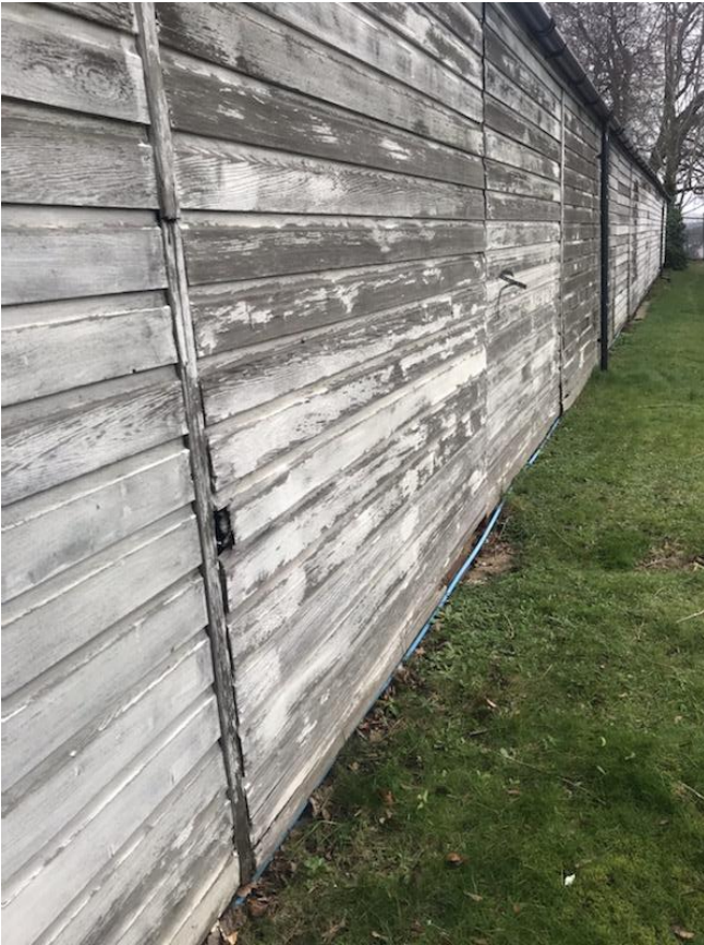
263. Rear elevation of saddling boxes in poor decorative order with some wet rot to the timber cladding.
