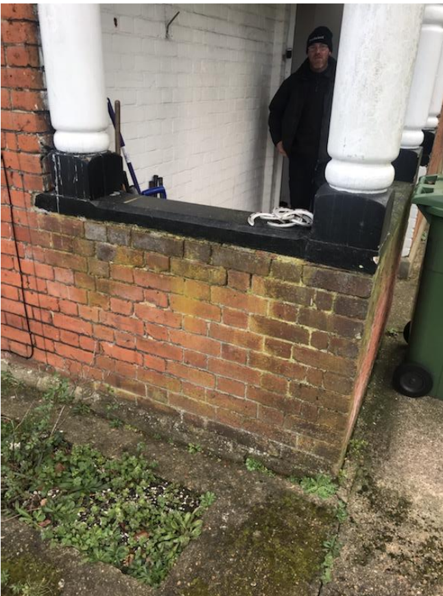
268. Damp stained and patch repointed external brickwork.
