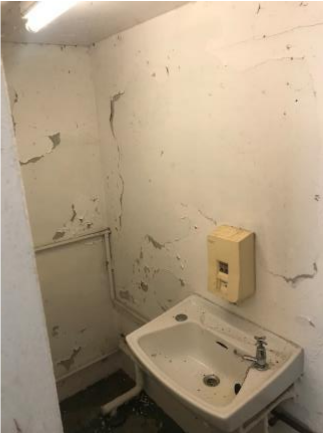
257. Damp walls and peeling paintwork to Stable Toilet.
