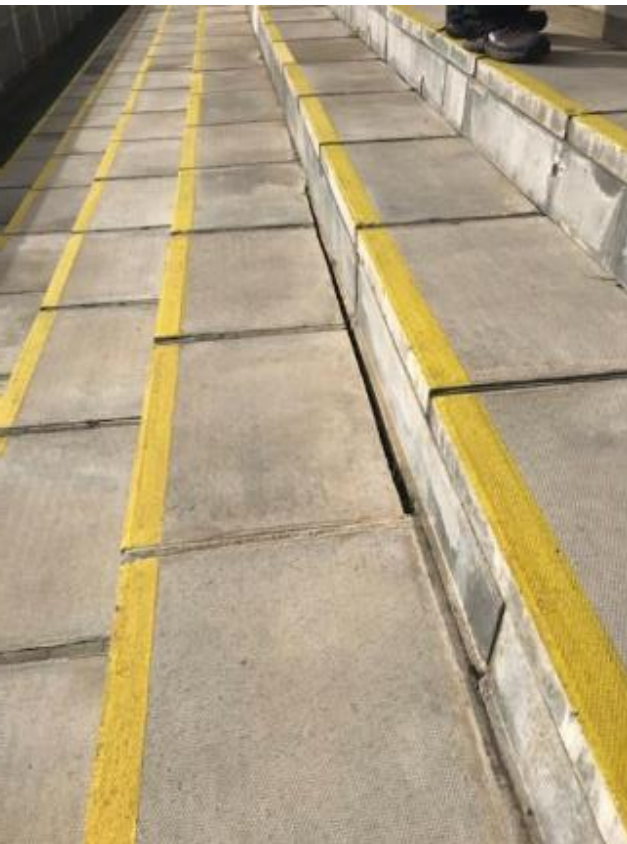
28. Open joints between Terrace and stepping pavings due to thermal movement and causing internal water ingress below.
