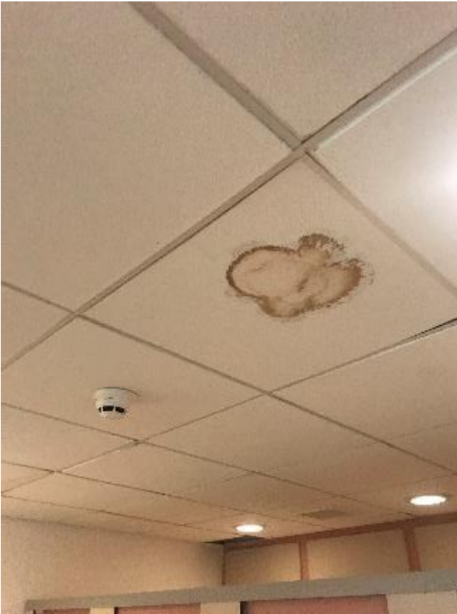
129. Example of water stained ceiling tiles in Ladies Toilets.
