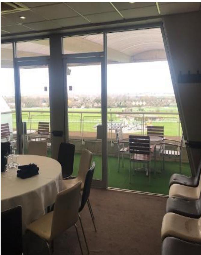
140. Typical view of Second Floor Box. Note : single glazed windows and doors are draughty and offer poor energy efficiency.
