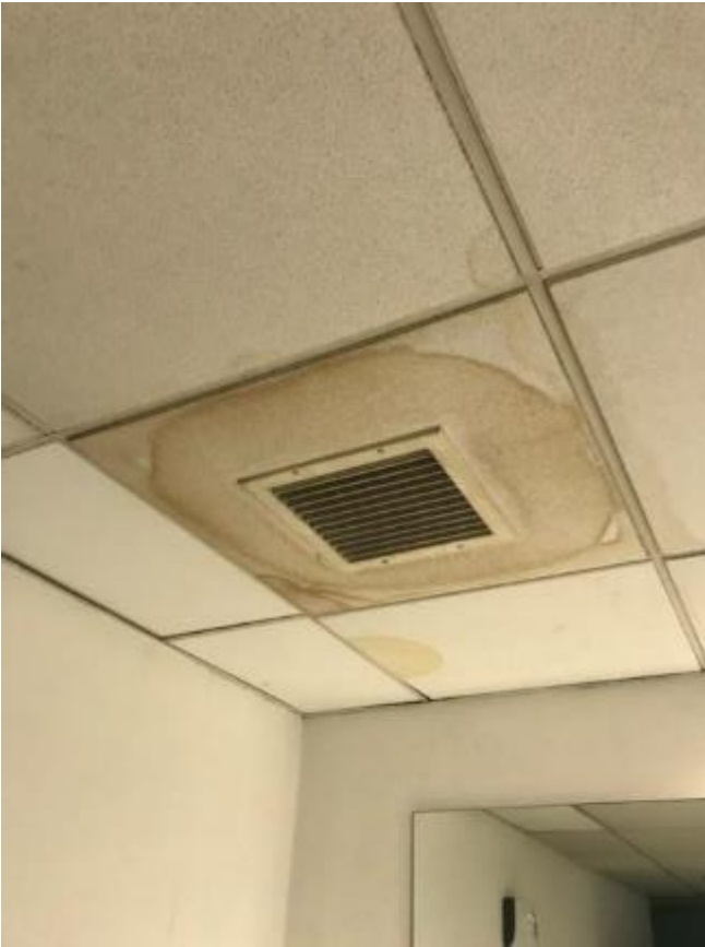
55. Example of stained ceiling tiles from leaks in Gents Toilets.
