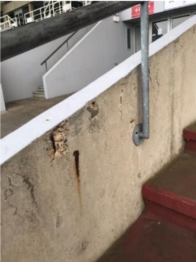
16. Example of spalling concrete retaining walls with exposed corroded steel reinforcement bars.
