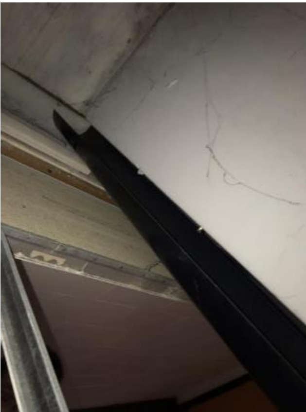
42. An example of the underlining and guttering installed above ceilings in an attempt to manage the extensive leaks through the steppings above.
