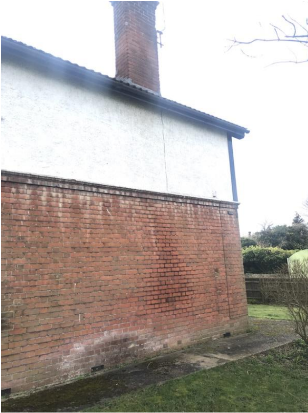
271. Damp and perished mortar pointing in the location of the chimney breast and at low level.
