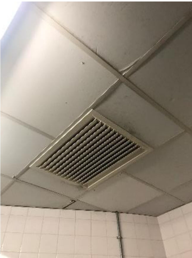
106. Example of ceiling tiles replaced following water ingress.
