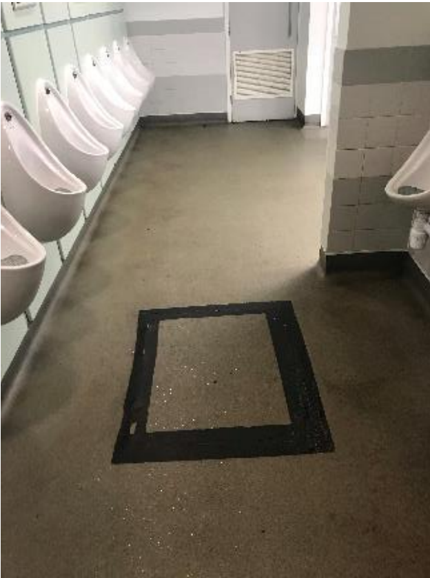
95. Heavy staining and patch repairs to vinyl floor around drainage access cover to Gents Toilets.
