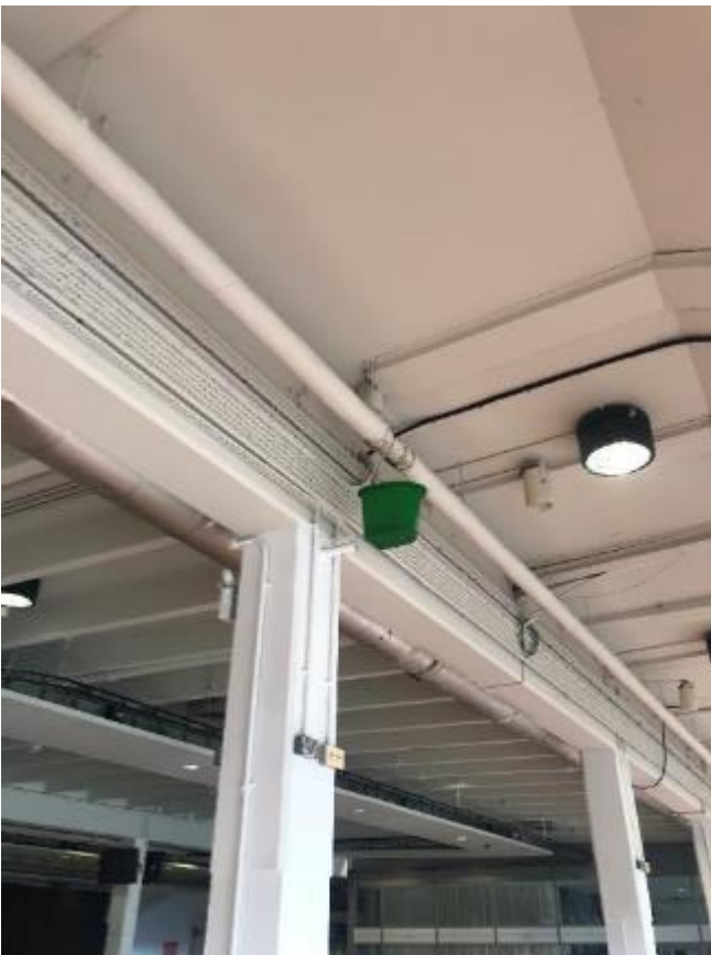
70. Buckets suspended from ceiling soffit to deal with persistent leaks.
