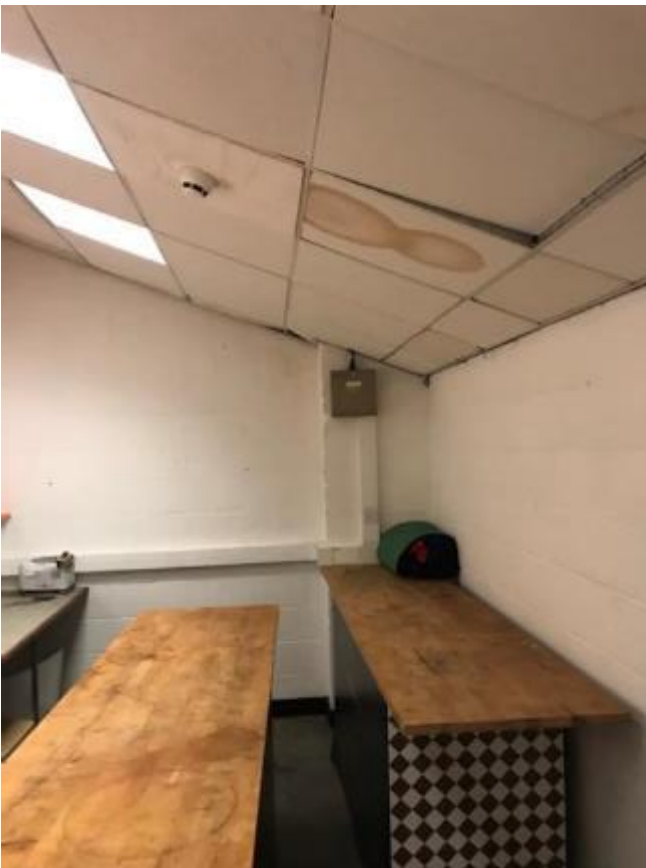
34. Leaks to ceiling tiles.
