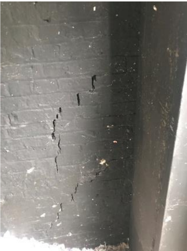
246. Cracked wall between stable 19 and stable 18.
