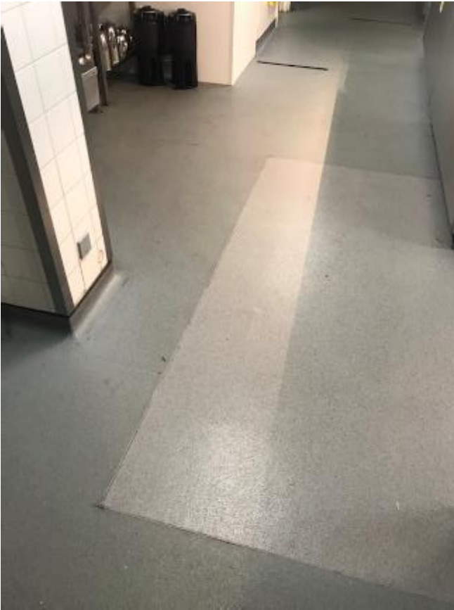
153. Example of soiled and patch repaired vinyl floor covering to second floor kitchen.
