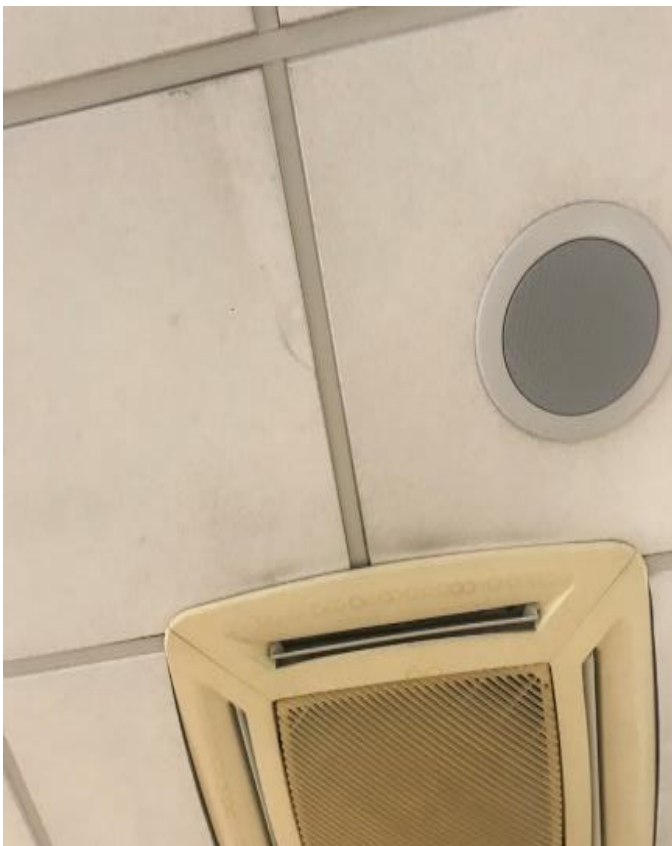
138. Close up of heavy soiling to ceiling in lobby area.
