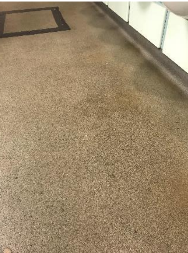
96. Heavy staining and patch repairs to vinyl floor around drainage access cover to Gents Toilets.
