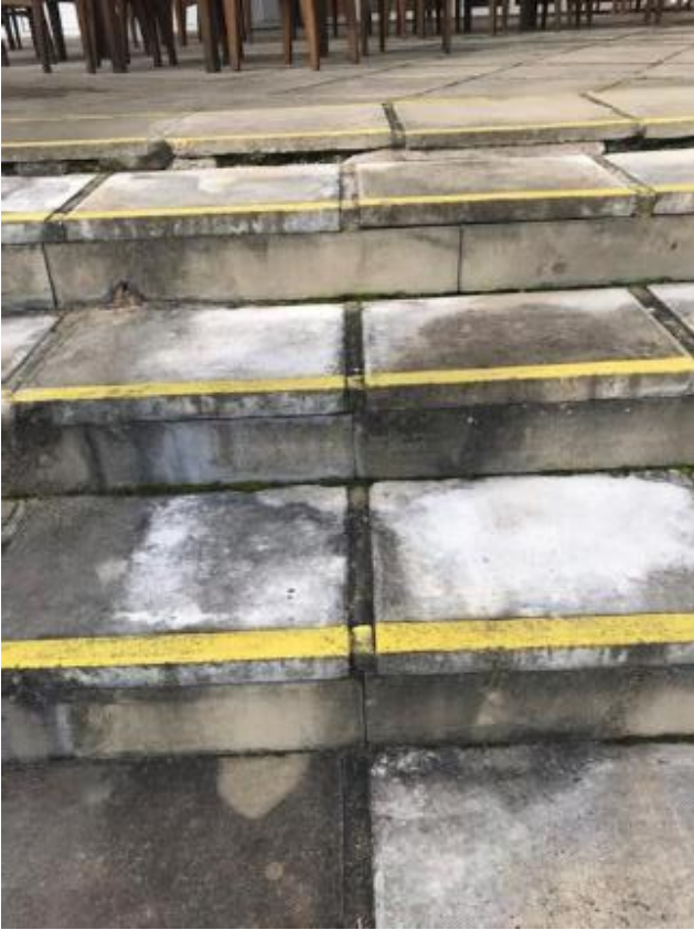
29. Open joints between Terrace and stepping pavings due to thermal movement and causing internal water ingress below.
