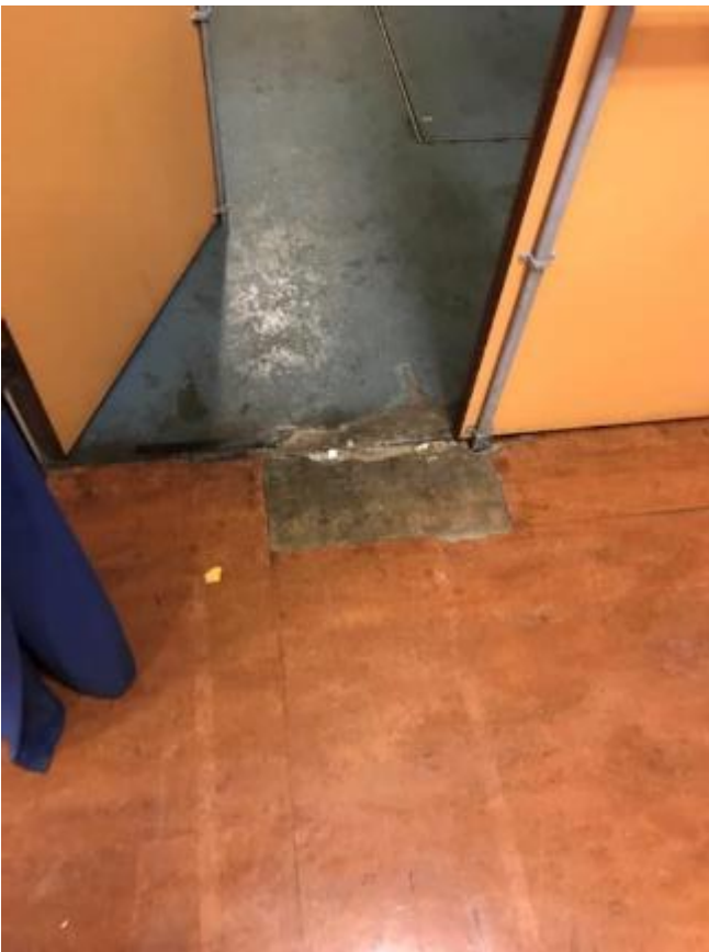
48. Example of damaged flooring adjacent to back of house/fire exit doors.
