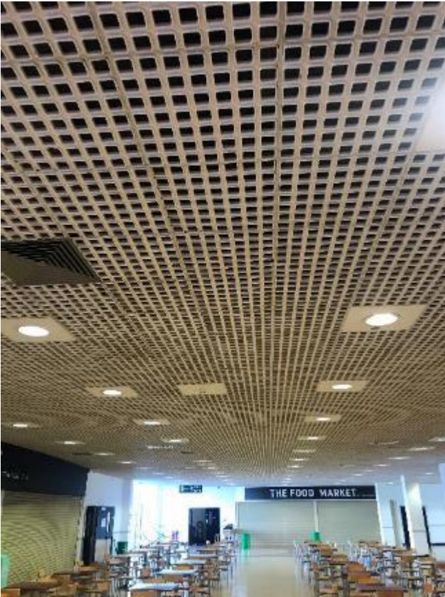
77. Dated stained and damaged ceiling to Food Court Area.
