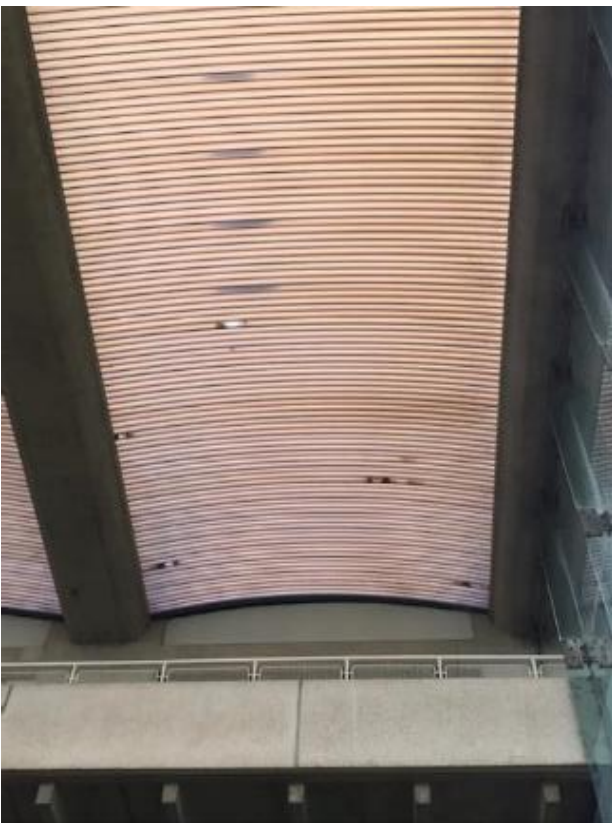
6. Typical view of the underside of the barrel vault canopy sections of roof indicating the damage to the brittle polycarbonate elements.
