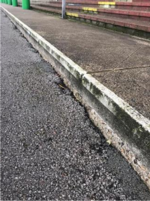
15. Consistent gap between tarmacadam hardstanding and Grandstand concrete stepping, likely to be caused by differential movement
