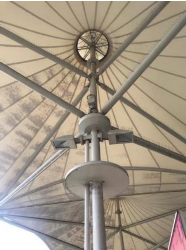
18. Soiled and degraded fabric canopy structure over terrace with leaking rainwater hoppers and pipework.
