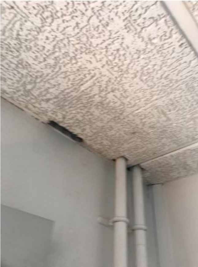
189. Close up example of damage to dated ceiling tiles.
