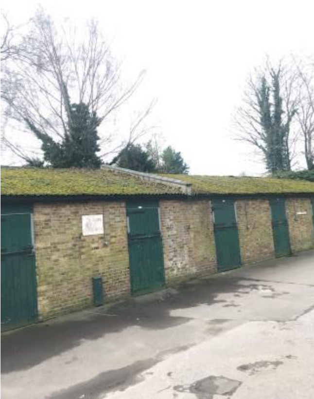
238. Substantial moss cover to brittle asbestos cement stable roofs.
