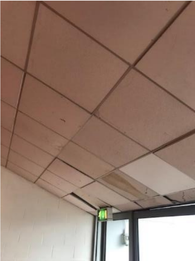
37. Leaks to ceiling tiles and ceiling tiles replaced where previously water damaged.
