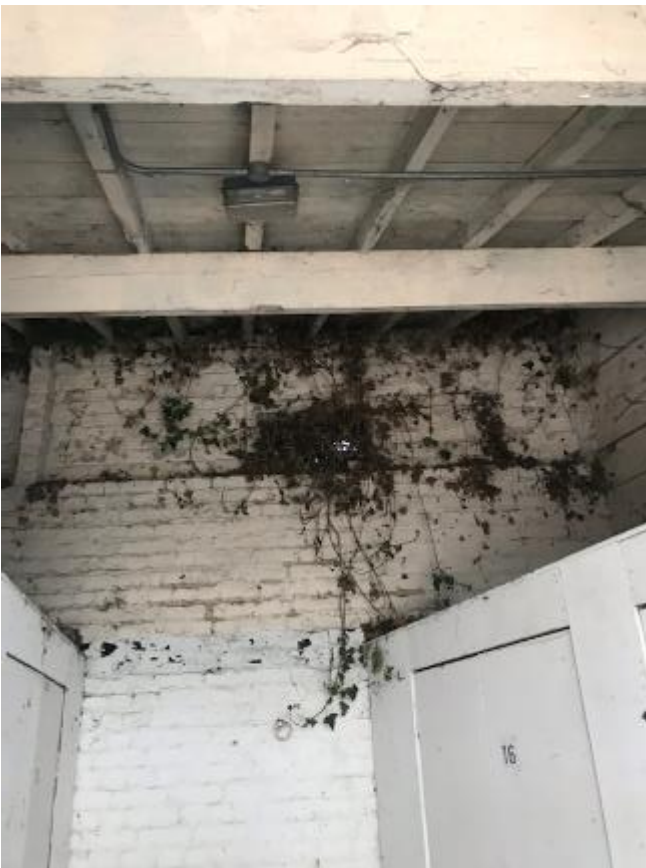
252. Vegetation growth through eaves and onto rear wall of Tack Boxes 13-18.
