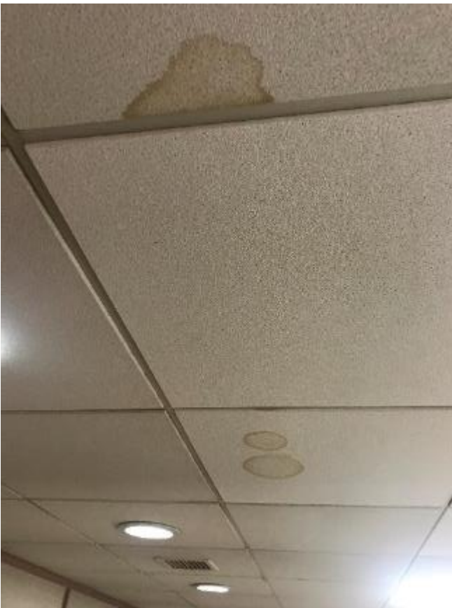
88. Example of water stained ceiling tiles in Ladies Toilets.
