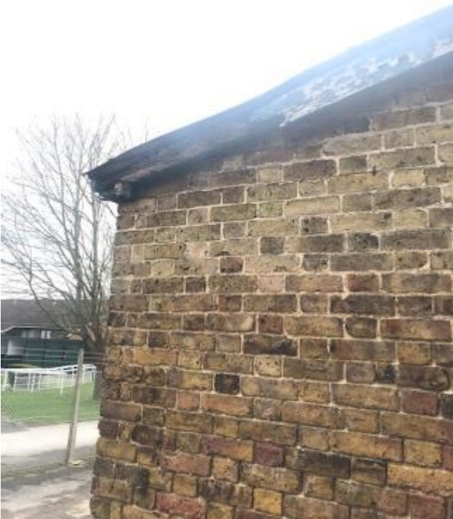
215. Barge boards and fascias are in poor decorative order with some wet rot/missing sections of timber.
