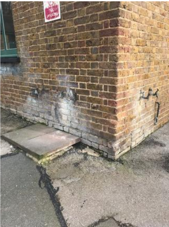
230. Decorations and brickwork to the gable elevation of stable 72 are in poor condition.
