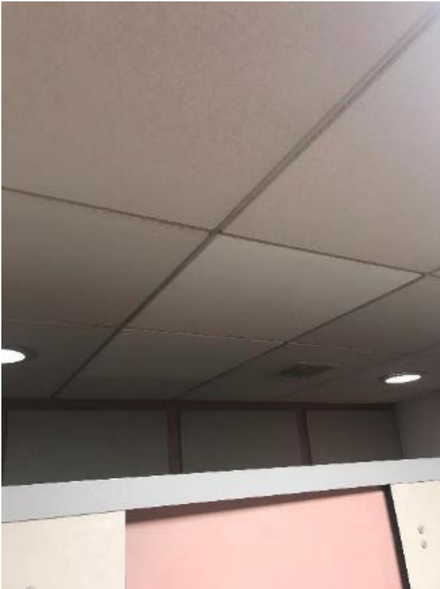
89. Example of replacement stained ceiling tiles which are non-matching due to age of surrounding tiles in Ladies Toilet.
