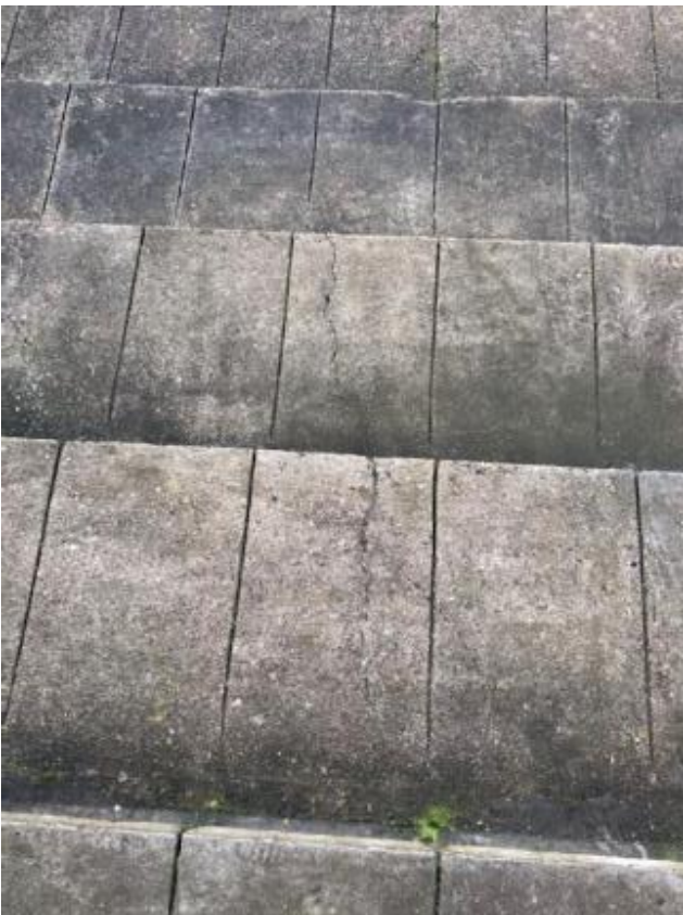
12. Example of cracked concrete steppings causing water ingress internally.
