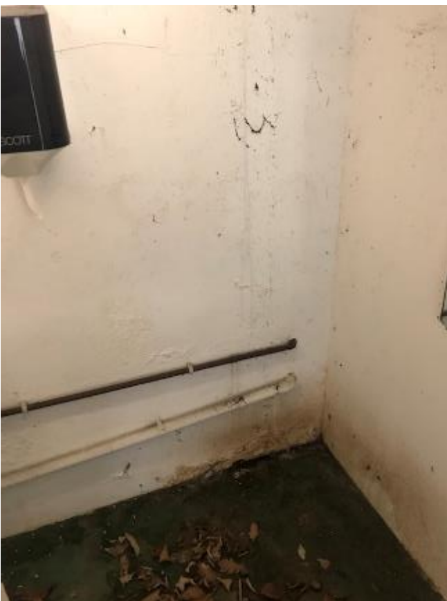
258. Damp walls and peeling paintwork to Stable Toilet.
