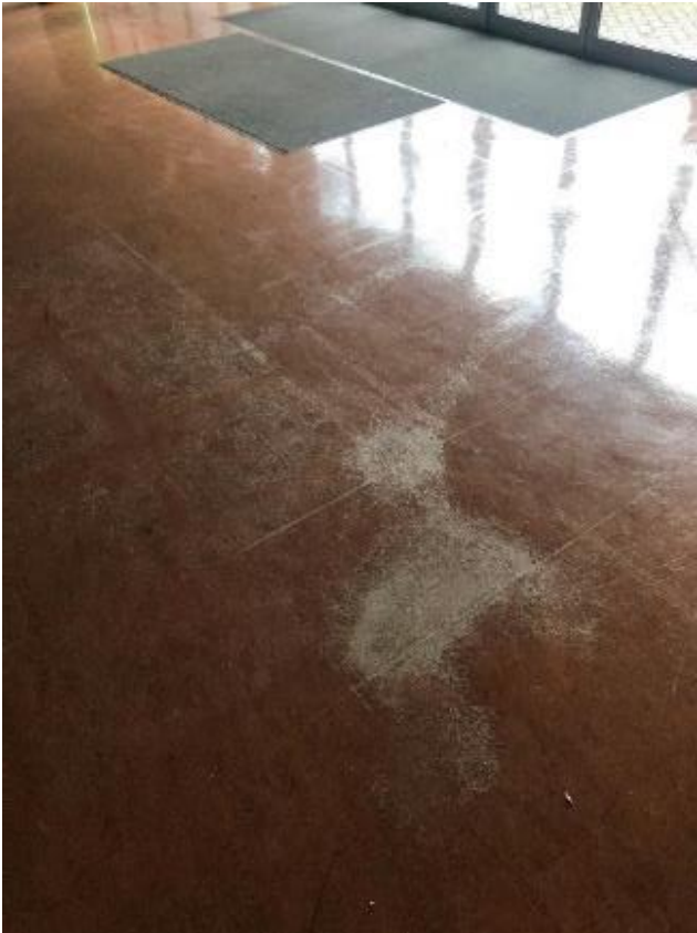
81. Example of heavily stained floor vinyl due to persistent leaks from Parade Ring Terrace.
