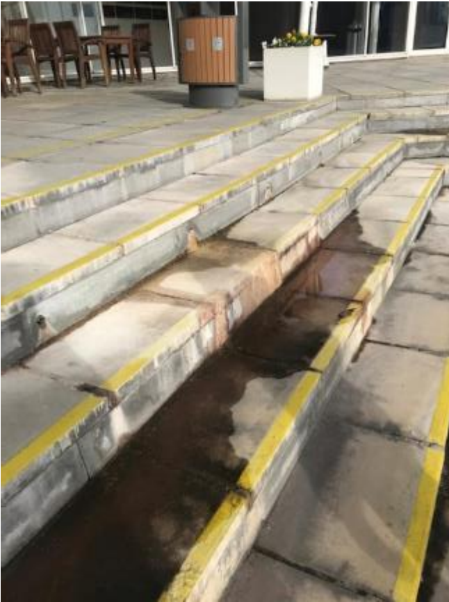
25. Rainwater leaking through the terrace pavings and steppings causing water ingress below.
