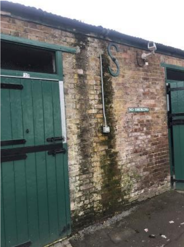
237. Leaking gutter, rotten fascia, damp and perished brickwork between stables 38 and 39.
