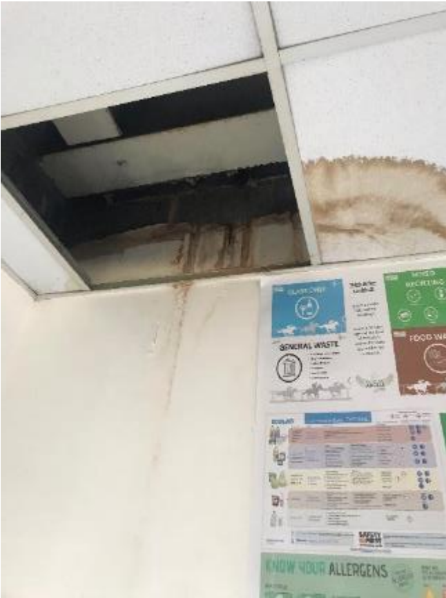
69. Missing ceiling tile and visible leaks.
