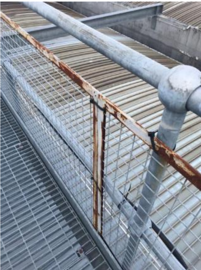
10. Example of typical corrosion to external metalwork/handrails.
