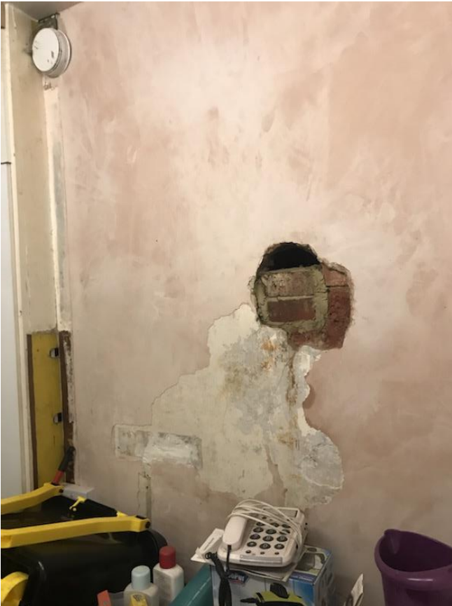
279. Damp plaster and brickwork to chimney breast.
