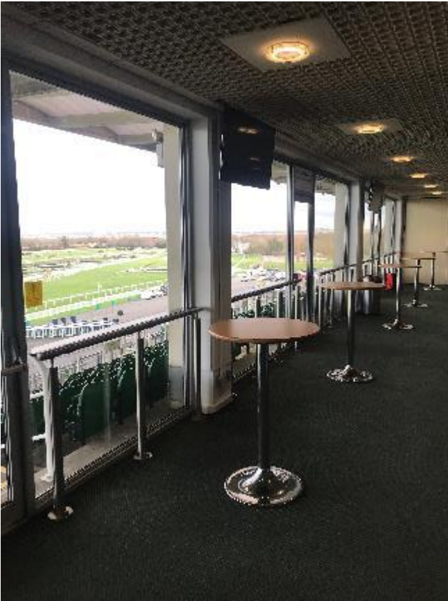
121. Large single glazed windows and doors are draughty with poor energy efficiency rating.
