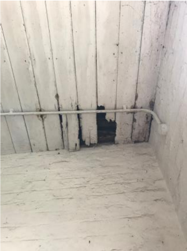
251. Lining soffit is rotten in part to stable 57.
