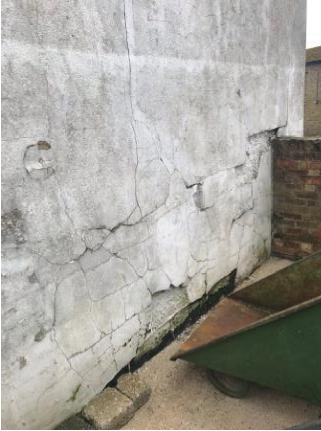
261. Cracked and blown render to gable elevation of Tack Boxes 7-12.
