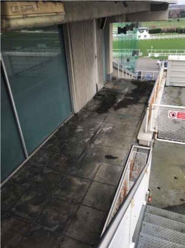
175. External escape stairwell from second floor terrace. Note: corrosion to balustrades and staining to pavings from roof/terrace leaks.
