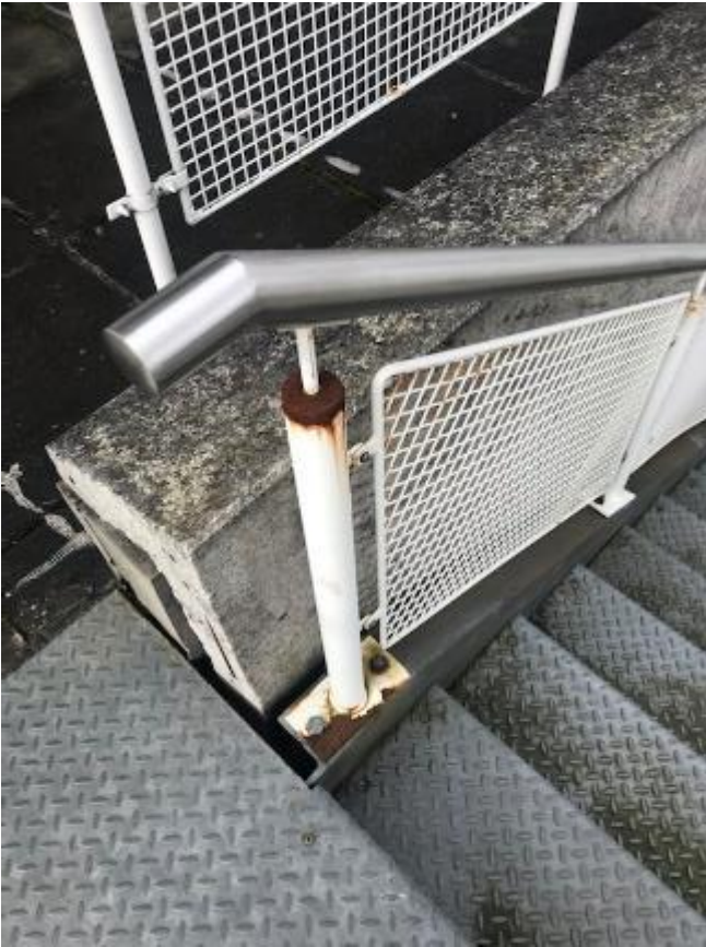
173. External escape stairwell from second floor terrace. Note: corrosion to balustrades.
