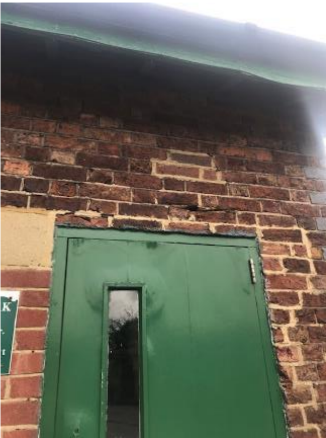
226. Patch repaired and cracked brickwork to Stable Managers Office.
