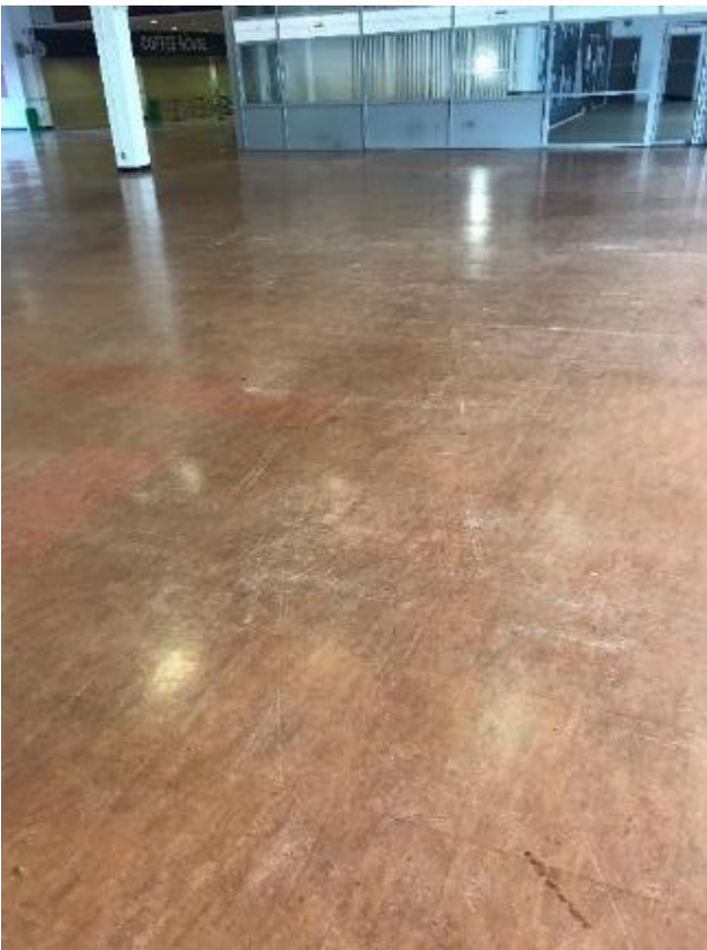
84. Consistently worn and discoloured vinyl floor in need of replacement.
