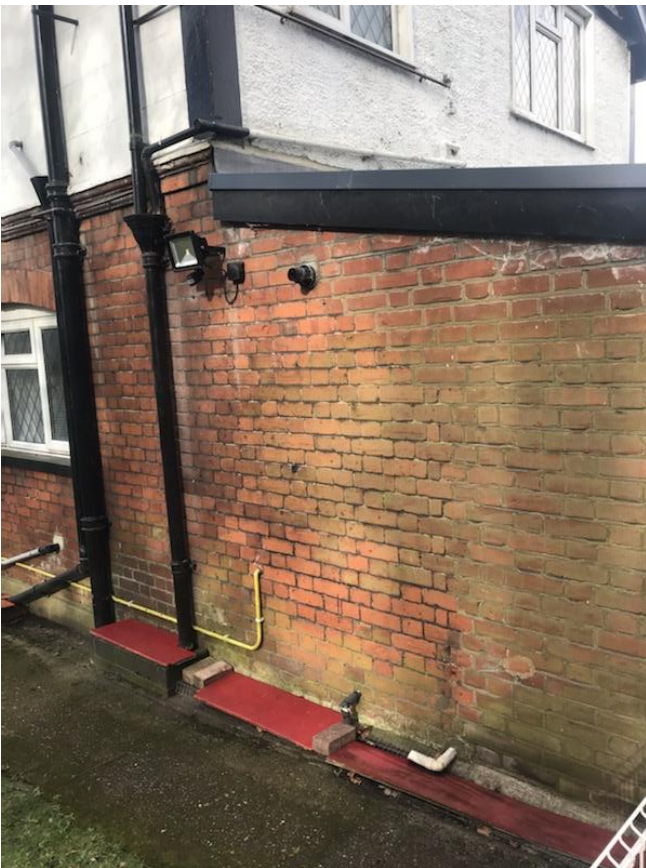
274. Damp stained and patch repaired brickwork to side elevation of lean-to extension.
