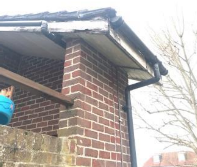
182. Fascias and soffits are in poor decorative order and partially rotten.
