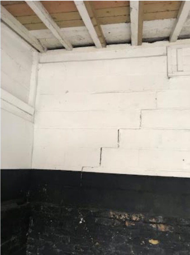
249. Stepped cracking to rear wall of stable 48.
