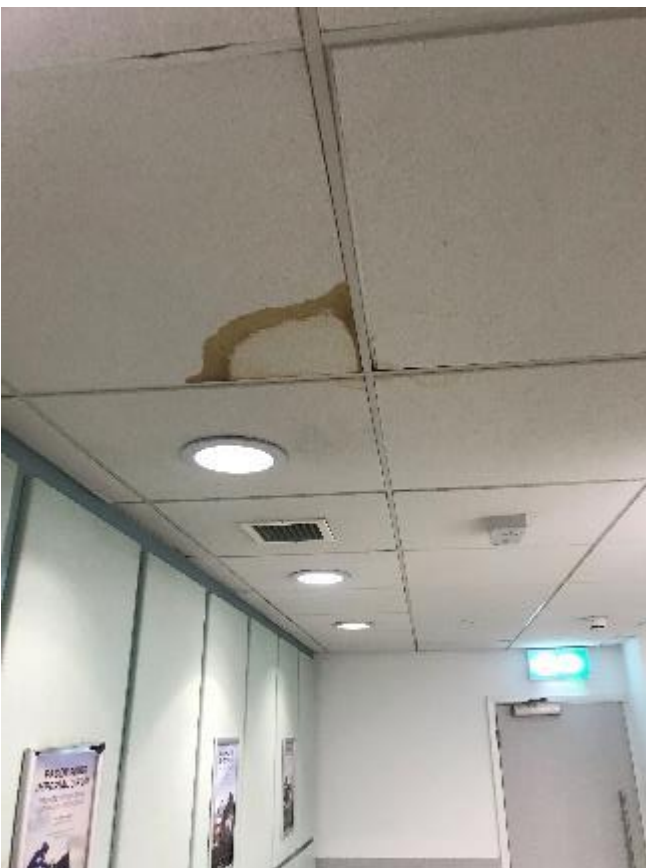
94. Example of water stained ceiling tiles in Gents Toilets.
