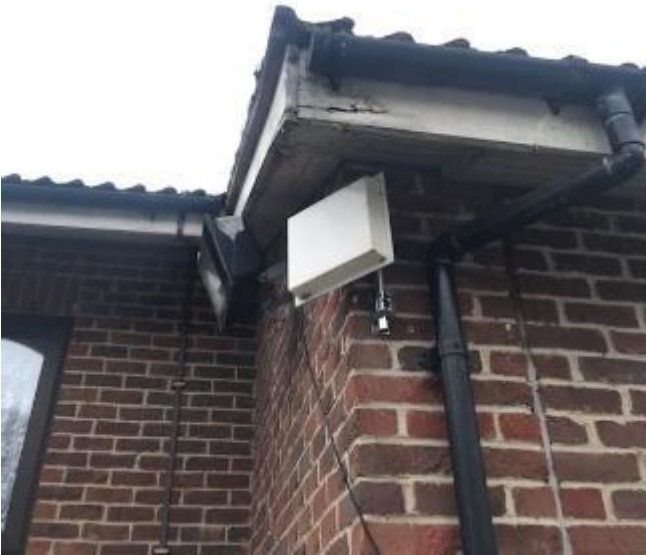
181. Fascias and soffits are in poor decorative order and partially rotten.
