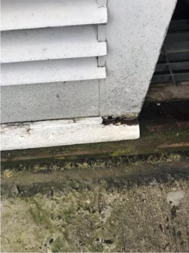
11. Example of rotten timber to external joinery/plant room doors.
