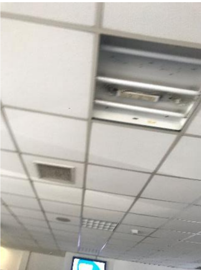
110. Example of faulty light fitting.
