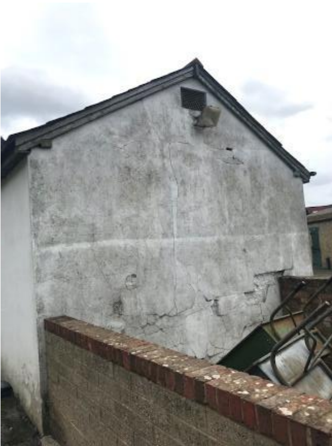
260. Cracked and blown render to gable elevation of Tack Boxes 7-12.
