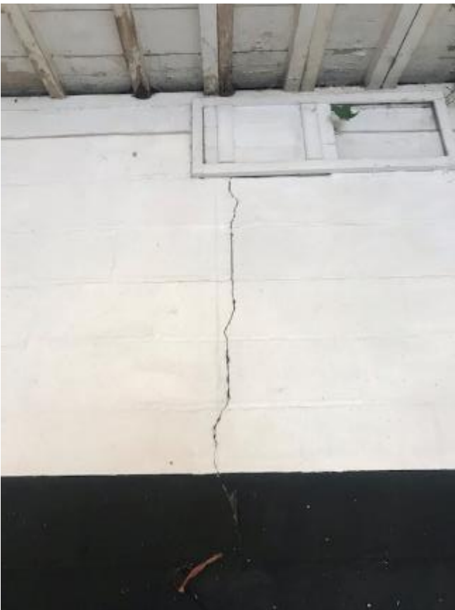
232. Cracking to rear wall of stable 50.
