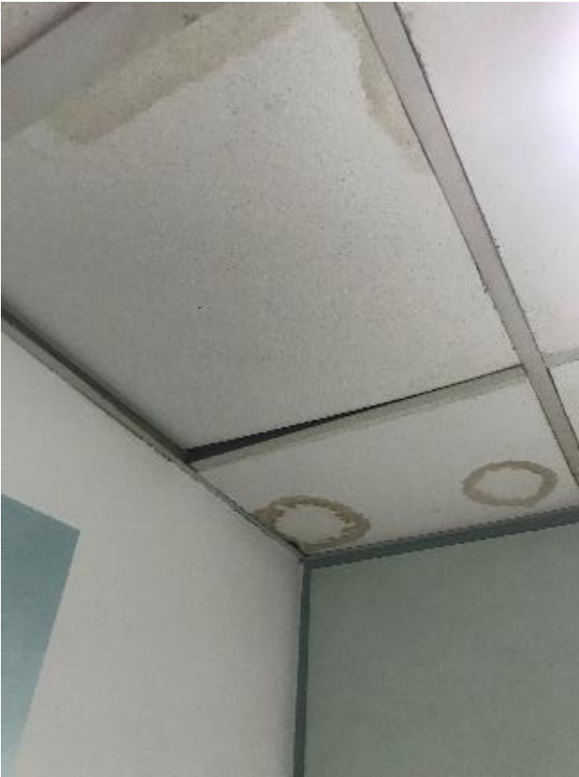
157. Example of stained ceiling tiles from roof leaks to Gents Toilets.
