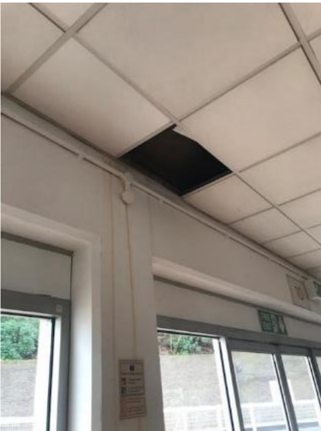
74. Water damaged ceiling tiles removed adjacent to doors below Parade Ring Terrace. Note: also run marks on wall from leaks.
