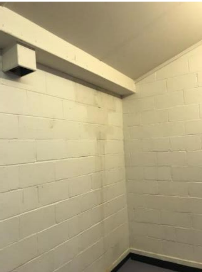
40. Damp staining to wall grinning through the painted finish.
