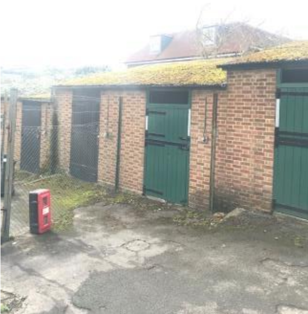
214. Stable Block 56-69. Note : substantial moss/vegetation cover to the brittle asbestos cement roofs.
