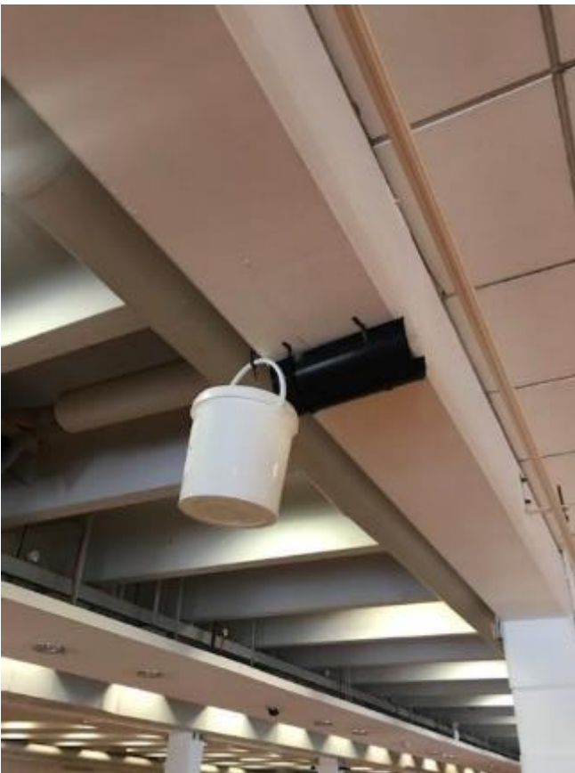
38. Example of bucket placed at ceiling level to deal with persistent leaks.
