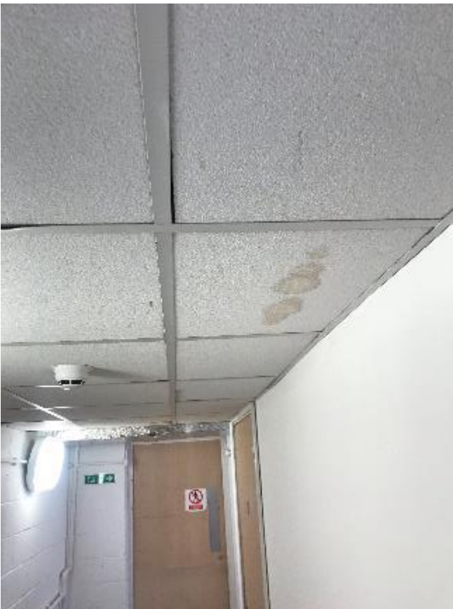
170. Example of stained ceiling tiles in second floor escape corridor.
