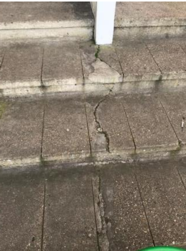
14. Example of cracked concrete steppings causing water ingress internally.
