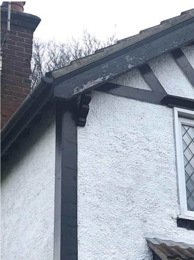
270. Peeling decorations to fascia/barge boards.
