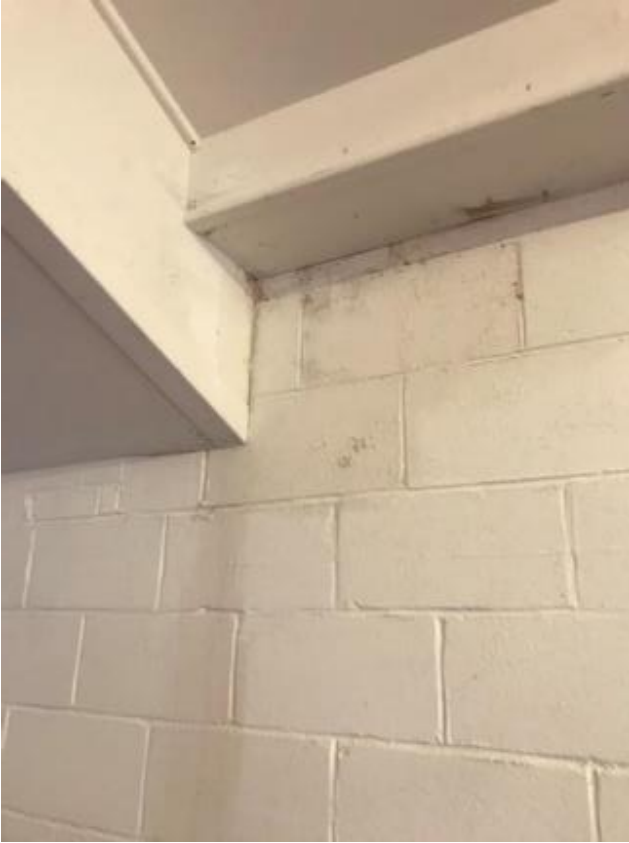
41. Damp staining to wall grinning through the painted finish.
