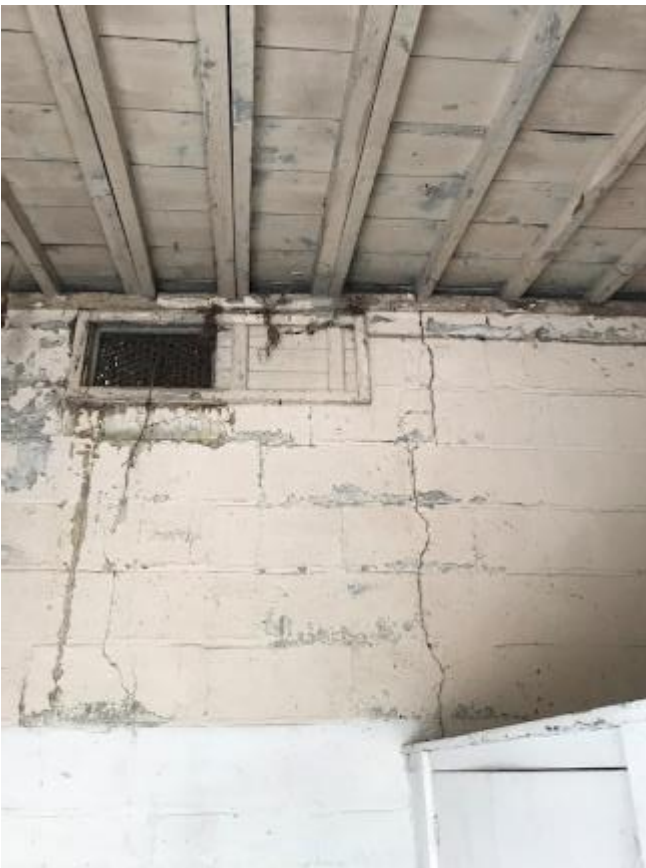
250. Cracked rear wall to Tack Boxes 1-6 together with peeling paintwork to timber soffit and blockwork wall.
