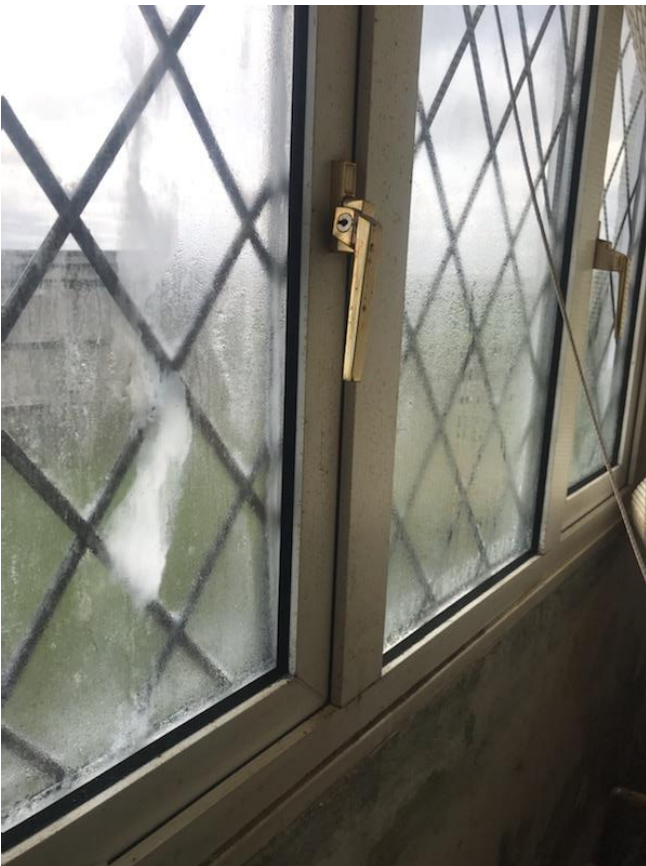
284. Condensation to double glazed windows.
