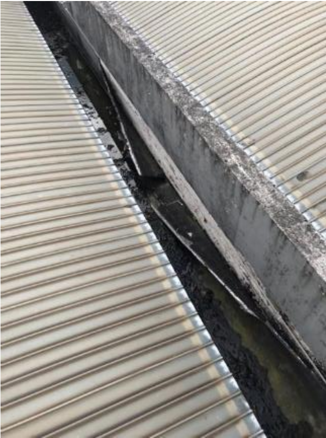
9. Close up of typical failed/delaminating gutter linings.
