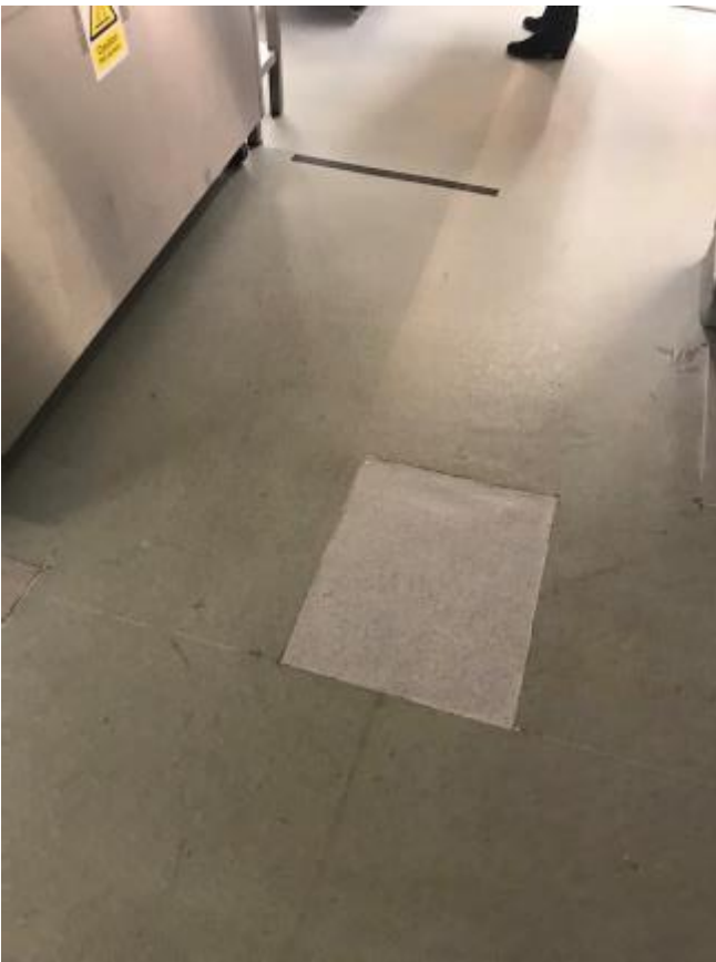
152. Example of soiled and patch repaired vinyl floor covering to second floor kitchen.
