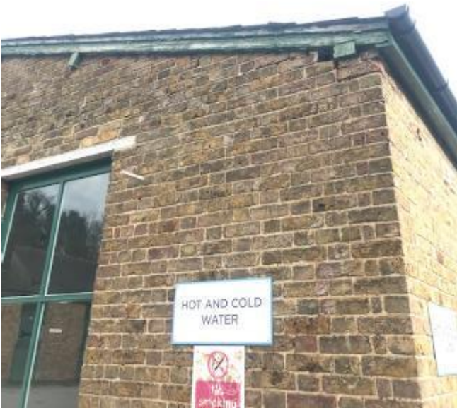
231. Decorations and brickwork to the gable elevation of stable 72 are in poor condition.
