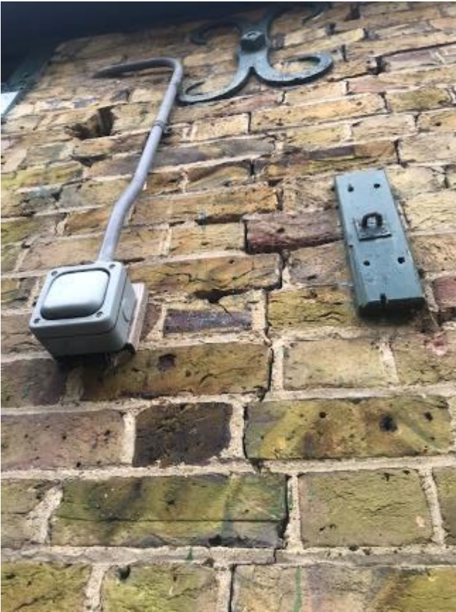
245. Cracked and damaged brickwork to front wall of stable 19.
