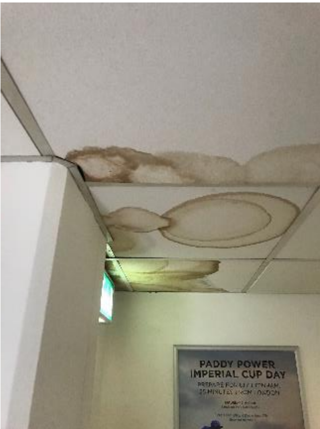
158. Example of stained ceiling tiles from roof leaks to Gents Toilets.
