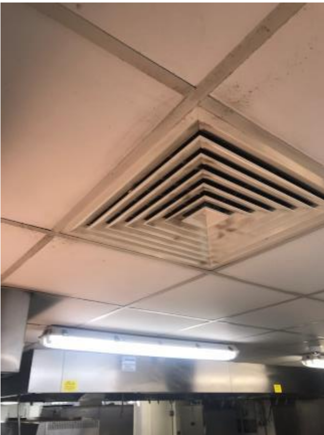
150. Close up of soiled ceiling and grille to second floor kitchen.
