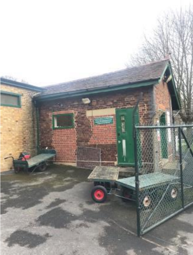
225. Patch repaired and cracked brickwork to Stable Managers Office.
