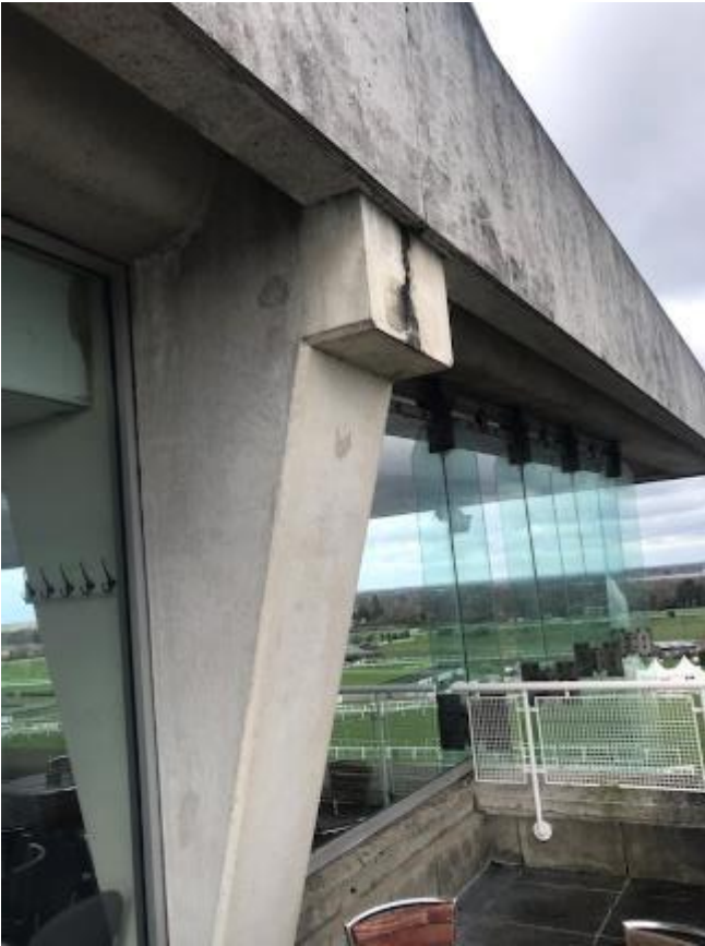
171. Leaks from roof/parapet onto second floor and terrace adjacent to second floor boxes.
