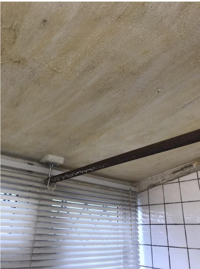
282. Damp ceiling in bathroom to lean to extension
