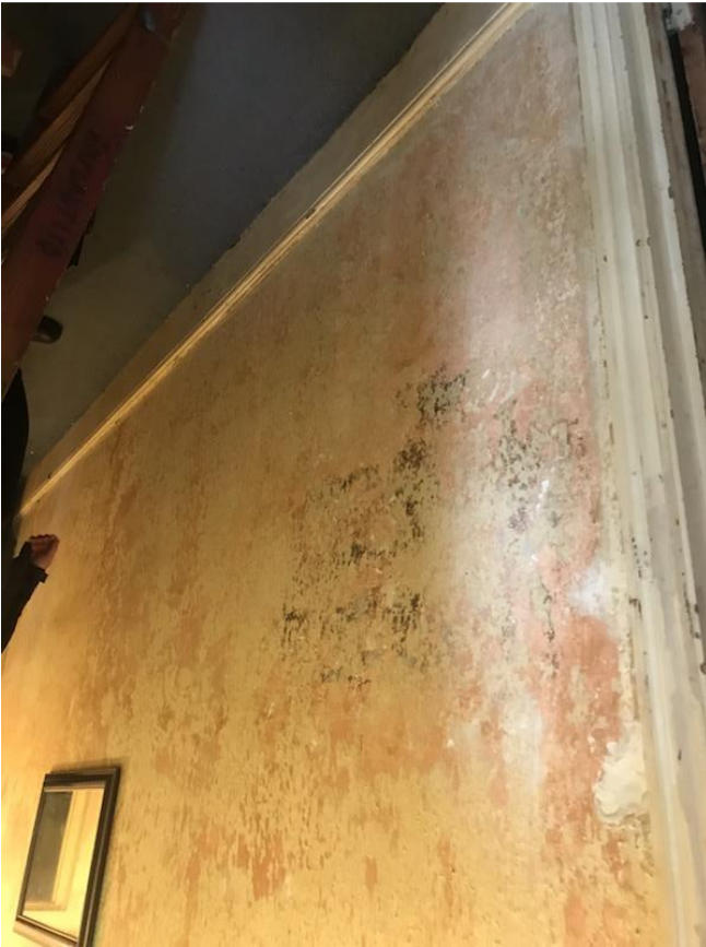
277. Damp to internal walls.
