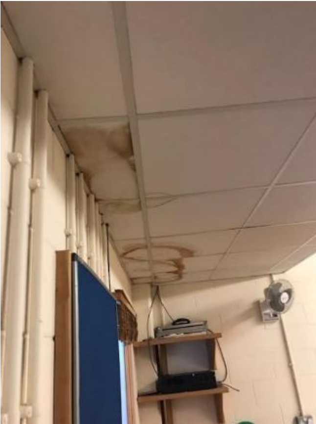
35. Leaks to ceiling tiles.
