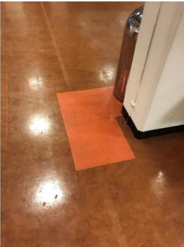
46. Floor covering patch repaired in non-matching colours, as original colour is no longer available.
