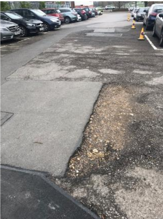
186. Car park surface in the vicinity of Sandown Lodge is breaking up.
