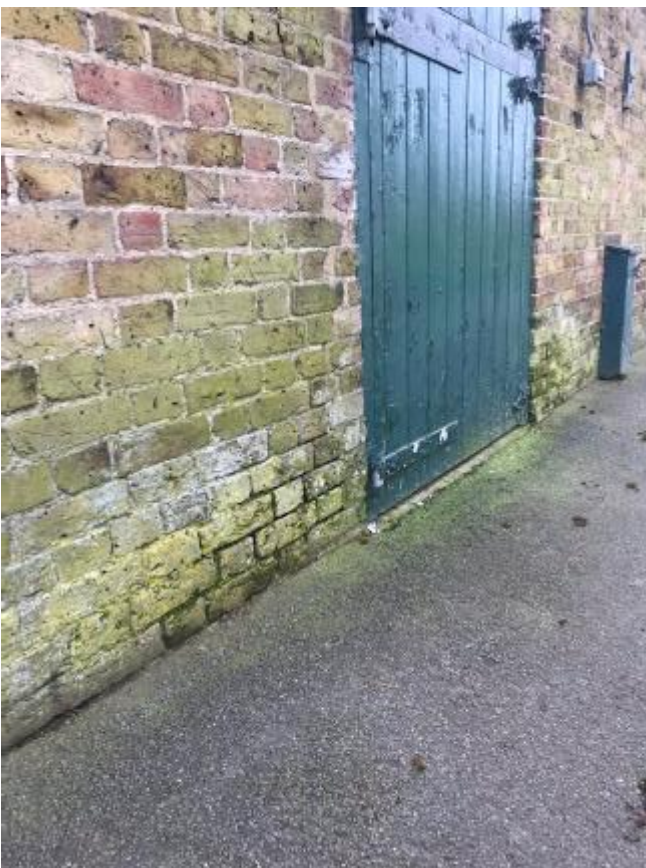
242. Close up of typical example of perished mortar to low level brickwork.
