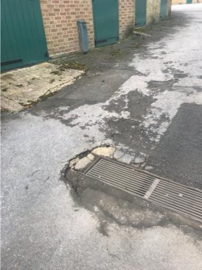
223. The yard surface is breaking up alongside stable block 56 – 69 and a trip hazard for horses and personnel alike.
