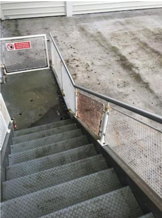
174. External escape stairwell from second floor terrace. Note: corrosion to balustrades.
