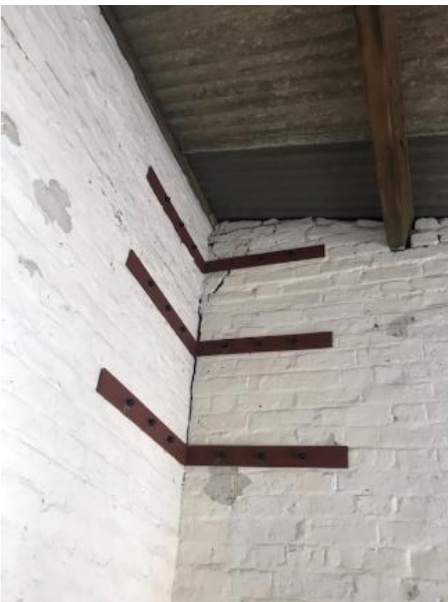
236. Metal strapping applied to restrain rear and side wall of stables 39-42.
