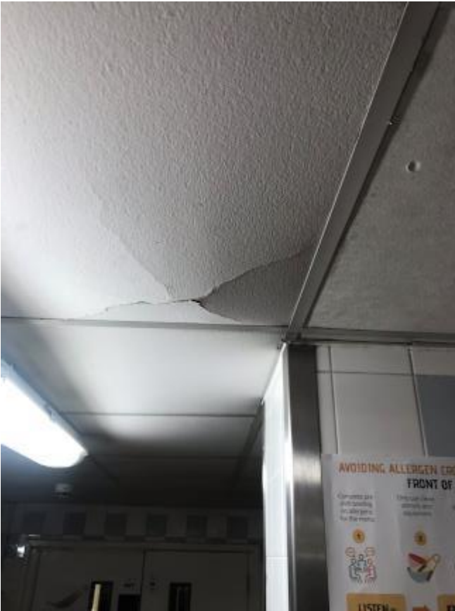
151. Close up of damage to kitchen ceiling.
