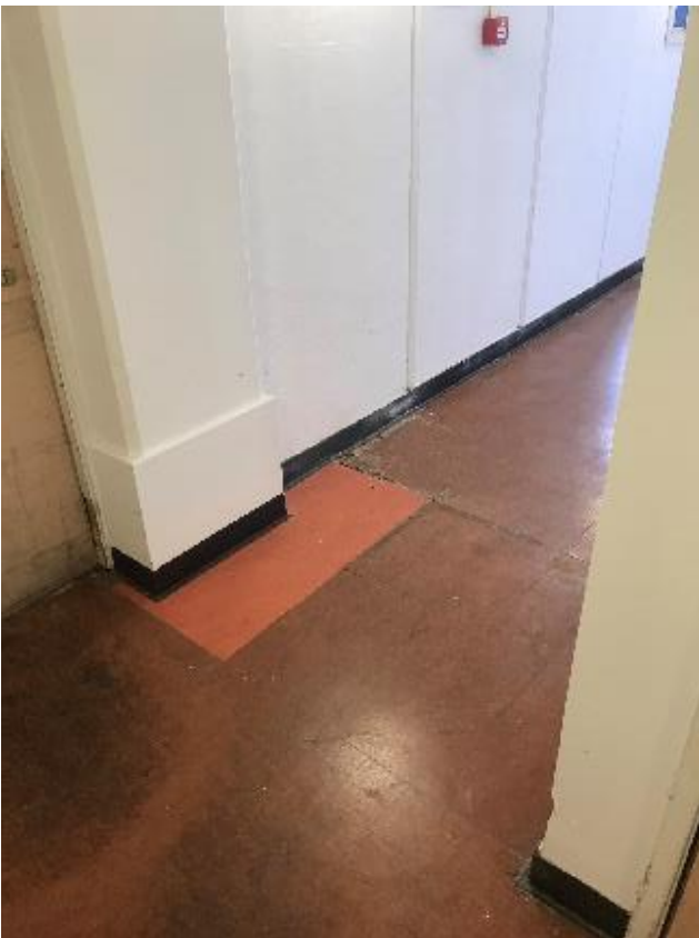
168. Close up of water damaged and patch repaired vinyl floor covering to second floor escape corridor (original colour of vinyl floor covering no longer available).
