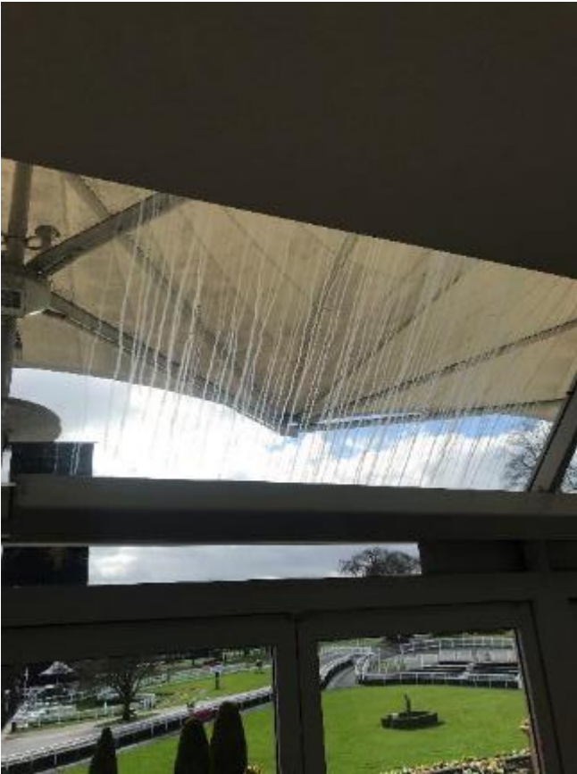
23. Water staining to corridor glazing from leaks from fabric canopy over the terrace.
