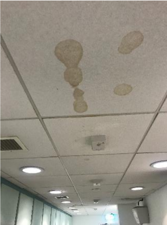
93. Example of water stained ceiling tiles in Gents Toilets.
