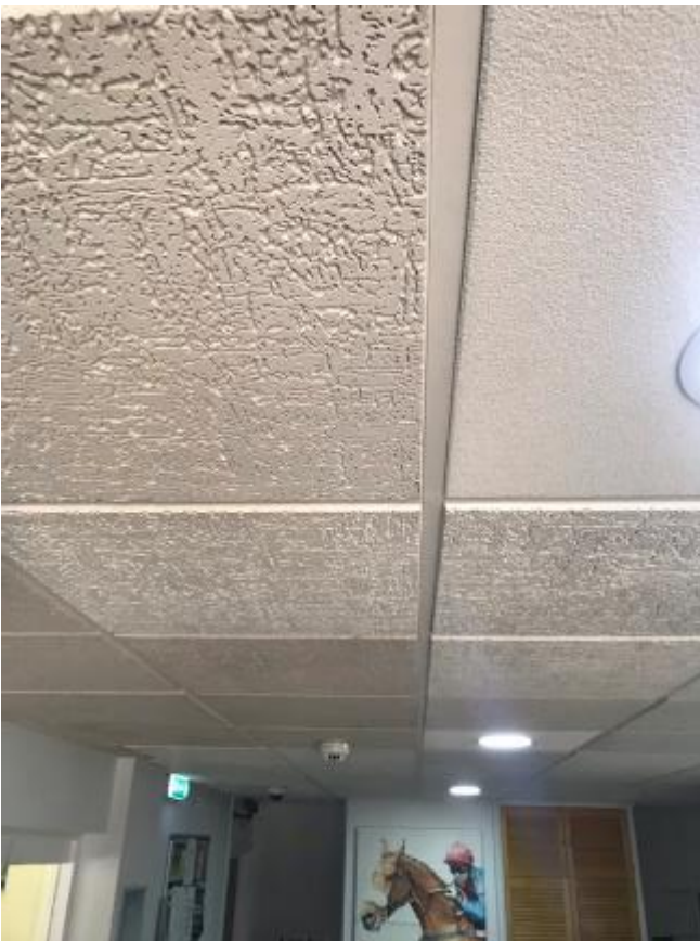
190. Close up example of non-matching ceiling tiles.
