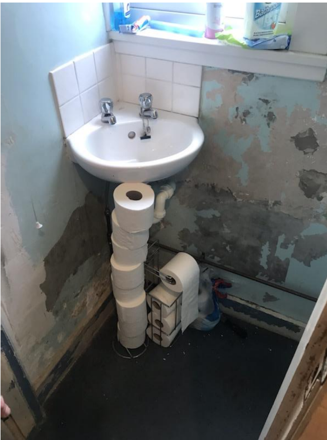
278. Damp plaster to bathroom.
