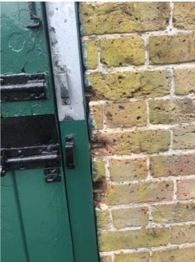
220. The brickwork is crumbling due to the weight of the doors and fixings for the door frames.
