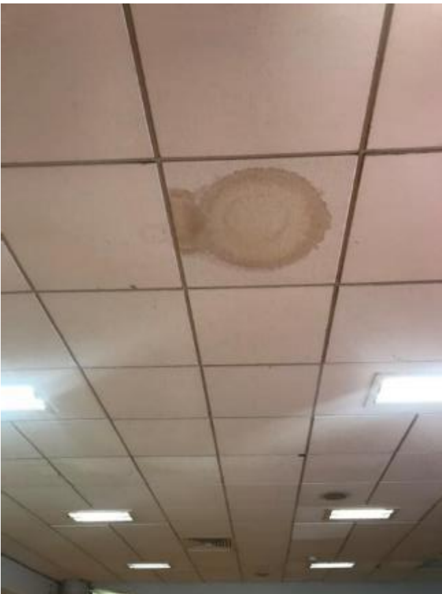
36. Leaks to ceiling tiles.
