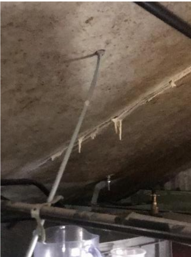
72. Example of buckets strategically placed above ceilings to Champagne Bar to catch leaks.
