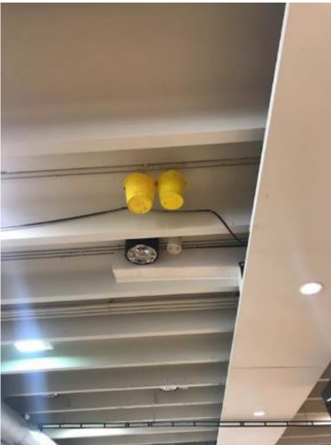
68. Buckets suspended from ceiling soffit to deal with persistent leaks.
