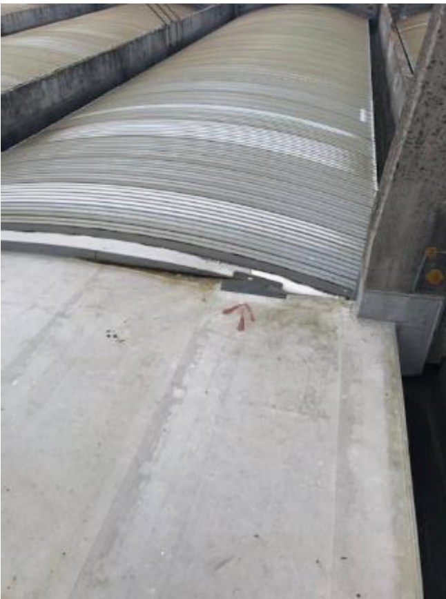
8. Typical example of patch repairs to abutment of flat roof sections and barrel vault canopy sections.
