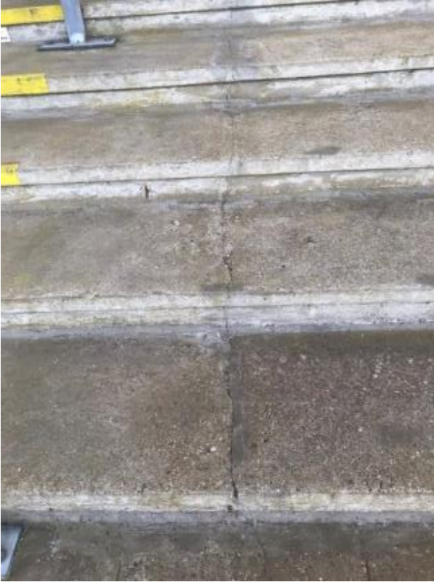
13. Example of cracked concrete steppings causing water ingress internally.
