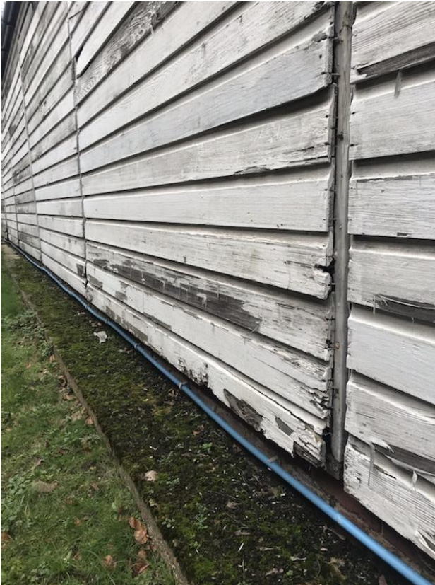
265. Rear elevation of saddling boxes in poor decorative order with some wet rot to the timber cladding.
