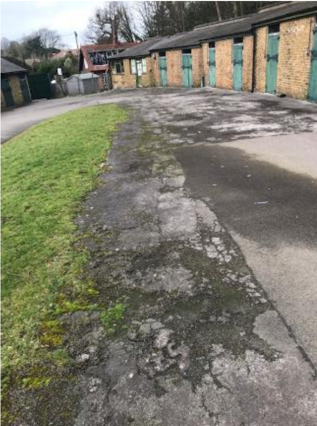
253. Yard surface is breaking up adjacent to stables 104-110.
