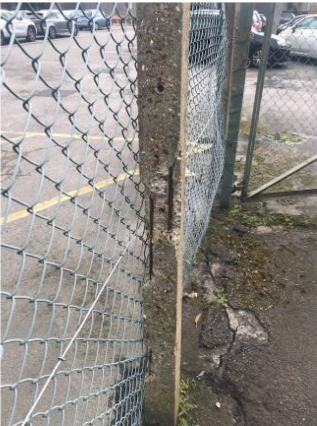
224. The perimeter concrete fence posts are spalling in part exposing the corroded reinforcement.
