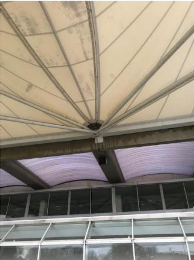
19. Soiled and degraded fabric canopy structure over terrace with leaking rainwater hoppers and pipework.
