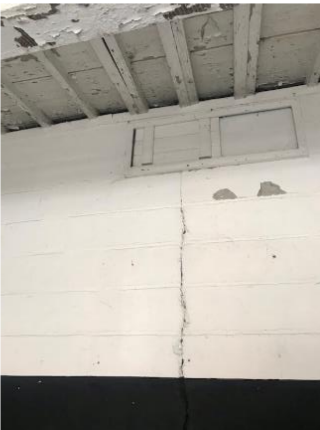
234. Leaking roof, rotten timber soffit and peeling decorations to stable 46.
