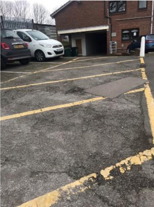
185. Car park surface in the vicinity of Sandown Lodge is breaking up.
