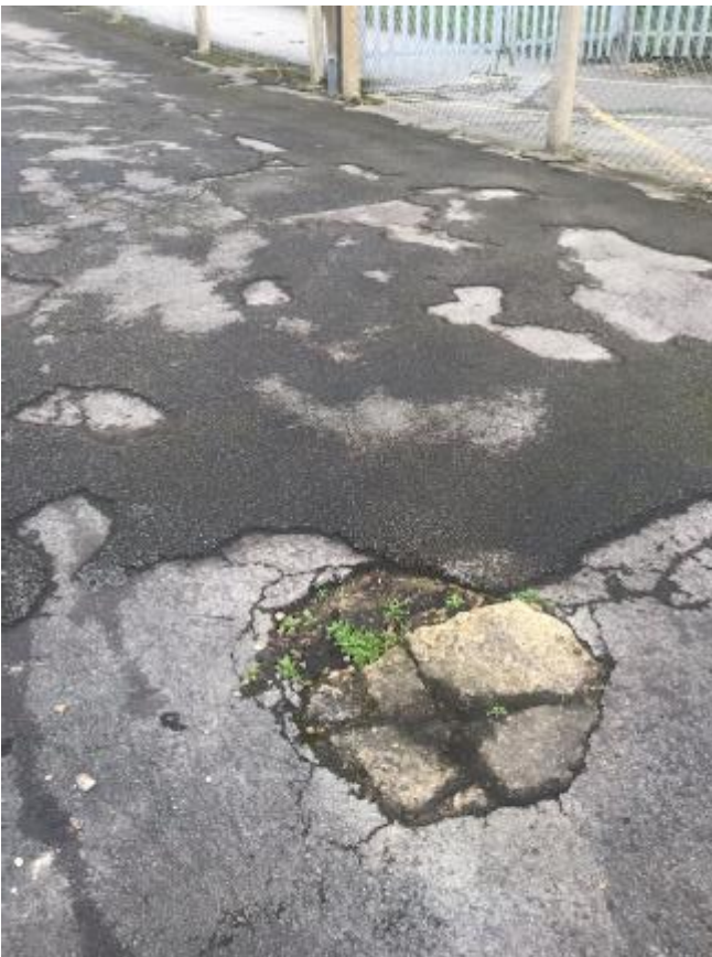
222. The yard surface is breaking up alongside stable block 56 – 69 and a trip hazard for horses and personnel alike.
