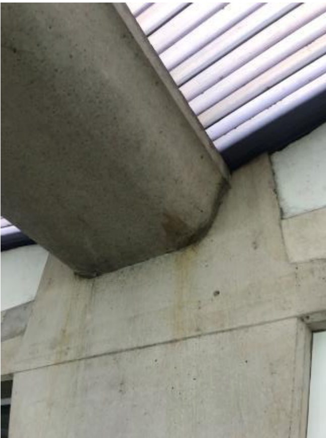
146. Close up example of leaks from Grandstand gutter above balconies to Second Floor Boxes.
