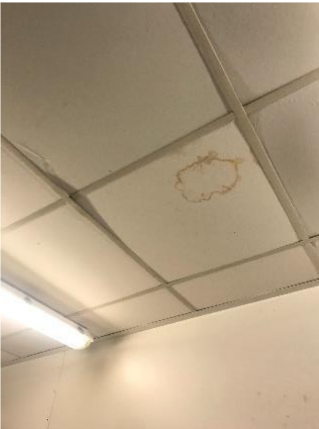
104. Example of water ingress to ceiling.
