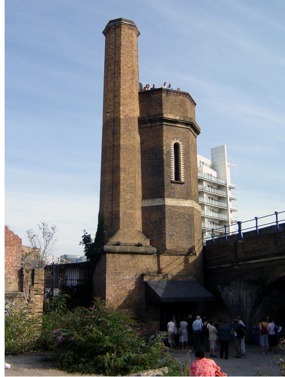
Figure 11: The accumulator tower on the Mill Place site
