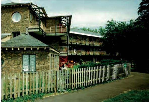
Figure 24: In this housing association scheme, solar shading is provided by balconies and overhangs
