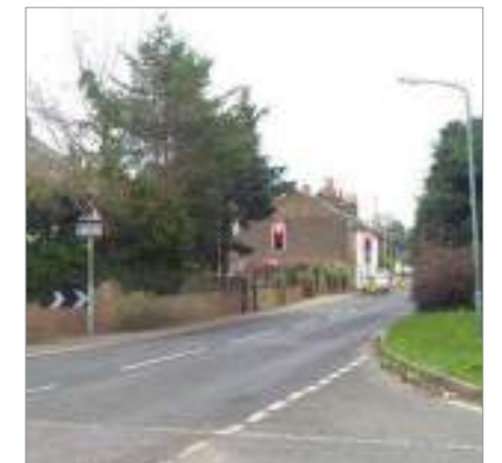
Photo 10 View of traffic lights in Lower Rainham Road B2004
