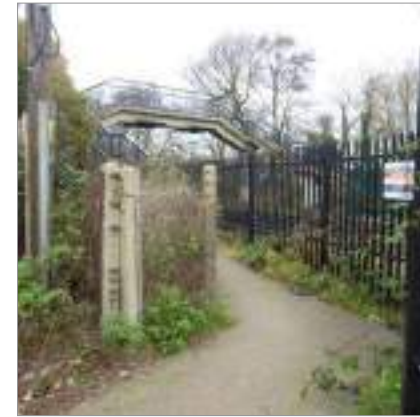
Photo 7 View of footbridge over railway at Bloor's Lane
