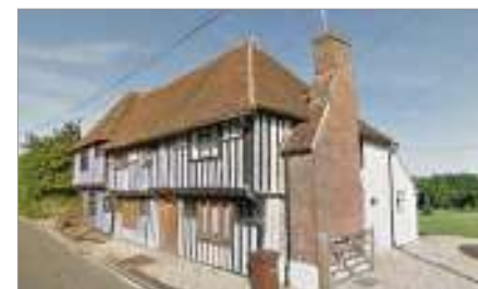
Photo 23 - Chapel House timber framed with red clay roof tiles and chimney
