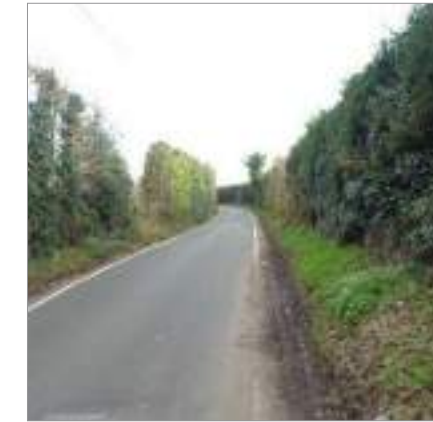
Photo 1 - View north along Pump Lane
