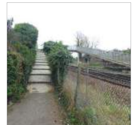
Photo 12 View of footbridge over railway at Lower Tydall Lane
