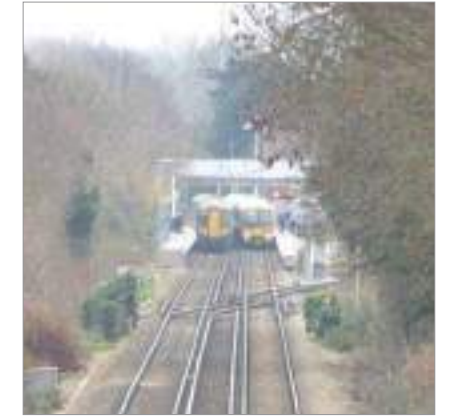
Photo 8 Rainham Station from Bloor's Lane footbridge
