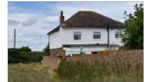
Photo 21 - white timber boarding on red brick with red clay roof tiles on Pump Lane
