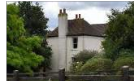
Photo 20 - light coloured render on Pump Farmhouse with red clay roof tiles and chimney
