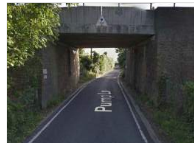
Photo 17 - Pump Lane road bridge under the railway as it exists
