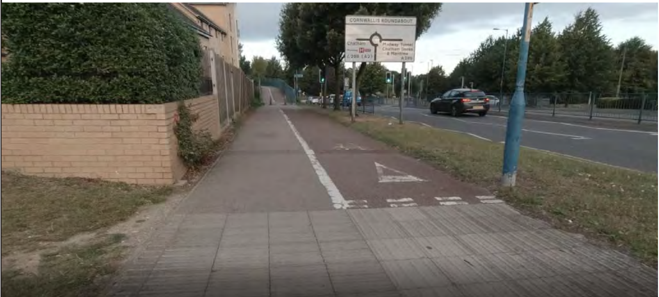
Image 2 – Segregated Footway/Cycleway at Cornwallis Roundabout
