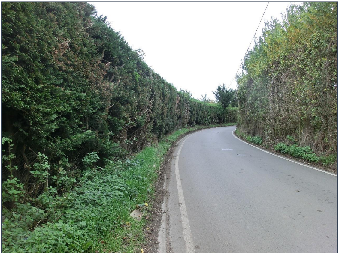
Fig 10. Pump Lane, looking back towards railway bridge from a point approximately 140m north of the railway
