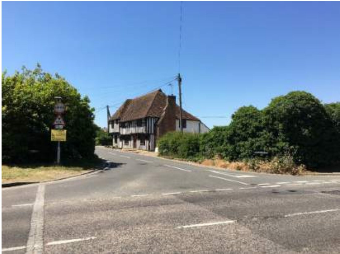
Plate 18 Chapel House, view south-west
