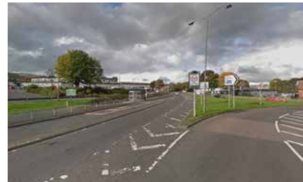
03 West view Bank Street
