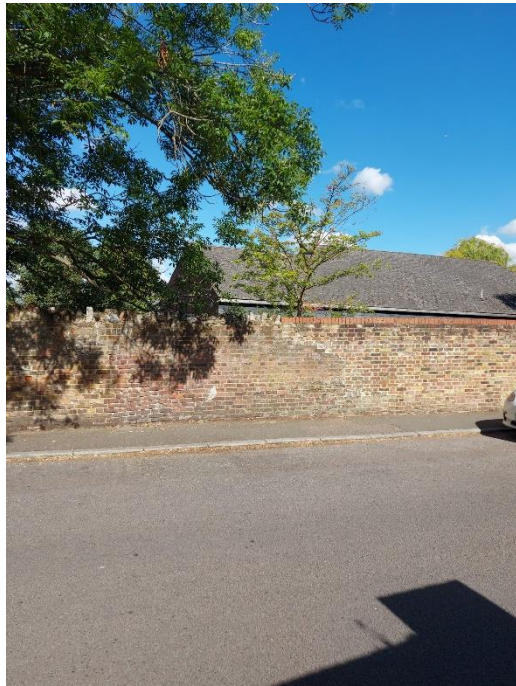
Figure 4: photograph from the footpath on South side of Crown Street
