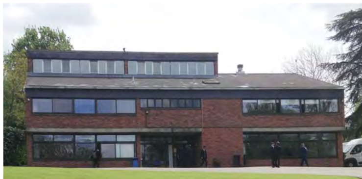
Figure 8 – Oldfield House, north-facing elevation
