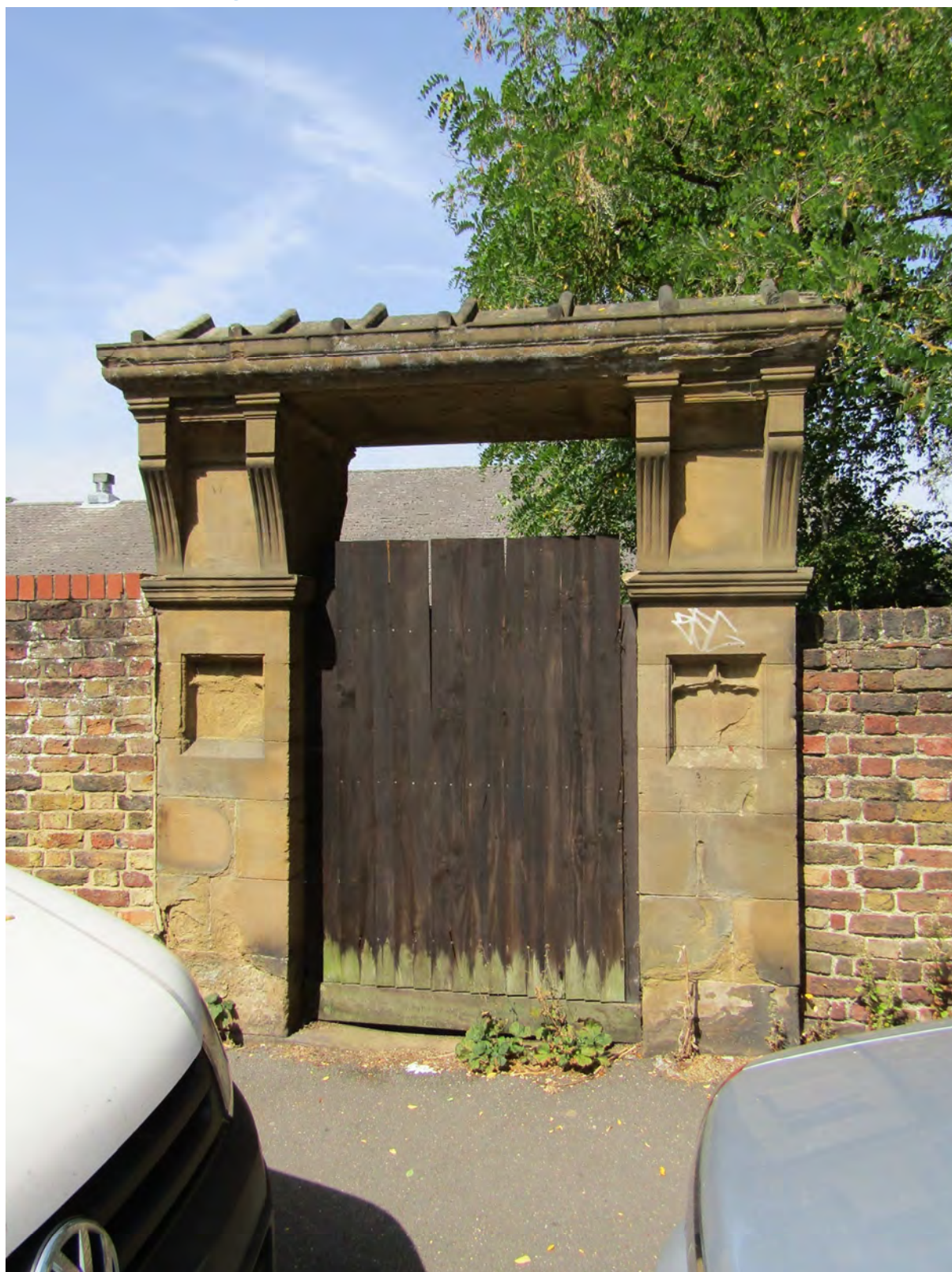
Figure 3 - established brick boundary wall and decorative stone piers
