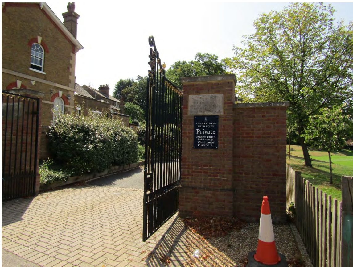
Figure 13 - modern gates piers to entrance of Field House and the rear of the former Police Station
