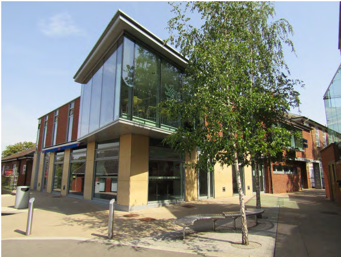
Figure 22 - contemporary architecture with a simple palate that reflects the materials on site
