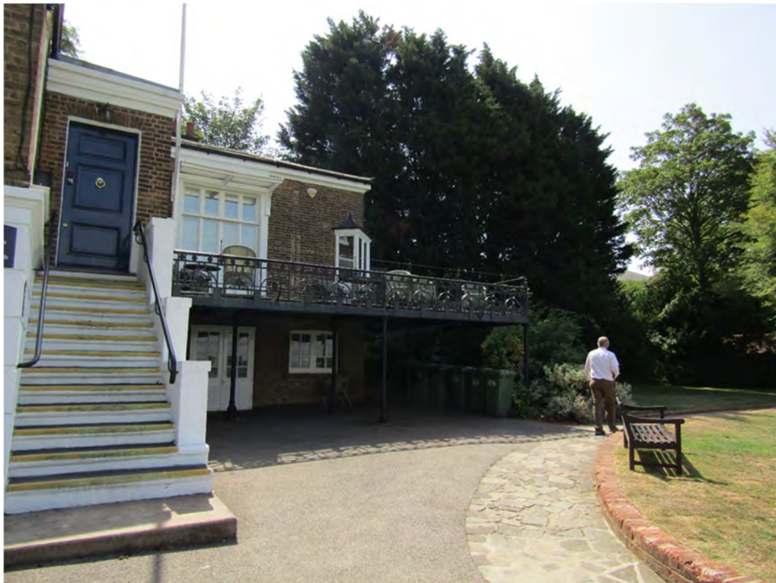
Figure 15 - view from Field House looking up towards site
