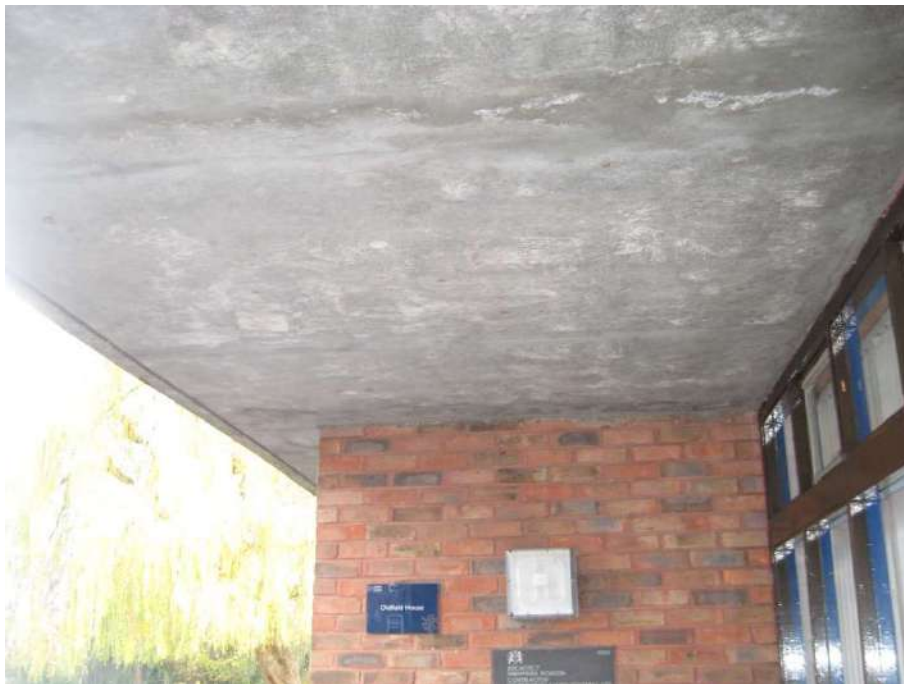
Tight sealed concrete undercroft at building entrance
