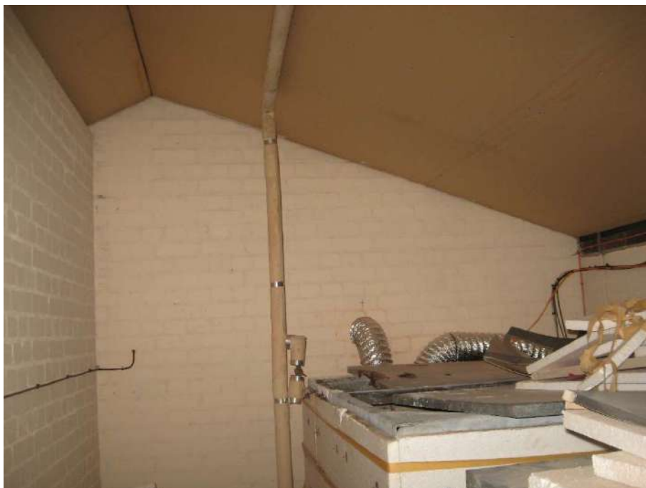
Roof void in south west of the building. Sealed and no evidence of bats
