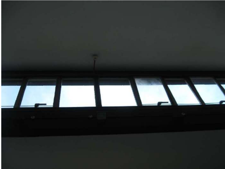
Glazed lobby interior – second floor
