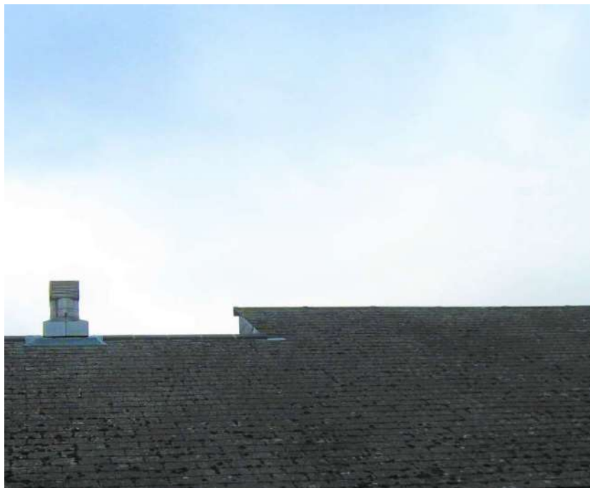
Tightly sealed, intact tiles on roof
