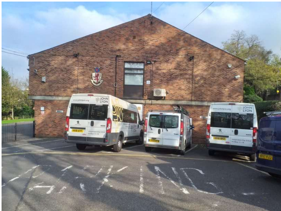
South western elevation of Oldfield House
