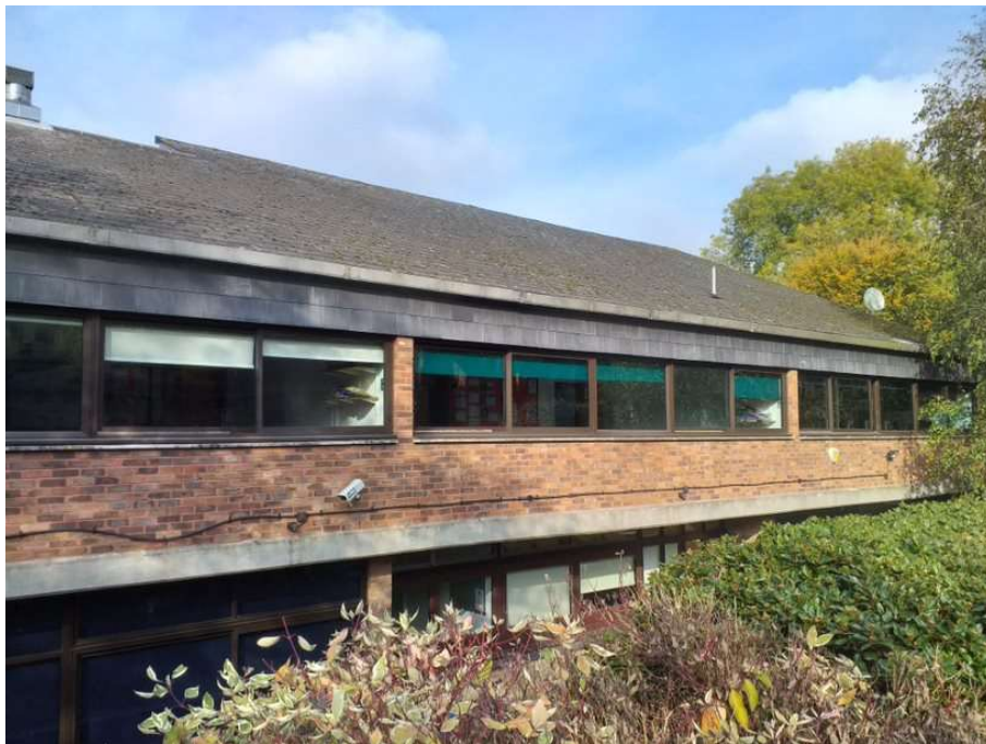
Tightly sealed, intact tiles on roof
