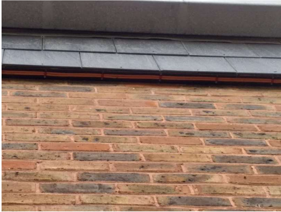
Soffit, gutter and tiles forming a tight, intact seal around the building
