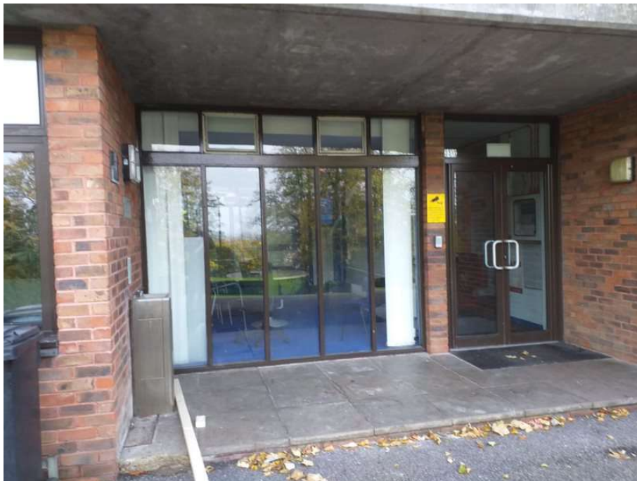
Tight sealed concrete undercroft at building entrance
