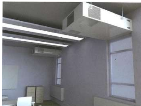
Figure 5 – NVHR 1100 units exposed in a classroom
