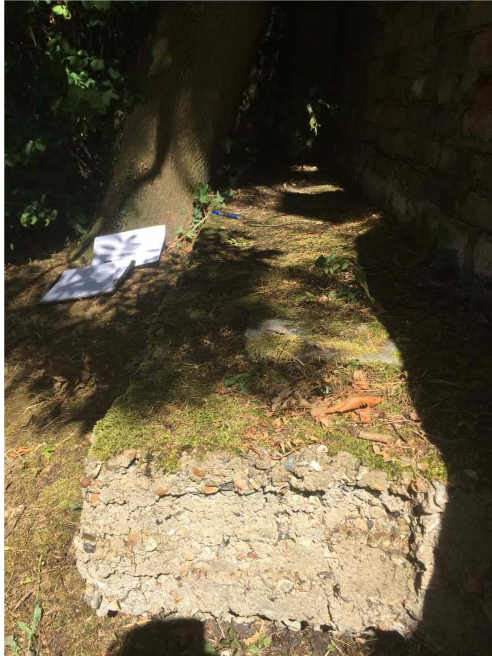
Photo No. 2 to show root-collar buttresses close to base of the boundary wall (pen included for scale)
