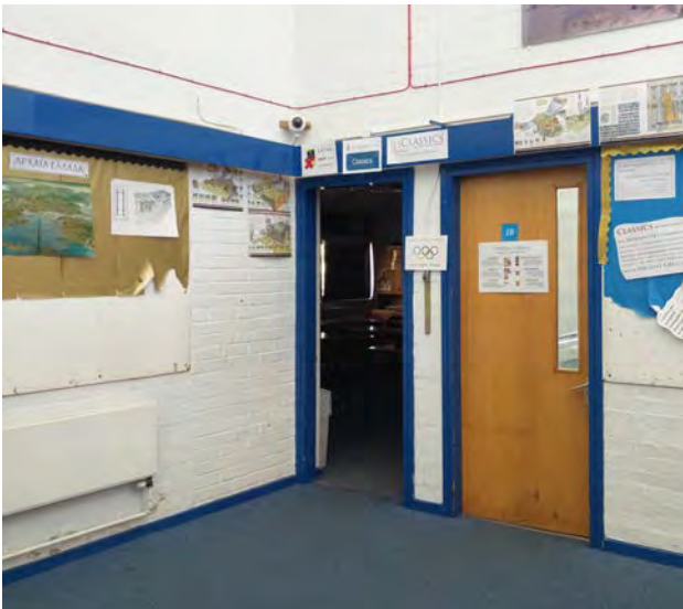
Existing Doors are not Fire Regulations compliant
