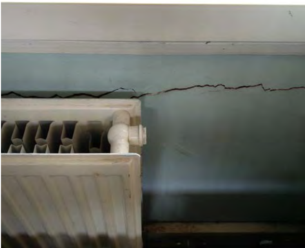
Cracked existing wall does not take the load of radiators.
