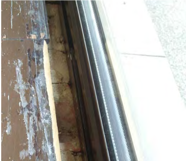
Brick upstand exposed, causing a cold bridge.
