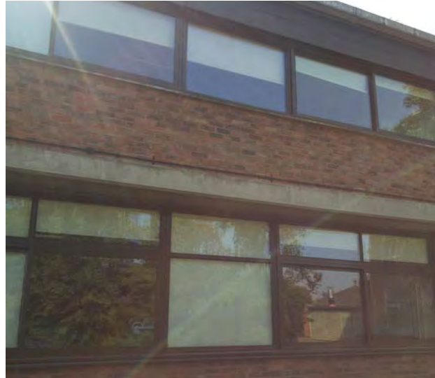
Close up view of the bowing concrete slab to Oldfield House
