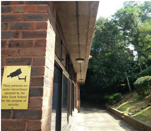
Exposed Concrete Slab with cold bridge
