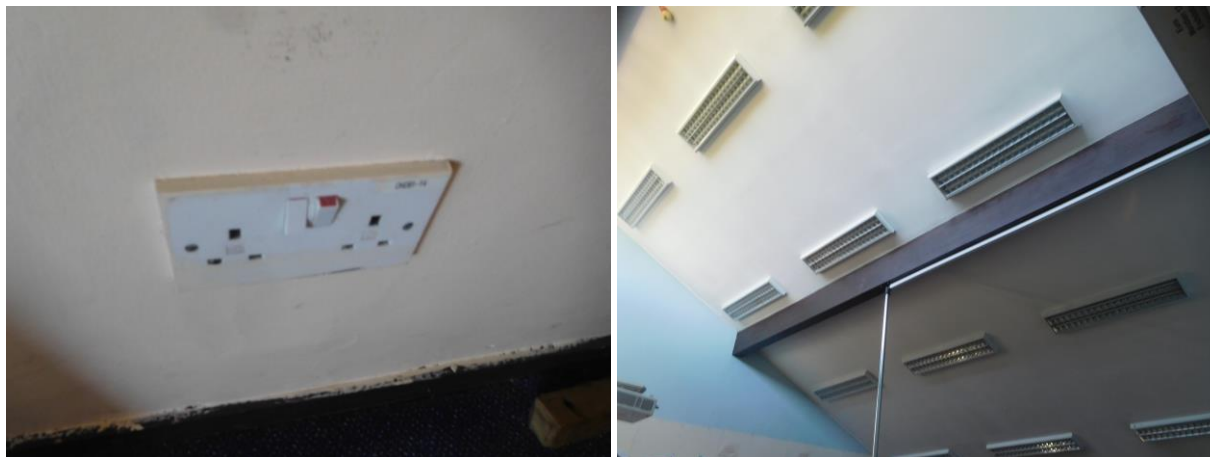
Photos show one of the sockets typical of those located throughout the building and a bank of T12 lighting units to one of the classrooms.
