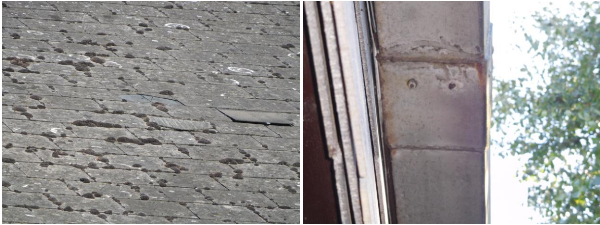
Photos show broken and loose slates to the Rear Elevation and typical deterioration of one of the joints to the steel gutters.
