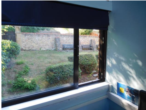
Photo shows one of the original sliding aluminium double glazed windows in its fully open position.
