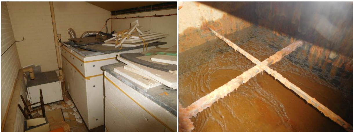
Photos show the 3No water tanks and the inside of one of the cold water storage tanks.
