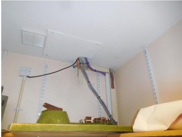
Photo shows unsecure cabling going through the ceiling within the First Floor Office.
