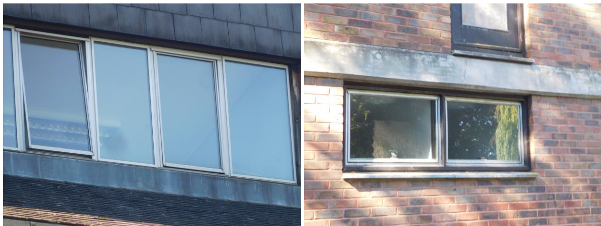
Photos show a section of the North lights to the roof and two of the timber framed windows with aluminium inserts.
