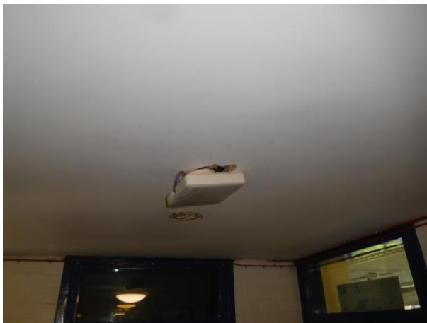
Photo shows a wireless router falling away from the plaster ceiling where its fixings have failed.
