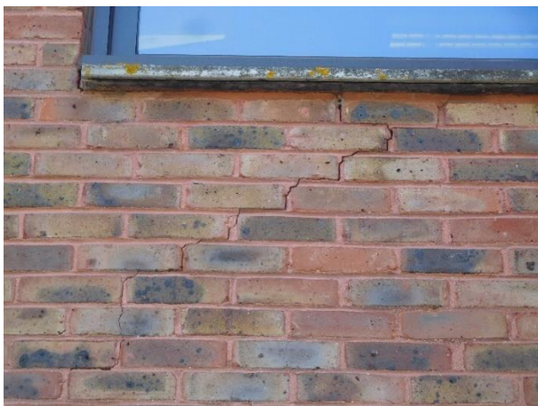
Photo showing the largest crack, located to the RHS of the Front Elevation.
