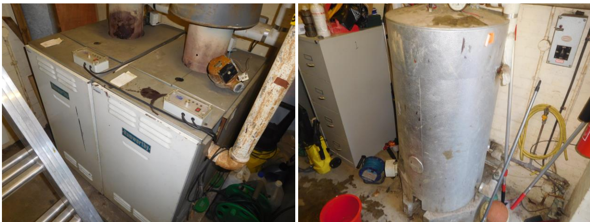
Photos show 2No Hamworthy boilers and the calorifier situated to the main Plant Room.
