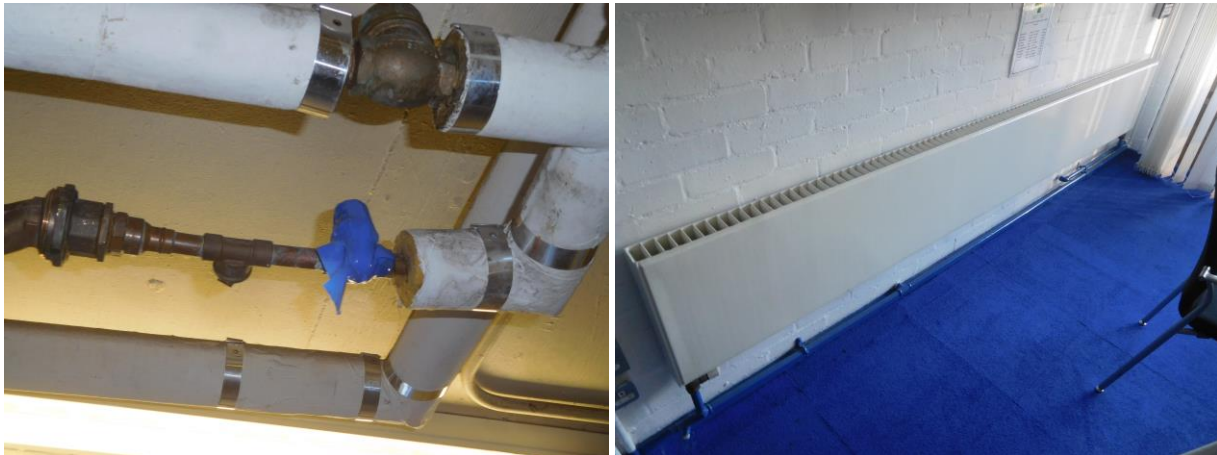
Photos show section of leaking hot water pipework to Plant Room and one of the original radiators found throughout the block.
