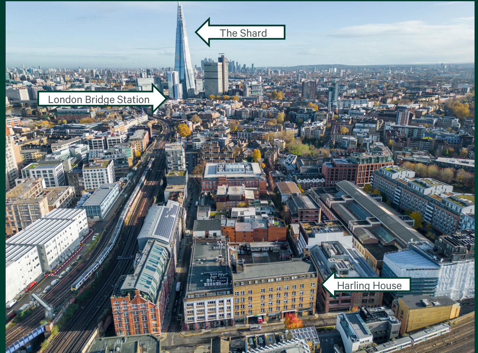
Aerial View of Yard to the East
