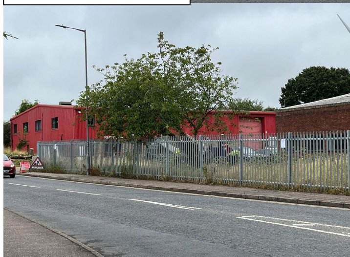
Site before demolition
