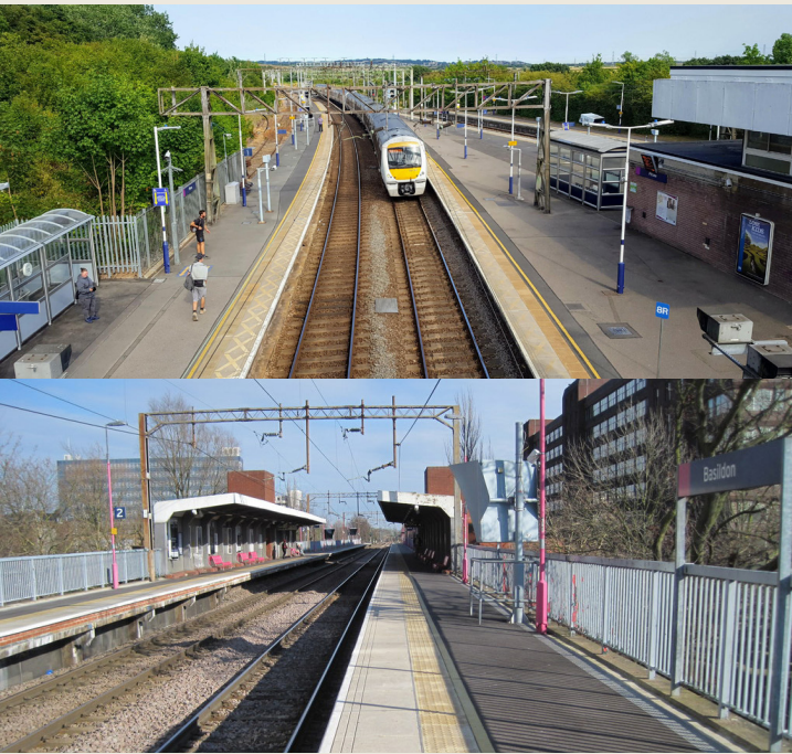
Pitsea & Basildon railway station Key commuter transport link for services towards London and South Essex.
